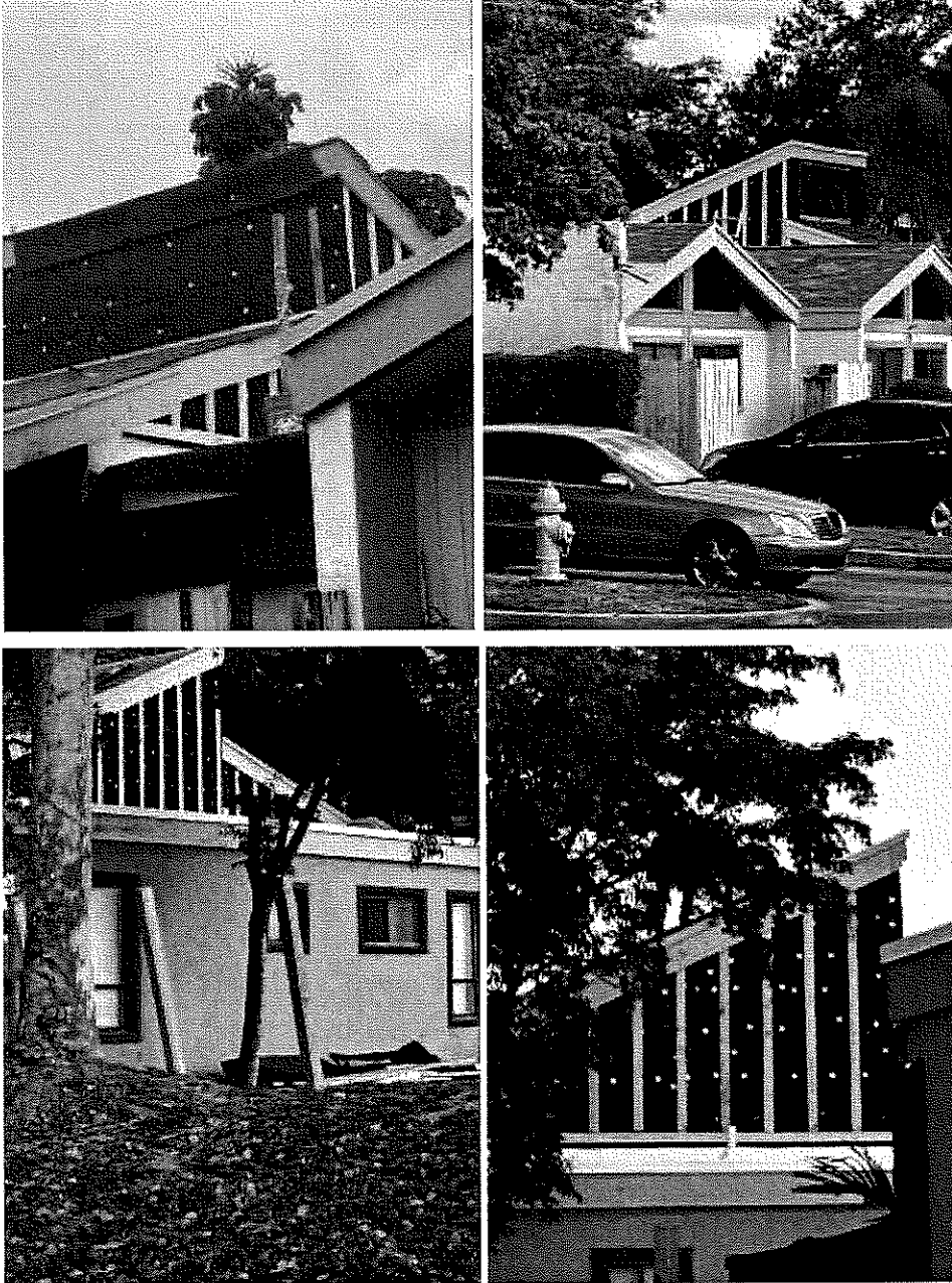
Figure 3: Furring Strips Installed On My Home, Other Phase 2 & Phase 1 Buildings
