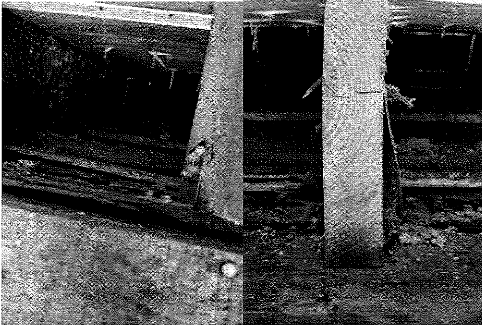
Figure 2: May 2 nd , 2025 - Images Of Missing Roof Insulation On Whistleblower's Unit
