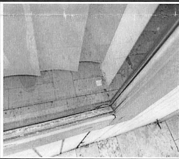
Photo 3 : Existing non-impact-rated window frame
