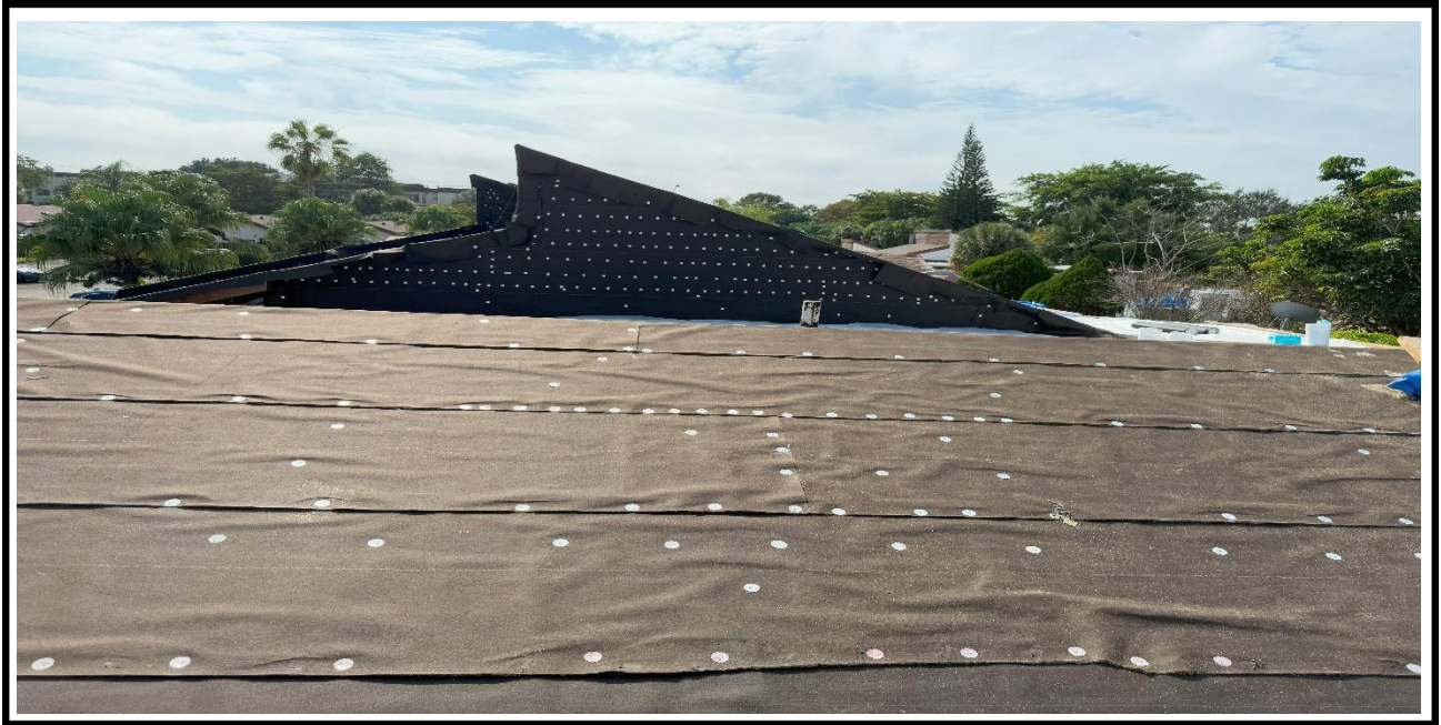
6 – Ongoing, Ongoing, Laying down the waterproofing Sheets and tin caps, BLDG 14.
