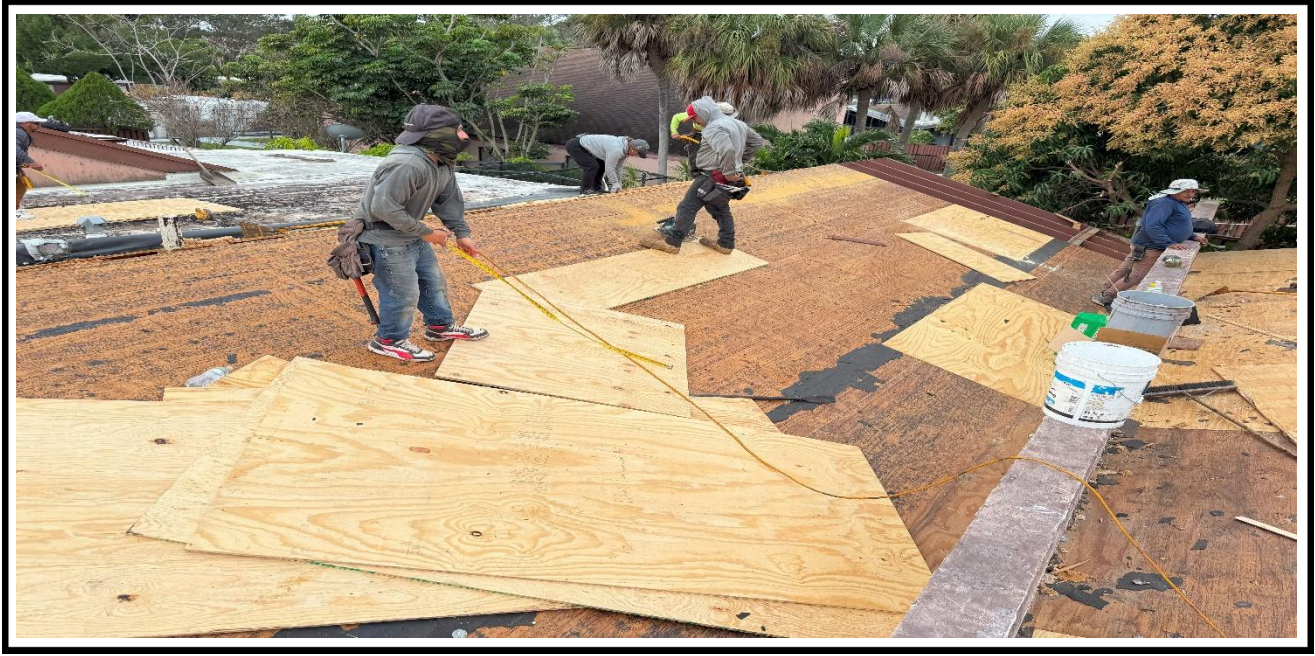
1 – Ongoing, Replacement of the deteriorated plywood on top of the roof, BLDG 14.
