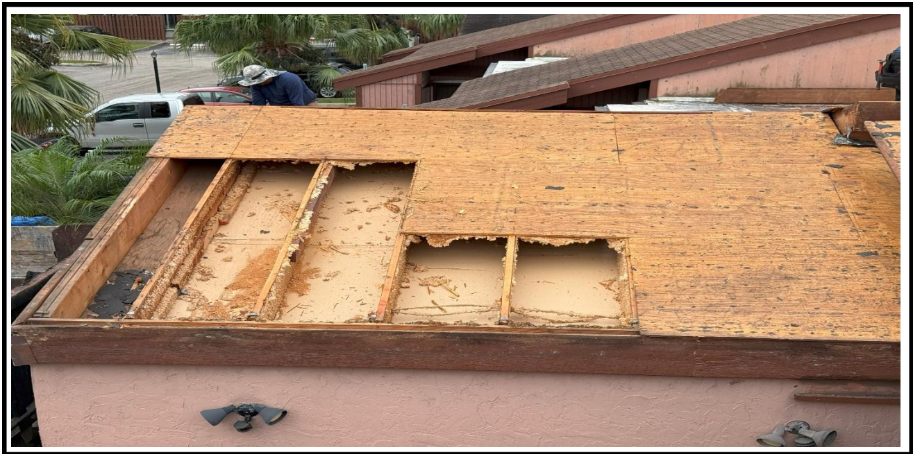
2 – Ongoing, Replacement of the deteriorated plywood on top of the roof, BLDG 14.
