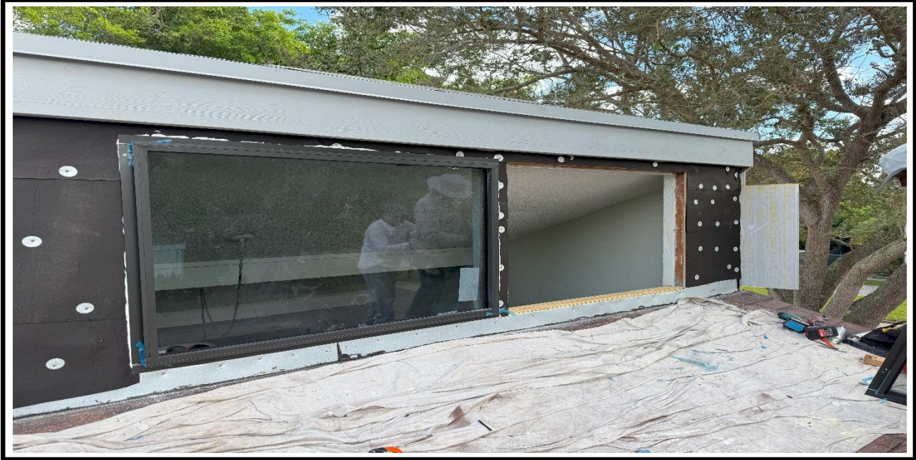
12 – Ongoing, Installation of the new top windows.
