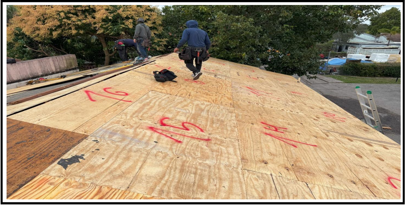
3 – Ongoing, Replacement of the deteriorated plywood on top of the roof, BLDG 14.
