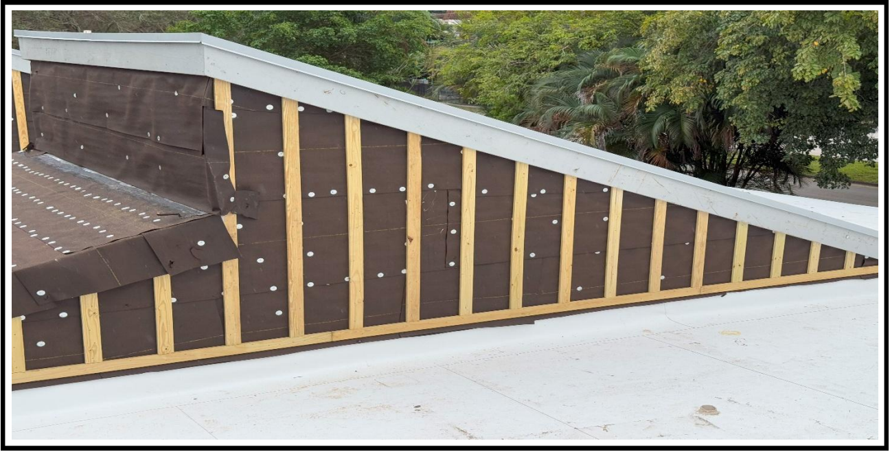
9 – Ongoing, Installation of the fascia board / drip edges / siding wood strips, BLDG 07.
