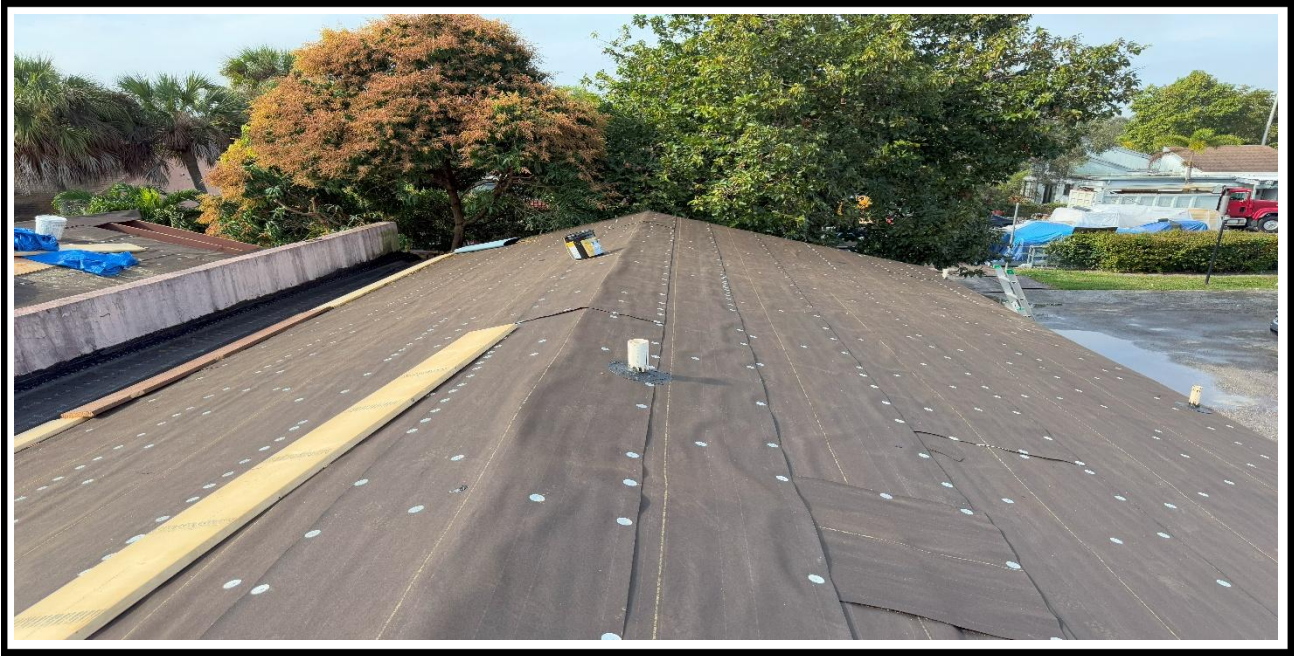
5 – Ongoing, Ongoing, Laying down the waterproofing Sheets and tin caps, BLDG 14.
