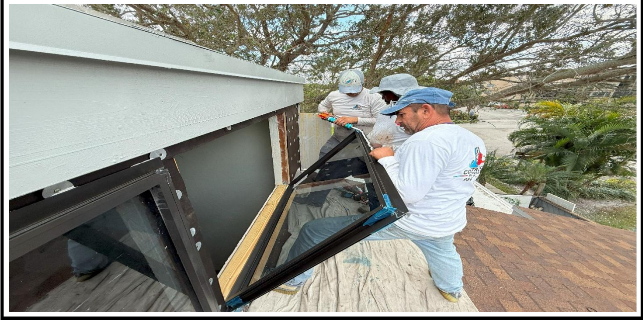
11 – Ongoing, Installation of the new top windows.
