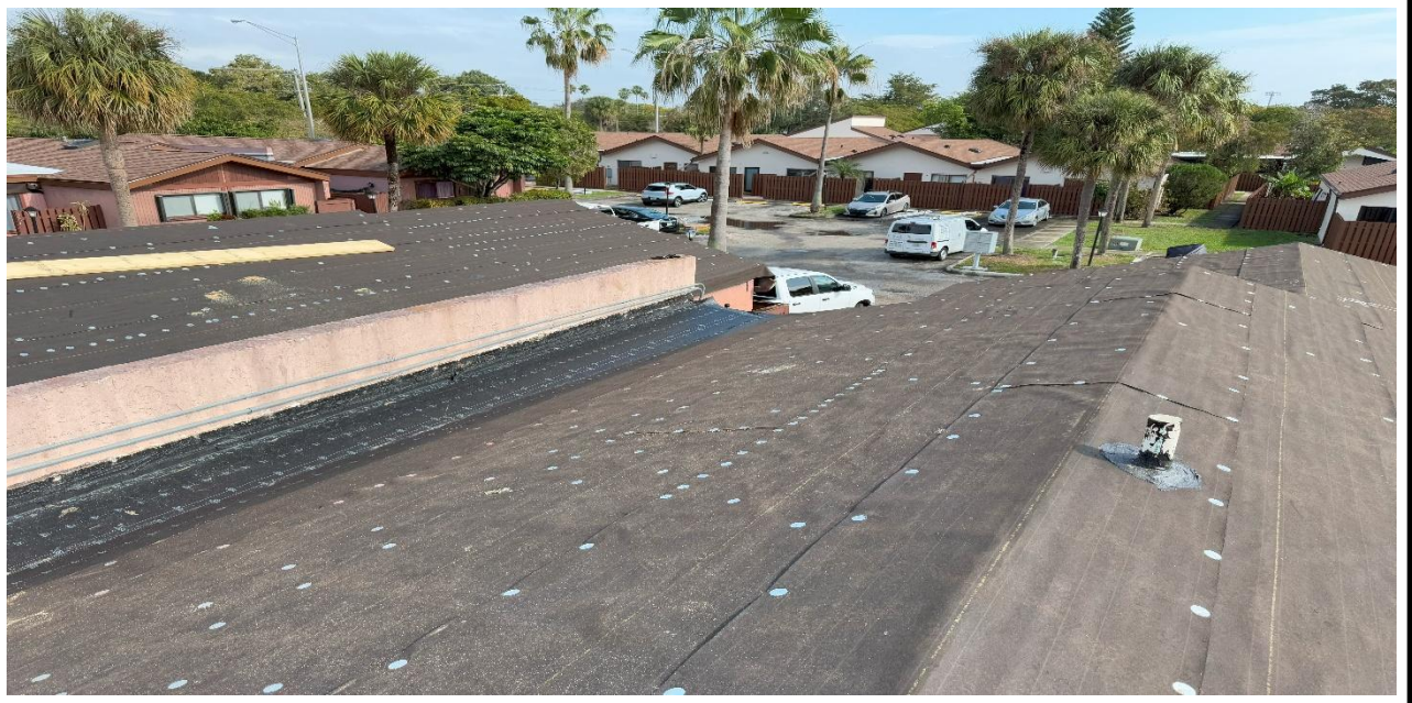
7 – Ongoing, Ongoing, Laying down the waterproofing Sheets and tin caps, BLDG 14.
