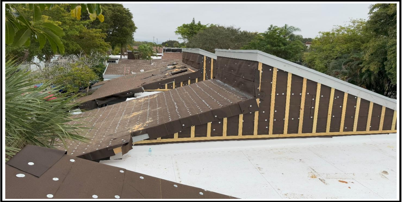
10 – Ongoing, Installation of the fascia board / drip edges / siding wood strips, BLDG 07.
