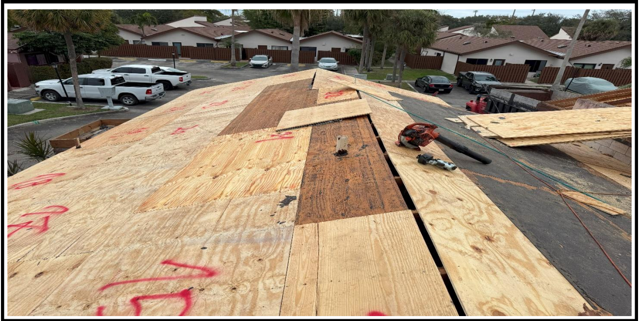
4 – Ongoing, Replacement of the deteriorated plywood on top of the roof, BLDG 14.
