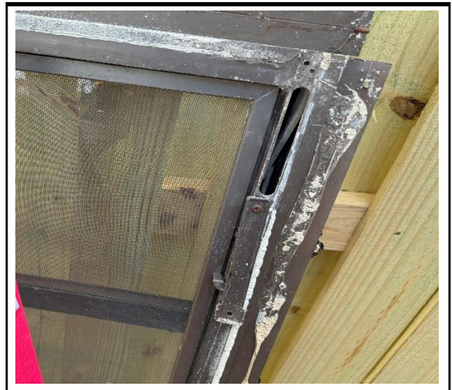
Photo 4 : Loose Components
