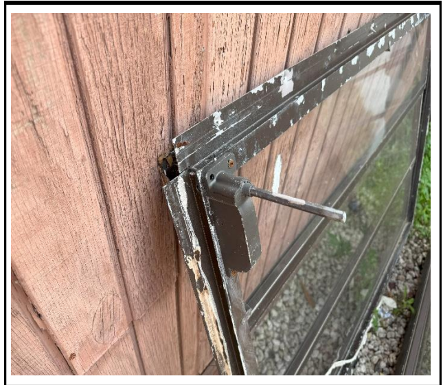
Photo 2 : Broken Latch
