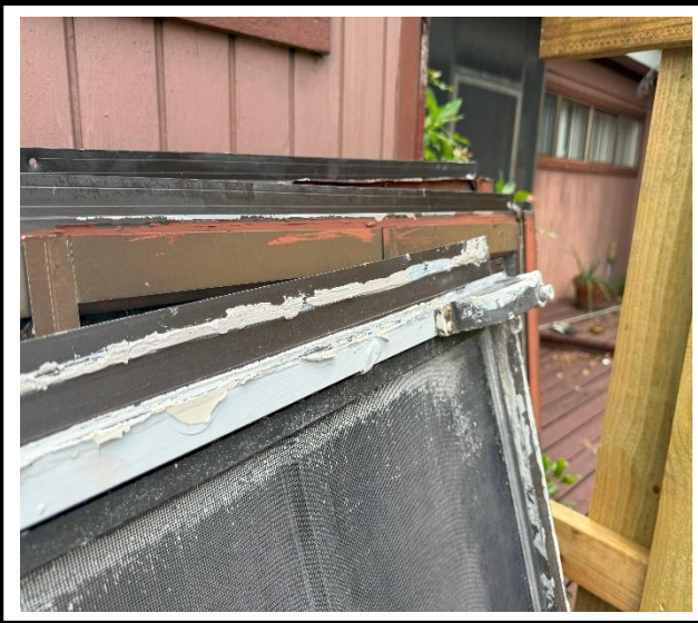
Photo 1 : Broken Latch
