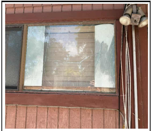
Photo 4 : Existing non-impact-rated window frame
