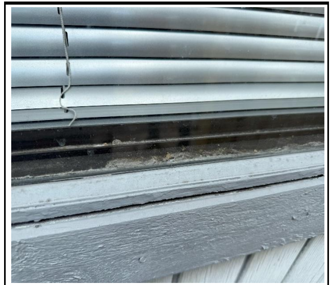
Photo 4 : Existing non-impact-rated window frame
