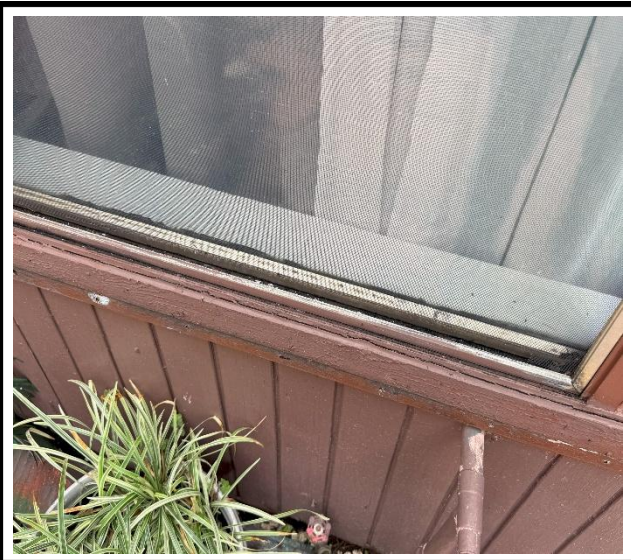
Photo 3 : Existing non-impact-rated window frame
