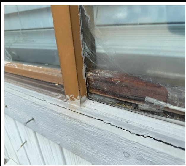
Photo 3 : Existing non-impact-rated window frame
