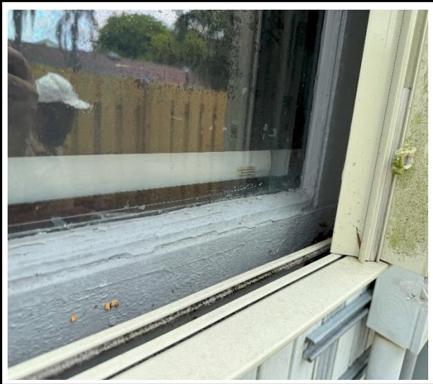
Photo 3 : Existing non-impact-rated window frame
