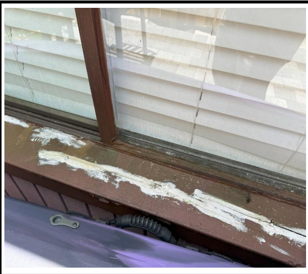
Photo 3 : Existing non-impact-rated window frame
