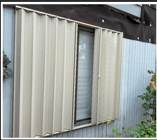
Photo 1 : Existing non-impact-rated window frame
