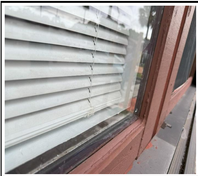
Photo 4 : Existing non-impact-rated window frame
