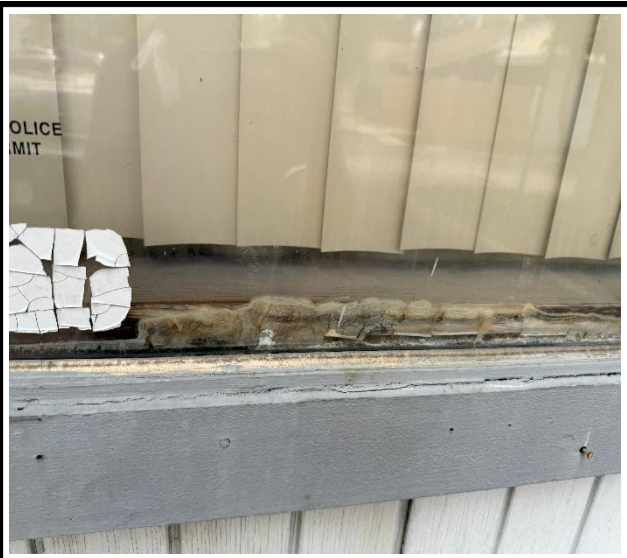
Photo 3 : Existing non-impact-rated window frame
