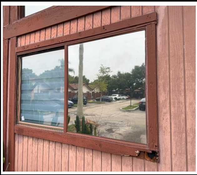
Photo 1 : Existing non-impact-rated window frame
