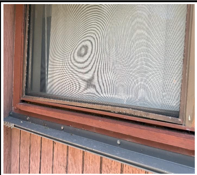
Photo 3 : Existing non-impact-rated window frame
