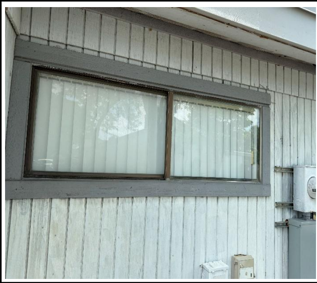
Photo 1 : Existing non-impact-rated window frame
