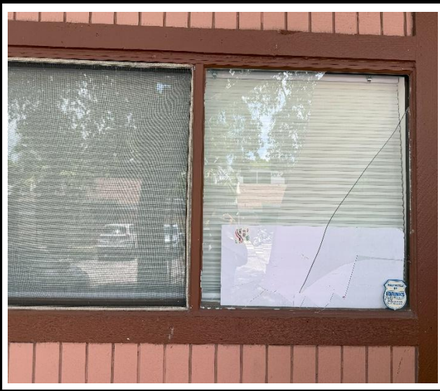
Photo 1 : Existing non-impact-rated window frame
