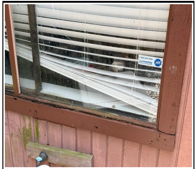
Photo 2 : Existing non-impact-rated window frame
