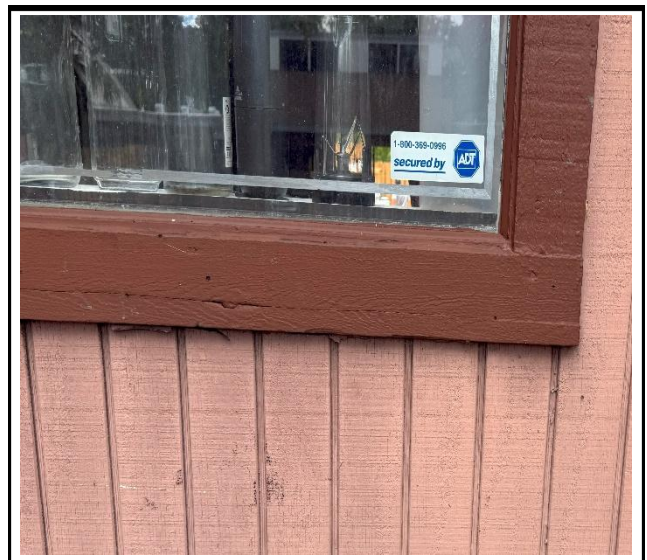
Photo 4 : Existing non-impact-rated window frame
