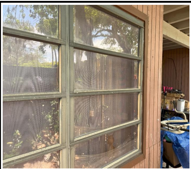
Photo 3 : Existing non-impact-rated window frame
