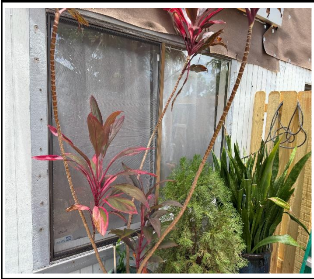
Photo 1 : Existing non-impact-rated window frame
