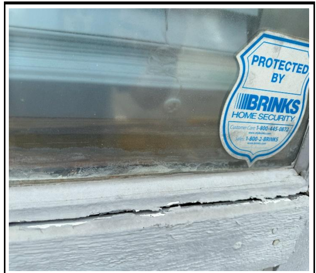
Photo 4 : Existing non-impact-rated window frame
