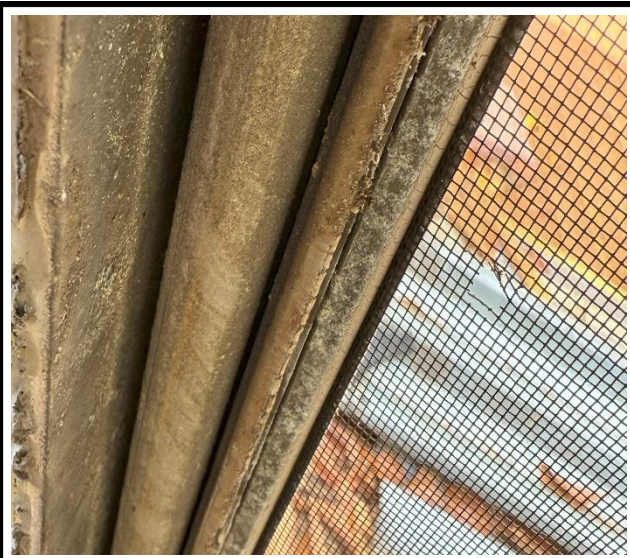
Photo 3 : Existing non-impact-rated window frame
