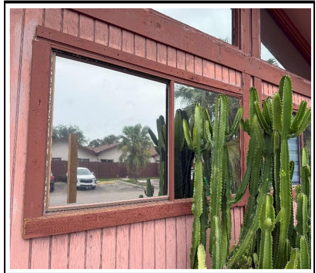
Photo 2 : Existing non-impact-rated window frame
