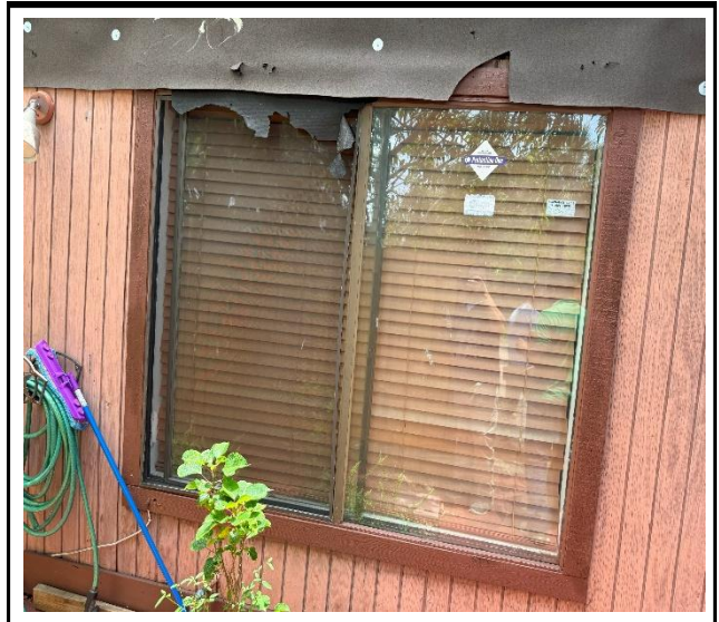
Photo 2 : Existing non-impact-rated window frame
