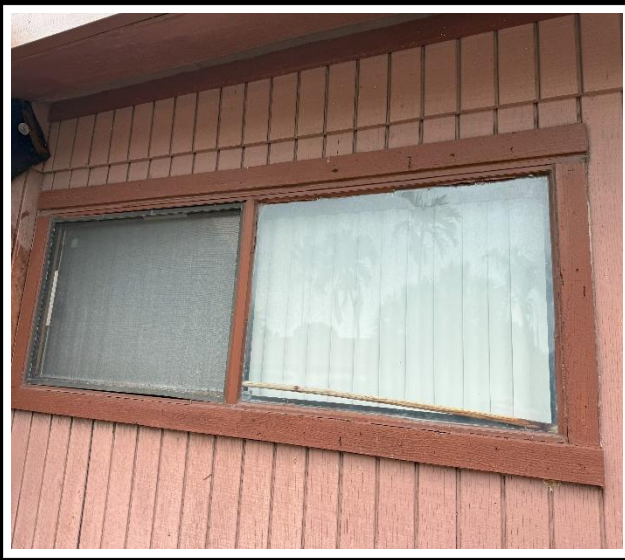
Photo 1 : Existing non-impact-rated window frame
