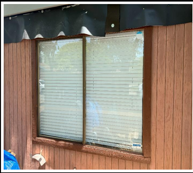
Photo 1 : Existing non-impact-rated window frame
