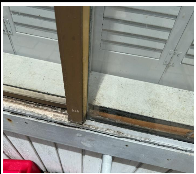
Photo 3 : Existing non-impact-rated window frame
