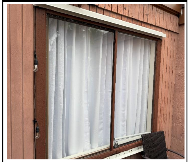
Photo 2 : Existing non-impact-rated window frame
