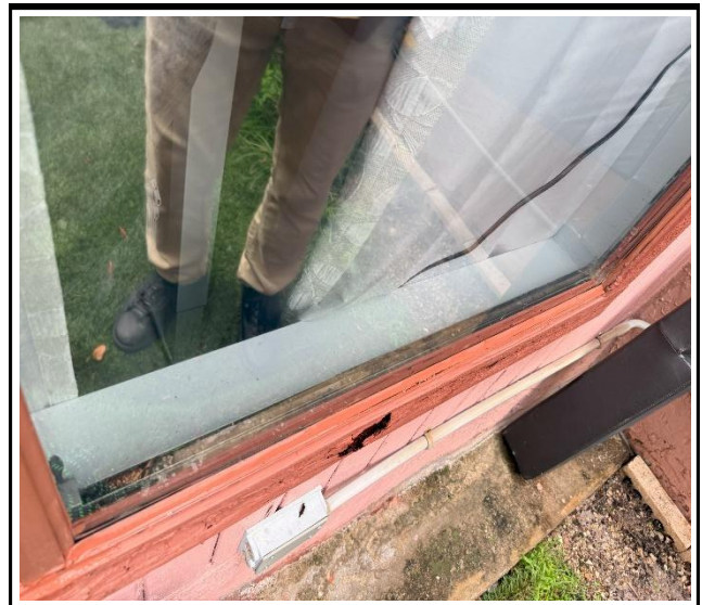
Photo 4 : Existing non-impact-rated window frame
