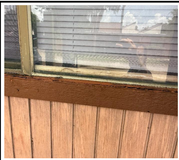
Photo 3 : Existing non-impact-rated window frame
