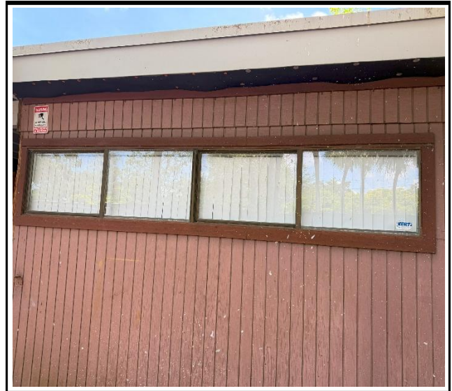
Photo 2 : Existing non-impact-rated window frame
