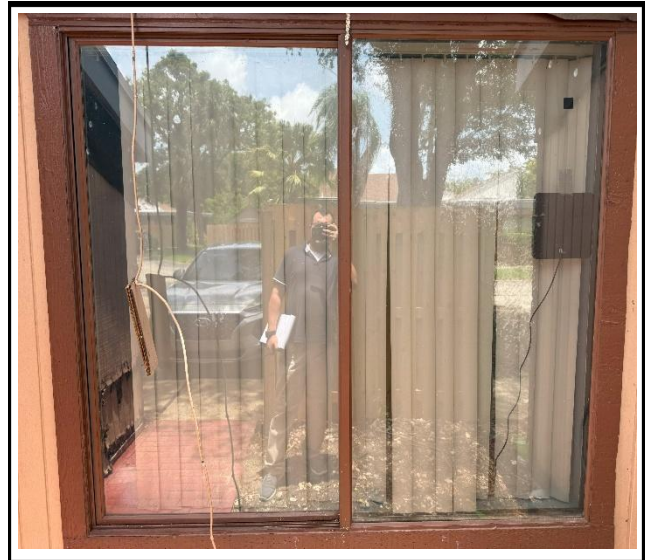
Photo 2 : Existing non-impact-rated window frame
