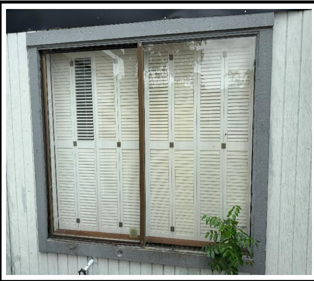
Photo 1 : Existing non-impact-rated window frame
