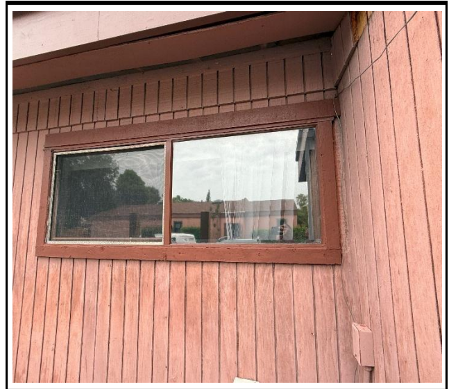
Photo 2 : Existing non-impact-rated window frame
