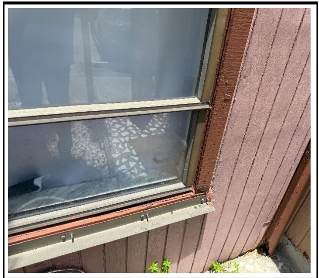
Photo 2 : Existing non-impact-rated window frame
