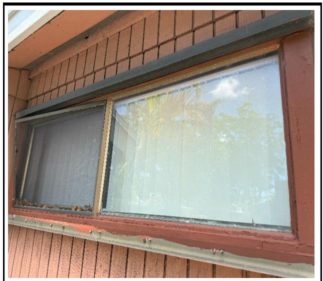
Photo 4 : Existing non-impact-rated window frame
