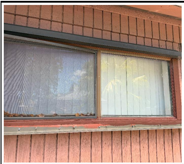
Photo 3 : Existing non-impact-rated window frame
