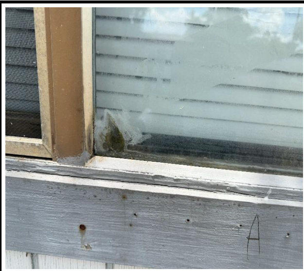
Photo 3 : Existing non-impact-rated window frame
