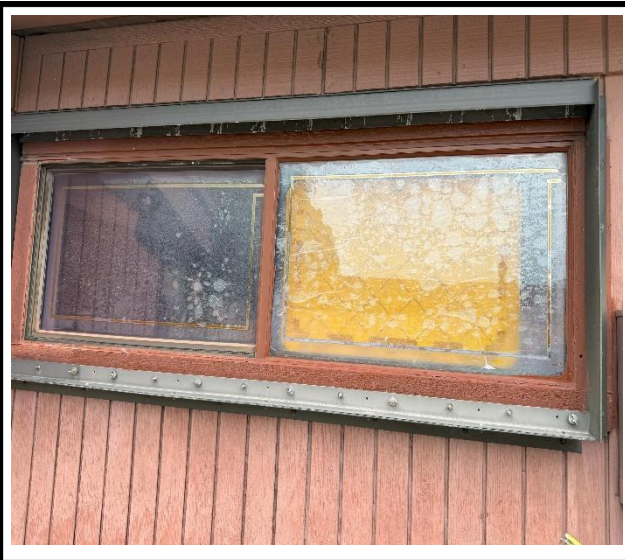
Photo 3 : Existing non-impact-rated window frame
