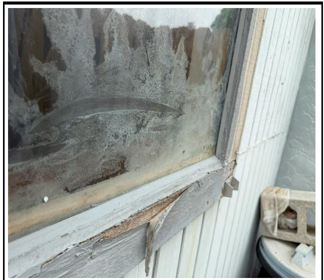
Photo 4 : Existing non-impact-rated window frame
