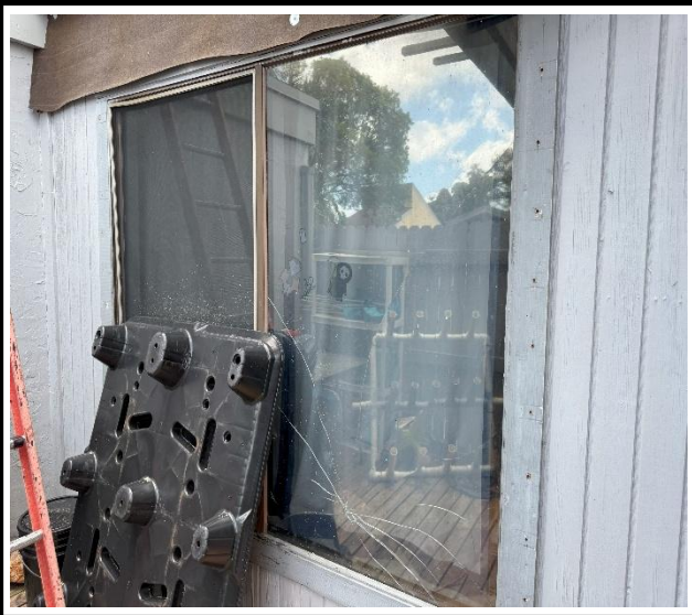
Photo 1 : Existing non-impact-rated window frame
