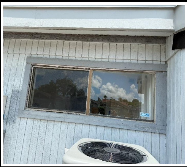
Photo 1 : Existing non-impact-rated window frame
