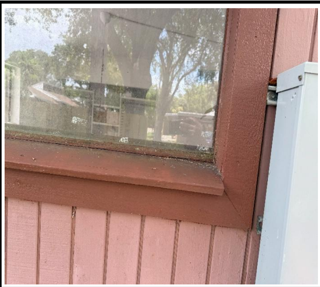
Photo 3 : Existing non-impact-rated window frame
