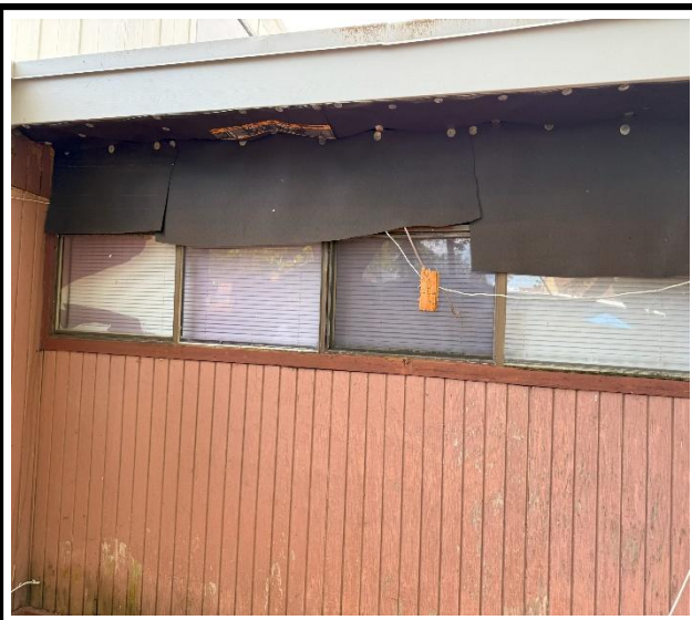
Photo 3 : Existing non-impact-rated window frame
