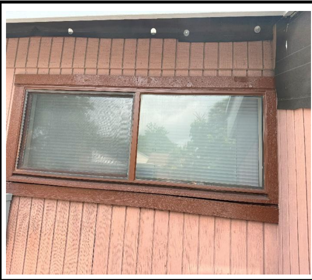
Photo 1 : Existing non-impact-rated window frame
