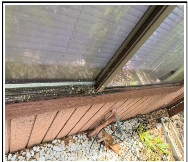
Photo 4 : Existing non-impact-rated window frame
