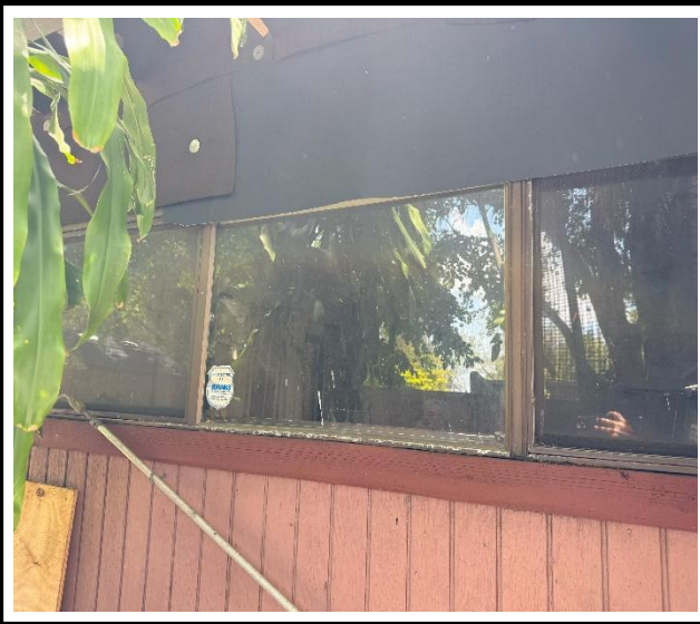
Photo 1 : Existing non-impact-rated window frame
