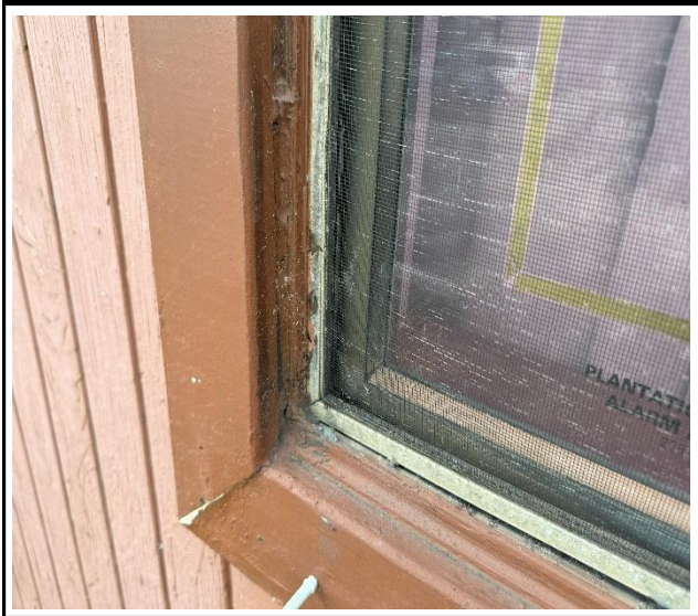
Photo 3 : Existing non-impact-rated window frame
