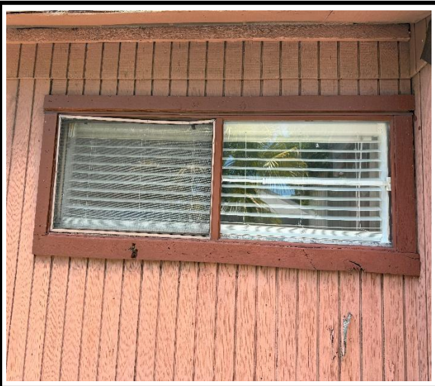
Photo 1 : Existing non-impact-rated window frame
