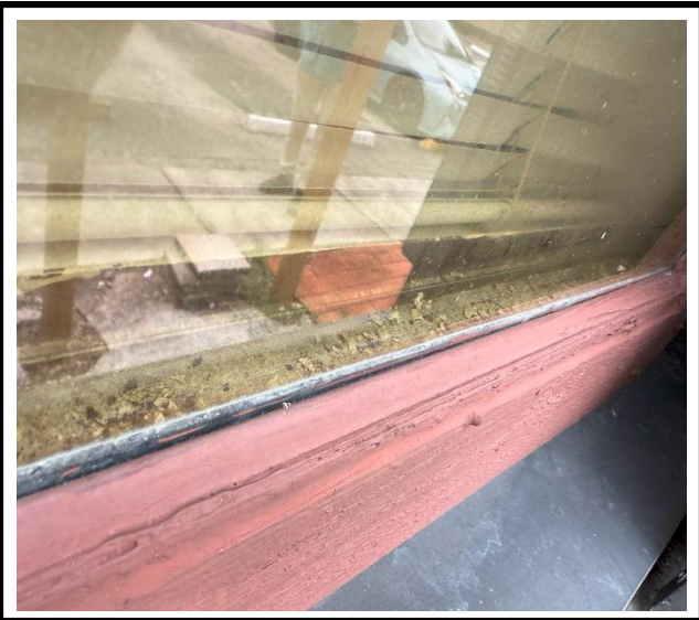
Photo 3 : Existing non-impact-rated window frame
