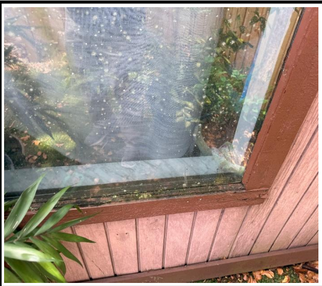
Photo 3 : Existing non-impact-rated window frame
