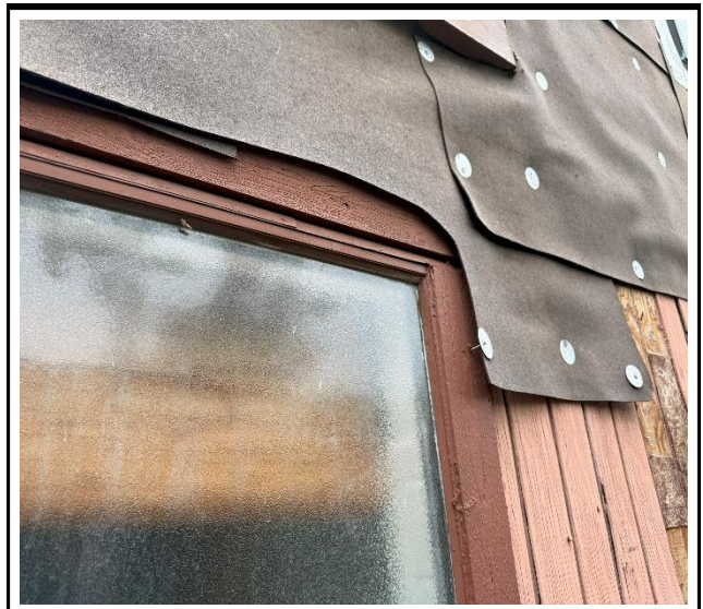
Photo 4 : Existing non-impact-rated window frame
