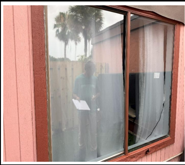
Photo 1 : Existing non-impact-rated window frame
