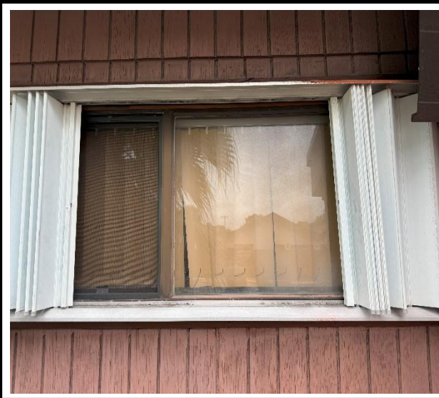
Photo 3 : Existing non-impact-rated window frame
