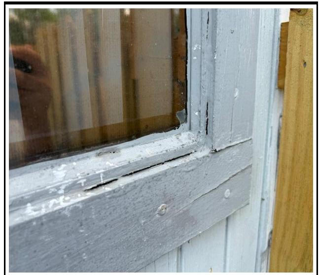
Photo 4 : Existing non-impact-rated window frame
