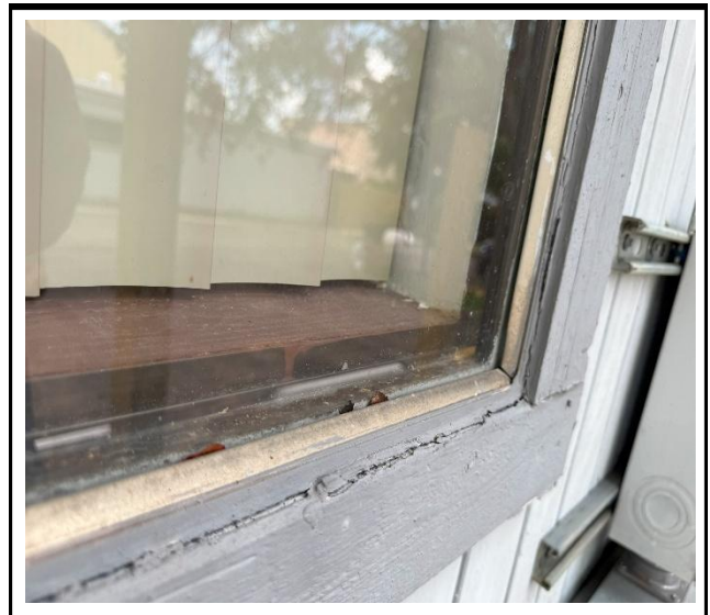
Photo 4 : Existing non-impact-rated window frame
