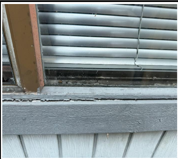
Photo 3 : Existing non-impact-rated window frame
