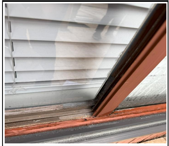
Photo 2 : Existing non-impact-rated window frame
