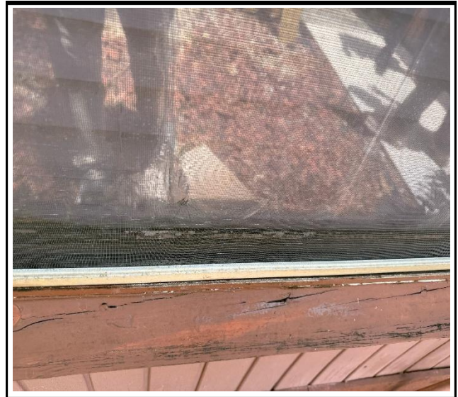
Photo 2 : Existing non-impact-rated window frame
