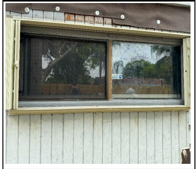
Photo 2 : Existing non-impact-rated window frame
