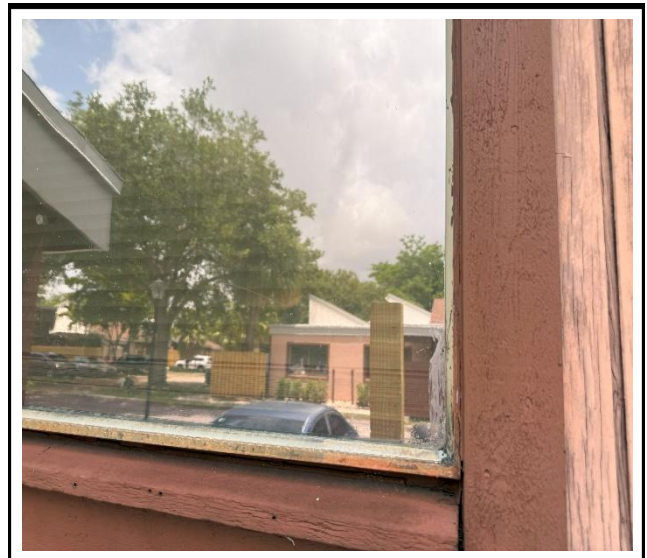
Photo 4 : Existing non-impact-rated window frame
