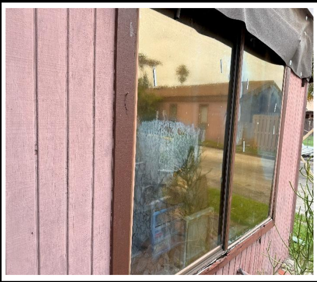
Photo 1 : Existing non-impact-rated window frame
