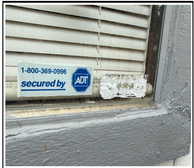
Photo 4 : Existing non-impact-rated window frame
