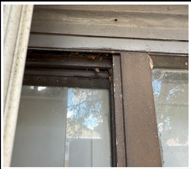
Photo 3 : Existing non-impact-rated window frame
