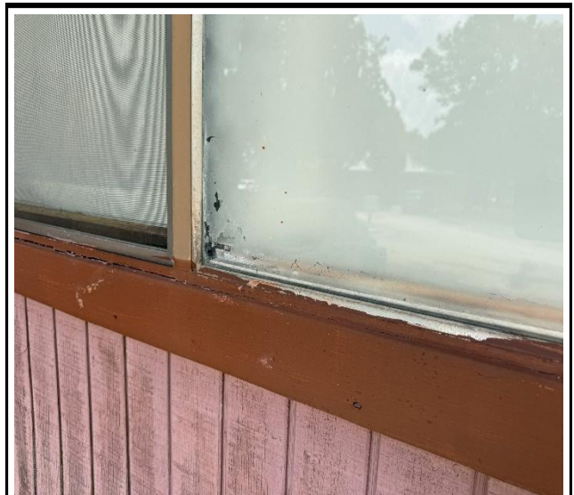
Photo 4 : Existing non-impact-rated window frame
