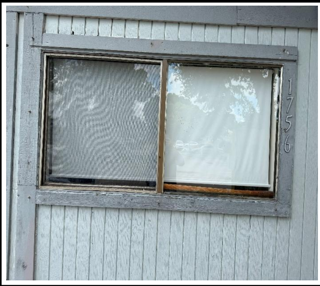
Photo 1 : Existing non-impact-rated window frame
