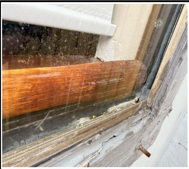
Photo 3 : Existing non-impact-rated window frame
