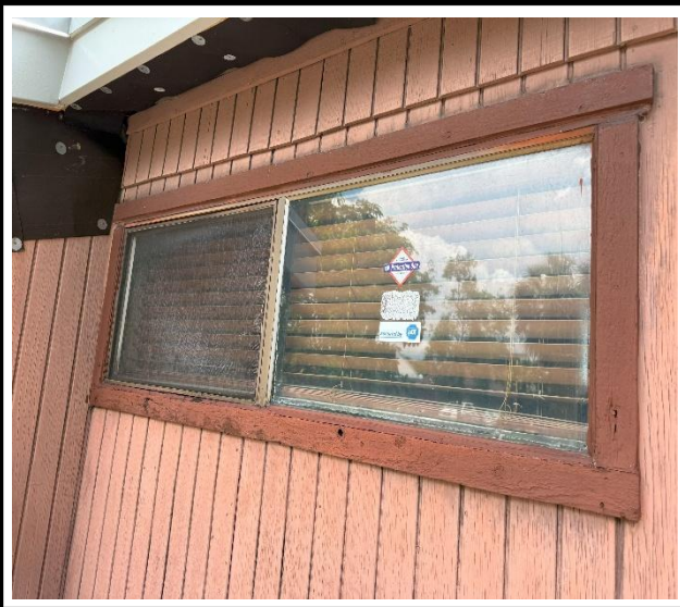
Photo 1 : Existing non-impact-rated window frame
