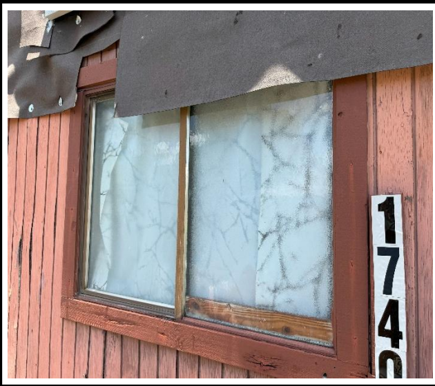
Photo 1 : Existing non-impact-rated window frame
