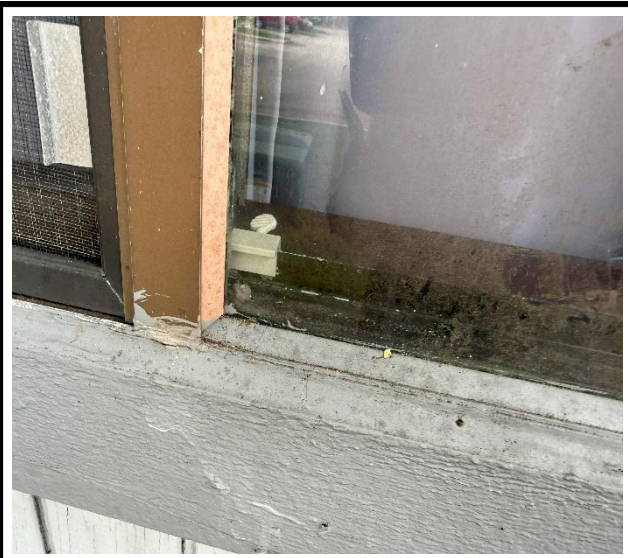
Photo 3 : Existing non-impact-rated window frame
