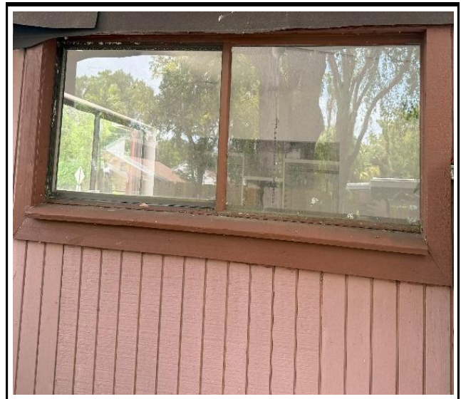
Photo 4 : Existing non-impact-rated window frame
