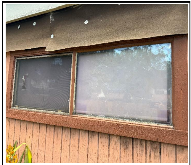
Photo 4 : Existing non-impact-rated window frame
