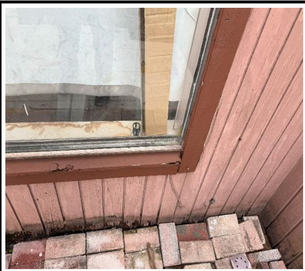
Photo 3 : Existing non-impact-rated window frame
