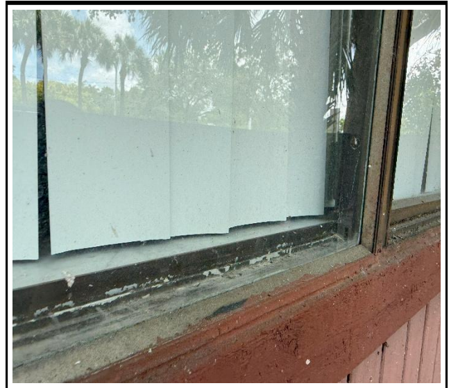
Photo 4 : Existing non-impact-rated window frame
