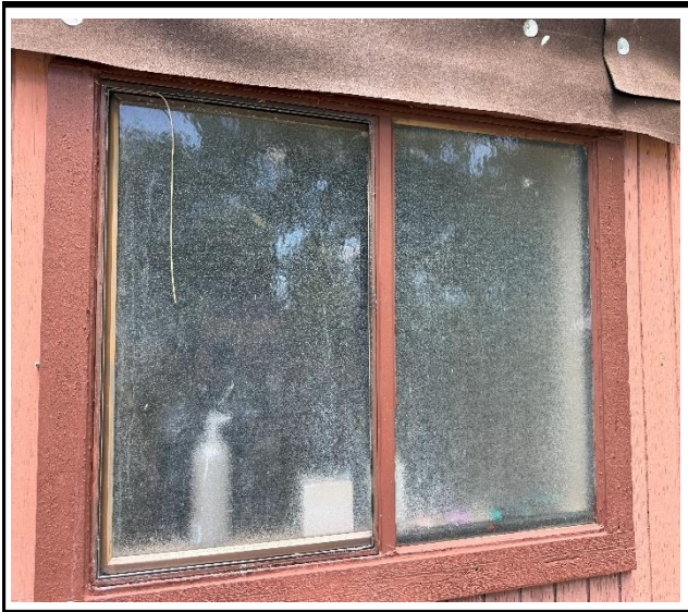
Photo 1 : Existing non-impact-rated window frame
