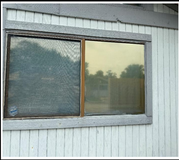
Photo 1 : Existing non-impact-rated window frame
