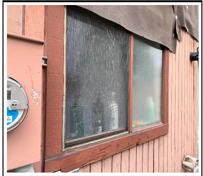
Photo 2 : Existing non-impact-rated window frame
