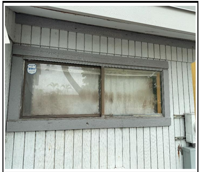
Photo 2 : Existing non-impact-rated window frame
