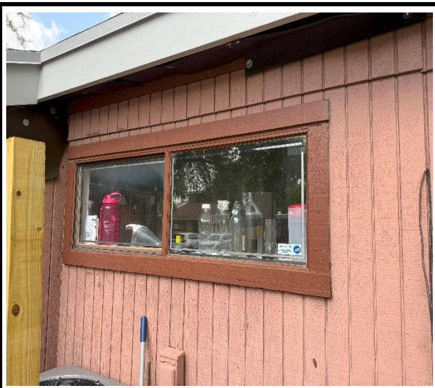
Photo 3 : Existing non-impact-rated window frame
