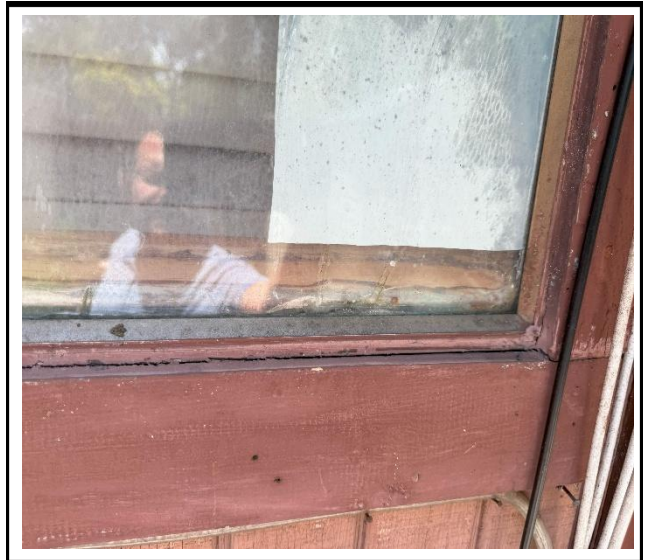
Photo 2 : Existing non-impact-rated window frame
