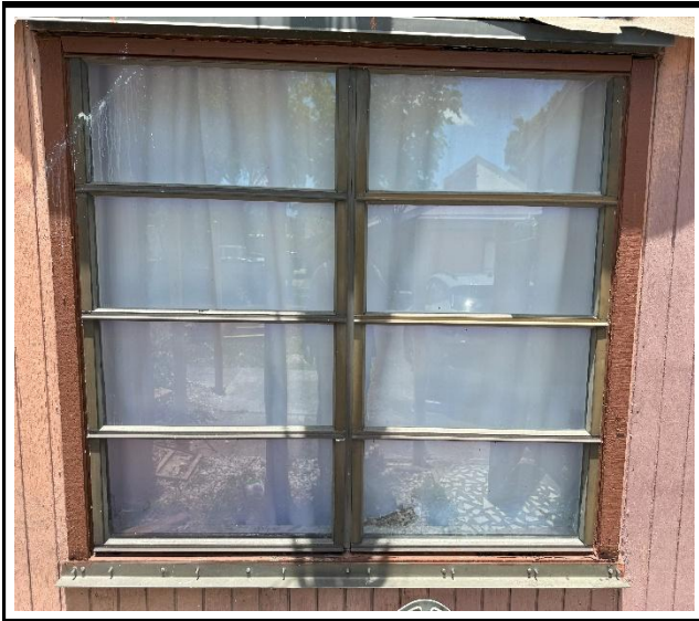
Photo 1 : Existing non-impact-rated window frame
