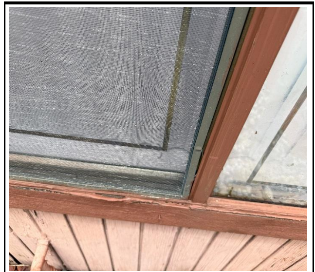
Photo 4 : Existing non-impact-rated window frame
