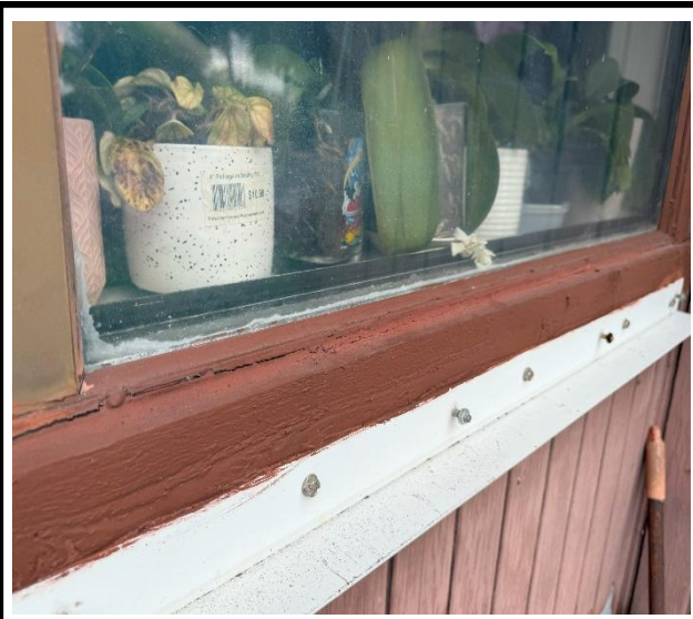
Photo 3 : Existing non-impact-rated window frame
