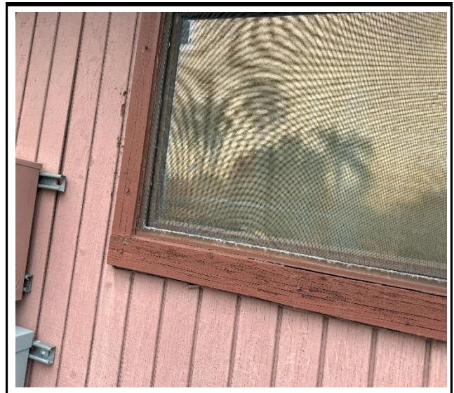
Photo 4 : Existing non-impact-rated window frame
