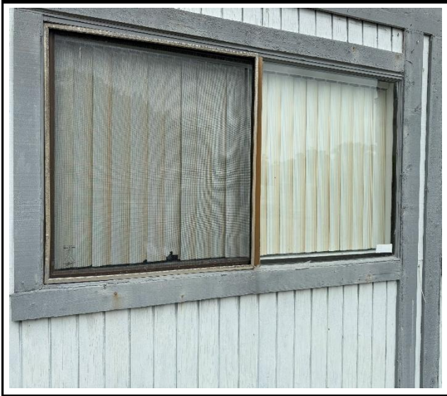
Photo 1 : Existing non-impact-rated window frame
