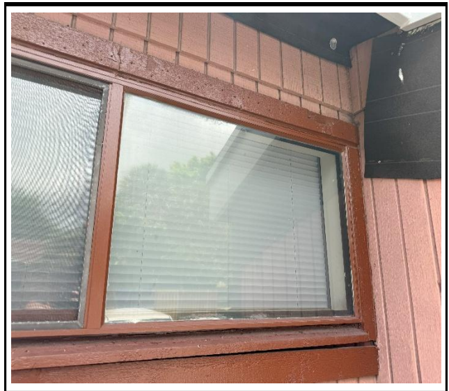
Photo 2 : Existing non-impact-rated window frame
