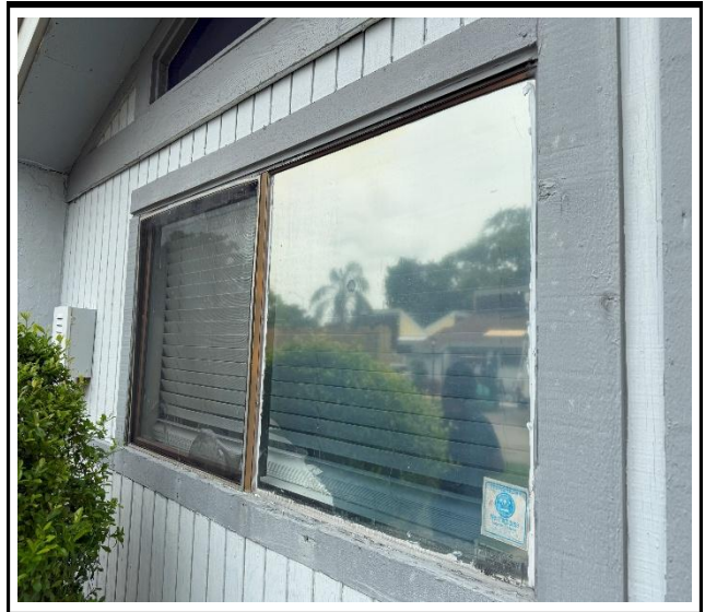
Photo 2 : Existing non-impact-rated window frame
