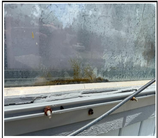
Photo 2 : Existing non-impact-rated window frame
