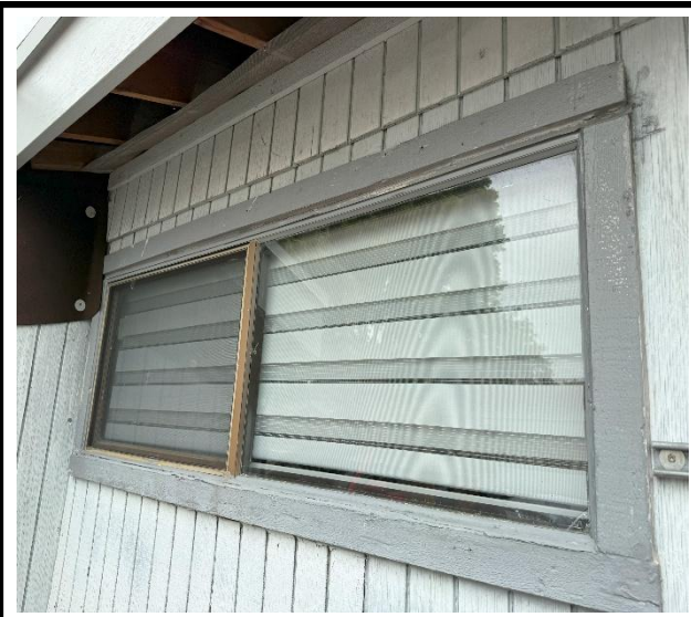
Photo 3 : Existing non-impact-rated window frame
