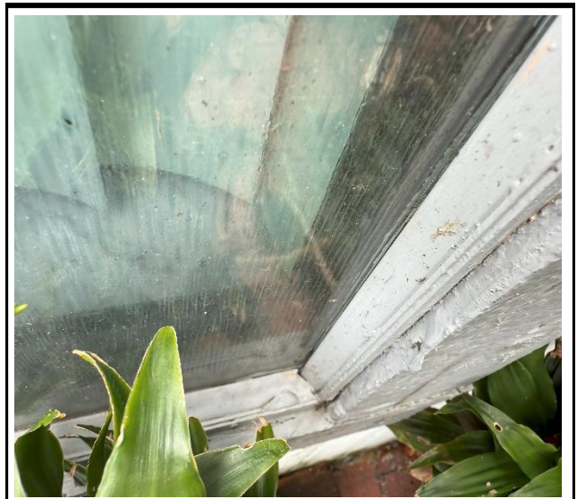
Photo 4 : Existing non-impact-rated window frame
