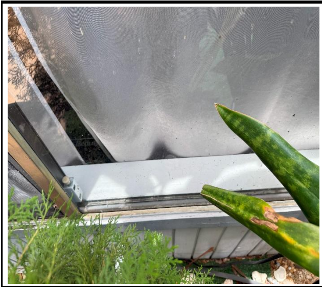
Photo 3 : Existing non-impact-rated window frame
