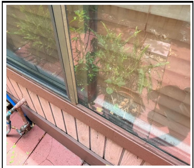
Photo 4 : Existing non-impact-rated window frame
