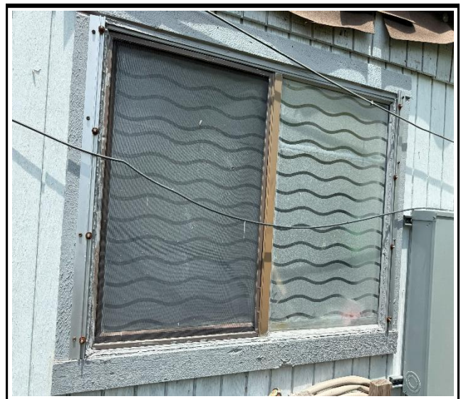
Photo 4 : Existing non-impact-rated window frame
