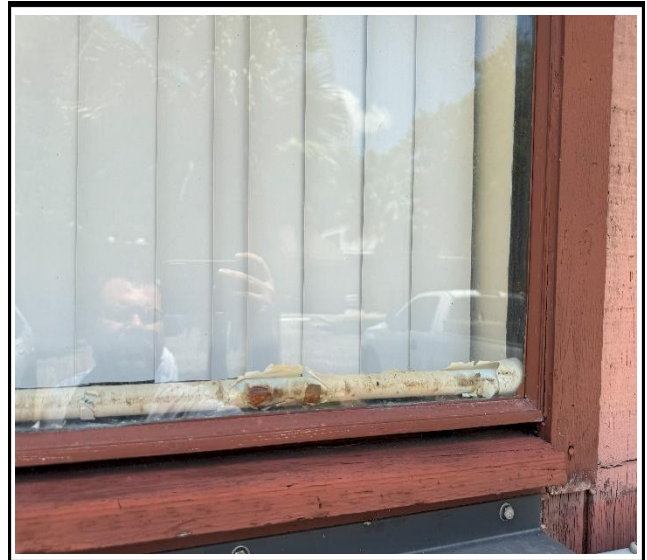
Photo 2 : Existing non-impact-rated window frame
