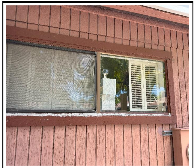
Photo 2 : Existing non-impact-rated window frame
