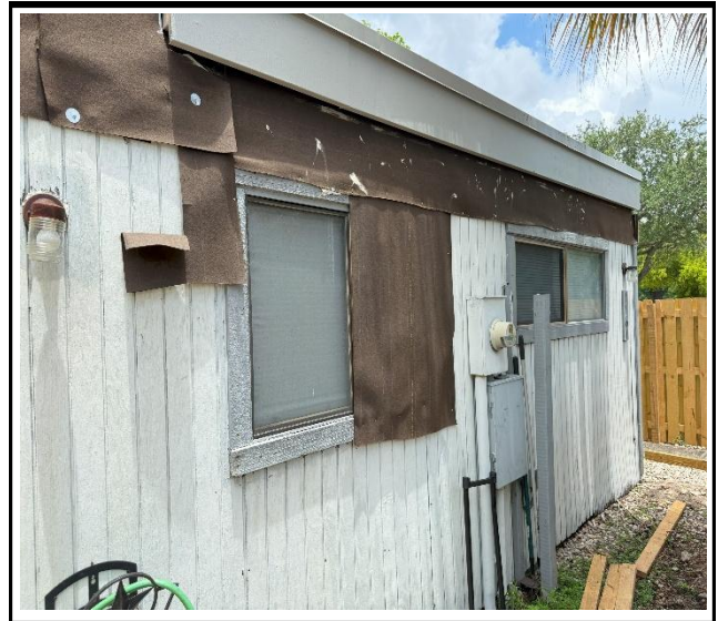
Photo 2 : Existing non-impact-rated window frame
