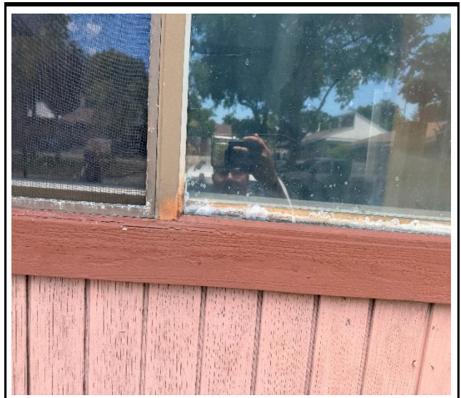
Photo 4 : Existing non-impact-rated window frame
