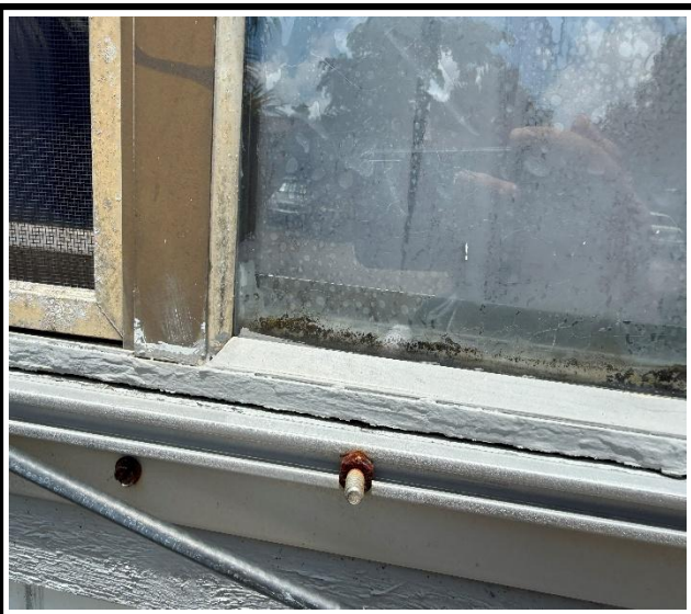
Photo 3 : Existing non-impact-rated window frame
