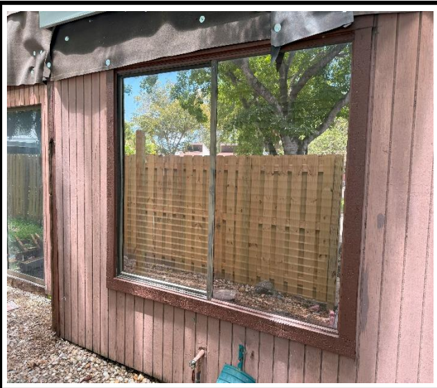
Photo 1 : Existing non-impact-rated window frame
