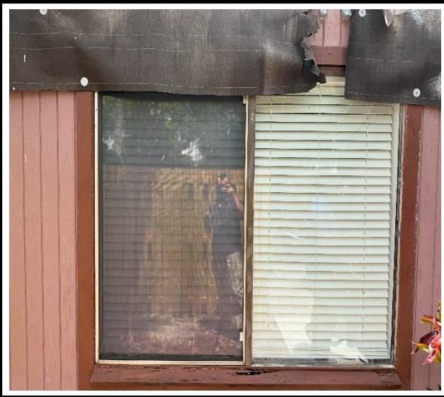
Photo 1 : Existing non-impact-rated window frame
