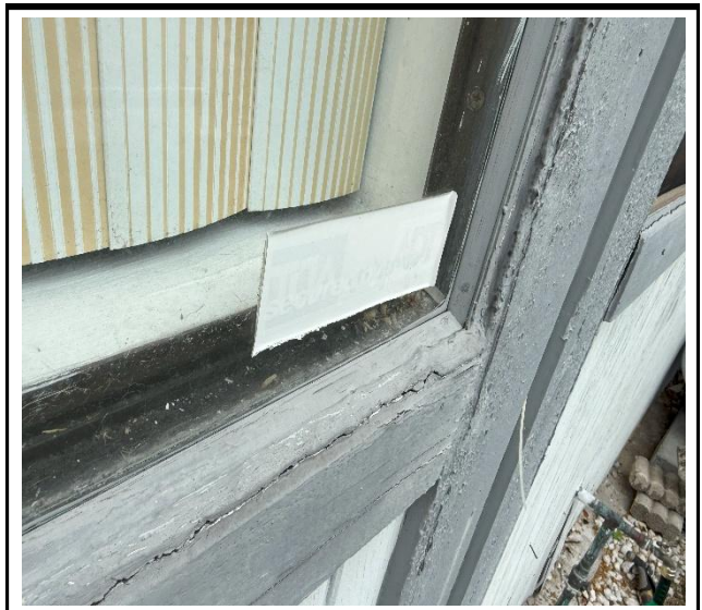
Photo 4 : Existing non-impact-rated window frame
