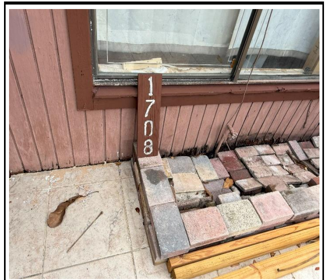
Photo 4 : Existing non-impact-rated window frame
