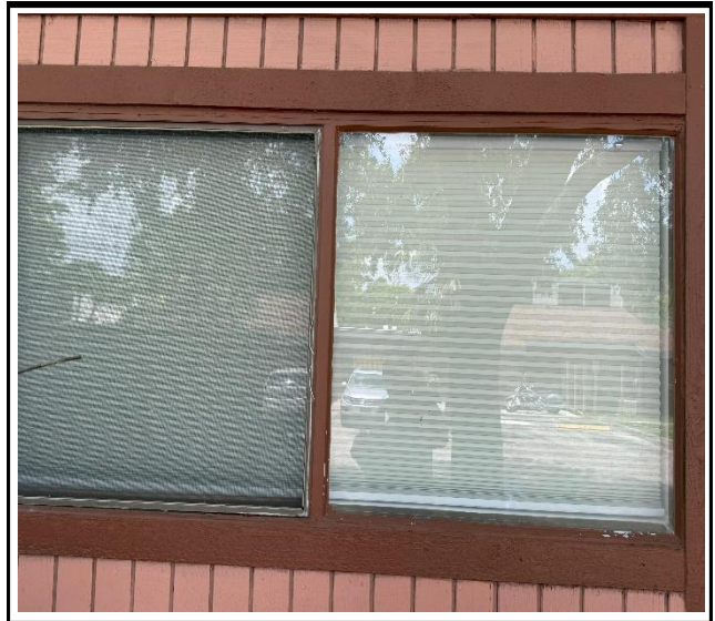
Photo 2 : Existing non-impact-rated window frame
