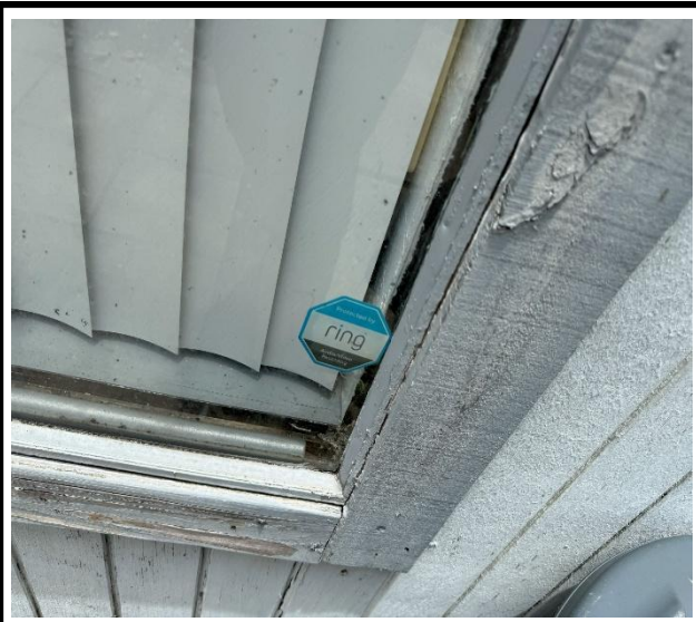
Photo 3 : Existing non-impact-rated window frame
