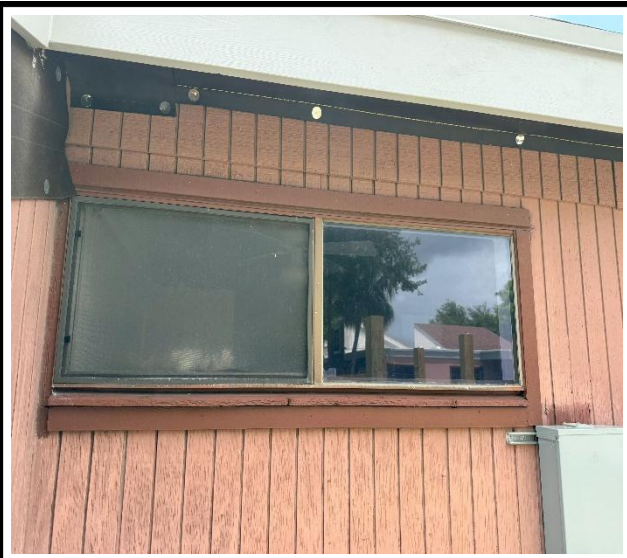
Photo 3 : Existing non-impact-rated window frame
