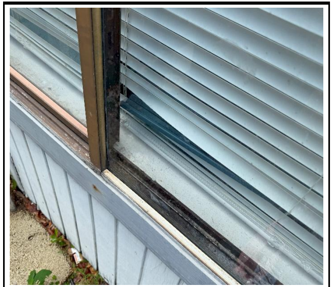
Photo 4 : Existing non-impact-rated window frame
