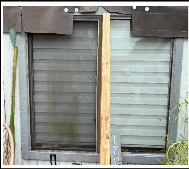
Photo 1 : Existing non-impact-rated window frame
