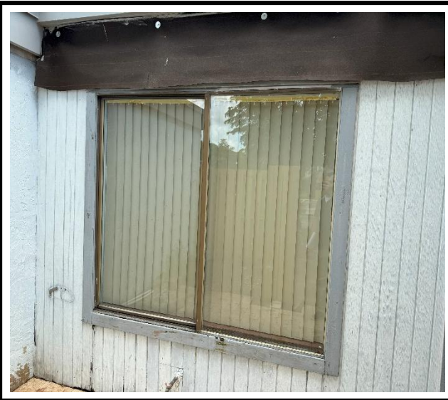
Photo 1 : Existing non-impact-rated window frame
