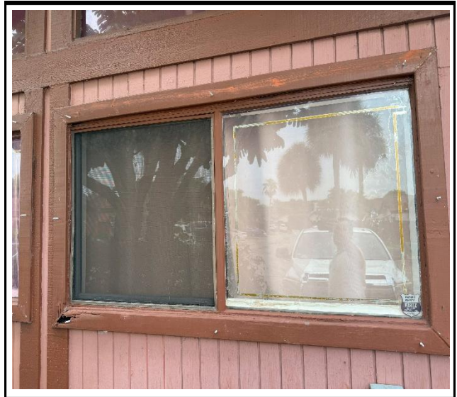
Photo 2 : Existing non-impact-rated window frame
