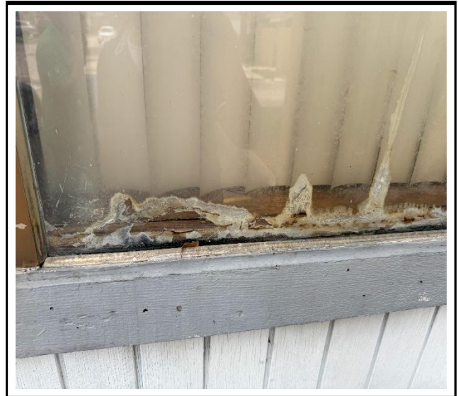
Photo 2 : Existing non-impact-rated window frame
