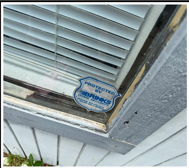
Photo 3 : Existing non-impact-rated window frame
