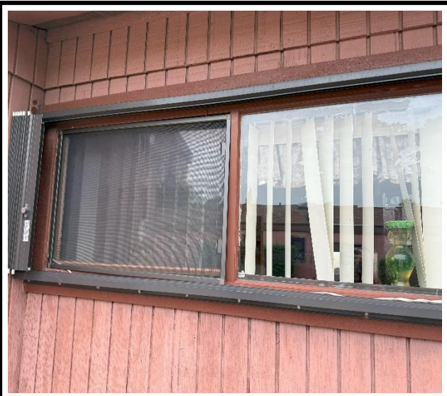
Photo 3 : Existing non-impact-rated window frame
