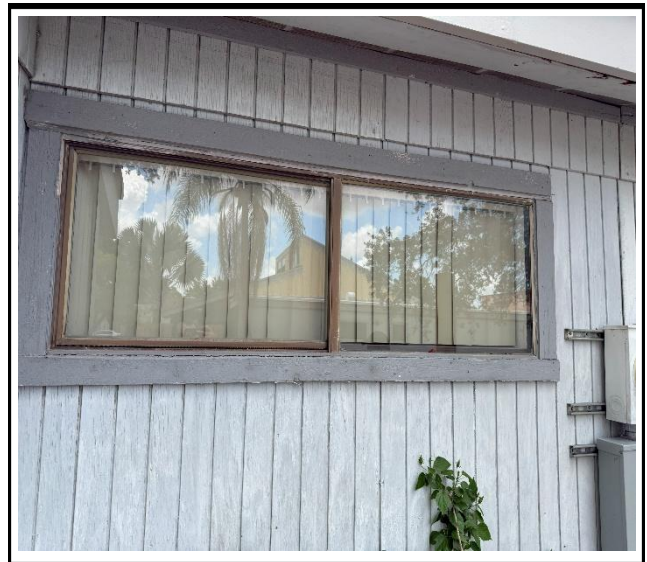
Photo 2 : Existing non-impact-rated window frame
