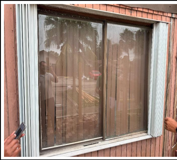
Photo 1 : Existing non-impact-rated window frame
