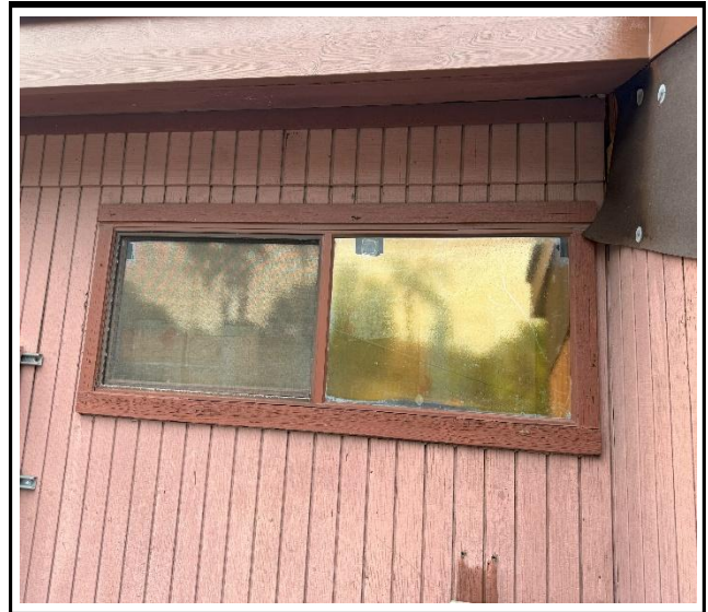
Photo 2 : Existing non-impact-rated window frame
