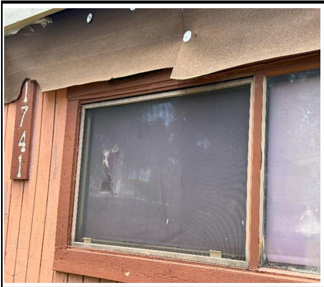
Photo 3 : Existing non-impact-rated window frame
