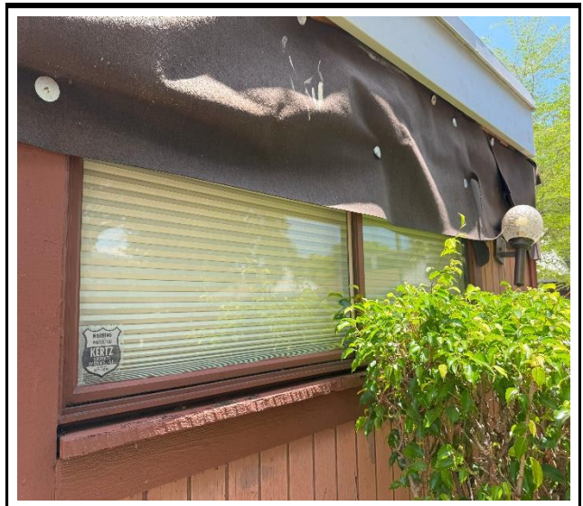
Photo 2 : Existing non-impact-rated window frame
