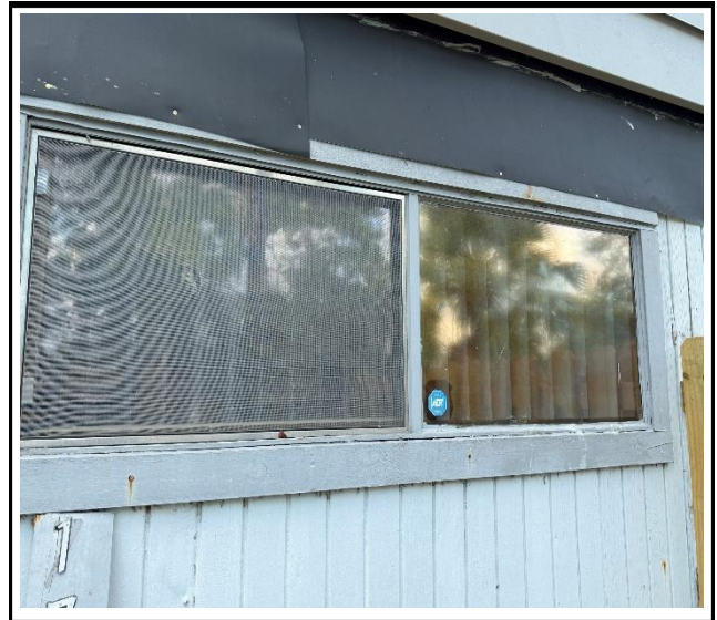
Photo 2 : Existing non-impact-rated window frame
