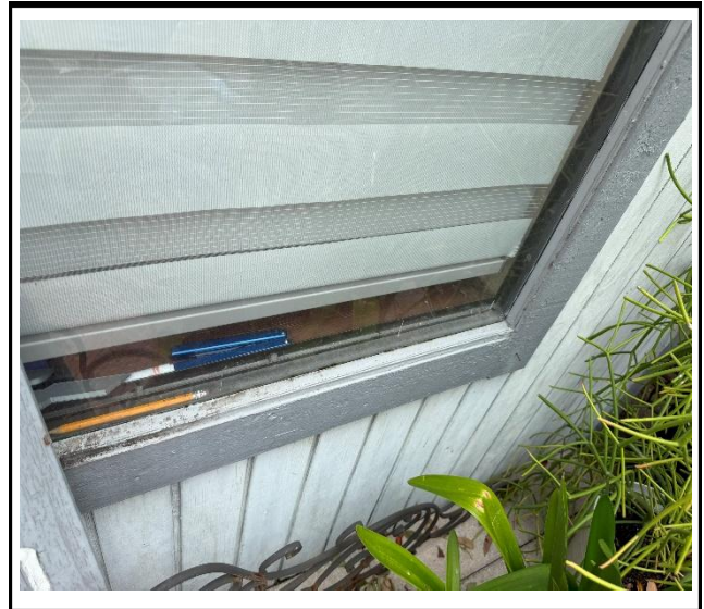
Photo 2 : Existing non-impact-rated window frame
