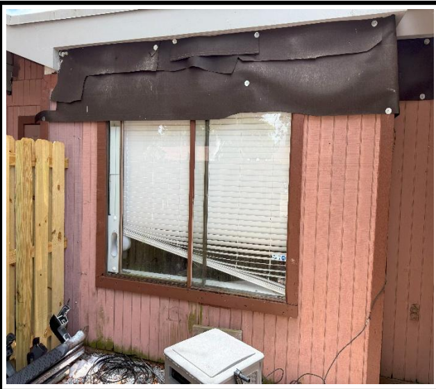
Photo 1 : Existing non-impact-rated window frame
