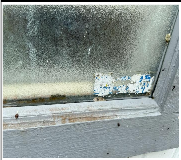
Photo 3 : Existing non-impact-rated window frame
