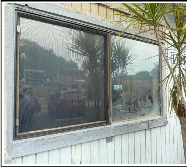
Photo 1 : Existing non-impact-rated window frame
