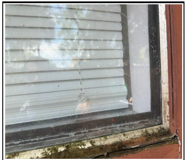
Photo 4 : Existing non-impact-rated window frame
