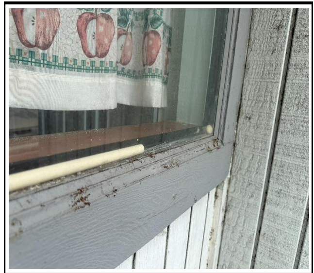
Photo 2 : Existing non-impact-rated window frame
