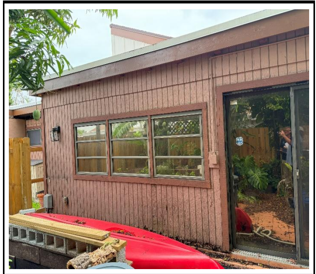
Photo 2 : Existing non-impact-rated window frame
