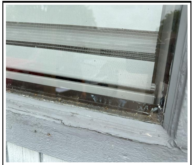
Photo 4 : Existing non-impact-rated window frame
