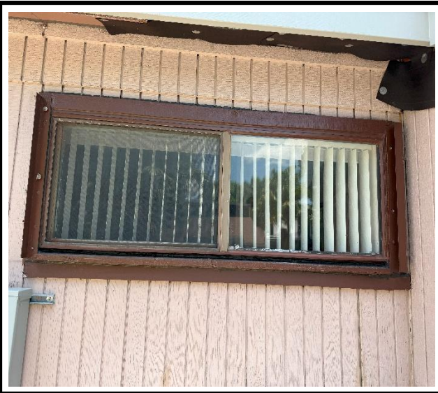
Photo 1 : Existing non-impact-rated window frame
