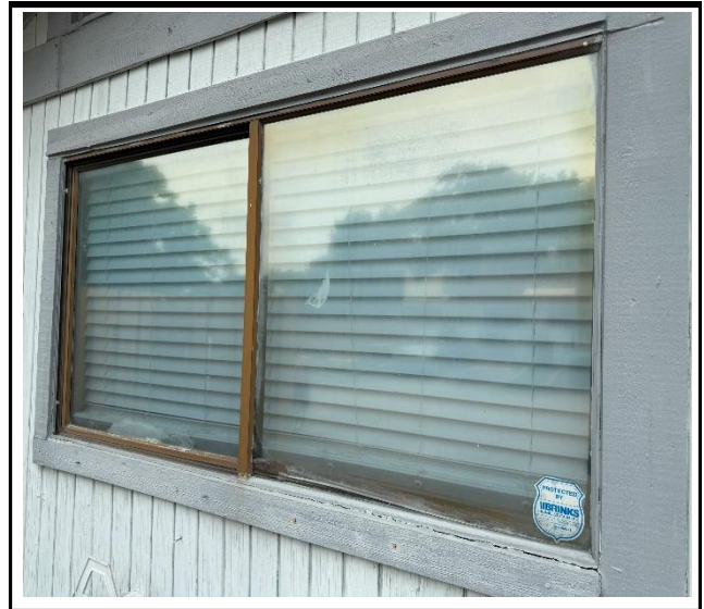
Photo 2 : Existing non-impact-rated window frame
