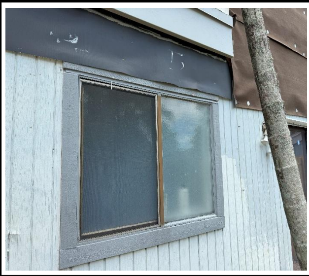
Photo 1 : Existing non-impact-rated window frame
