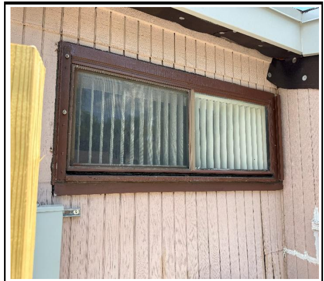
Photo 4 : Existing non-impact-rated window frame
