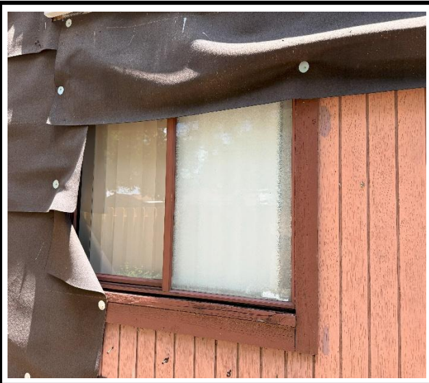
Photo 1 : Existing non-impact-rated window frame
