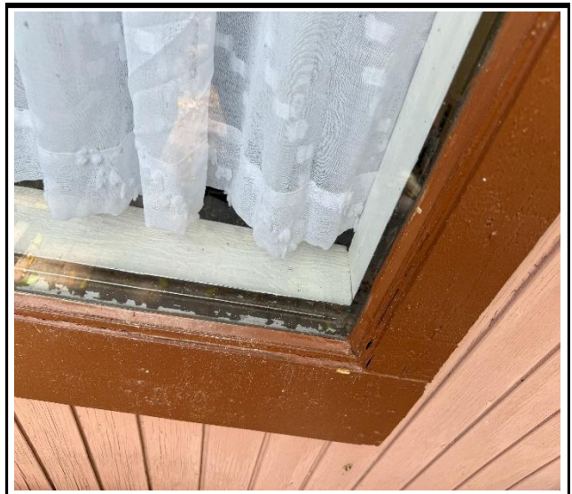
Photo 4 : Existing non-impact-rated window frame
