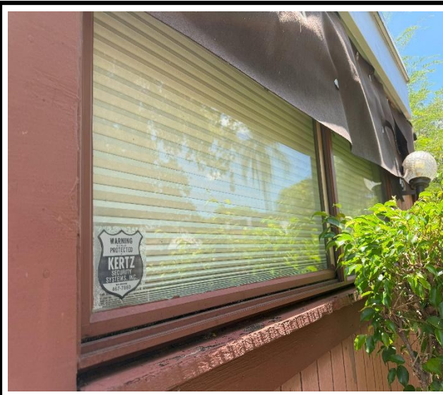
Photo 3 : Existing non-impact-rated window frame
