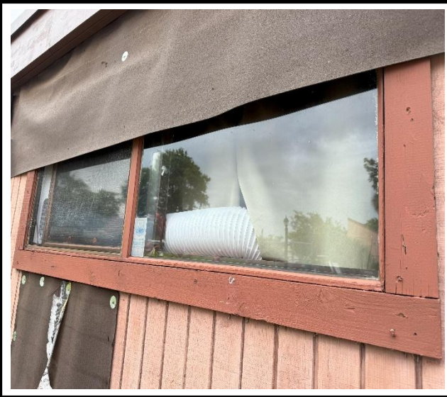
Photo 1 : Existing non-impact-rated window frame
