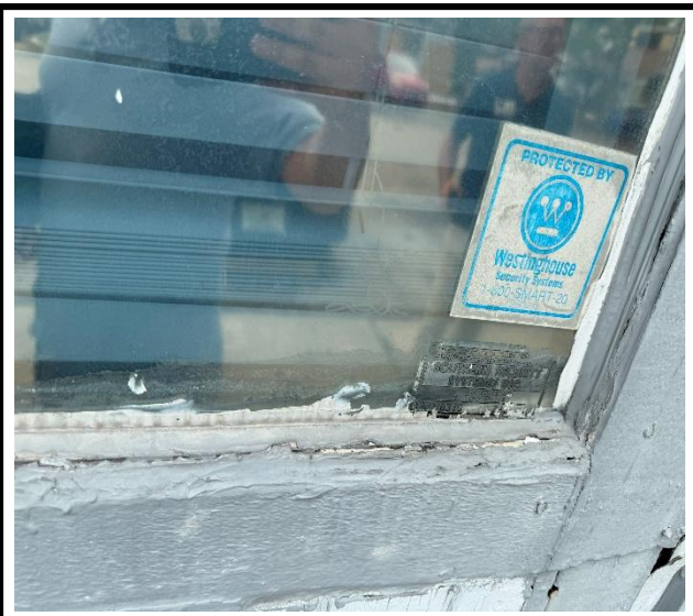
Photo 3 : Existing non-impact-rated window frame
