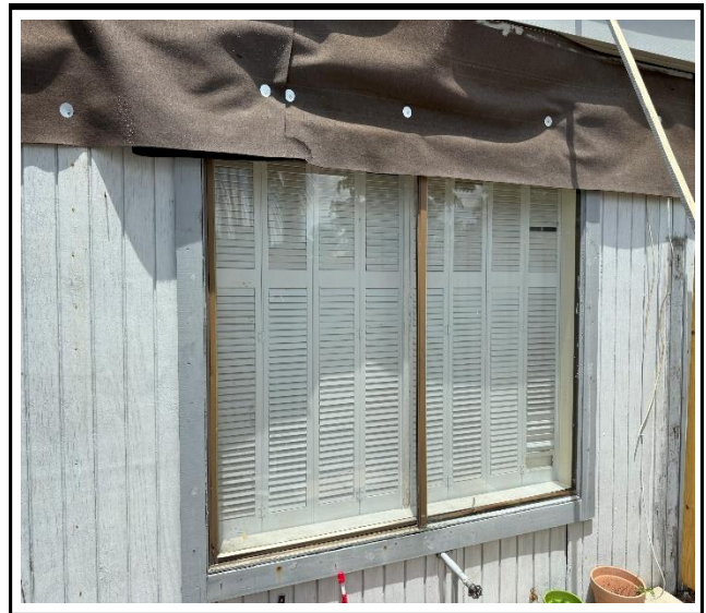
Photo 2 : Existing non-impact-rated window frame
