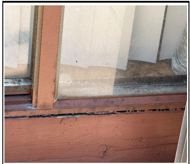
Photo 4 : Existing non-impact-rated window frame
