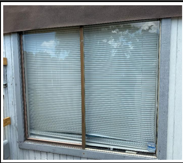
Photo 1 : Existing non-impact-rated window frame
