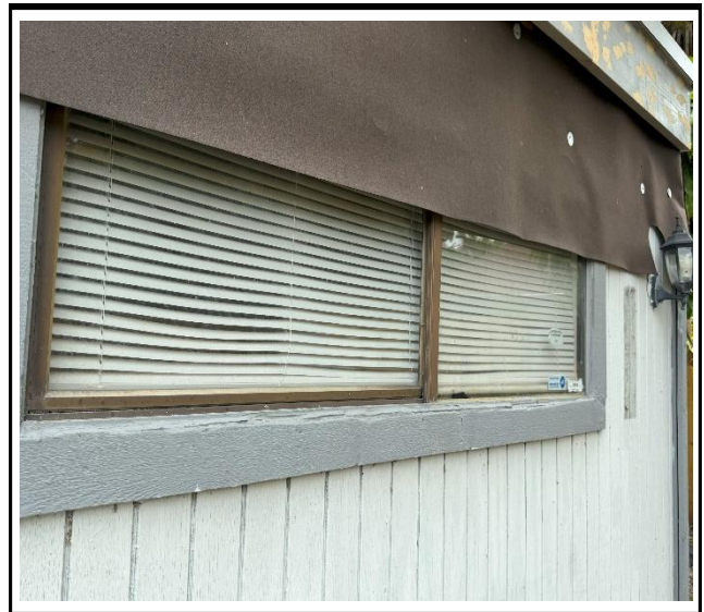
Photo 2 : Existing non-impact-rated window frame
