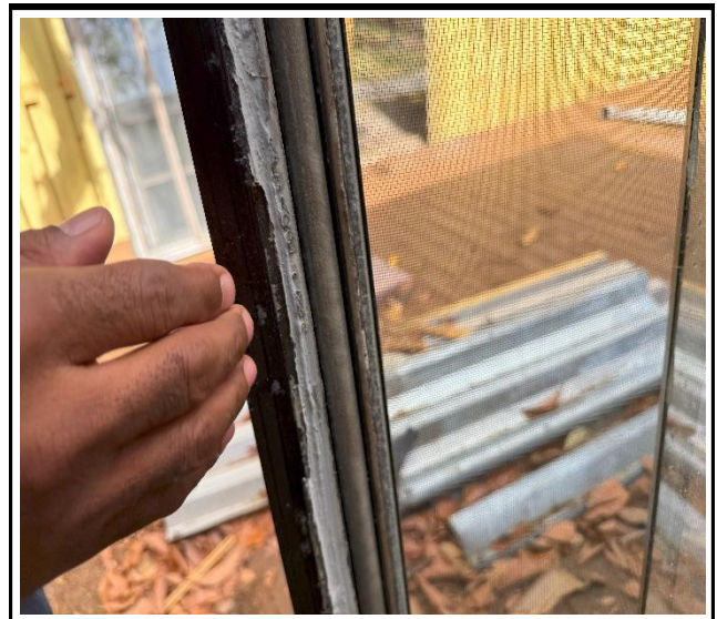
Photo 4 : Existing non-impact-rated window frame
