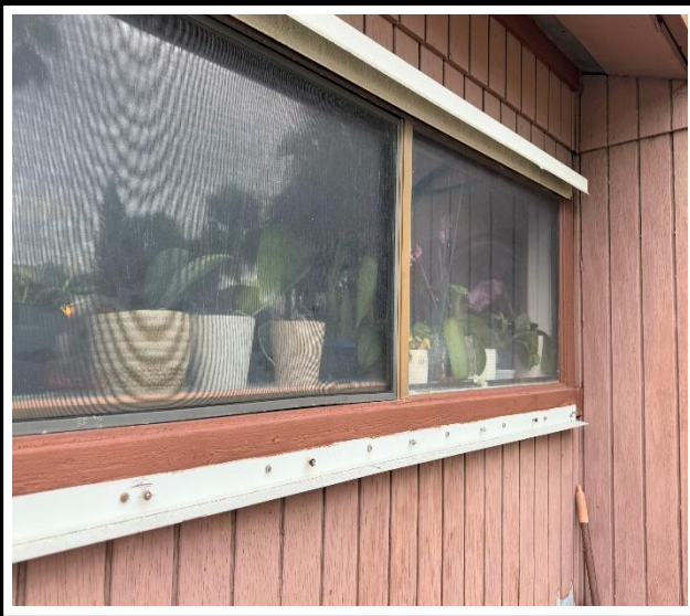
Photo 1 : Existing non-impact-rated window frame
