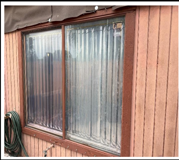
Photo 1 : Existing non-impact-rated window frame
