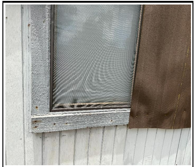
Photo 4 : Existing non-impact-rated window frame
