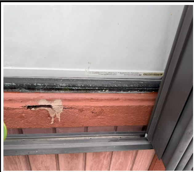
Photo 3 : Existing non-impact-rated window frame
