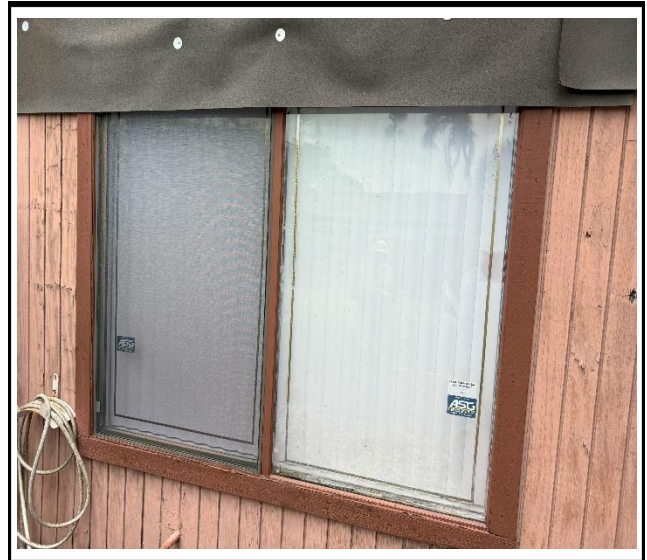
Photo 2 : Existing non-impact-rated window frame
