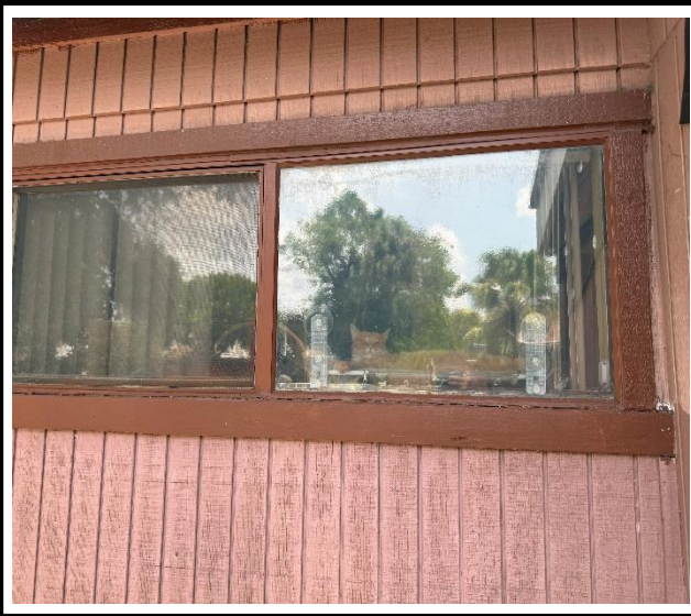
Photo 1 : Existing non-impact-rated window frame
