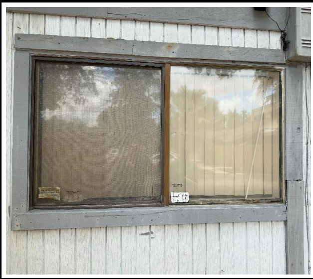
Photo 1 : Existing non-impact-rated window frame
