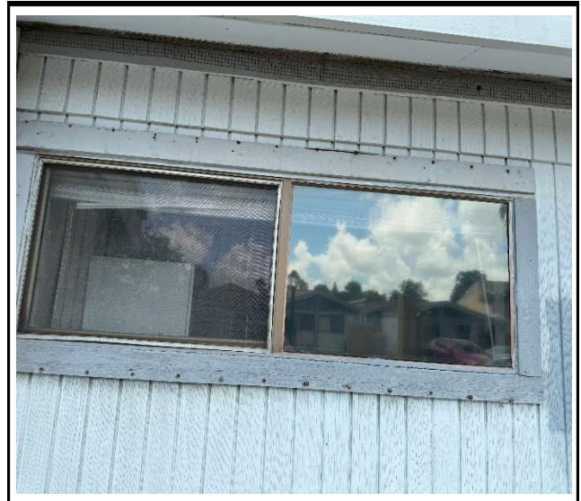
Photo 2 : Existing non-impact-rated window frame
