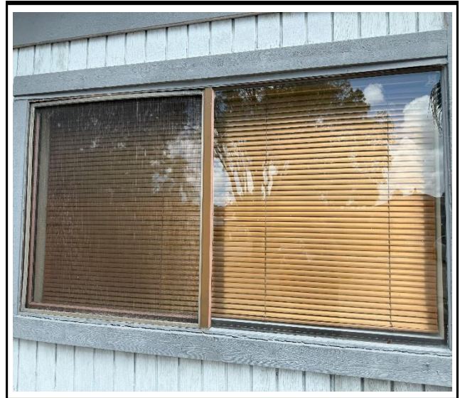
Photo 2 : Existing non-impact-rated window frame
