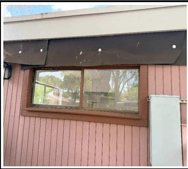
Photo 1 : Existing non-impact-rated window frame
