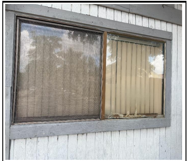
Photo 4 : Existing non-impact-rated window frame
