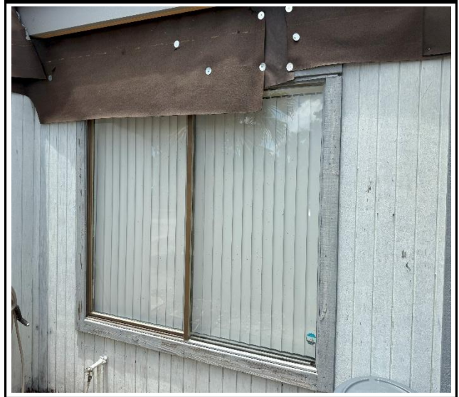
Photo 2 : Existing non-impact-rated window frame
