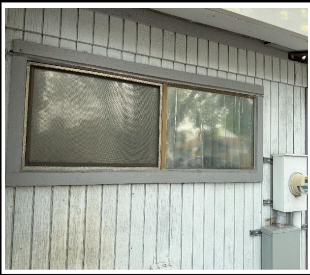
Photo 1 : Existing non-impact-rated window frame
