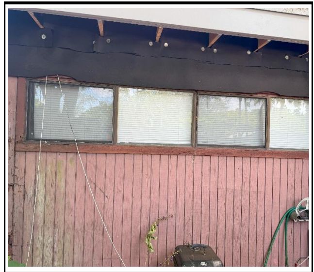
Photo 2 : Existing non-impact-rated window frame
