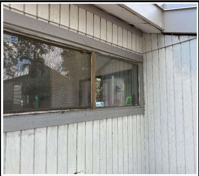
Photo 2 : Existing non-impact-rated window frame
