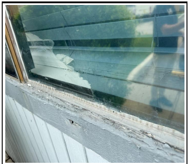
Photo 4 : Existing non-impact-rated window frame
