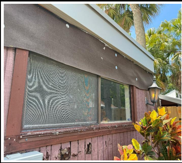
Photo 1 : Existing non-impact-rated window frame
