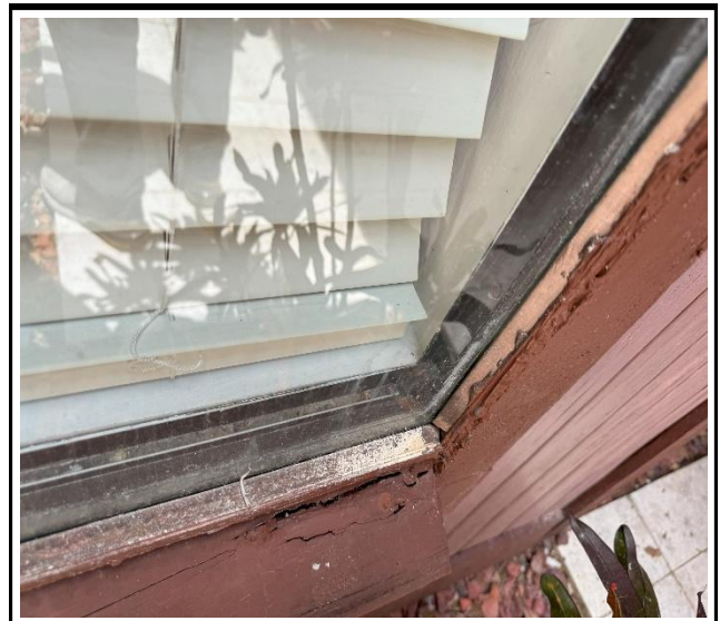
Photo 4 : Existing non-impact-rated window frame
