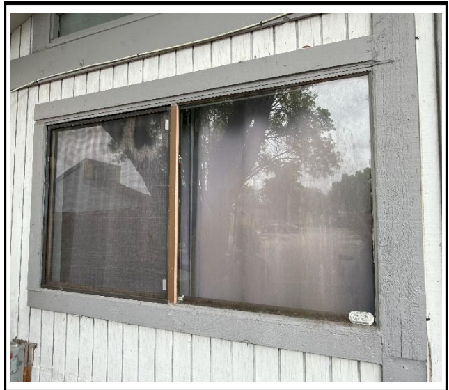
Photo 2 : Existing non-impact-rated window frame
