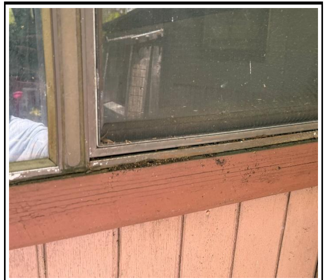
Photo 4 : Existing non-impact-rated window frame
