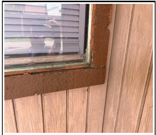
Photo 2 : Existing non-impact-rated window frame
