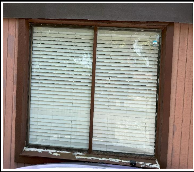
Photo 1 : Existing non-impact-rated window frame
