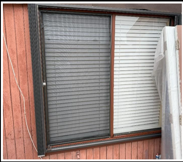
Photo 1 : Existing non-impact-rated window frame
