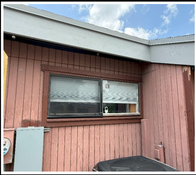
Photo 1 : Existing non-impact-rated window frame
