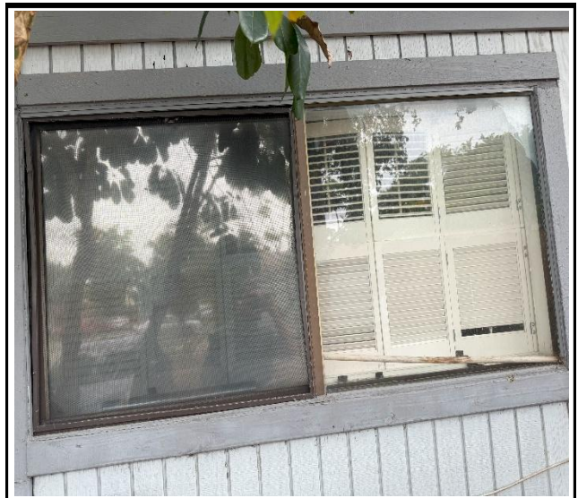
Photo 4 : Existing non-impact-rated window frame
