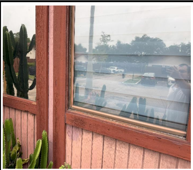
Photo 3 : Existing non-impact-rated window frame
