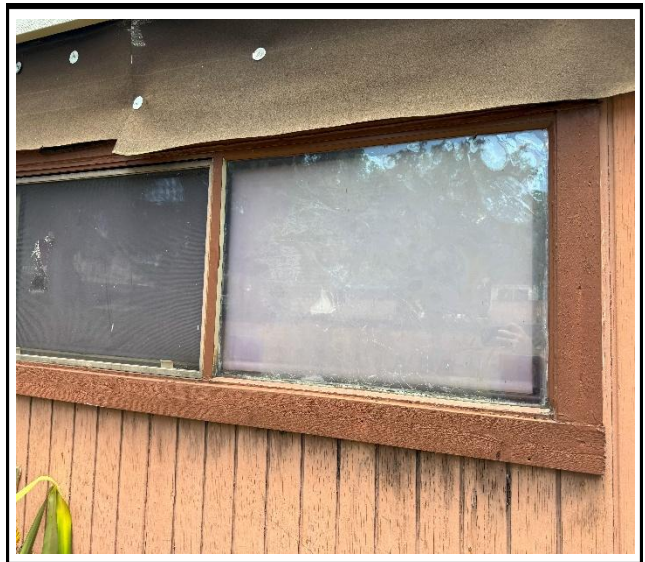
Photo 2 : Existing non-impact-rated window frame
