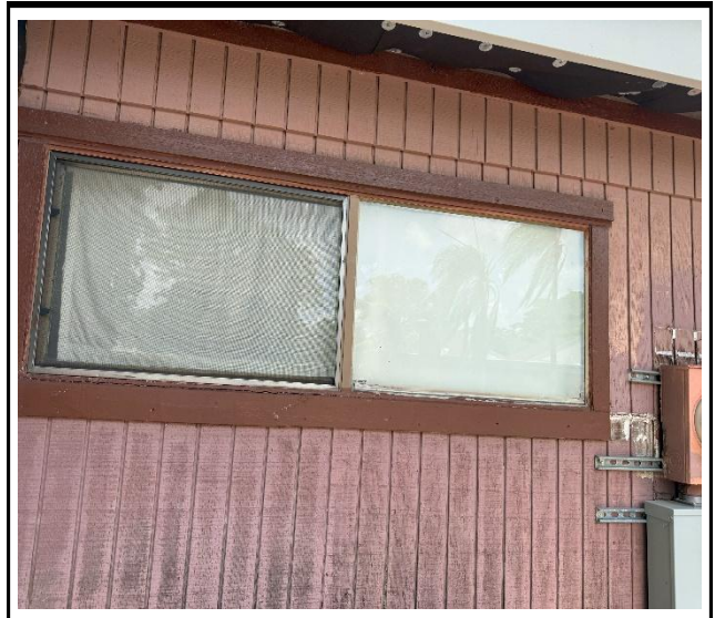
Photo 2 : Existing non-impact-rated window frame
