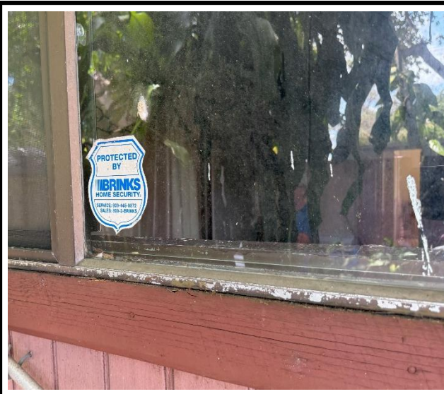
Photo 3 : Existing non-impact-rated window frame
