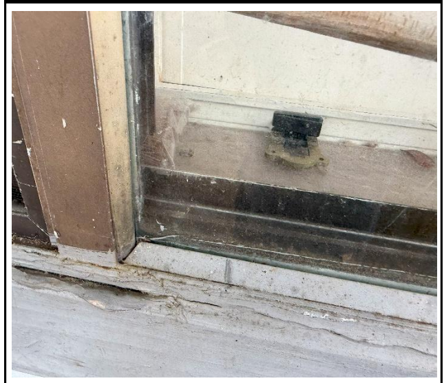
Photo 2 : Existing non-impact-rated window frame
