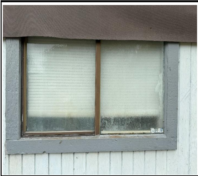
Photo 1 : Existing non-impact-rated window frame
