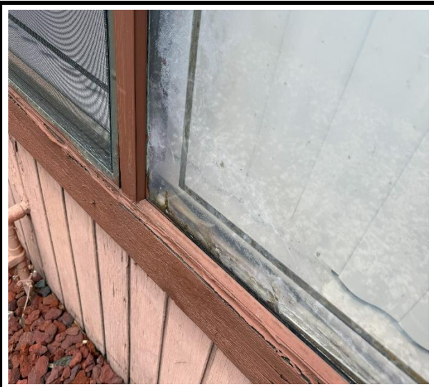
Photo 3 : Existing non-impact-rated window frame
