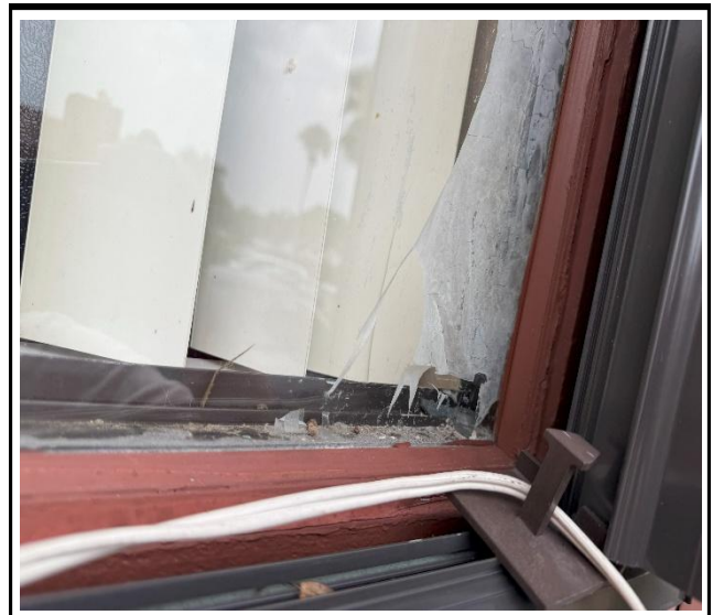
Photo 4 : Existing non-impact-rated window frame
