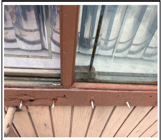
Photo 2 : Existing non-impact-rated window frame
