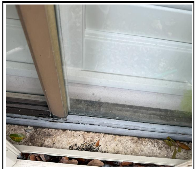
Photo 2 : Existing non-impact-rated window frame
