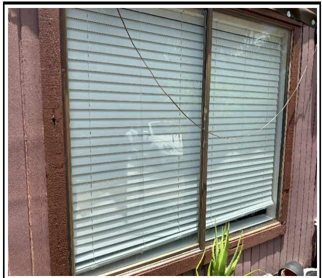
Photo 4 : Existing non-impact-rated window frame
