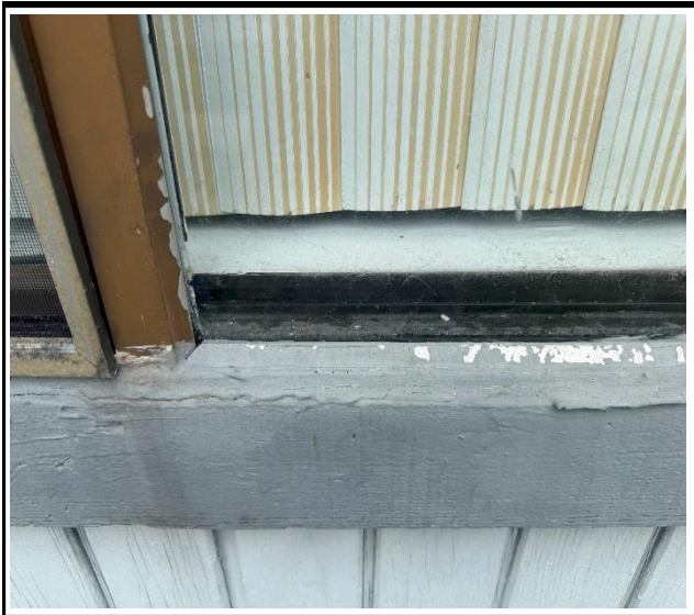
Photo 3 : Existing non-impact-rated window frame
