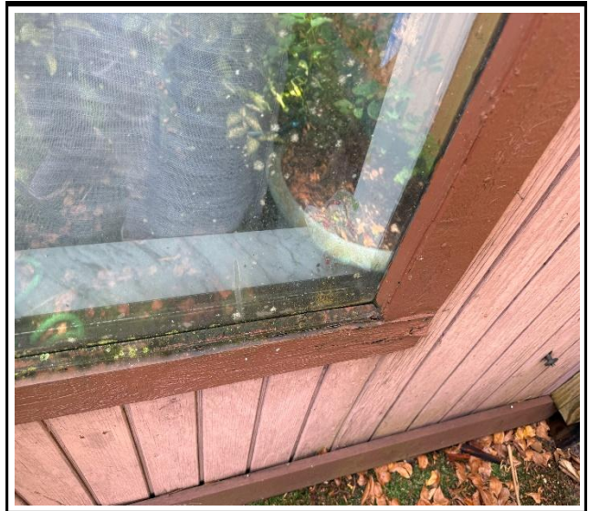
Photo 2 : Existing non-impact-rated window frame
