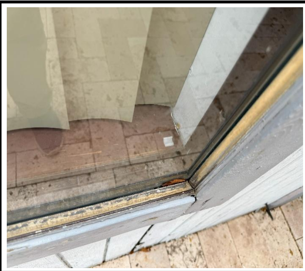
Photo 3 : Existing non-impact-rated window frame
