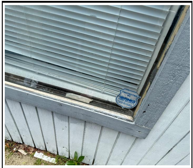
Photo 2 : Existing non-impact-rated window frame
