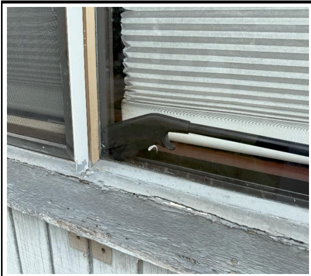
Photo 3 : Existing non-impact-rated window frame
