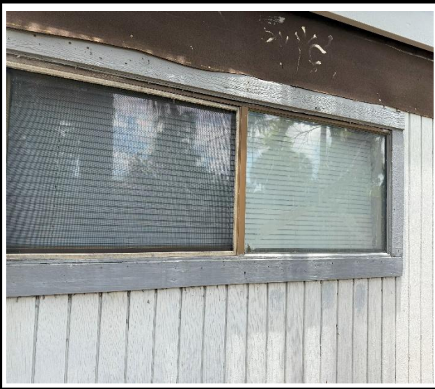
Photo 1 : Existing non-impact-rated window frame
