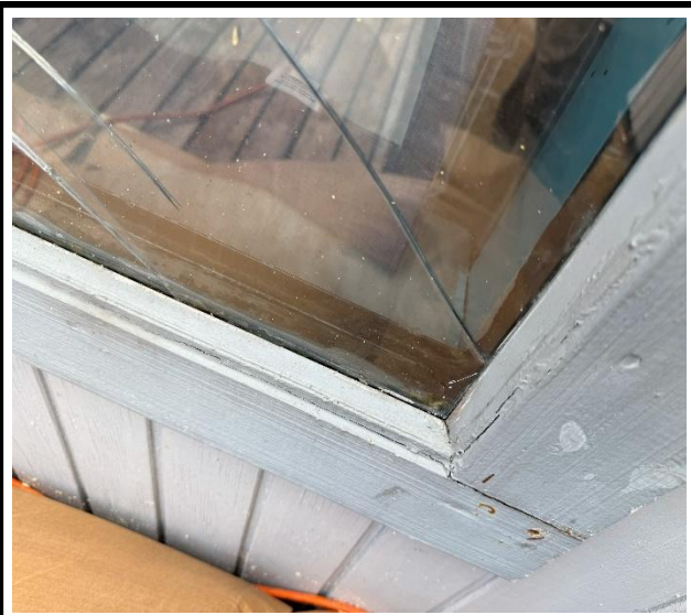
Photo 3 : Existing non-impact-rated window frame
