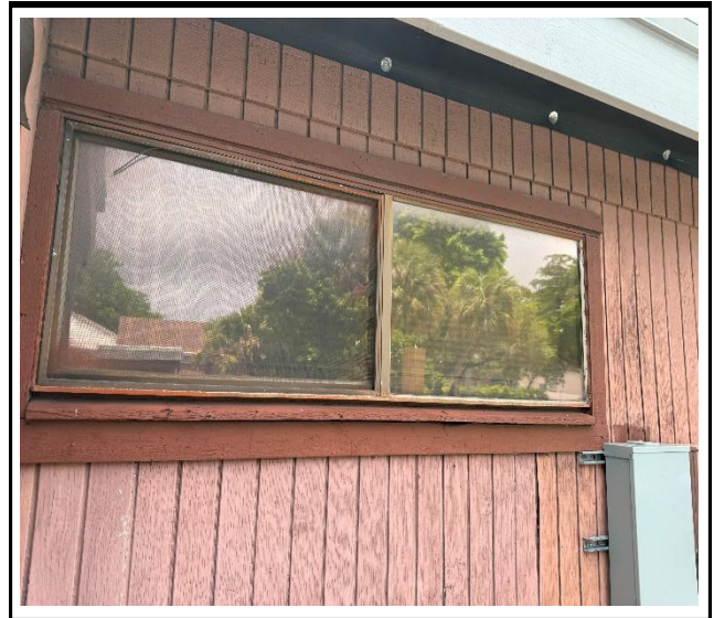
Photo 2 : Existing non-impact-rated window frame
