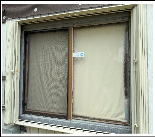
Photo 1 : Existing non-impact-rated window frame
