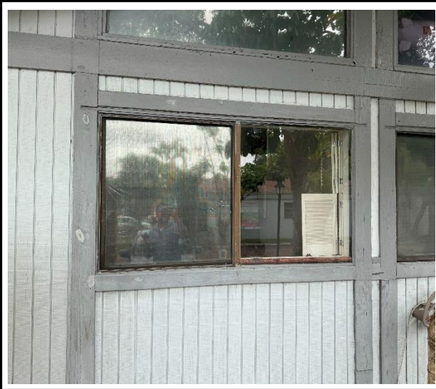
Photo 1 : Existing non-impact-rated window frame
