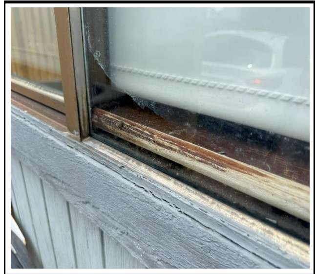
Photo 2 : Existing non-impact-rated window frame
