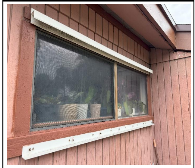
Photo 2 : Existing non-impact-rated window frame
