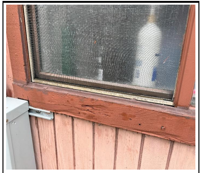
Photo 4 : Existing non-impact-rated window frame
