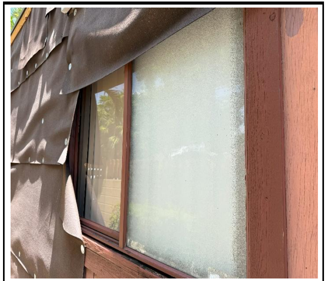
Photo 4 : Existing non-impact-rated window frame
