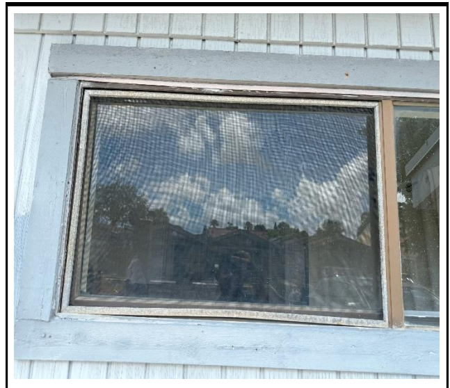
Photo 4 : Existing non-impact-rated window frame
