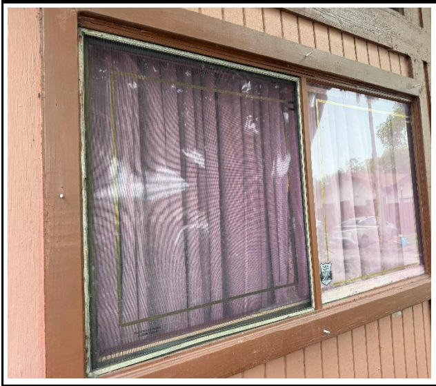
Photo 1 : Existing non-impact-rated window frame
