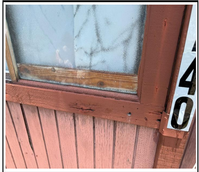
Photo 2 : Existing non-impact-rated window frame
