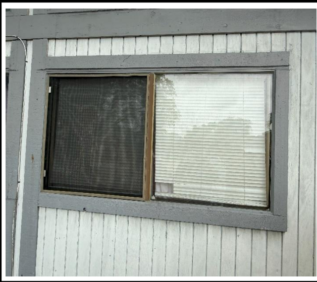
Photo 1 : Existing non-impact-rated window frame
