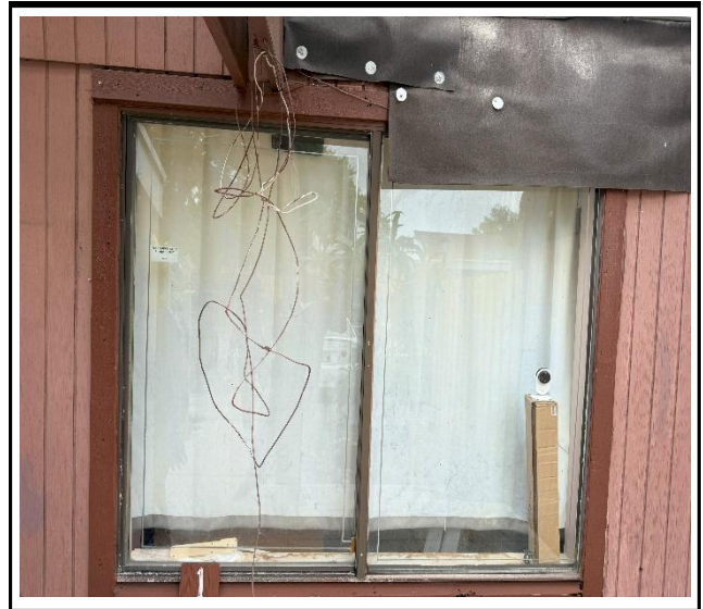
Photo 2 : Existing non-impact-rated window frame
