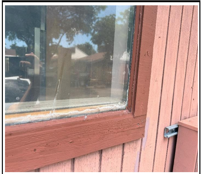
Photo 2 : Existing non-impact-rated window frame
