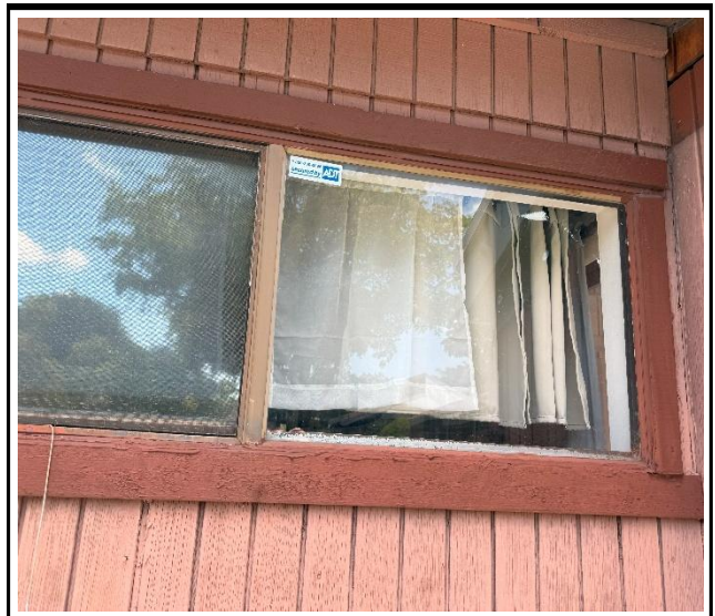
Photo 4 : Existing non-impact-rated window frame
