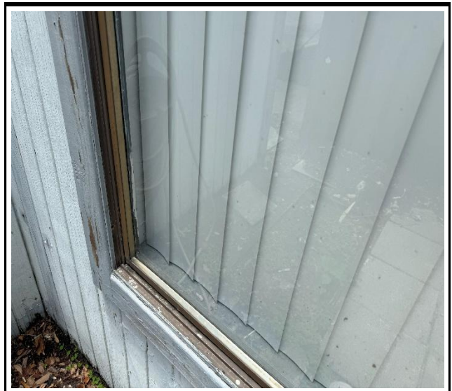
Photo 4 : Existing non-impact-rated window frame
