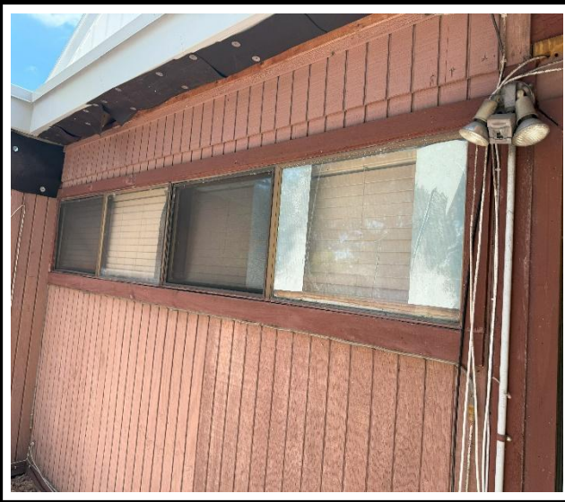
Photo 1 : Existing non-impact-rated window frame
