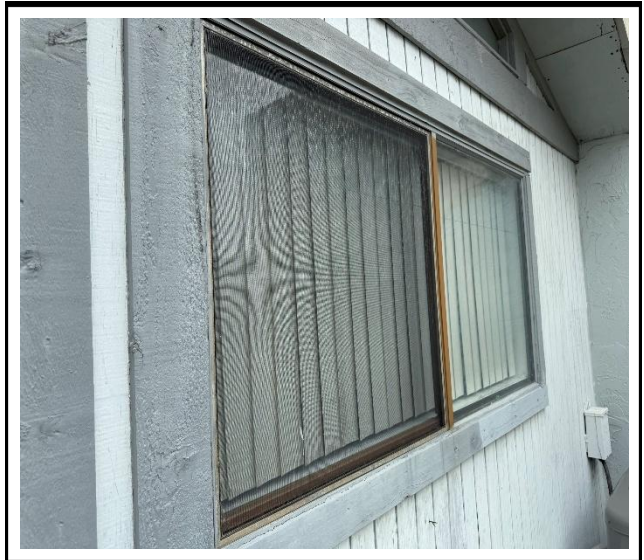
Photo 2 : Existing non-impact-rated window frame
