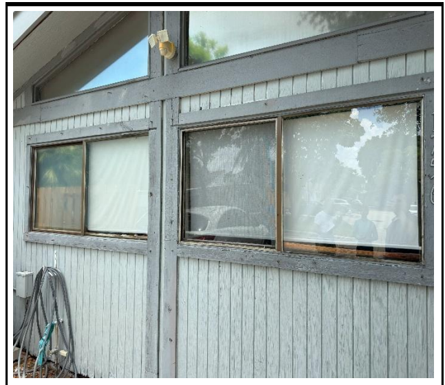
Photo 4 : Existing non-impact-rated window frame
