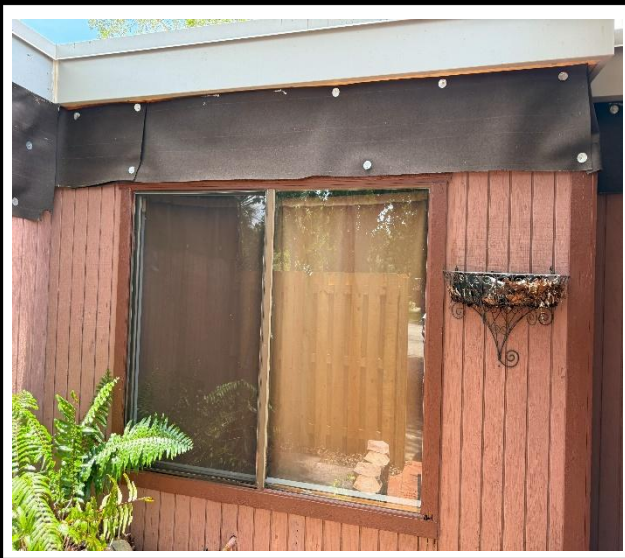
Photo 1 : Existing non-impact-rated window frame
