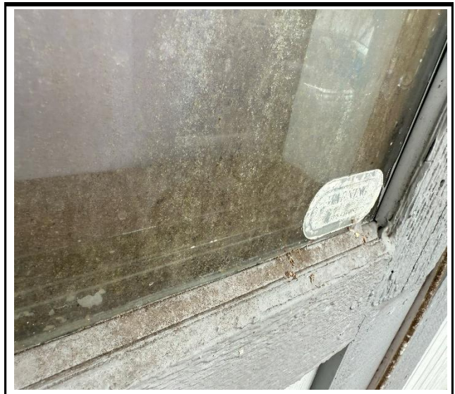
Photo 4 : Existing non-impact-rated window frame
