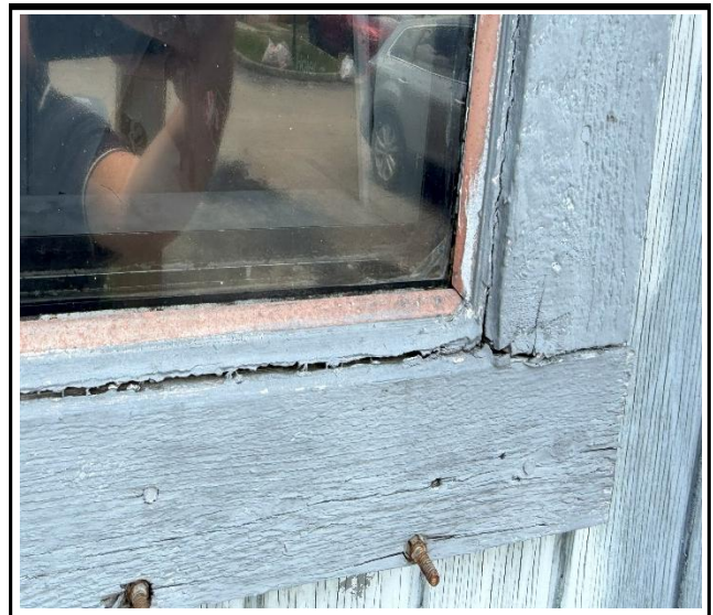
Photo 4 : Existing non-impact-rated window frame
