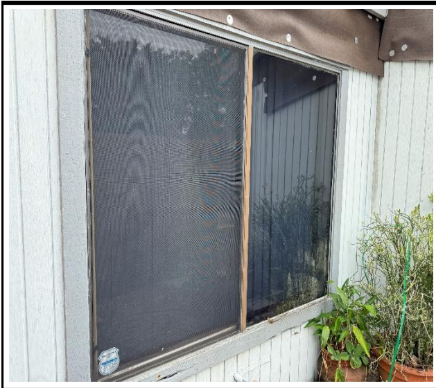
Photo 3 : Existing non-impact-rated window frame
