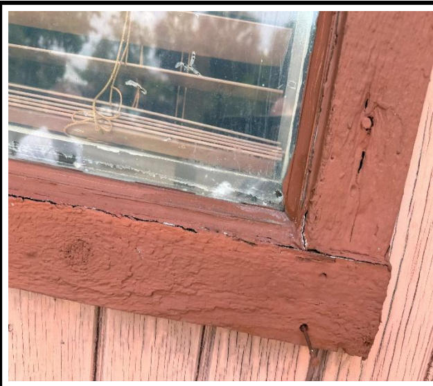
Photo 3 : Existing non-impact-rated window frame
