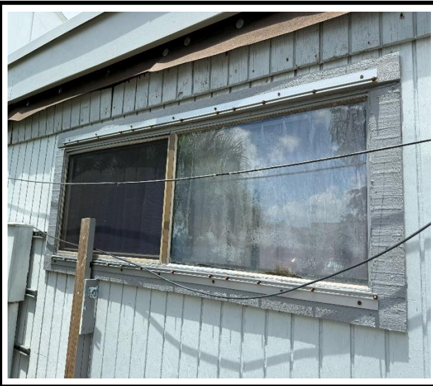
Photo 1 : Existing non-impact-rated window frame
