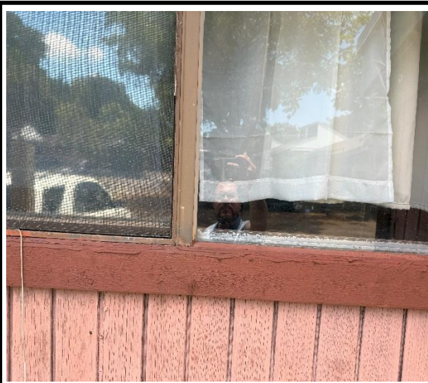
Photo 3 : Existing non-impact-rated window frame
