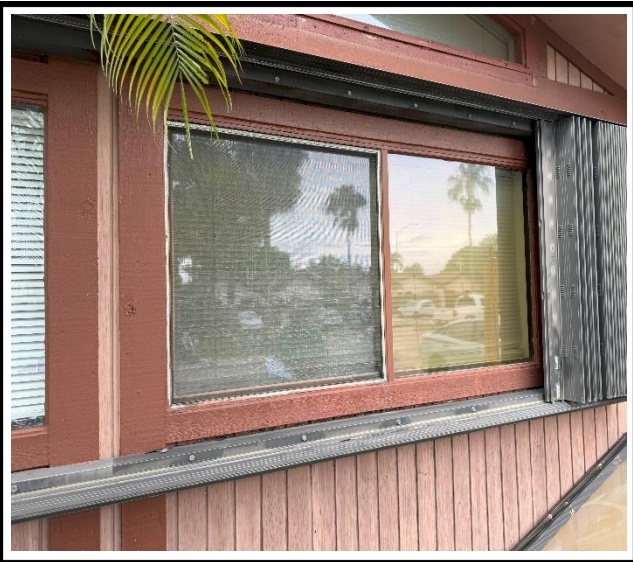
Photo 1 : Existing non-impact-rated window frame
