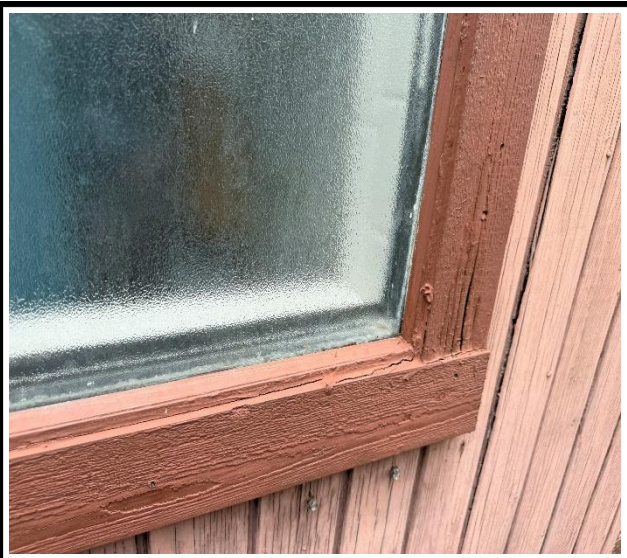
Photo 3 : Existing non-impact-rated window frame
