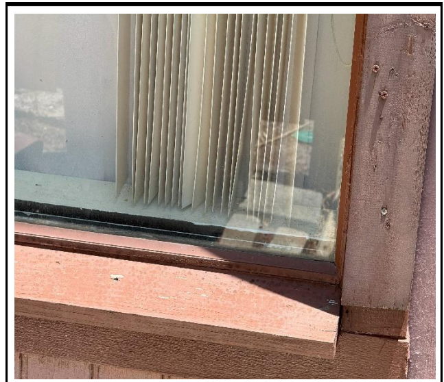
Photo 4 : Existing non-impact-rated window frame
