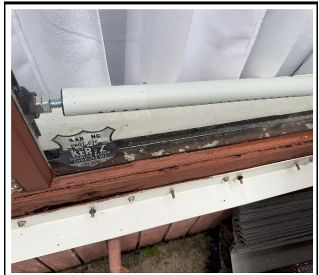
Photo 4 : Existing non-impact-rated window frame
