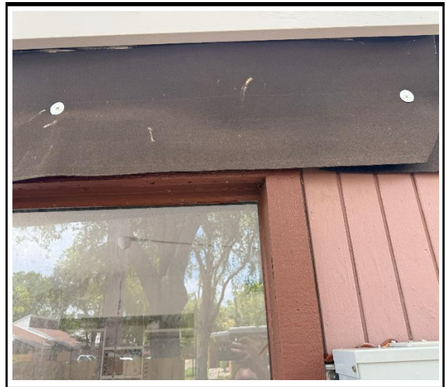
Photo 2 : Existing non-impact-rated window frame
