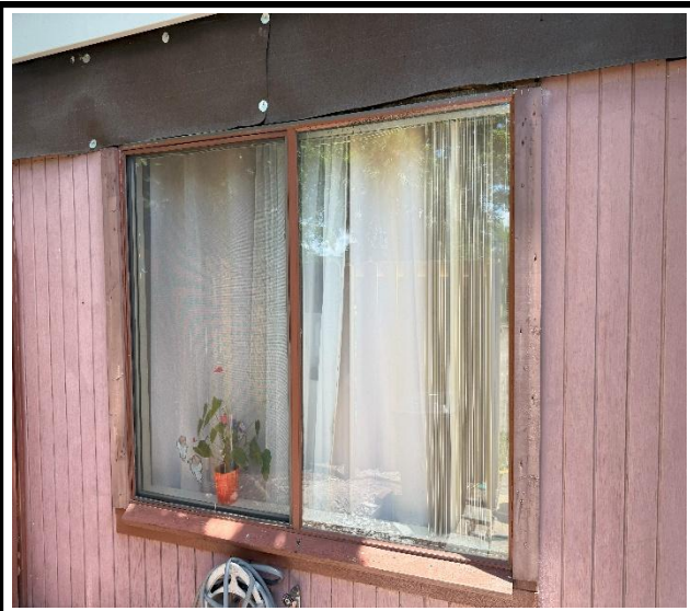
Photo 3 : Existing non-impact-rated window frame
