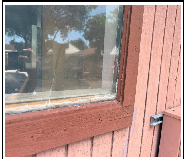
Photo 2 : Existing non-impact-rated window frame
