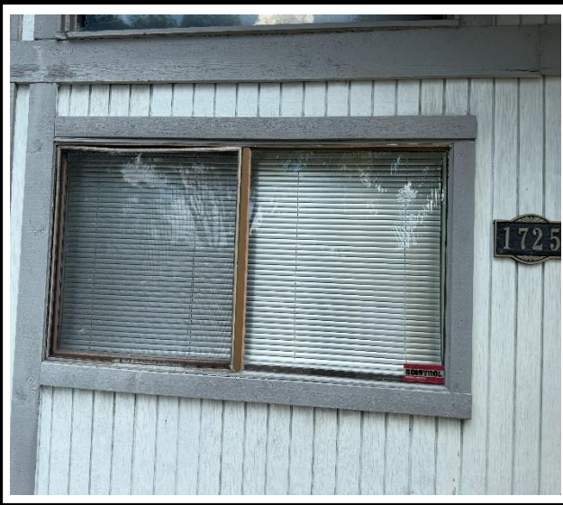
Photo 1 : Existing non-impact-rated window frame
