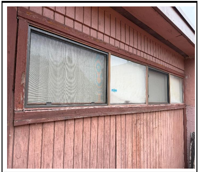
Photo 2 : Existing non-impact-rated window frame
