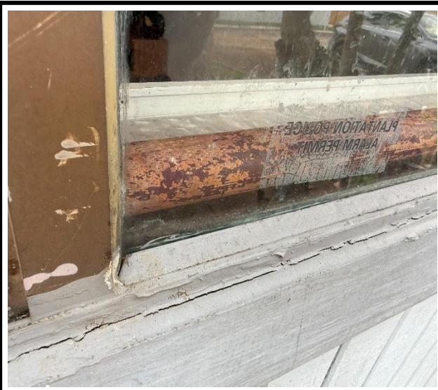
Photo 3 : Existing non-impact-rated window frame
