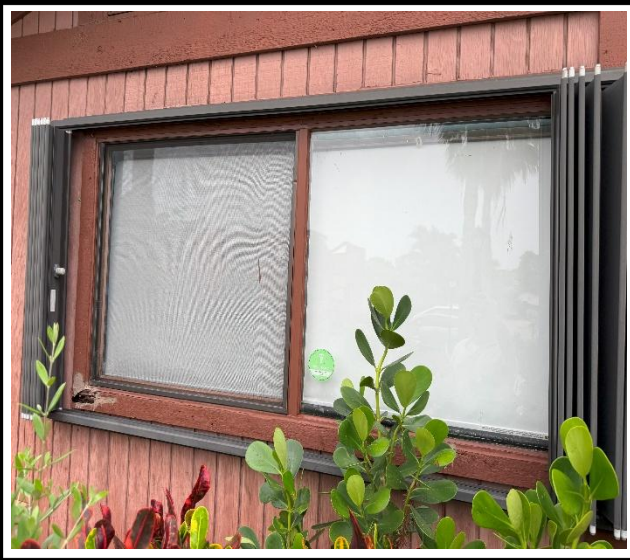
Photo 1 : Existing non-impact-rated window frame
