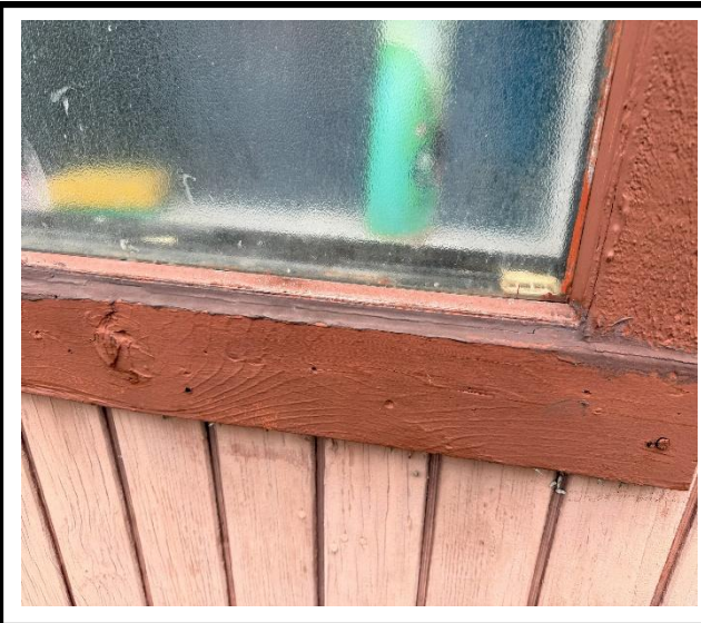
Photo 3 : Existing non-impact-rated window frame
