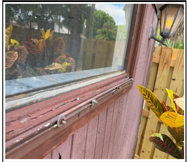
Photo 2 : Existing non-impact-rated window frame
