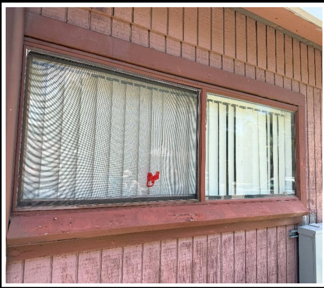
Photo 1 : Existing non-impact-rated window frame
