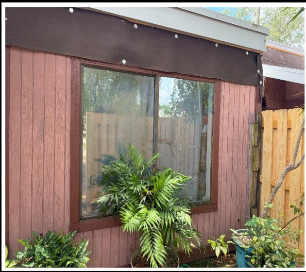
Photo 1 : Existing non-impact-rated window frame
