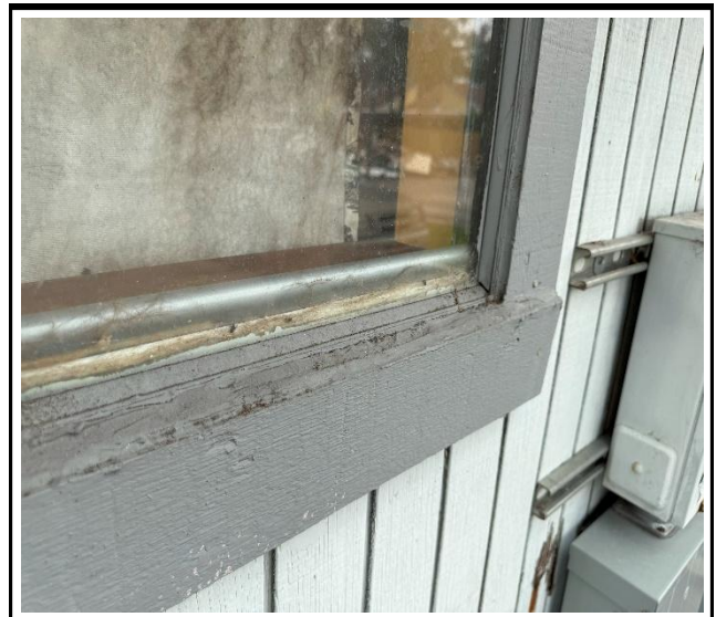
Photo 4 : Existing non-impact-rated window frame
