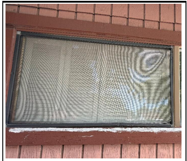
Photo 4 : Existing non-impact-rated window frame
