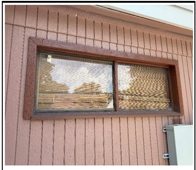
Photo 4 : Existing non-impact-rated window frame
