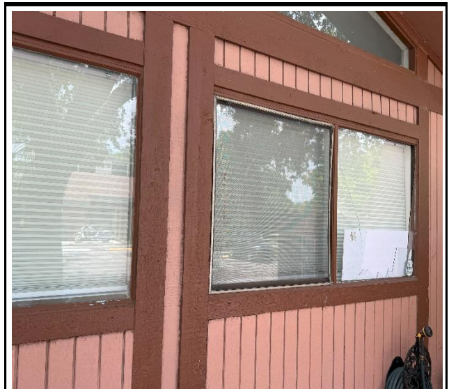
Photo 4 : Existing non-impact-rated window frame
