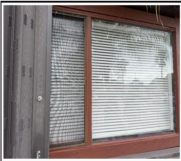
Photo 2 : Existing non-impact-rated window frame
