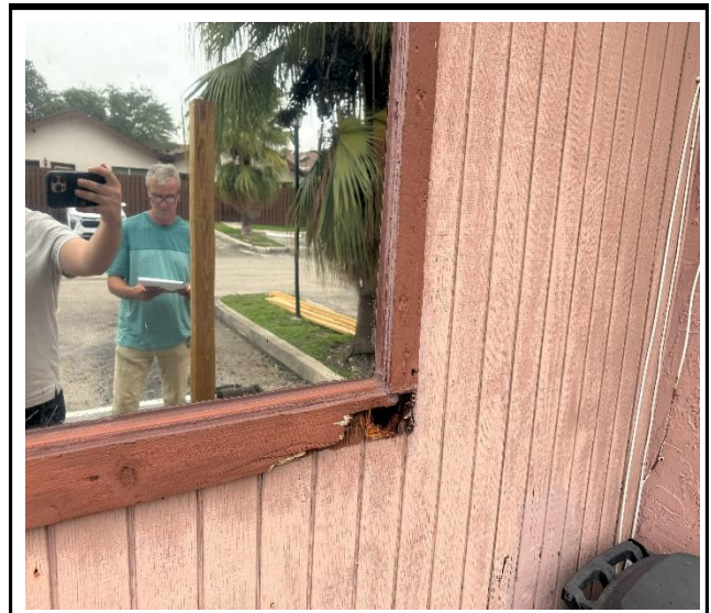
Photo 4 : Existing non-impact-rated window frame
