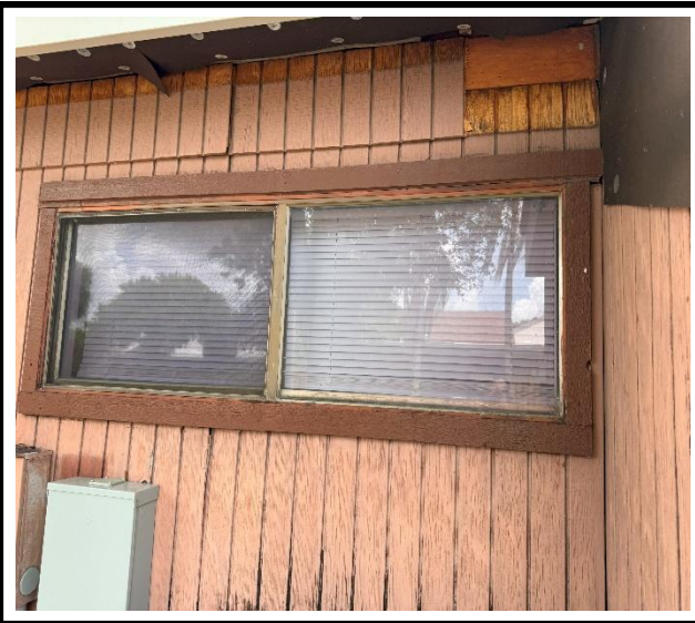
Photo 1 : Existing non-impact-rated window frame
