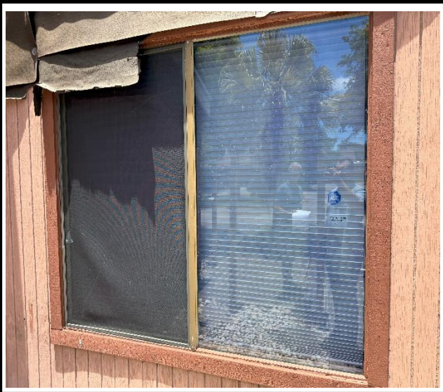
Photo 1 : Existing non-impact-rated window frame
