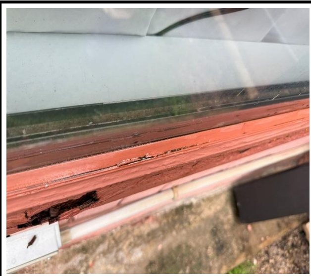
Photo 3 : Existing non-impact-rated window frame
