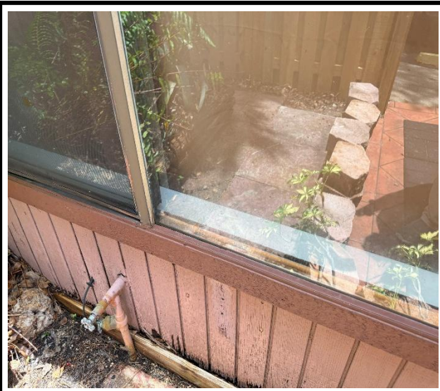
Photo 3 : Existing non-impact-rated window frame
