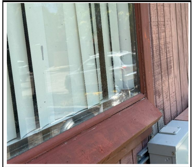
Photo 2 : Existing non-impact-rated window frame
