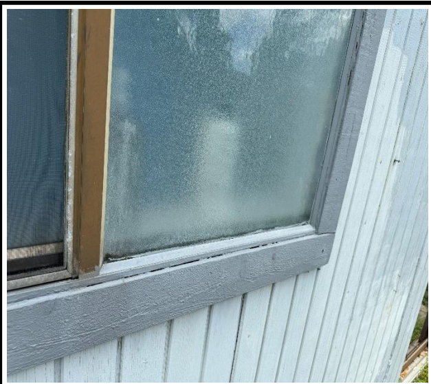
Photo 3 : Existing non-impact-rated window frame
