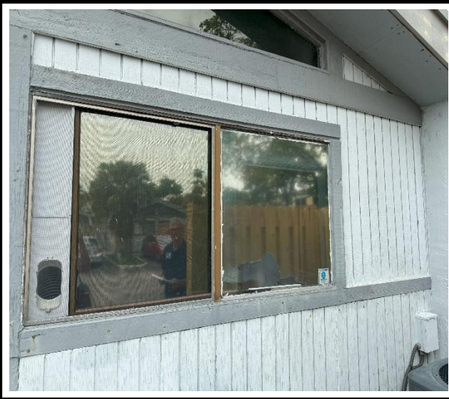
Photo 1 : Existing non-impact-rated window frame
