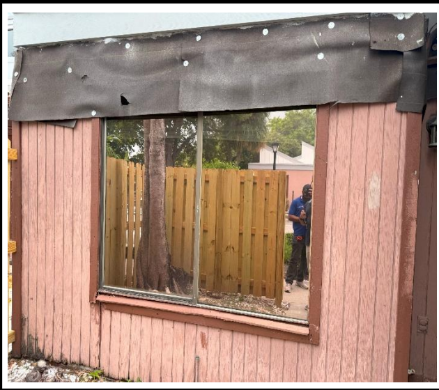
Photo 1 : Existing non-impact-rated window frame
