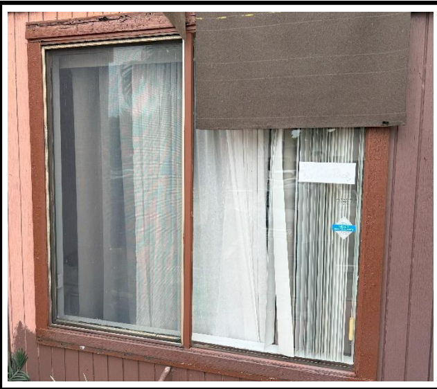
Photo 1 : Existing non-impact-rated window frame
