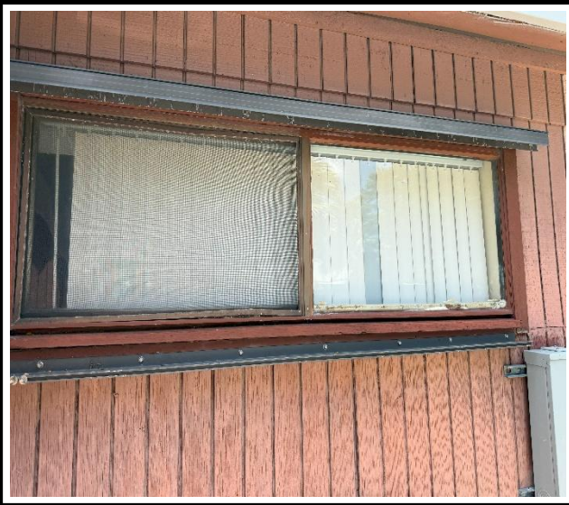
Photo 1 : Existing non-impact-rated window frame
