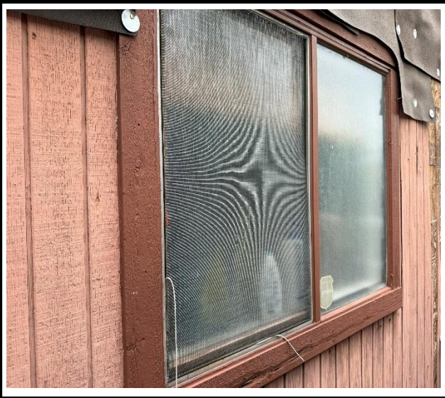
Photo 1 : Existing non-impact-rated window frame
