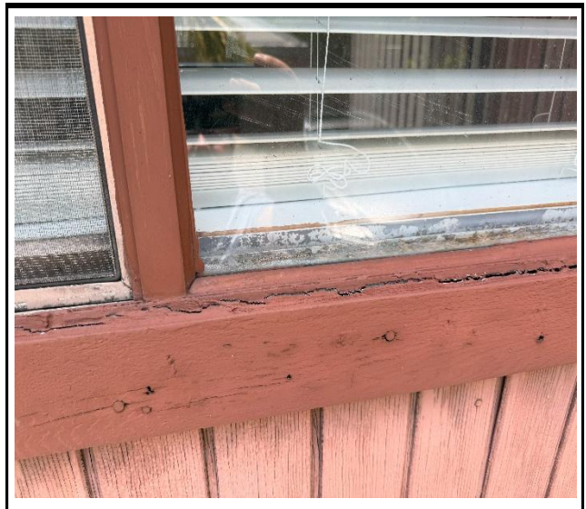
Photo 2 : Existing non-impact-rated window frame
