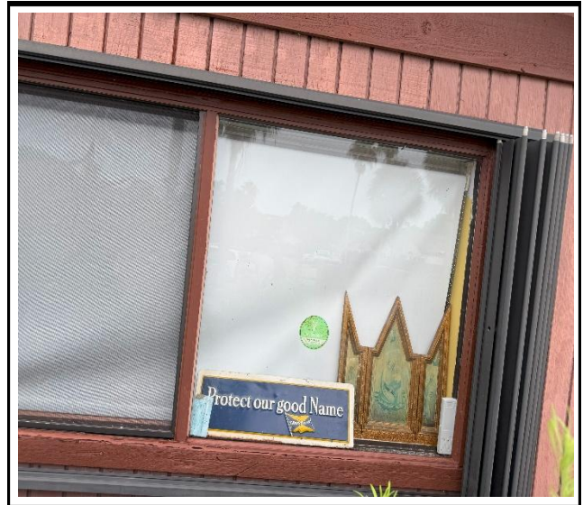
Photo 2 : Existing non-impact-rated window frame
