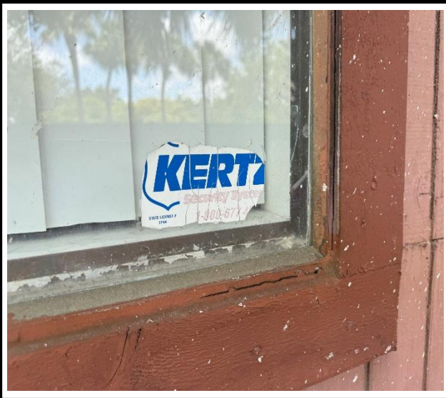
Photo 3 : Existing non-impact-rated window frame
