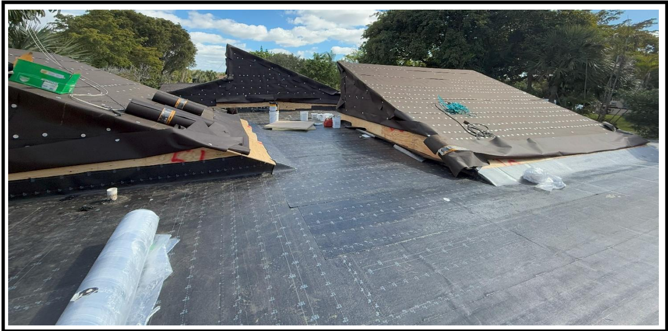
2 – Ongoing, Laying down the waterproof black paper on top of the plywood and adding the tin caps, BLDG 07.
