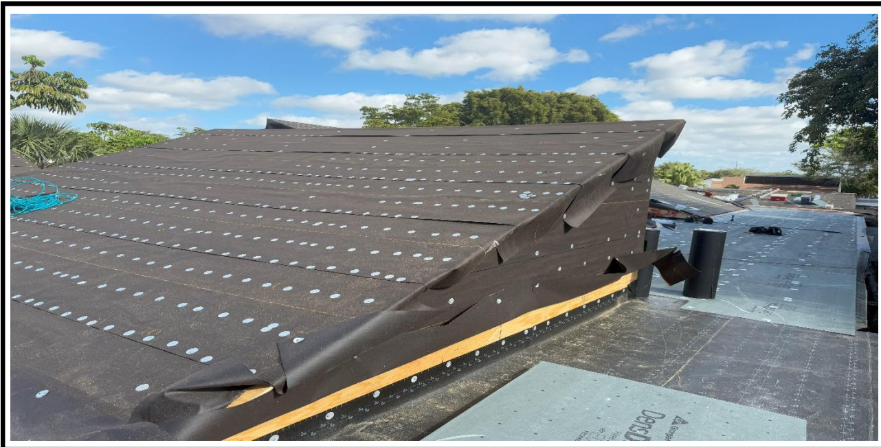
7 – Ongoing, Installation of the new plywood and the waterproof papers, BLDG 07.
