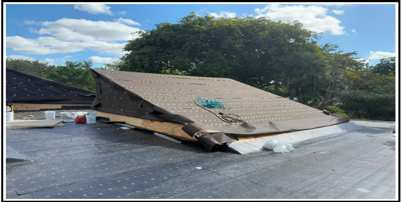
6 – Ongoing, Installation of the new plywood and the waterproof papers, BLDG 07.
