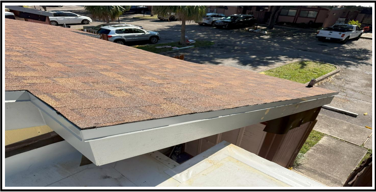
9 – Ongoing, Installation of the new shingles and fascia board, BLDG 02.
