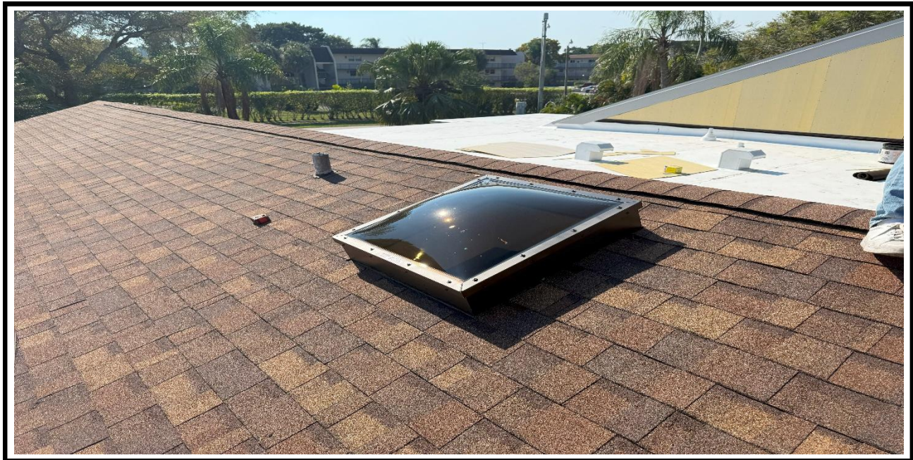
10 – Ongoing, Installation of the new shingles and sun screen, BLDG 02.
