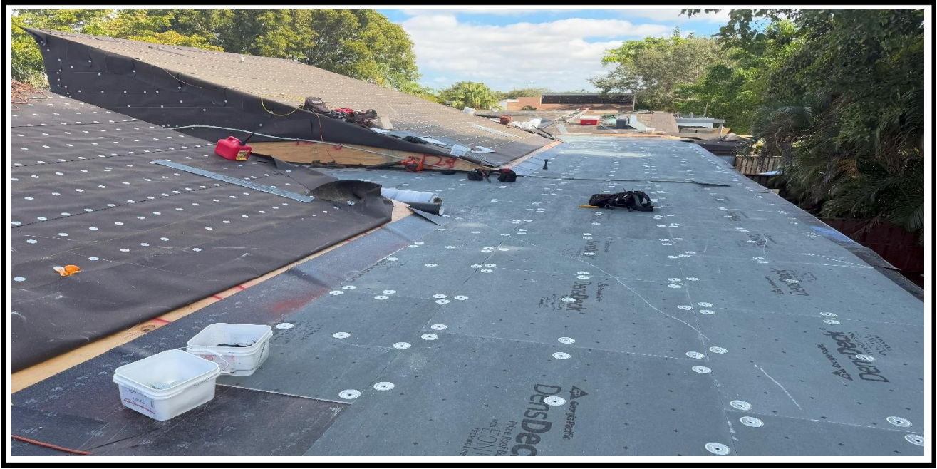
1 – Ongoing, Laying down the insulation sheets on top of the plywood and adding the tin caps, BLDG 07.
