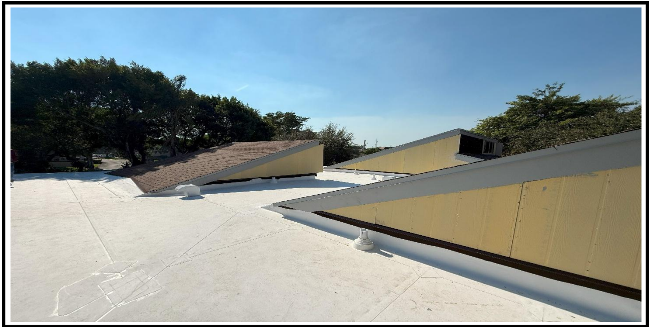
12 – Ongoing, Installation of the new shingles and fascia board, BLDG 02.
