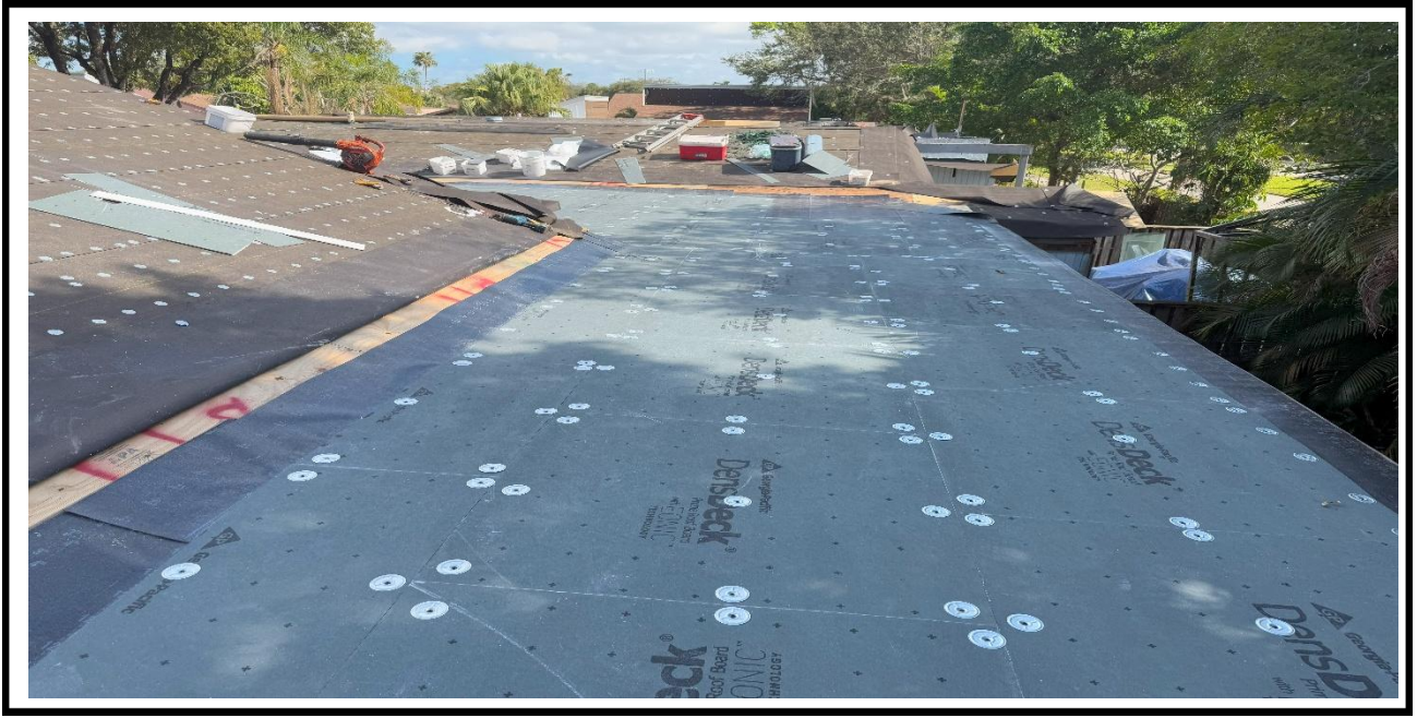
3 – Ongoing, Laying down the insulation sheets on top of the plywood and adding the tin caps, BLDG 07.
