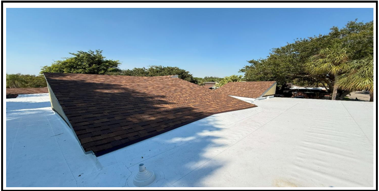
11 – Ongoing, Installation of the new TPO SHEETS, BLDG 02.
