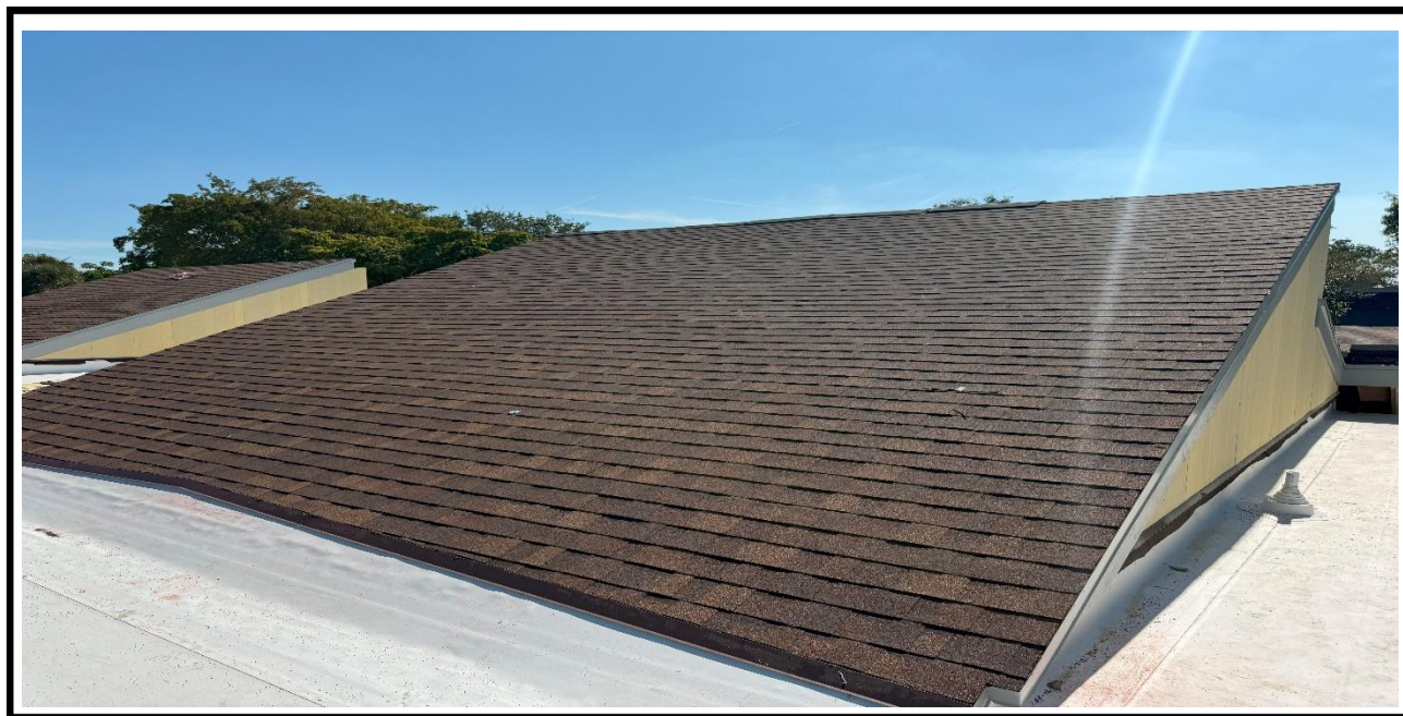
8 – Ongoing, Installation of the new shingles, BLDG 02.
