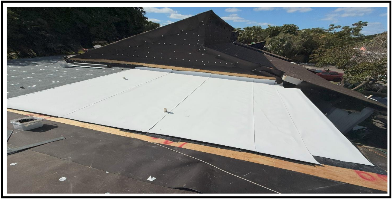
5 – Ongoing, Ongoing, Laying down the TPO Sheets, BLDG 07.
