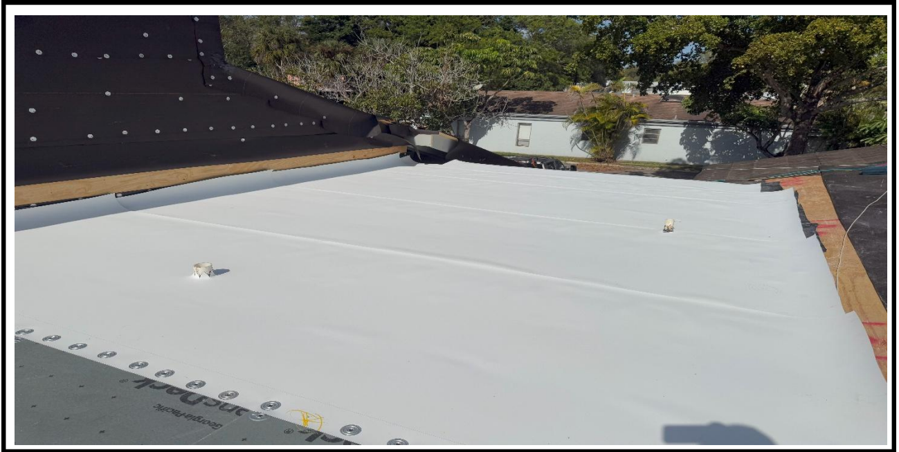
4 – Ongoing, Laying down the TPO Sheets, BLDG 07.
