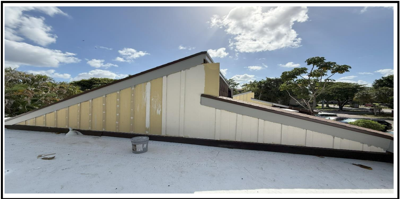
2 – Ongoing, Application of the first coat of the paint at Hardie Board, BLDG 06.
