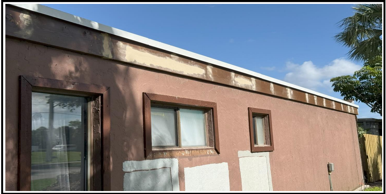
6 – Ongoing, Application Wood Filler Material at the Fascia Board, BLDG 6.
