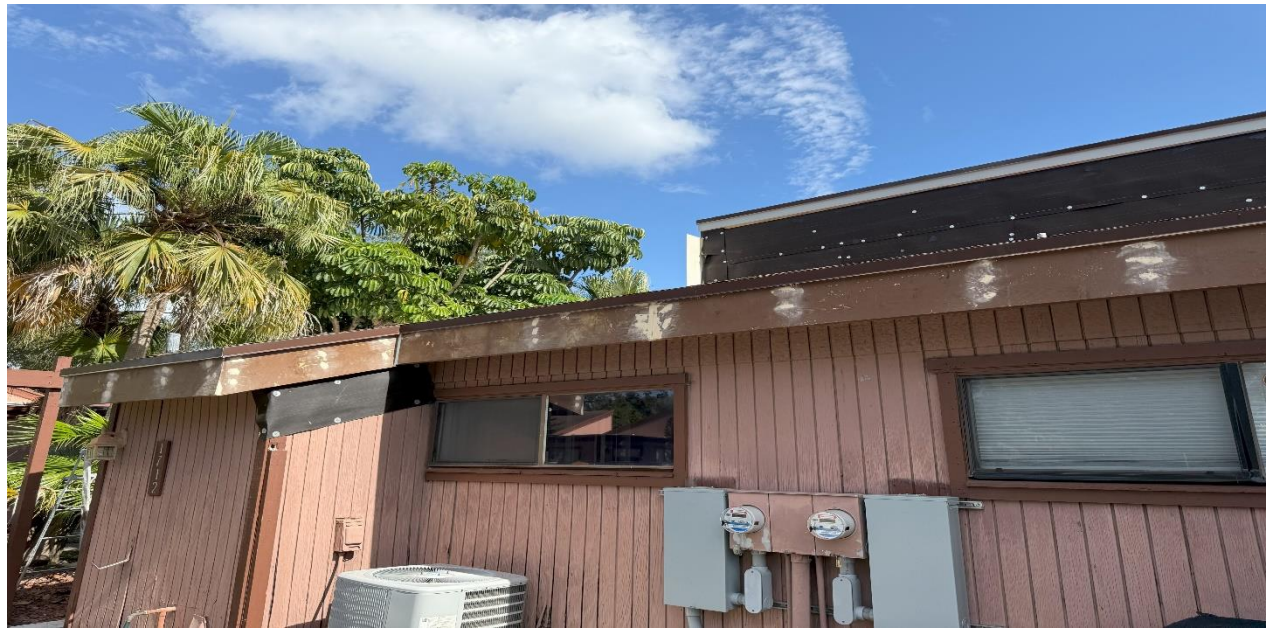
7 – Ongoing, Application Wood Filler Material at the Fascia Board, BLDG 6.
