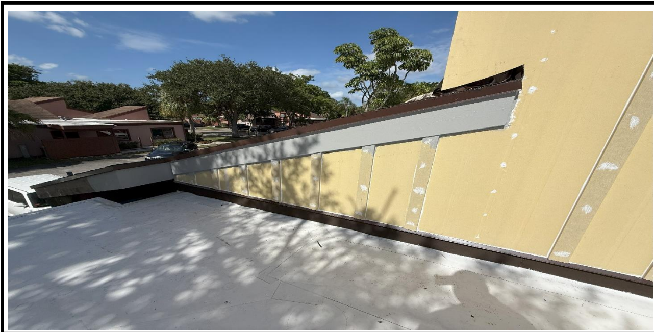
9 – Ongoing, Application of the Caulking Material at the Hardie Board, BLDG 6.
