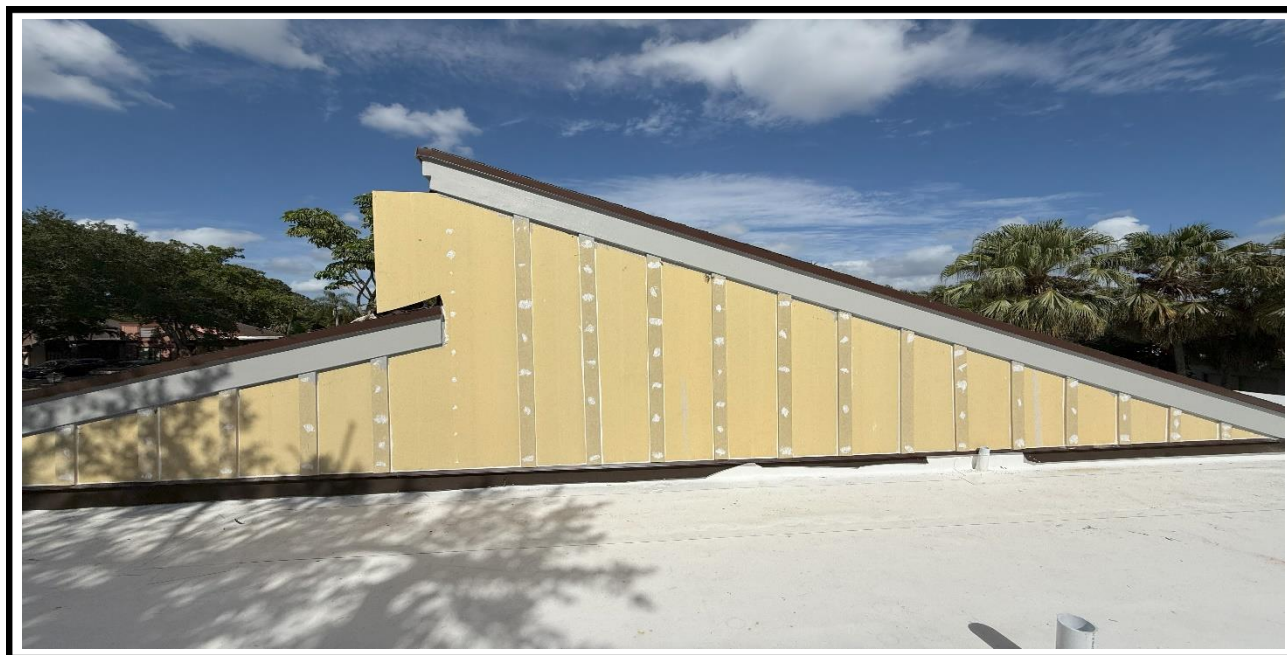
10 – Ongoing, Application of the Caulking Material at the Hardie Board, BLDG 6.
