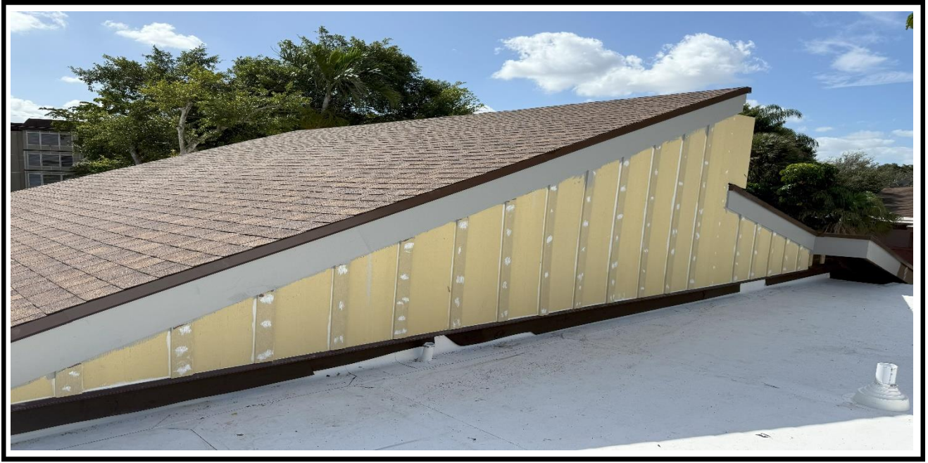
1 – Ongoing, Application of the caulking material at Hardie Board / Paint of fascia board, BLDG 06.
