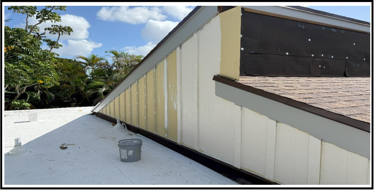
5 – Ongoing, Painting of the Hardie Board and Fascia Board, BLDG 06.
