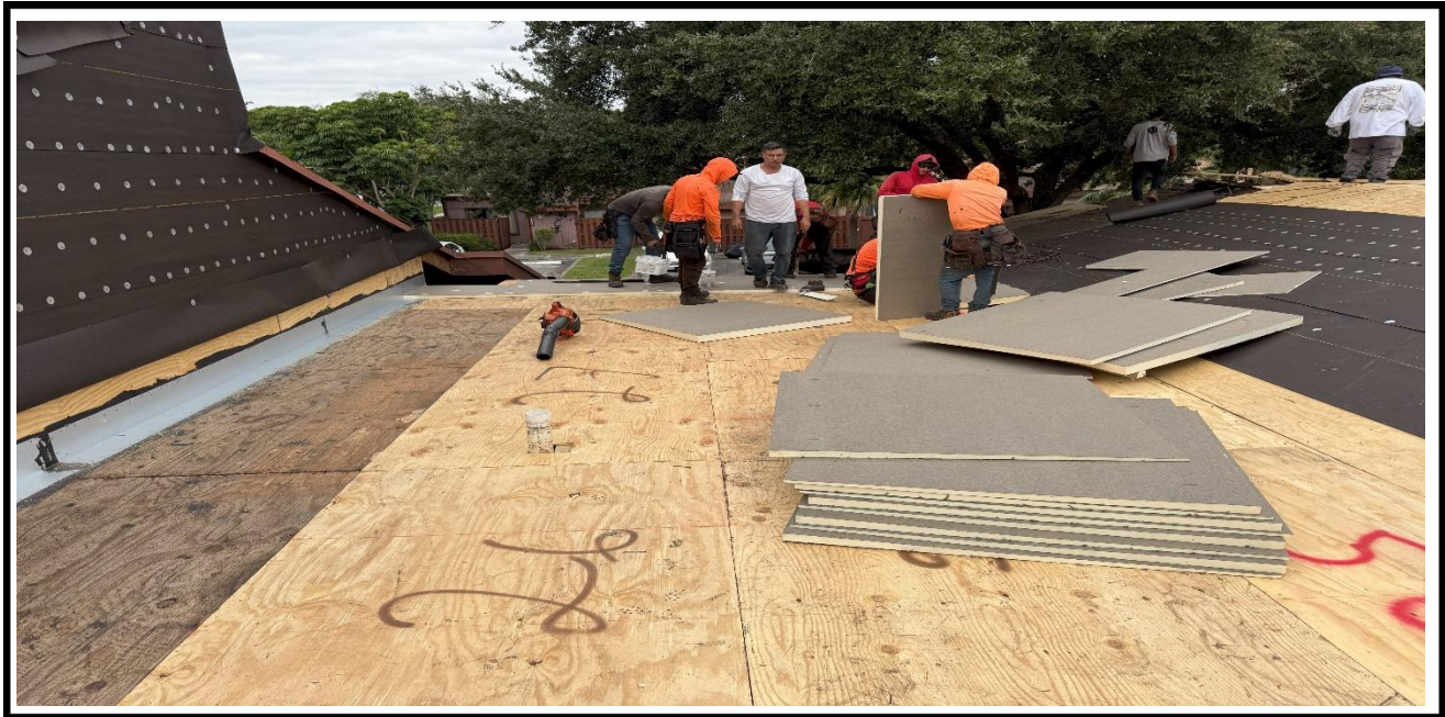
2 – Ongoing, Installation of the new plywood and insulation sheets, BLDG 01.
