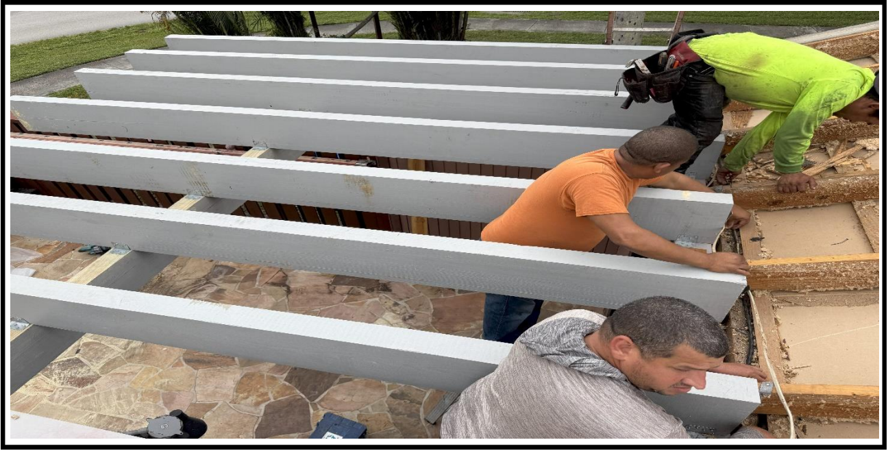
5 – Ongoing, Installation of the new wood beams after removal of the damaged beams, BLDG 01.
