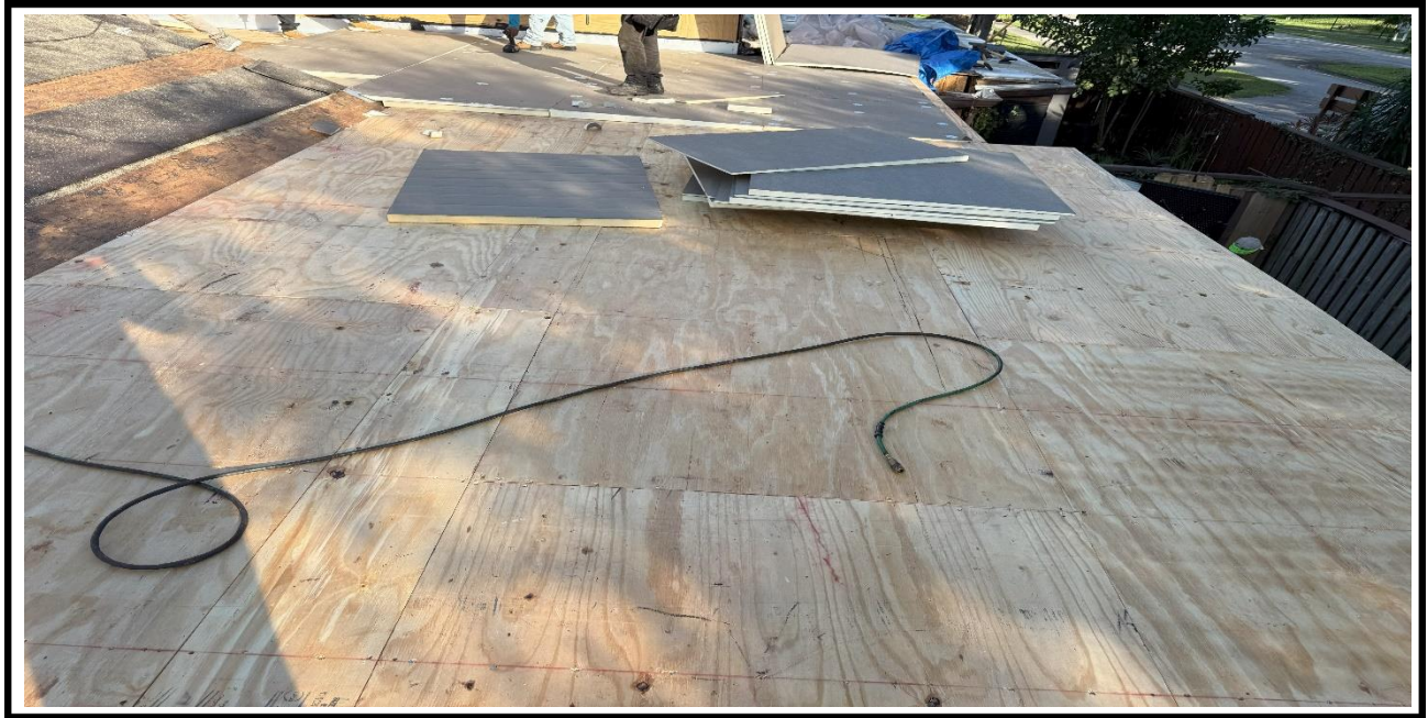
12 – Ongoing, Installation of new plywood on top of the roof, BLDG 01.
