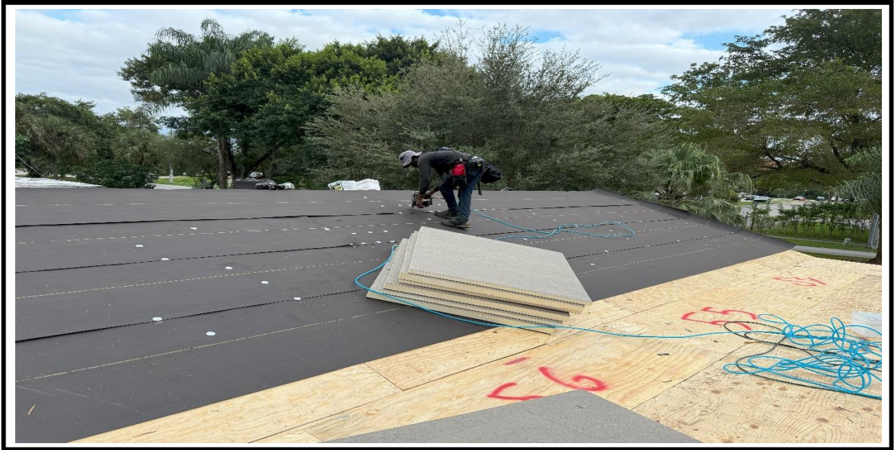
4 – Ongoing, Laying down the waterproof black paper on top of the plywood and adding the tin caps, BLDG 01.
