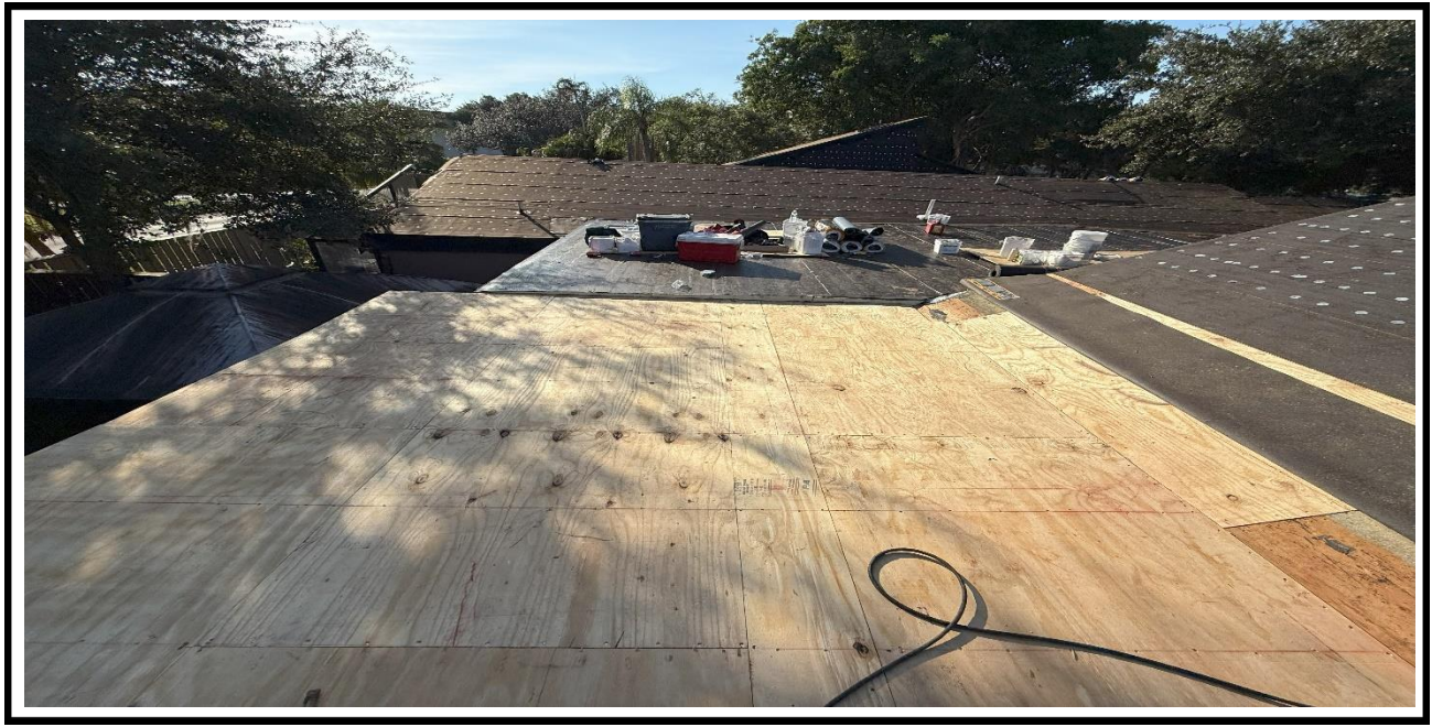
11 – Ongoing, Installation of new plywood on top of the roof, BLDG 01.
