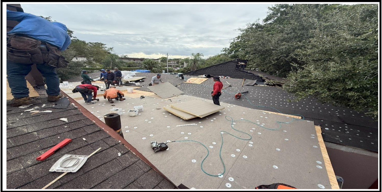
6 – Ongoing, Installation of the new insulation sheets on top of the plywood, BLDG 01.
