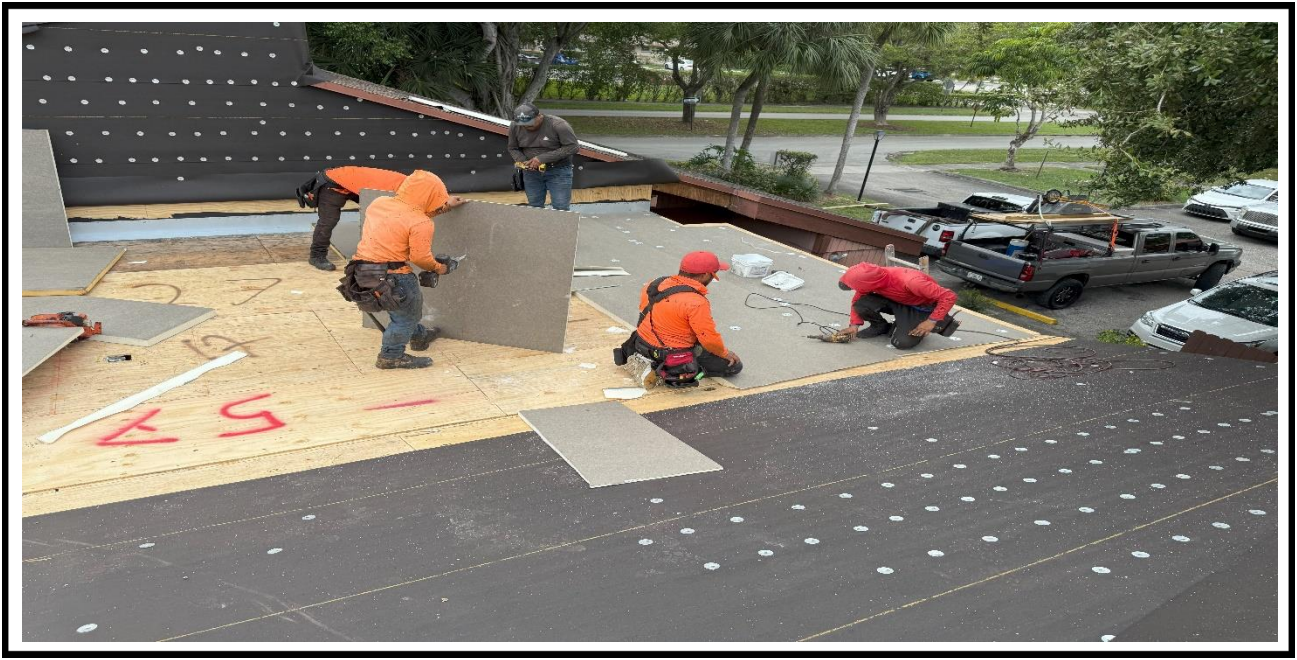
3 – Ongoing, Installation of the isolation sheets on top of the plywood and adding the tin caps, BLDG 01.
