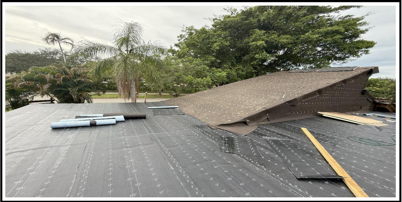
8 – Ongoing, Laying down the waterproof black papers on top of the plywood, BLDG 01.
