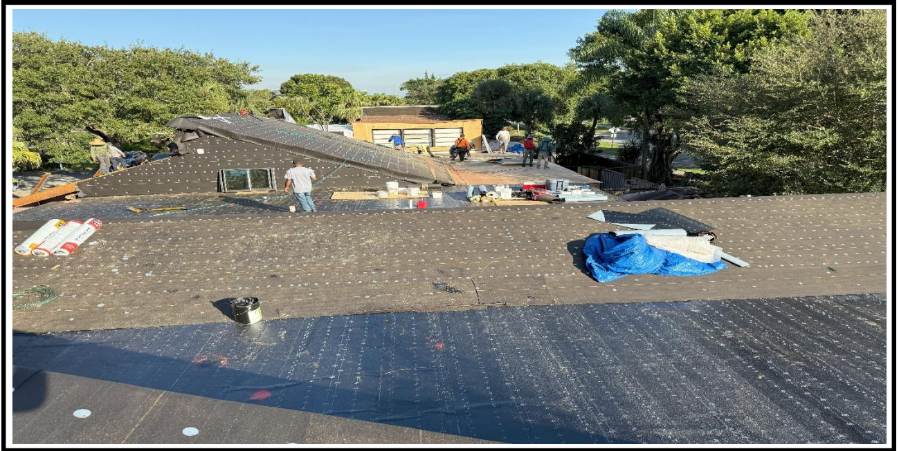
10 – Ongoing, Laying down the waterproof black papers on top of the plywood, BLDG 01.
