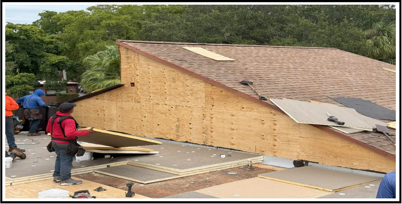
7 – Ongoing, Installation of the new plywood at the vertical sides of the building, BLDG 01.
