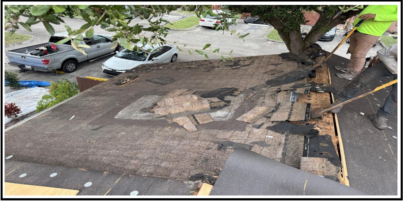
1 – Ongoing, Removal of the existing shingles on top of the roof, BLDG 01.
