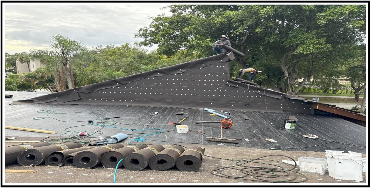
9 – Ongoing, Laying down the waterproof black papers on top of the plywood, BLDG 01.
