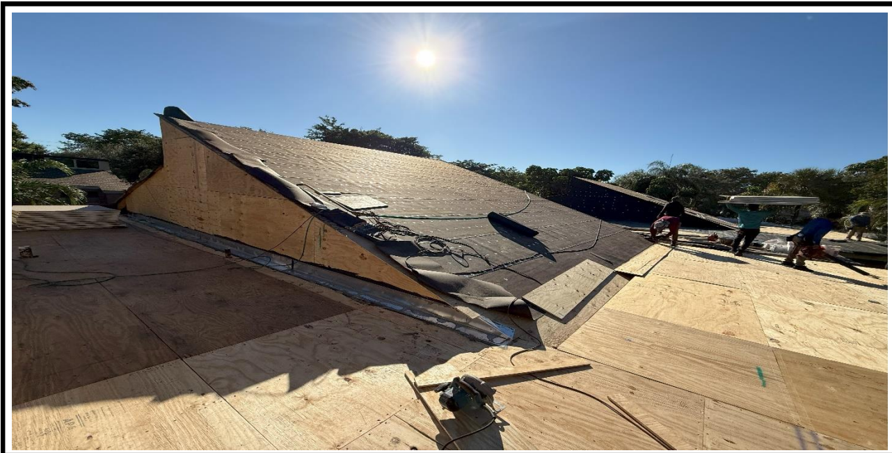
7 – Ongoing, Installation of the new plywood at the vertical sides of the building, BLDG 02.
