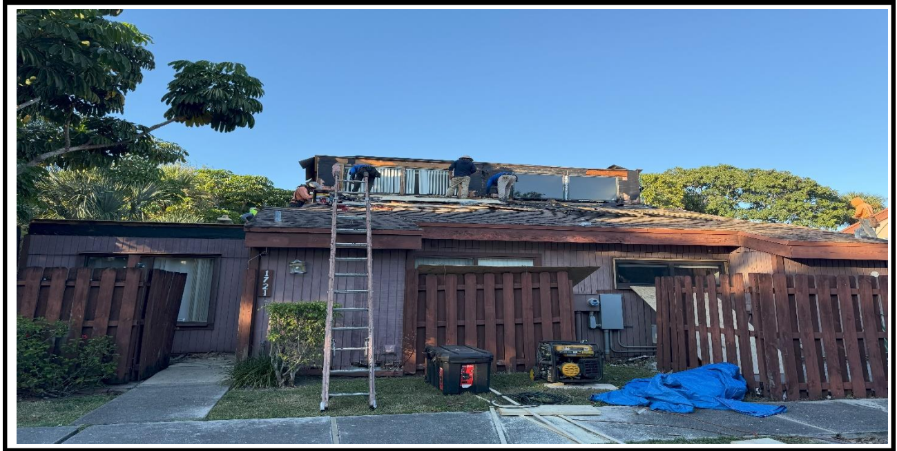
6 – Ongoing, Removal of the old roofing shingles and Hardie boards, BLDG 02.
