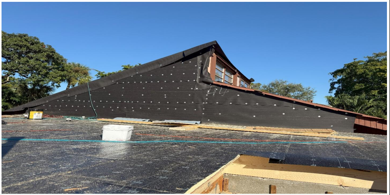
12 – Ongoing, Laying down the waterproof black paper on top of the plywood and adding the tin caps, BLDG 01.
