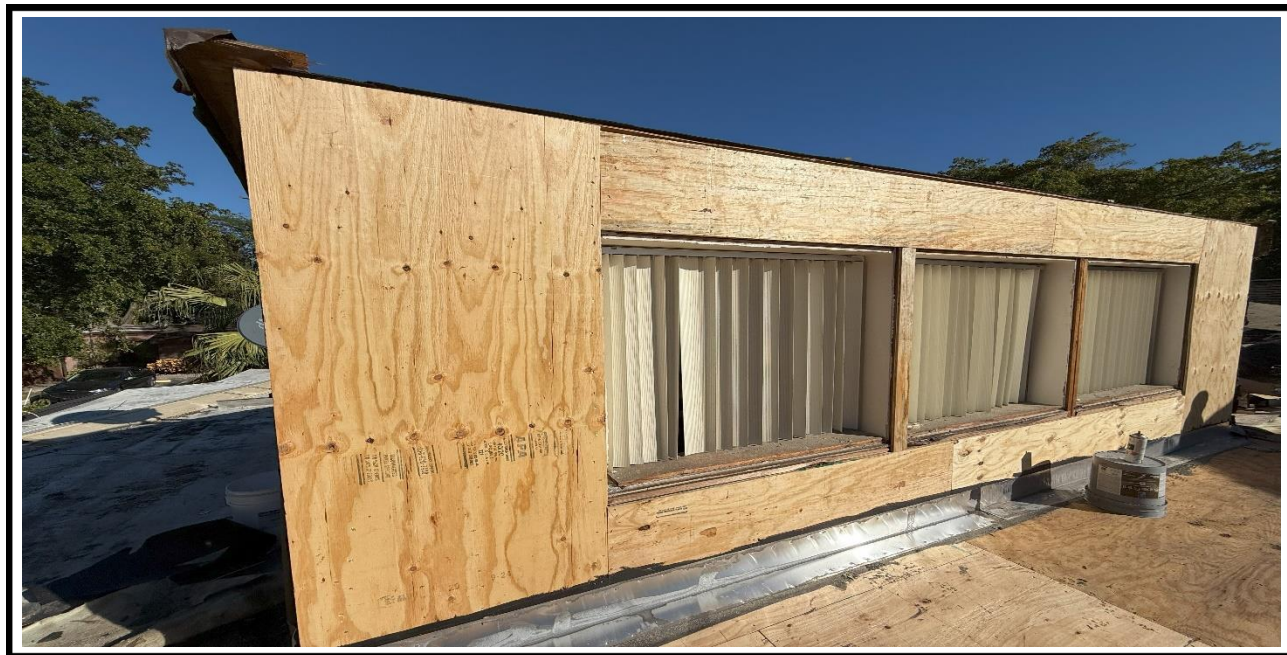
8 – Ongoing, Installation of the new plywood at the vertical sides of the building, BLDG 02.
