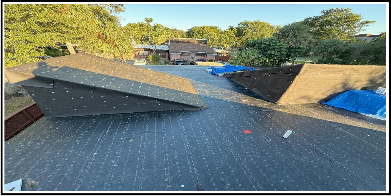
1 – Ongoing, Laying down the waterproof black paper on top of the plywood and adding the tin caps, BLDG 01.
