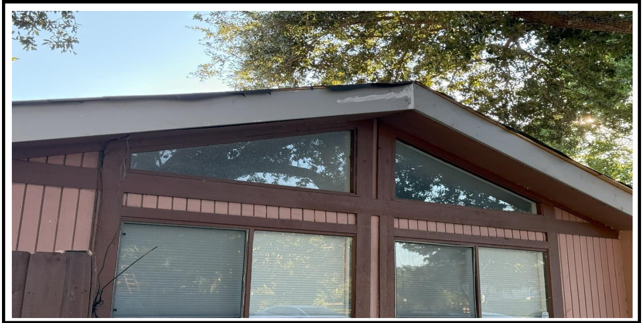
4 – Ongoing, Installation of the new fascia boards, BLDG 01.
