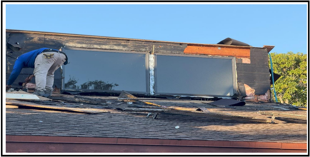
5 – Ongoing, Removal of the old roofing shingles and Hardie boards, BLDG 02.
