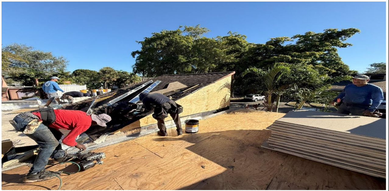
11 – Ongoing, Installation of the new insulation sheets and new plywood at the building, BLDG 02.
