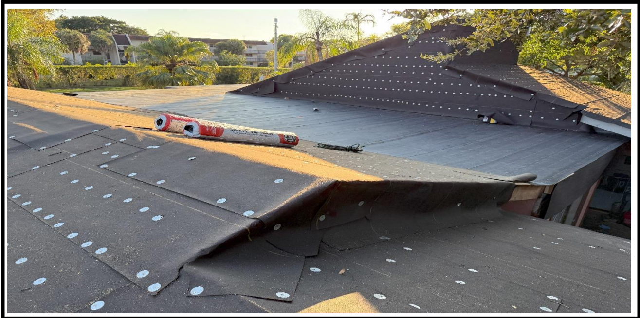
2 – Ongoing, Laying down the waterproof black paper on top of the plywood and adding the tin caps, BLDG 01.
