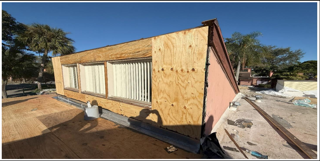
10 – Ongoing, Removal of the old roofing shingles and Hardie boards, BLDG 02.
