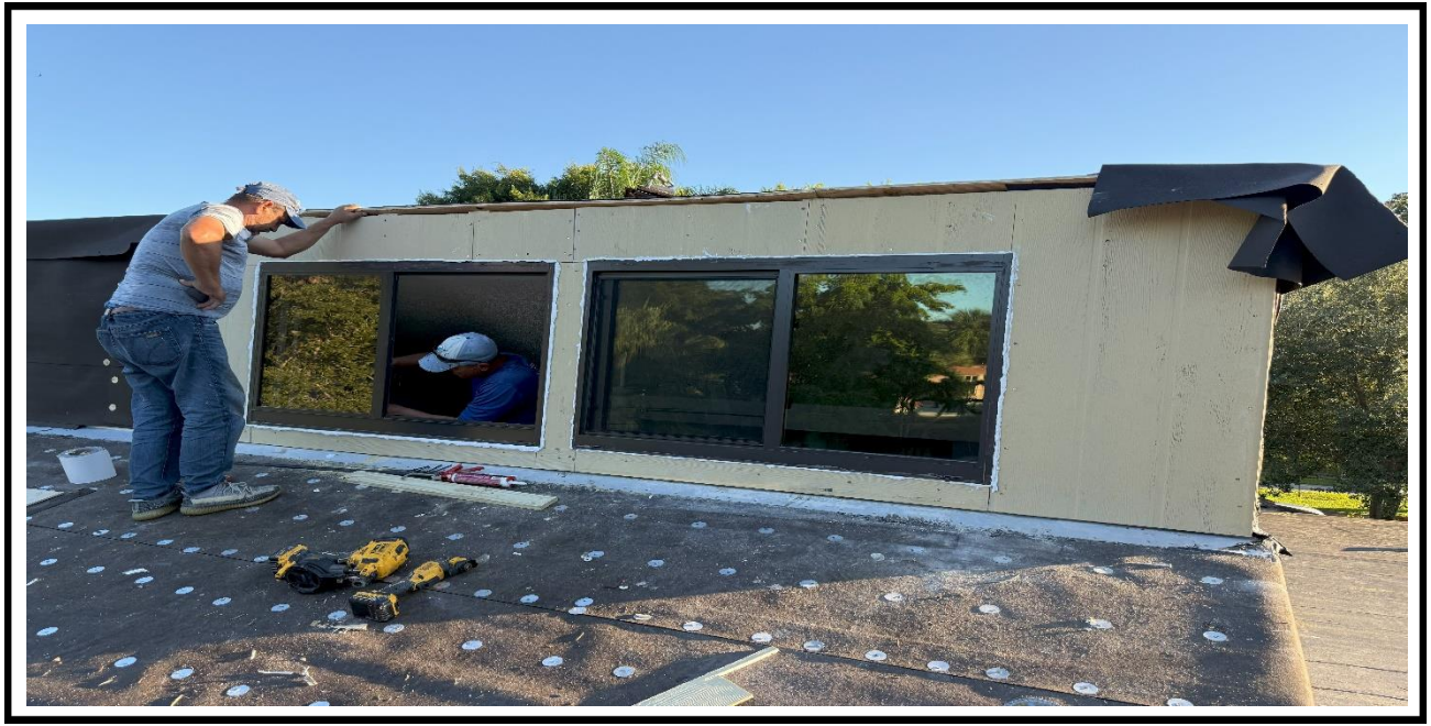
3 – Ongoing, Re-installation of the existing, good condition window, BLDG 01.
