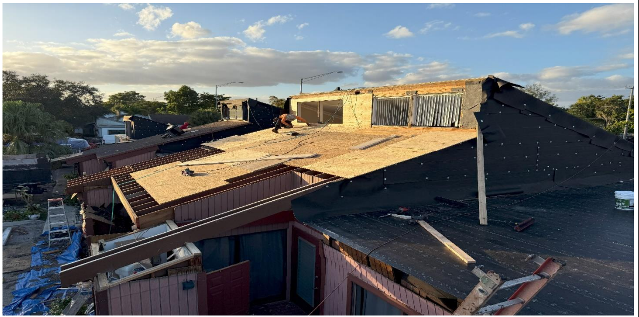
11 – Ongoing, Installation of the new insulation sheets and new plywood at the building, BLDG 15.
