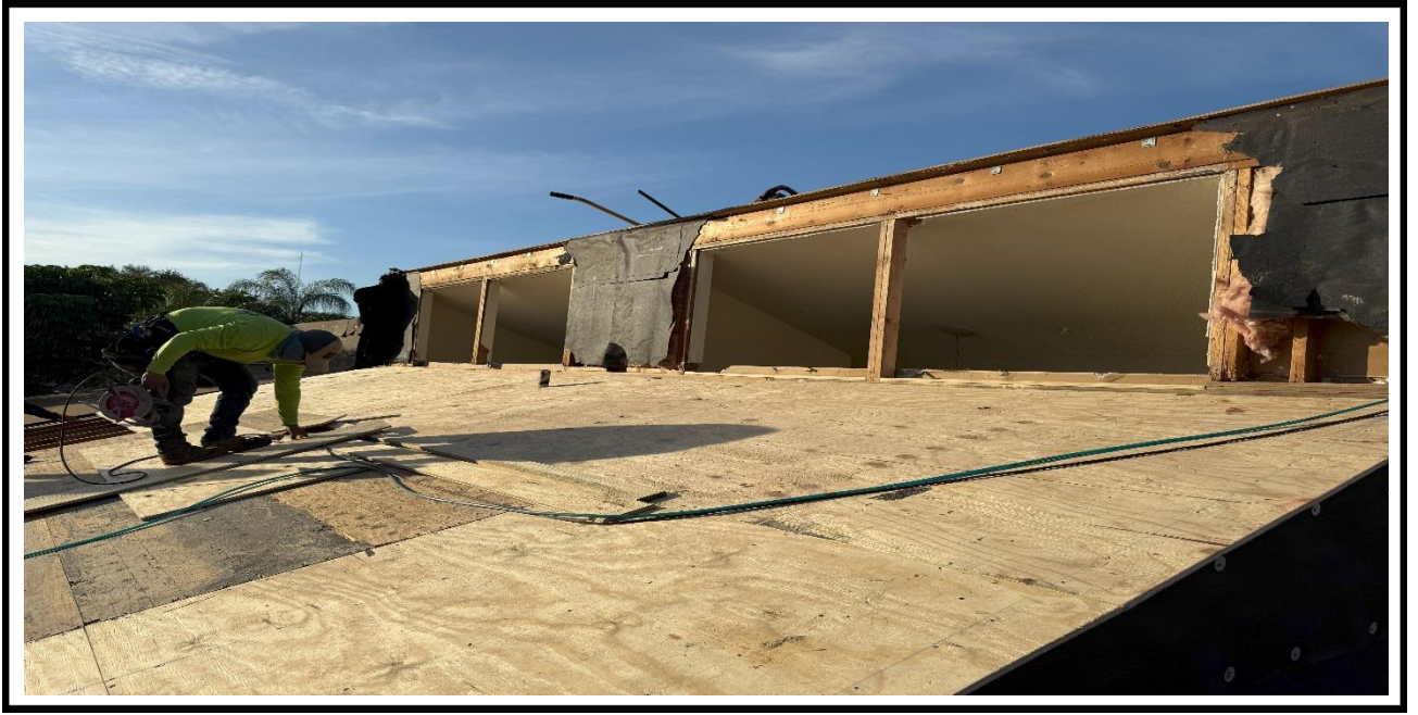
3 – Ongoing, Installation of the new plywood, BLDG 02.
