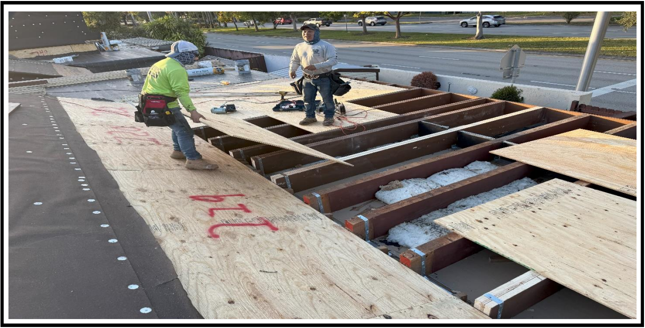
9 – Ongoing, Installation of the new plywood and wood beams, BLDG 15.
