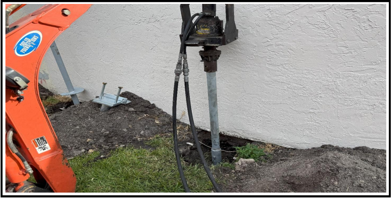
13 – Ongoing, Installation of the helical piles, BLDG 20.
