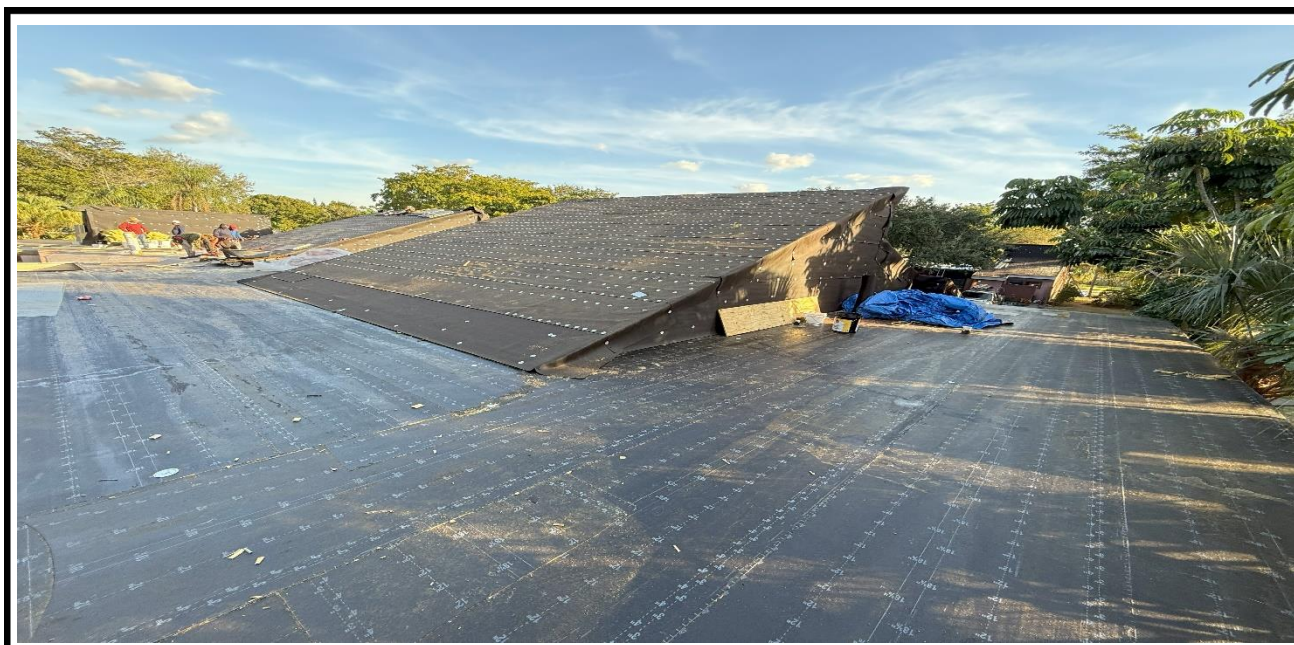
2 – Ongoing, Laying down the waterproof black paper on top of the plywood and adding the tin caps, BLDG 02.
