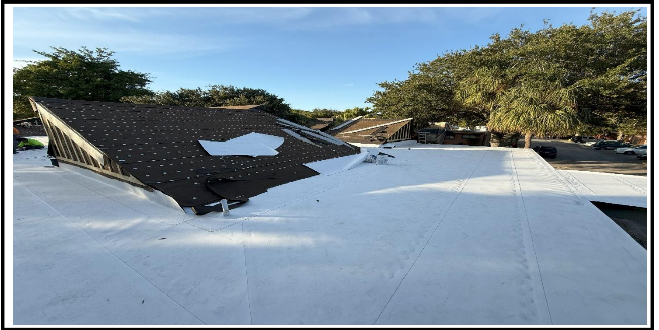
4 – Ongoing, Laying down the TPO Sheets, BLDG 02.
