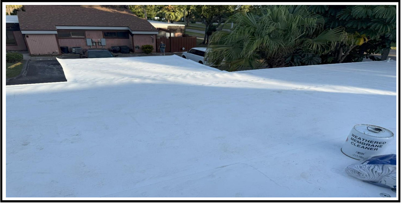
5 – Ongoing, Ongoing, Laying down the TPO Sheets, BLDG 01.
