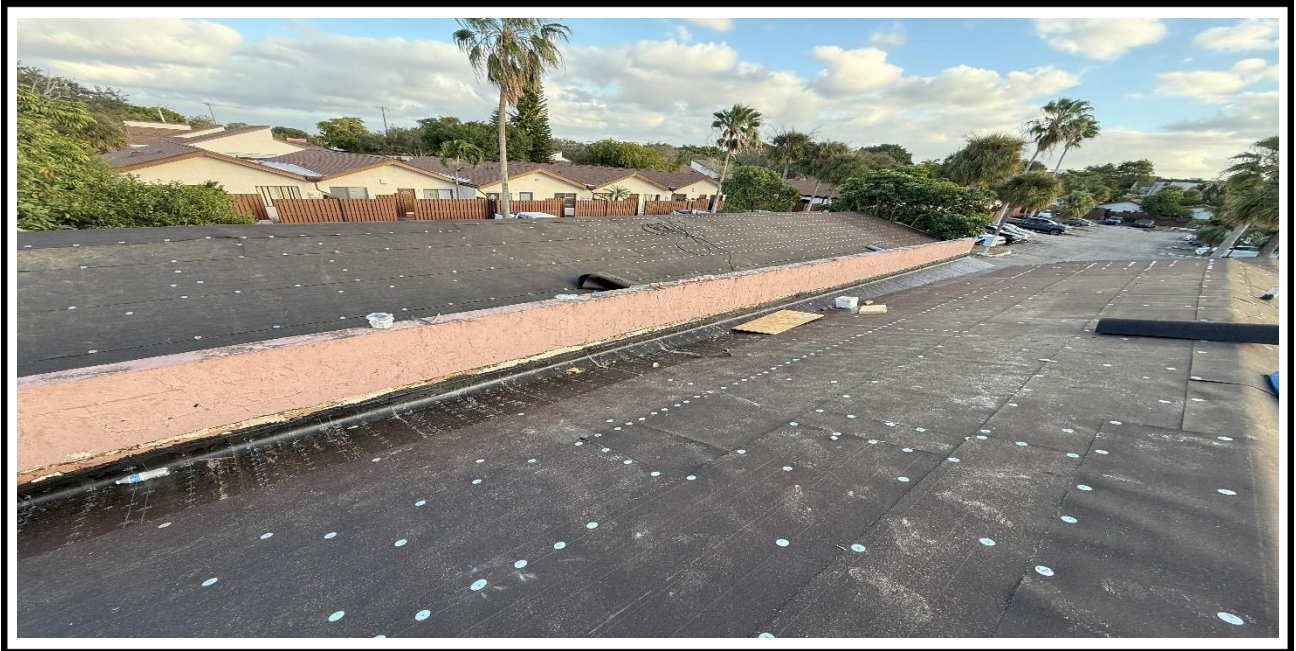
10 – Ongoing, Laying down the insulation sheets on top of the plywood and adding the tin caps, BLDG 15.
