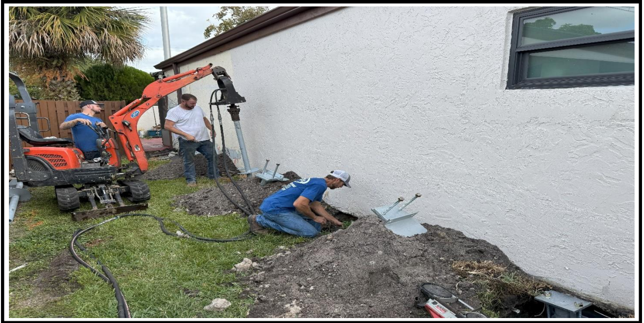
14 – Ongoing, Ongoing, Installation of the helical piles, BLDG 20.
