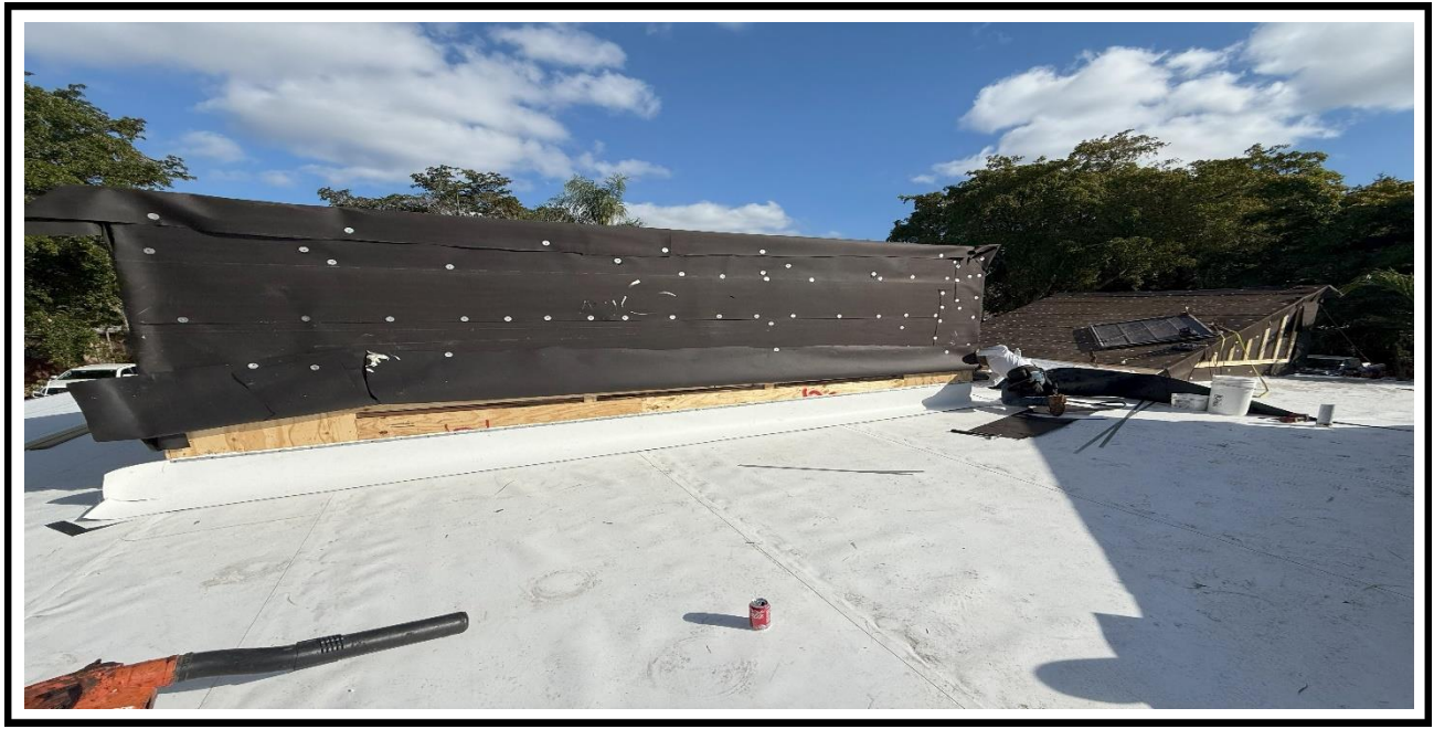
7 – Ongoing, Laying down the TPO Sheets at the vertical sides of the building, BLDG 02.
