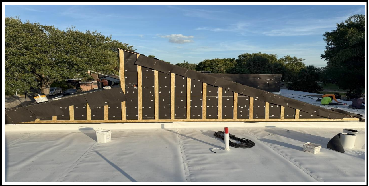
6 – Ongoing, Installation of the Hardie board strips on top of the waterproof papers, BLDG 02.
