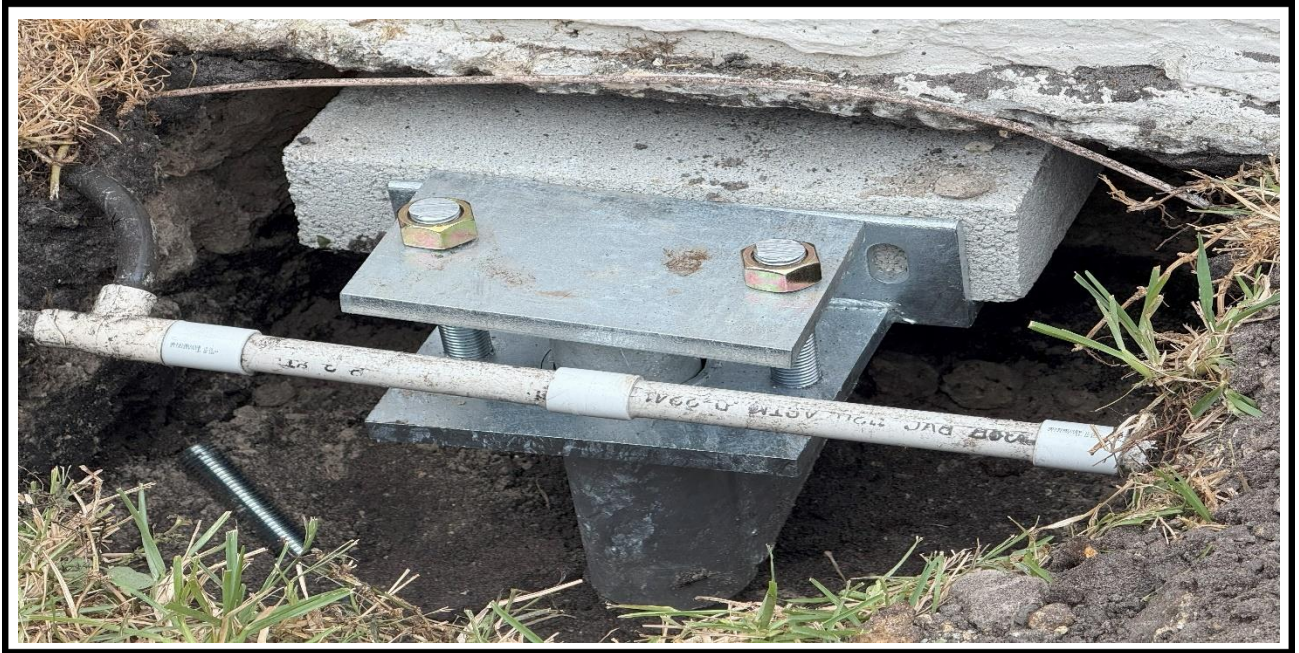
16 – Ongoing, Ongoing, Installation of the helical piles, BLDG 20.
