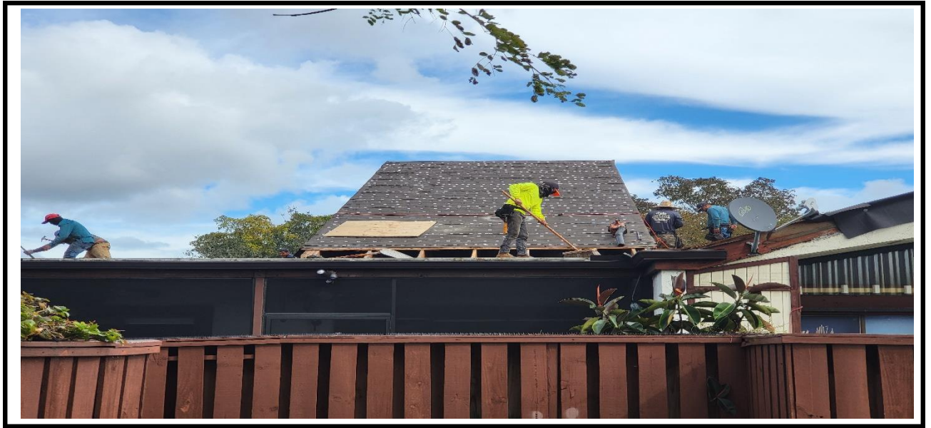
1 – Observed lay out of black papers after changing of deteriorated plywood
