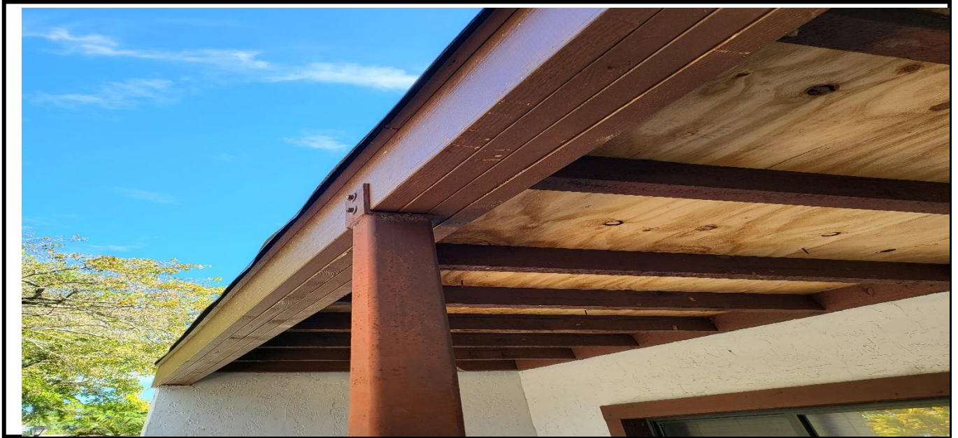
7 – Observed replacing of old deteriorated wood
