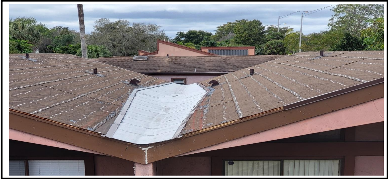
7 – Observed the ongoing work of slope correction
