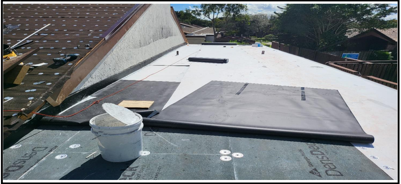
3 – Observed lay out of TPO sheets
