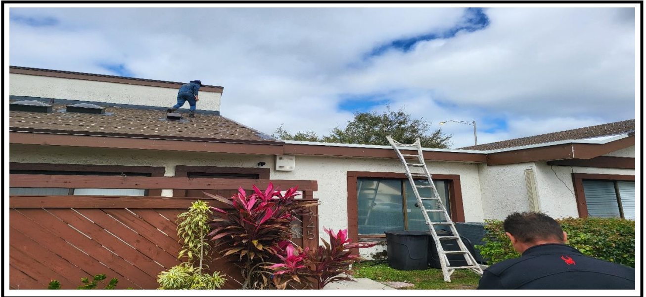
6 – Observed installing of drip edges
