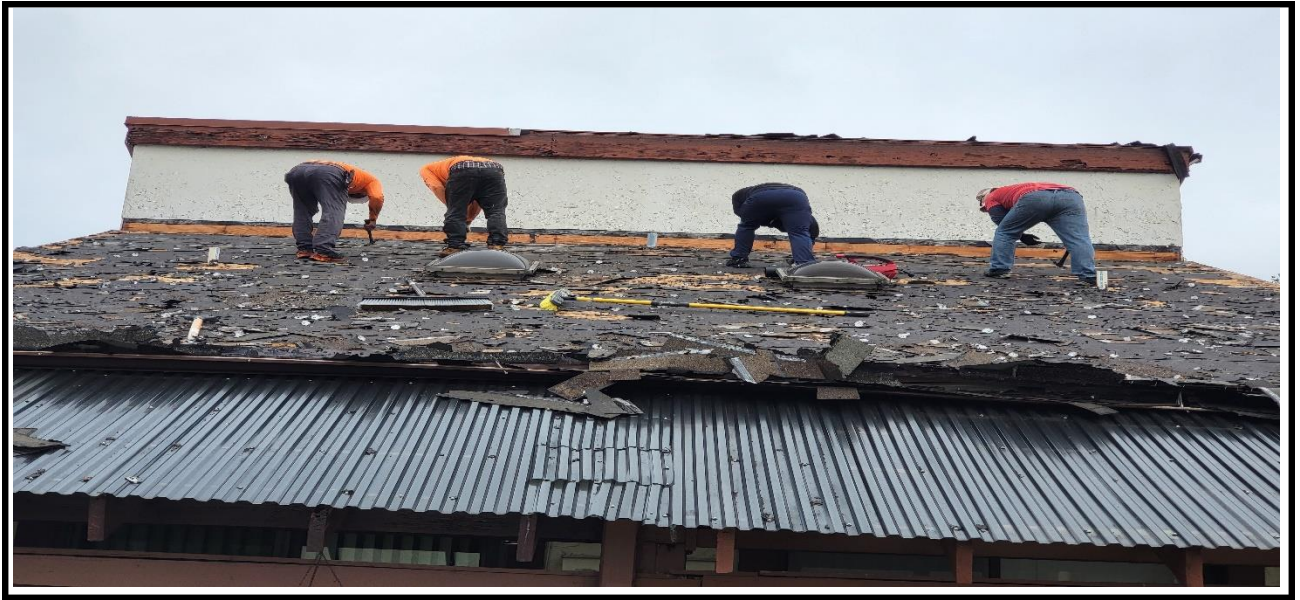
1 – Observed the removal of old roofing material, Shingles, and old black papers
