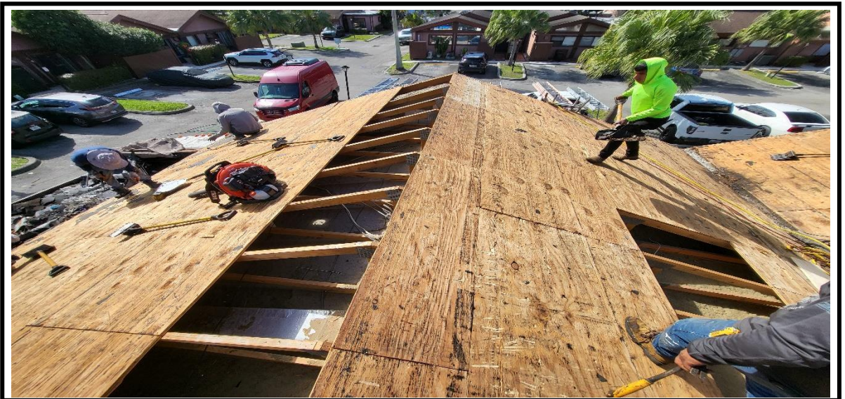
6 – Observed removal of the deteriorated plywood and check of roofing system
