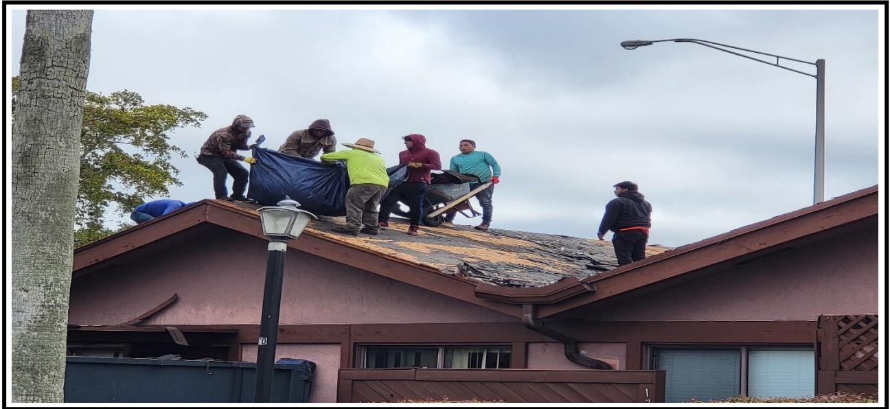
3 – Debris removal on top of roof.
