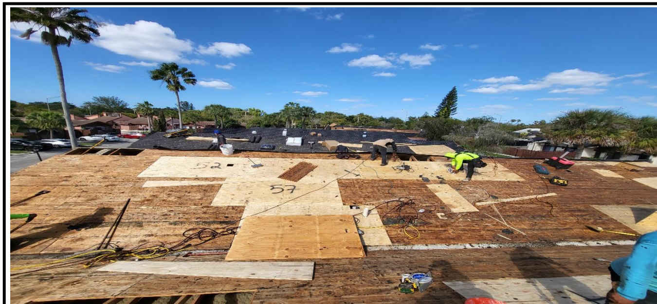
7 – Observed replacing of old deteriorated plywood
