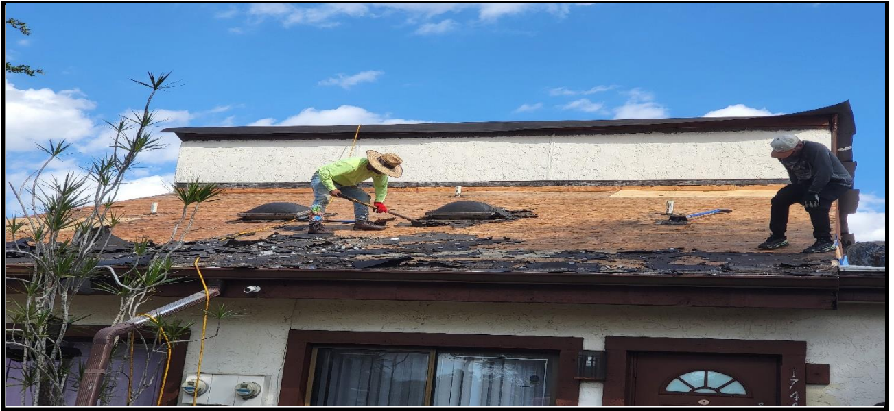
1 – Observed removal of of black papers, skylights, vents and fascia board
