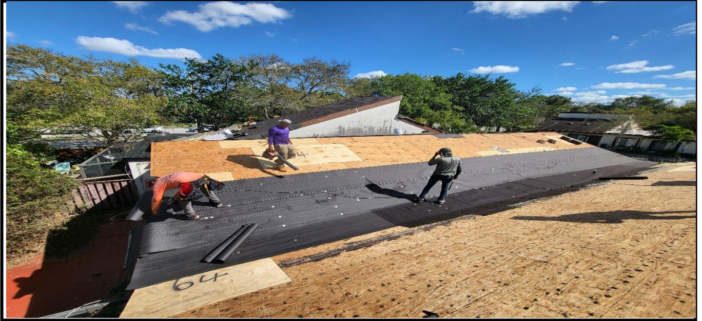
7 – Observed laydown of black papers on top of plywood
