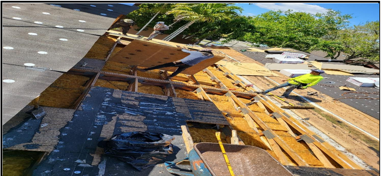
6 – Observed ongoing removal of old plywood
