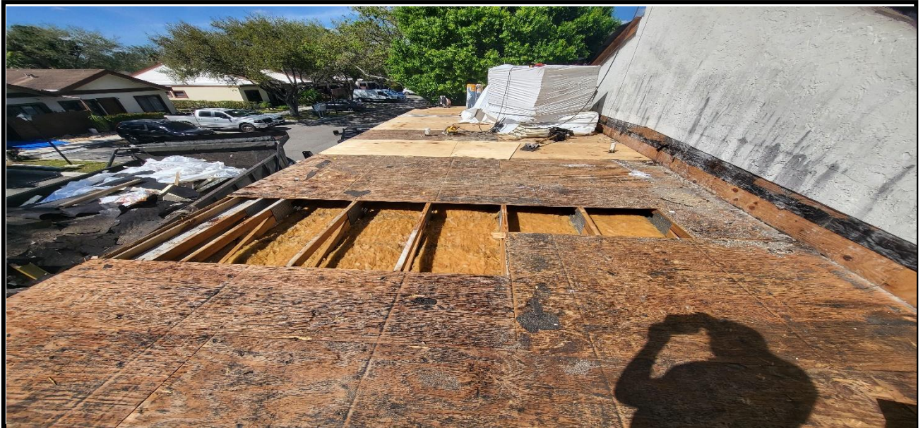
5 – Observed ongoing removal of old plywood
