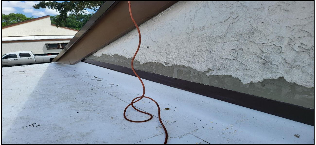
3 – Observed installation of counter flashing, fascia board and drip edges
