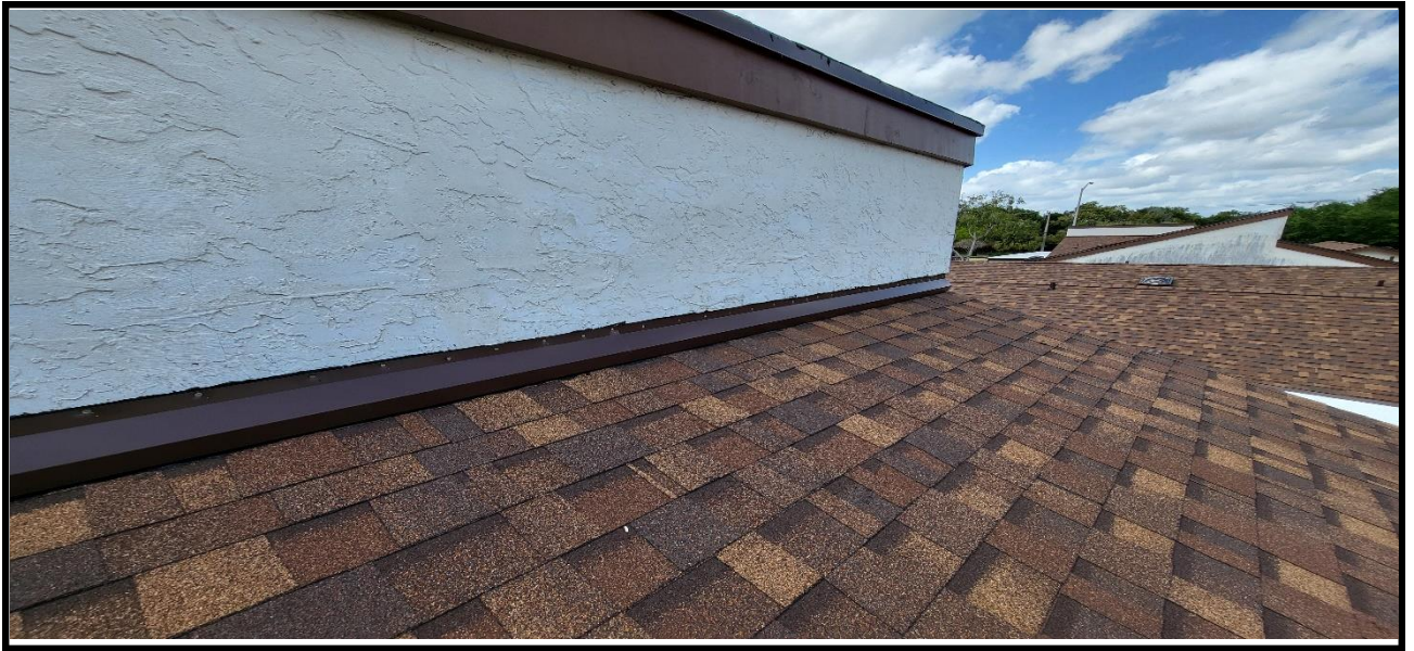
1 – Ongoing installation of counter flashing and stucco work
