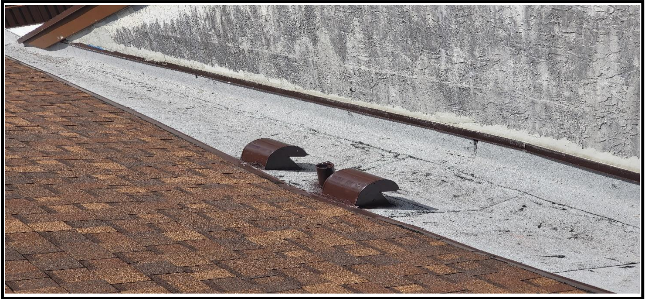
5 – Observed ongoing installation of vents, flashing and stucco work
