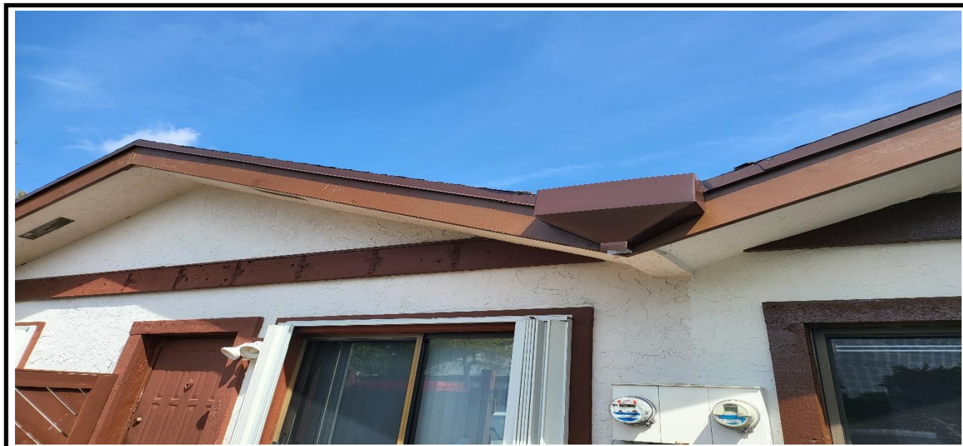
7 – Observed ongoing installation of fascia board and water collection system
