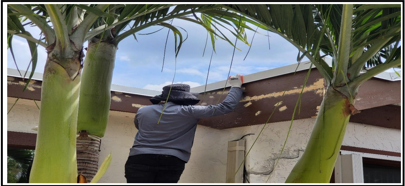
3 – Ongoing application of the wood filler material at fascia board
