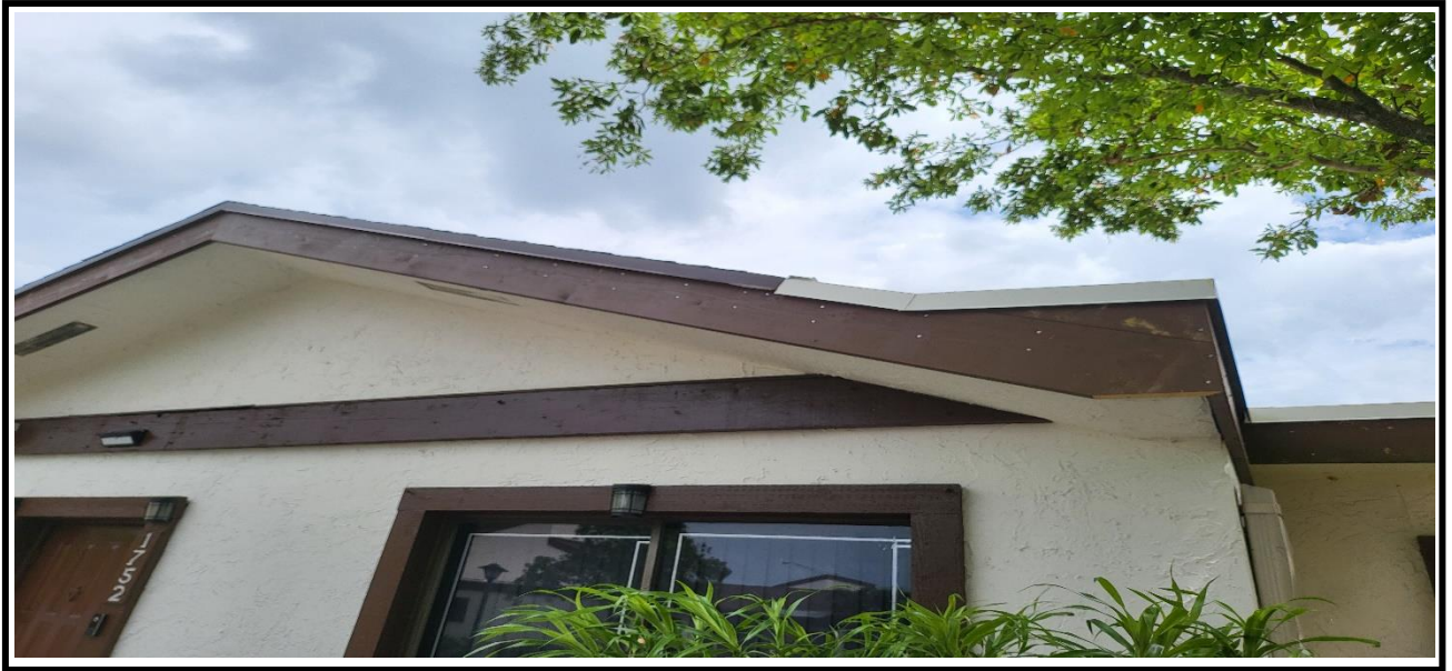
5 – Observed, ongoing, installation of drip edges and fascia board
