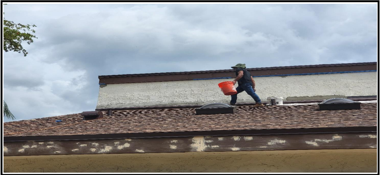
1 – Ongoing installation of counter flashing and stucco repair
