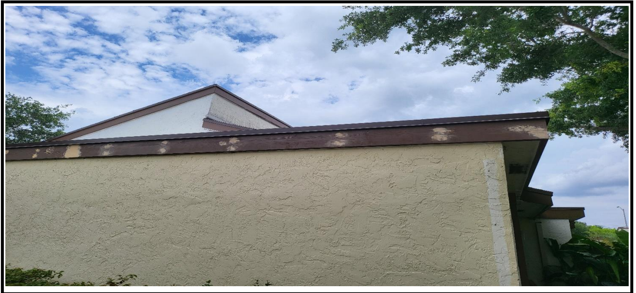
6 – Application of wood filler material at fascia board
