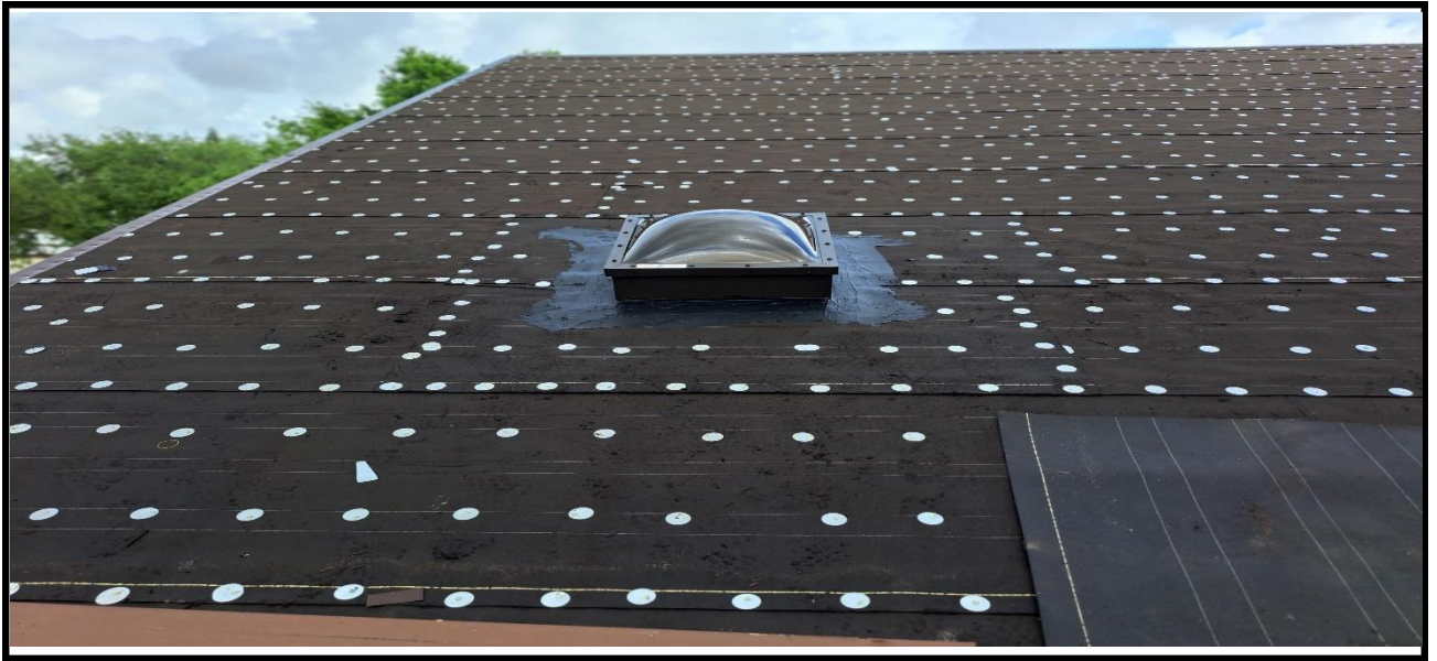
1 – Observed installation of black papers, skylights
