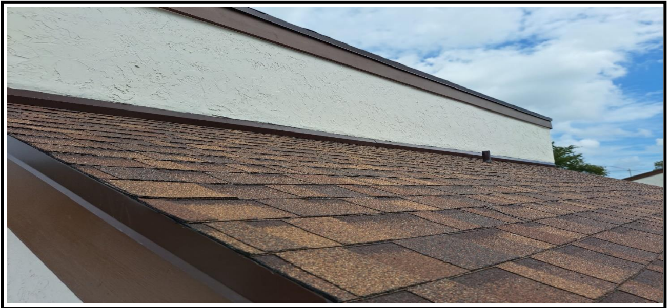
6 – Observed installing of roof shingles and fascia board
