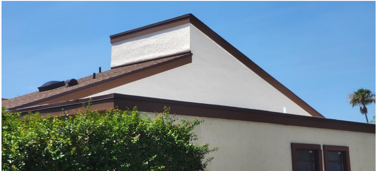
6 – After the application of the paint at sidewalls and fascia board.
