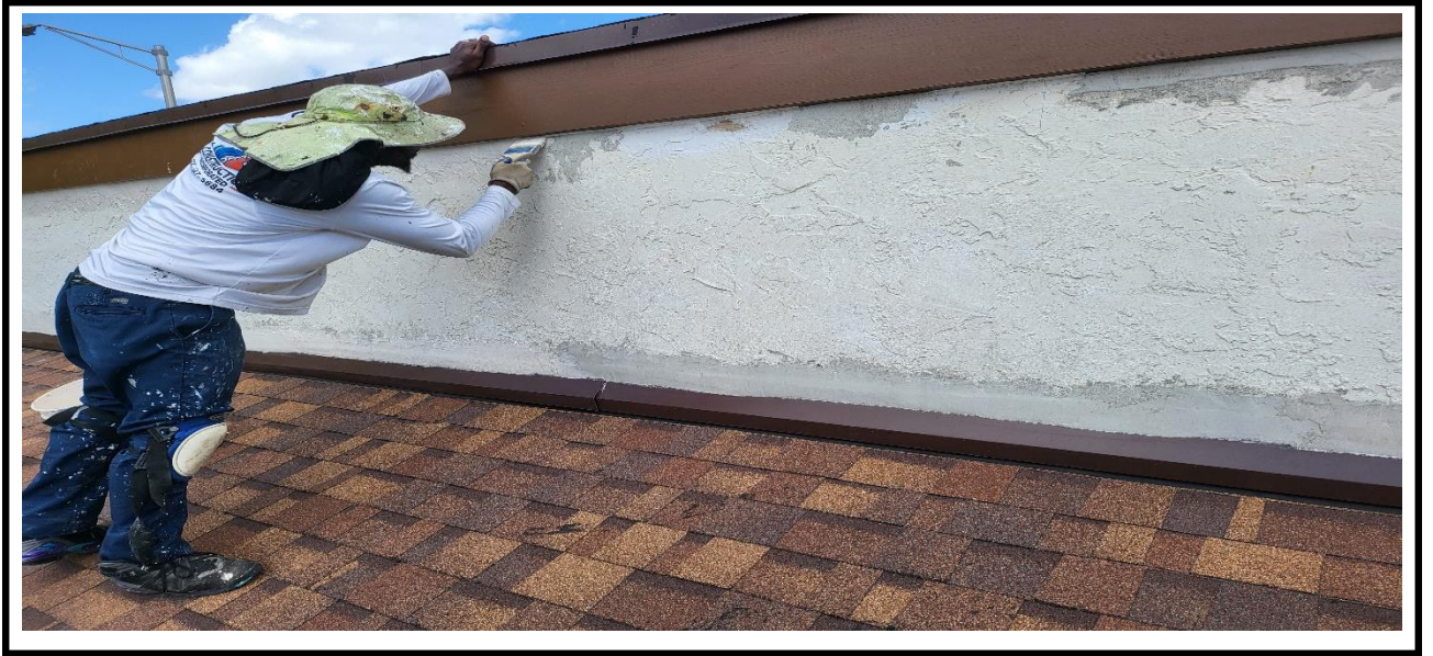
1 – Ongoing application of paint layers at new repaired areas
