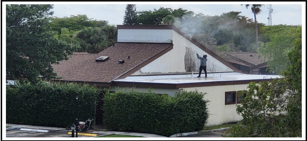
3 – Ongoing pressure washing at sidewall at second floors, to apply the paint layer
