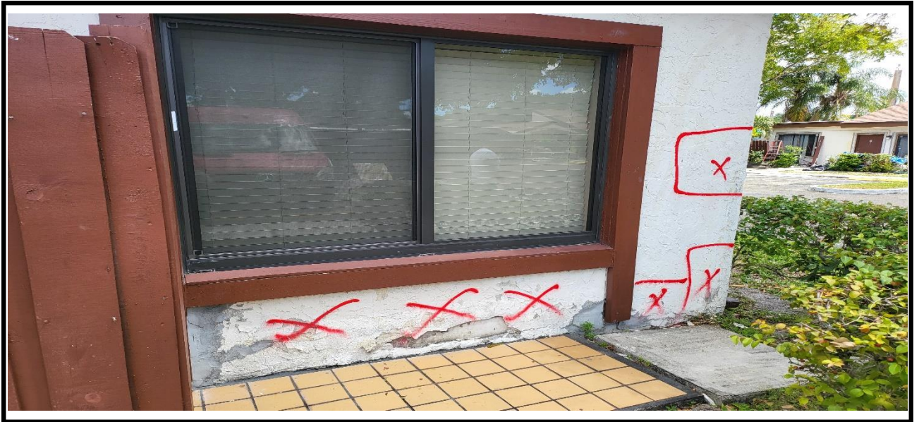
1 – Identification and marking of the delaminated stucco at exterior walls
