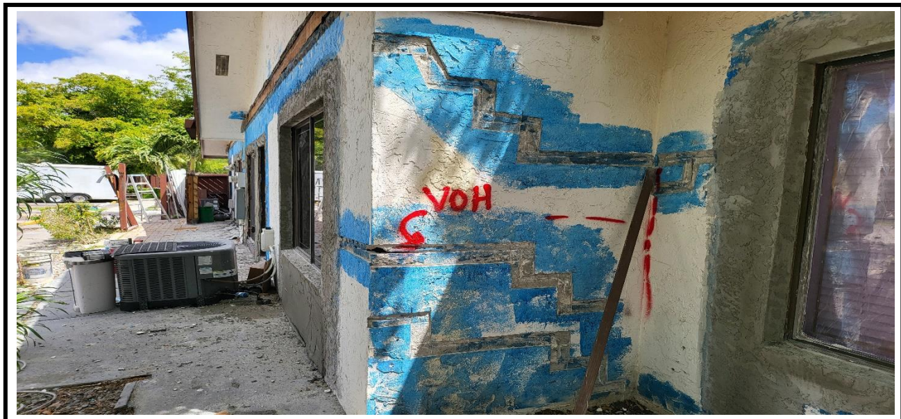
5 – Cutting and chipping of the delaminated and cracked stucco at the exterior walls.
