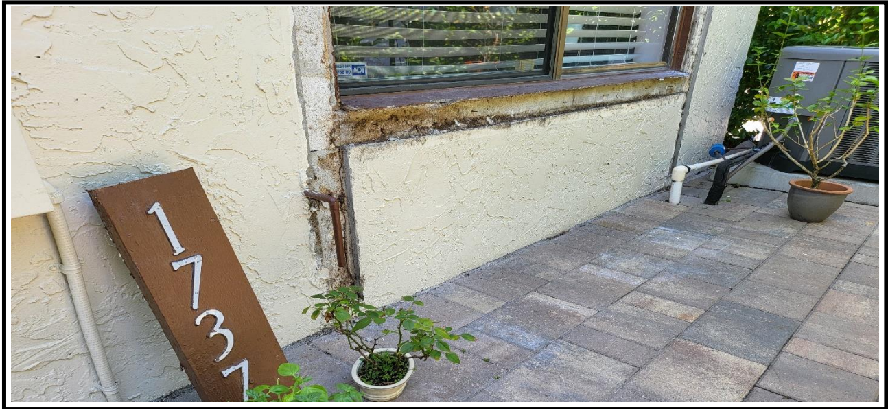
3 – Removal of the wood siding around the window perimeters at the exterior walls
