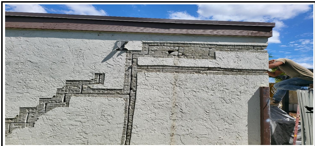
6 – Cutting and chipping of the cracked stucco at the exterior walls.
