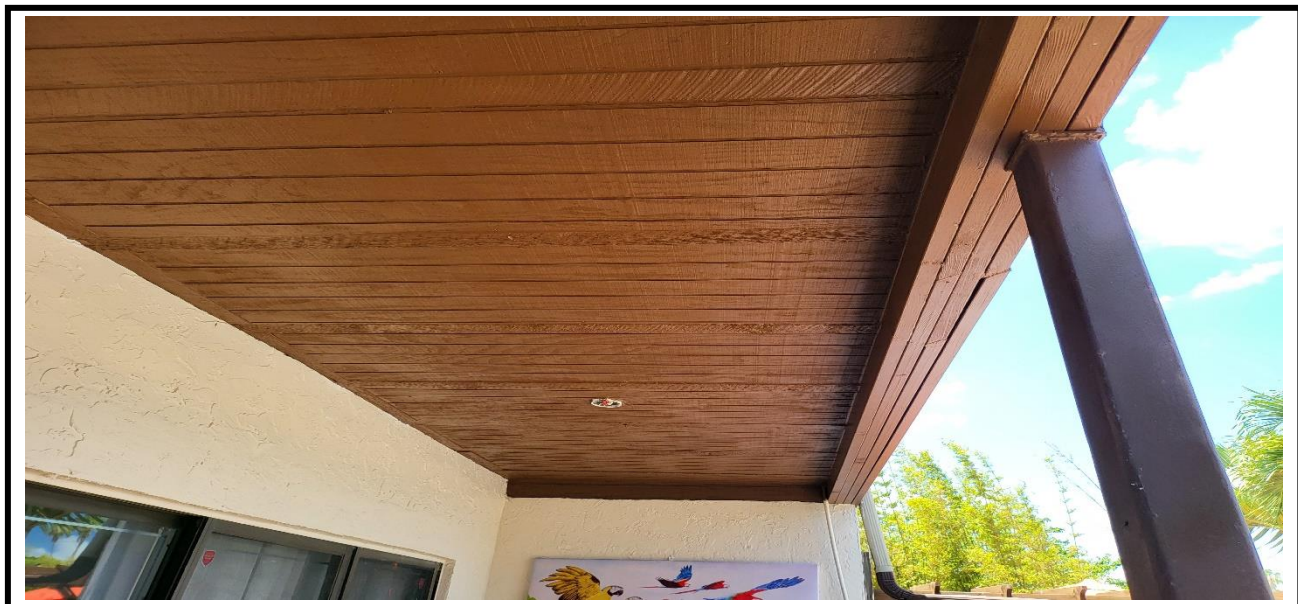
8 – Installation of the wood false ceiling at the back of the building.
