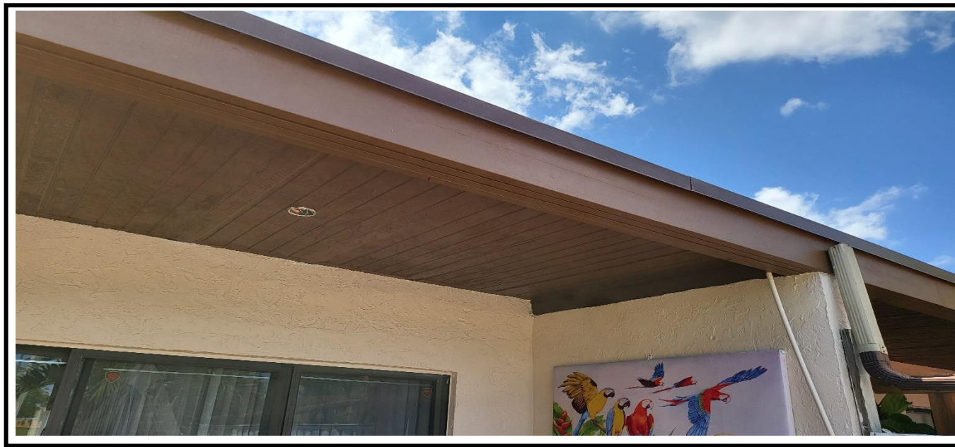
9 – Installation of the wood false ceiling at the back of the building.
