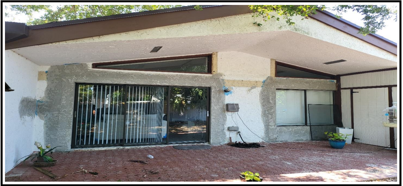
1 – Application of the new stucco at the exterior walls, around the window's perimeter.
