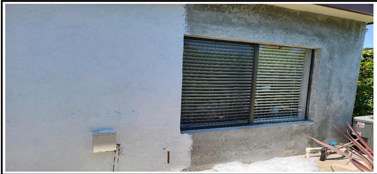
5 – Ongoing, Application of the new primer and paint at the exterior walls.
