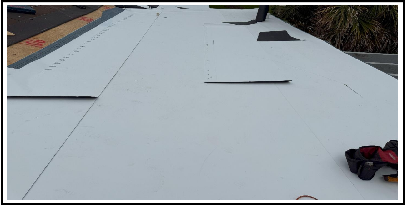
3 – Ongoing, Laying down the insulation sheets and tin caps / TPO sheets, BLDG 09.
