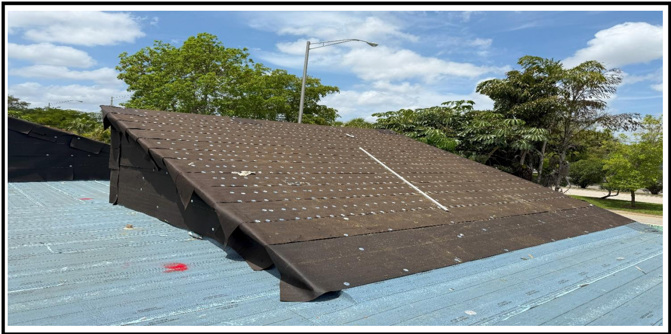
2 – Ongoing, Laying down the insulation sheets and tin caps / TPO sheets, BLDG 11.
