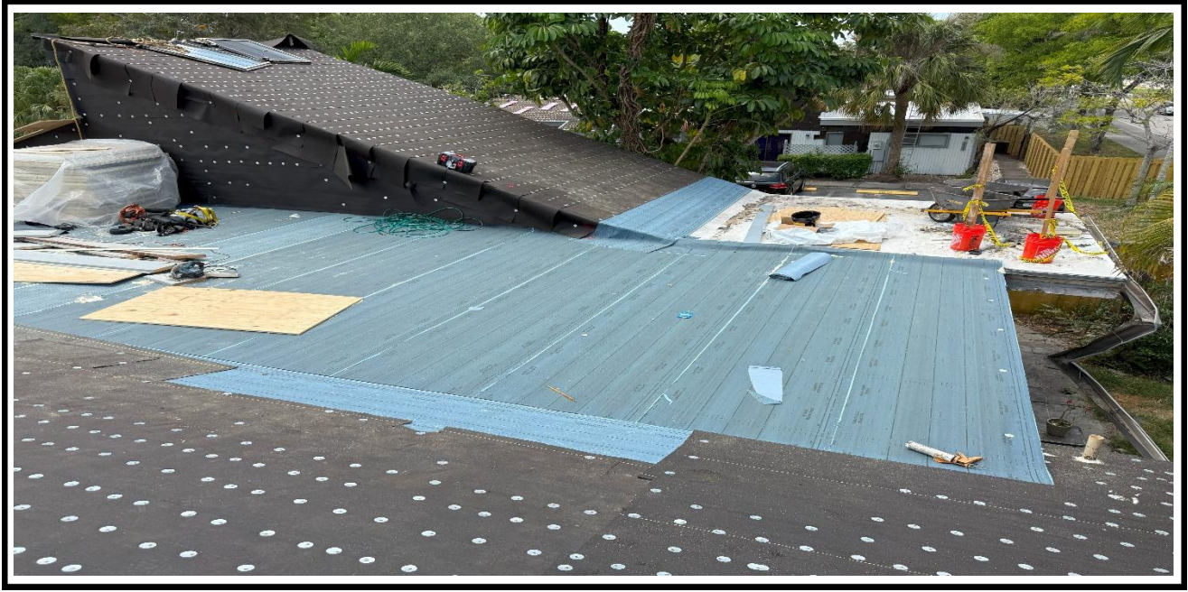
1 – Ongoing, Laying down the insulation sheets and tin caps / TPO sheets, BLDG 10.
