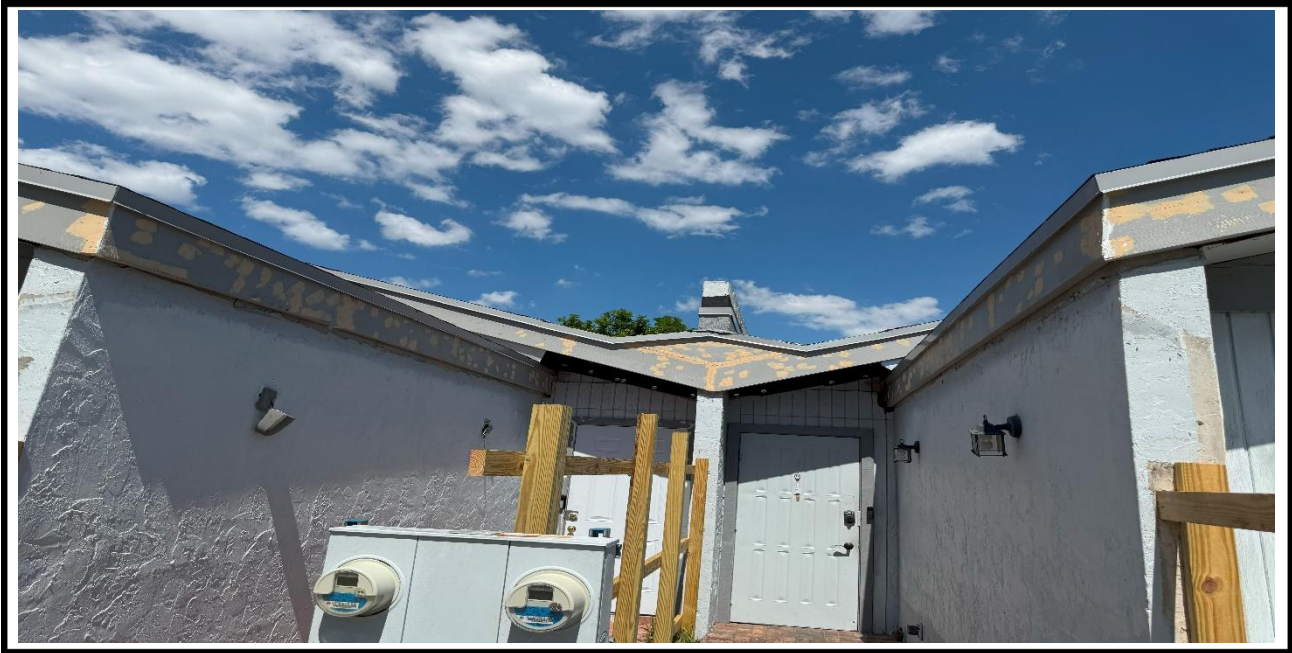
10 – Ongoing, , installation of the roofing shingles, fascia board and metal drip edges, BLDG 10.
