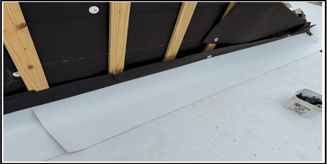
6 – Ongoing, installation of the waterproof sheets, wooden furring strips and TPO Sheets, BLDG 11.
