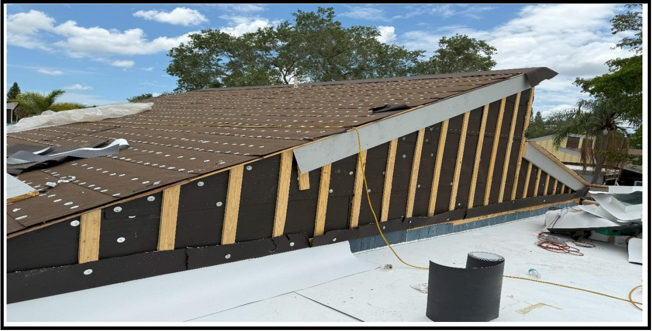
5 – Ongoing, installation of the waterproof sheets, wooden furring strips and TPO Sheets, BLDG 11.
