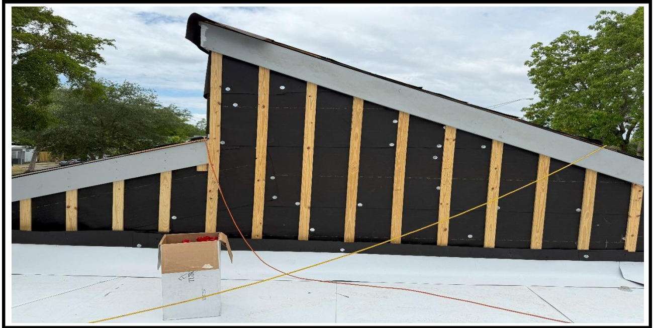
8 – Ongoing, Laying down the insulation sheets and tin caps / TPO sheets, BLDG 11.
