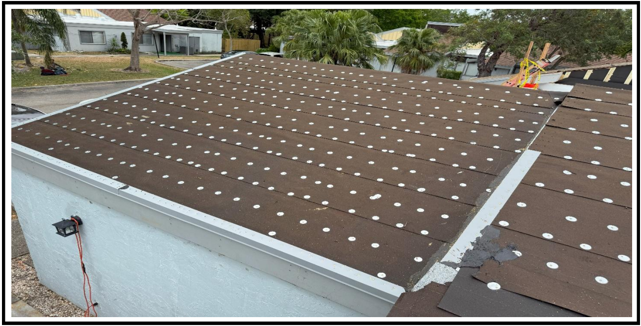
7 – Ongoing, Laying down the insulation sheets and tin caps and metal drip edges, BLDG 11.
