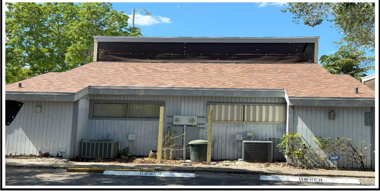
9 – Ongoing, installation of the roofing shingles, fascia board and metal drip edges, BLDG 10.
