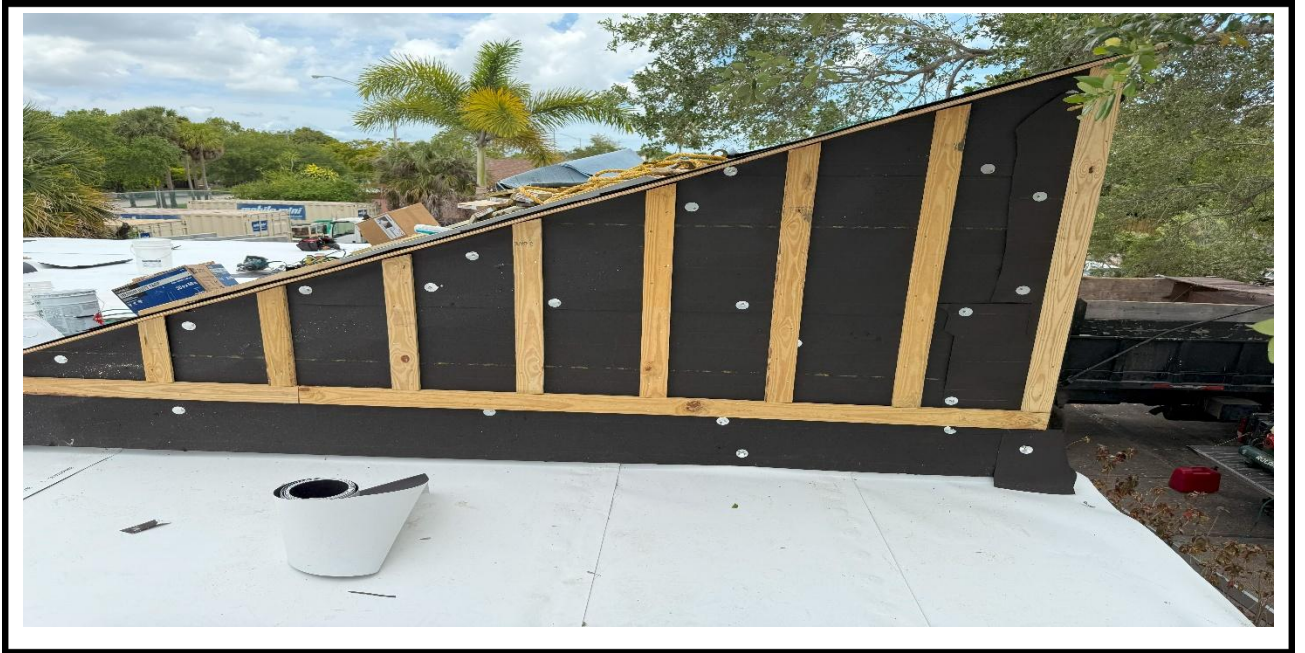
4 – Ongoing, installation of the waterproof sheets, wooden furring strips and TPO Sheets, BLDG 10.
