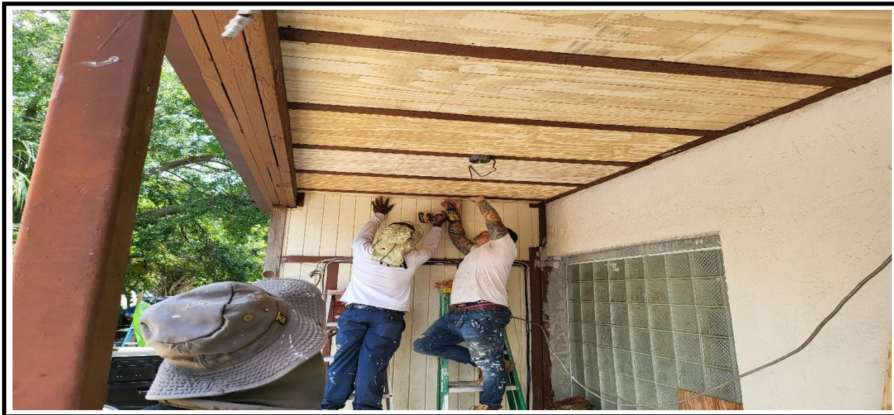
5 – Ongoing, Installation of the wood false ceiling at the back of the building.
