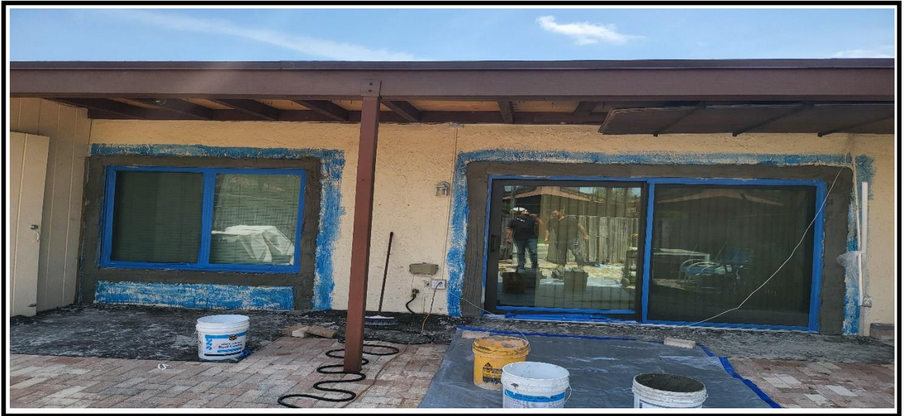
1 – Application of the new stucco at the exterior walls, around the window's perimeter.
