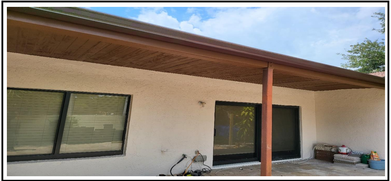
7 – Installation of the wood false ceiling at the back of the building.
