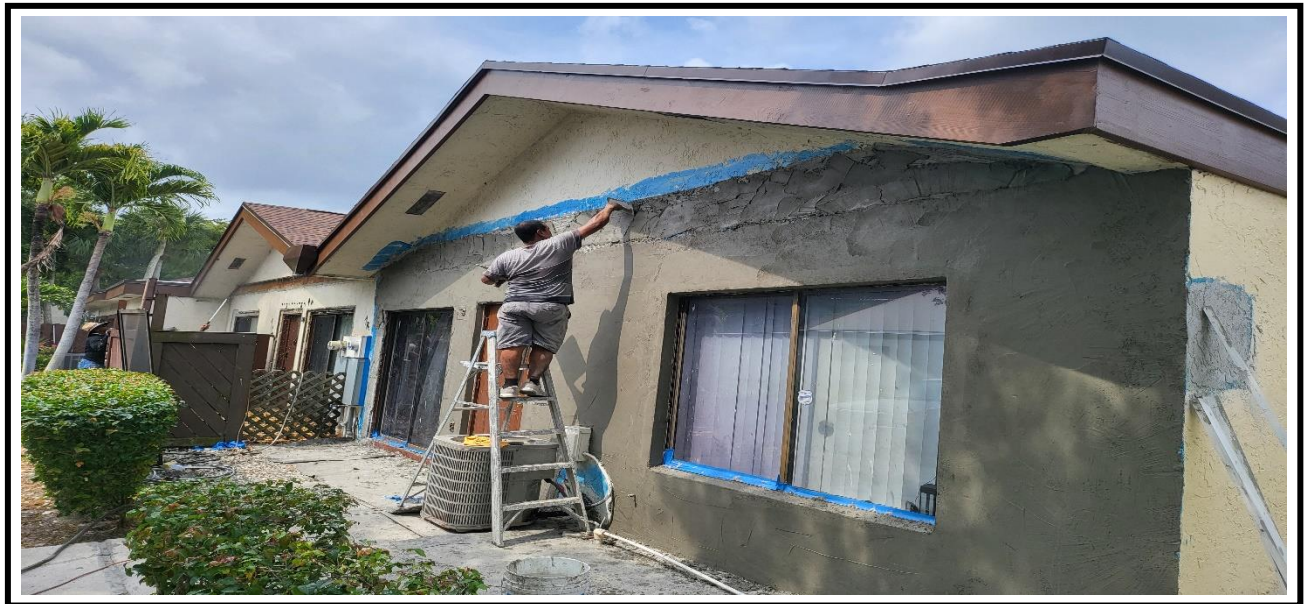
8 – Ongoing, the application of the new stucco at the exterior walls and around the window's perimeter.
