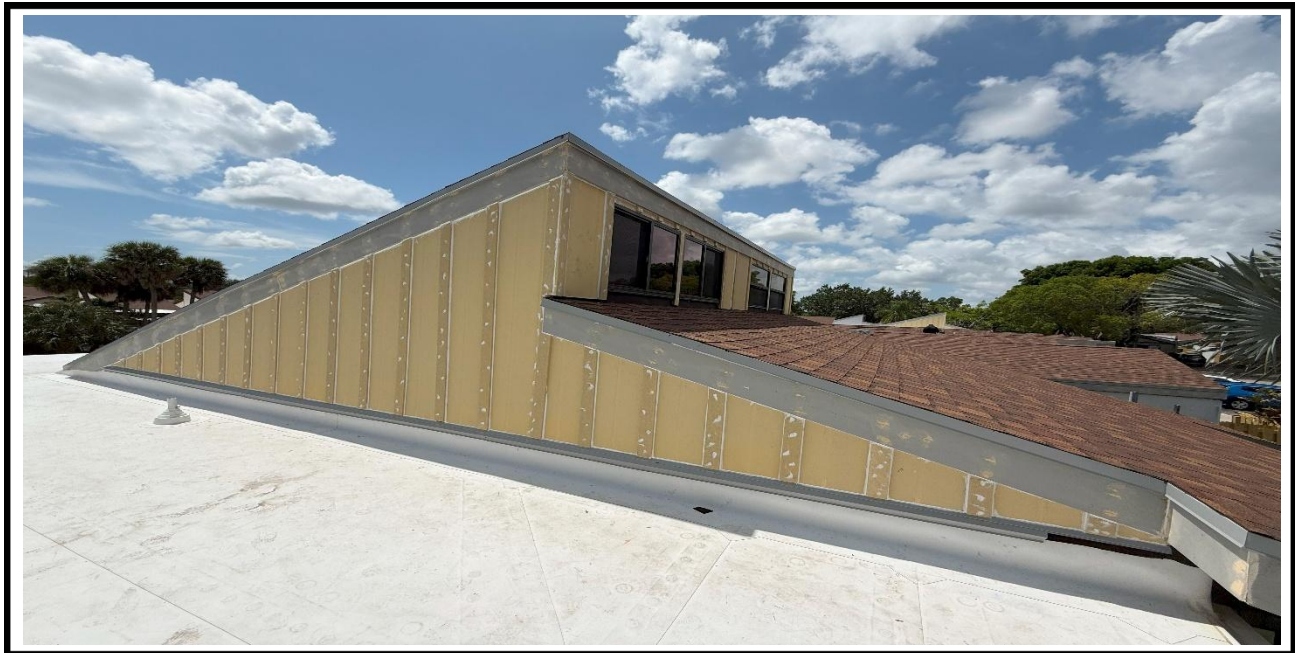
8 – Ongoing, installation of the roofing shingles and the furring strips on hardie board, BLDG 11.
