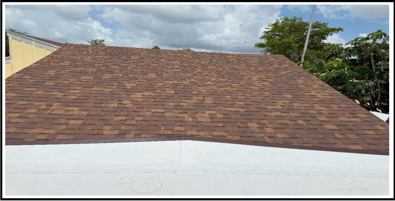
3 – Ongoing, Installation of the roofing shingles and TPO Sheets, BLDG 09.
