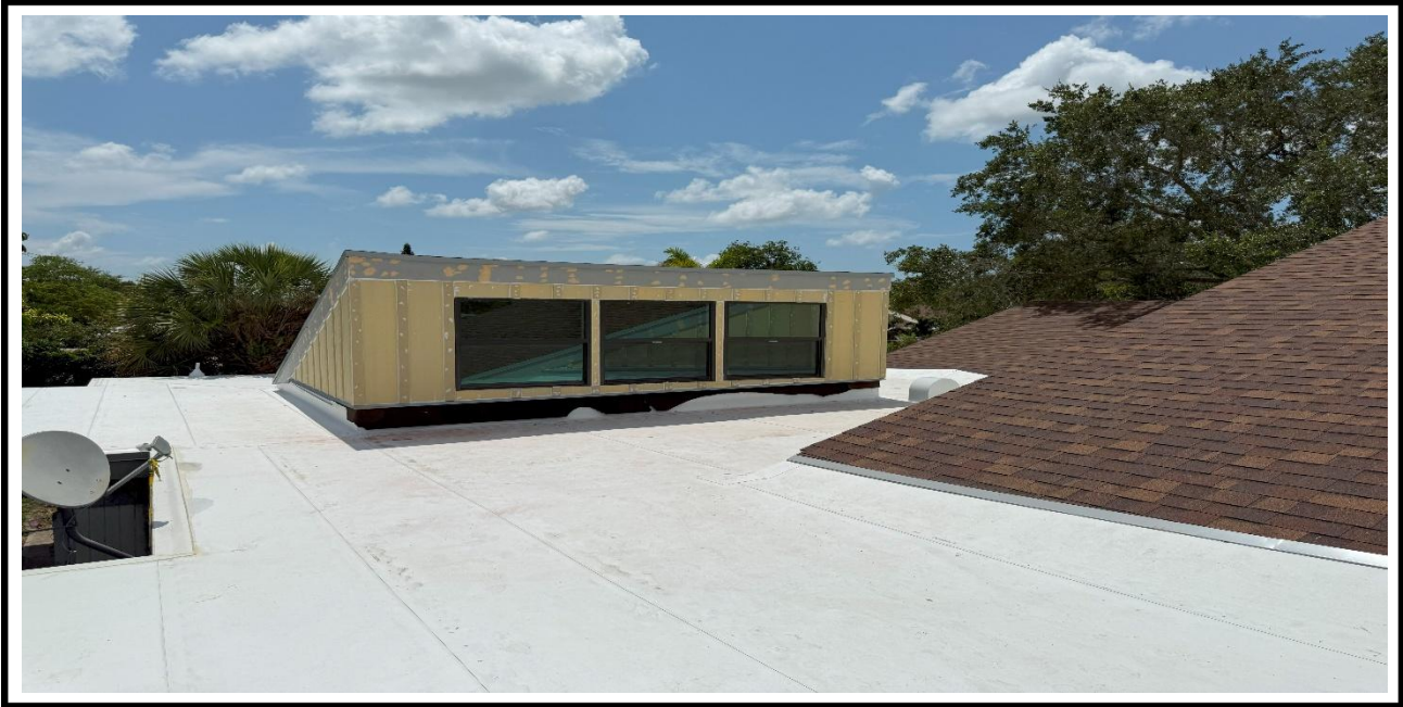
7 – Ongoing, installation of the roofing shingles and the furring strips on hardie board, BLDG 11.
