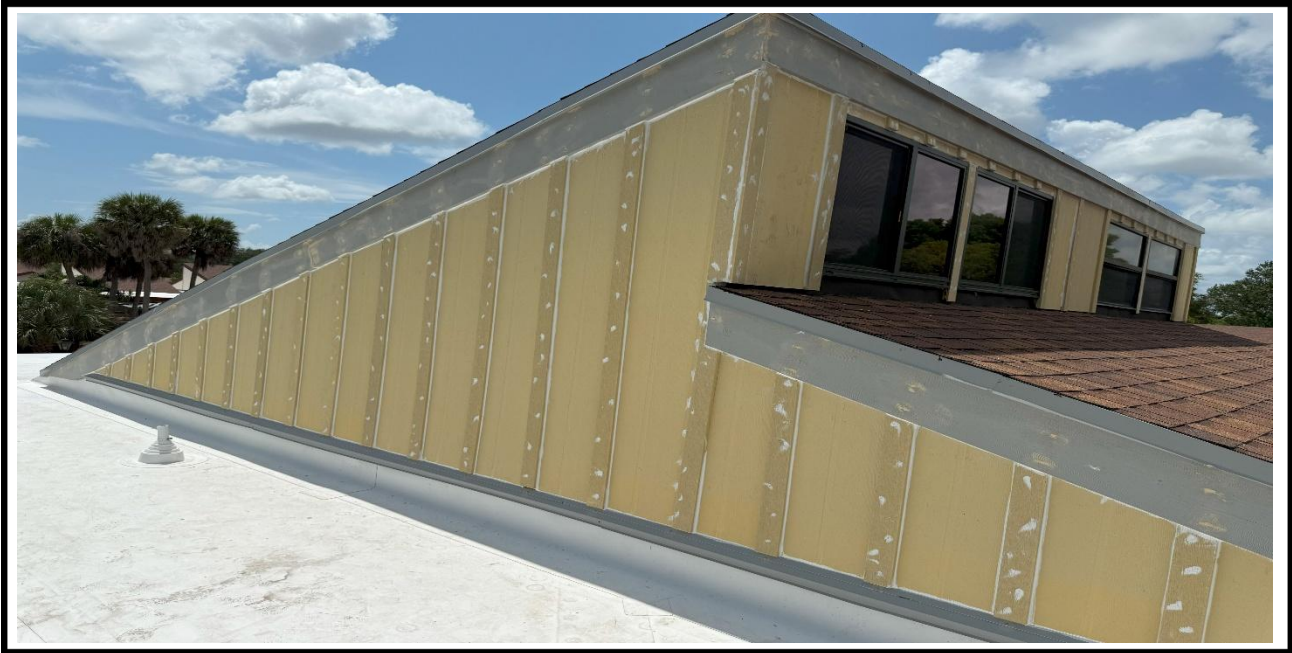
4 – Ongoing, Installation of the furring strips on hardie board, BLDG 09.
