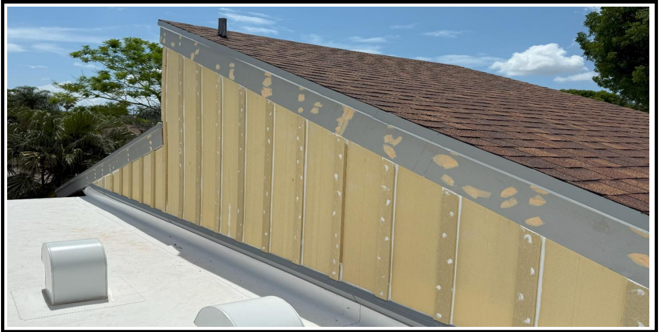
6 – Ongoing, installation of the roofing shingles and the furring strips on hardie board, BLDG 11.
