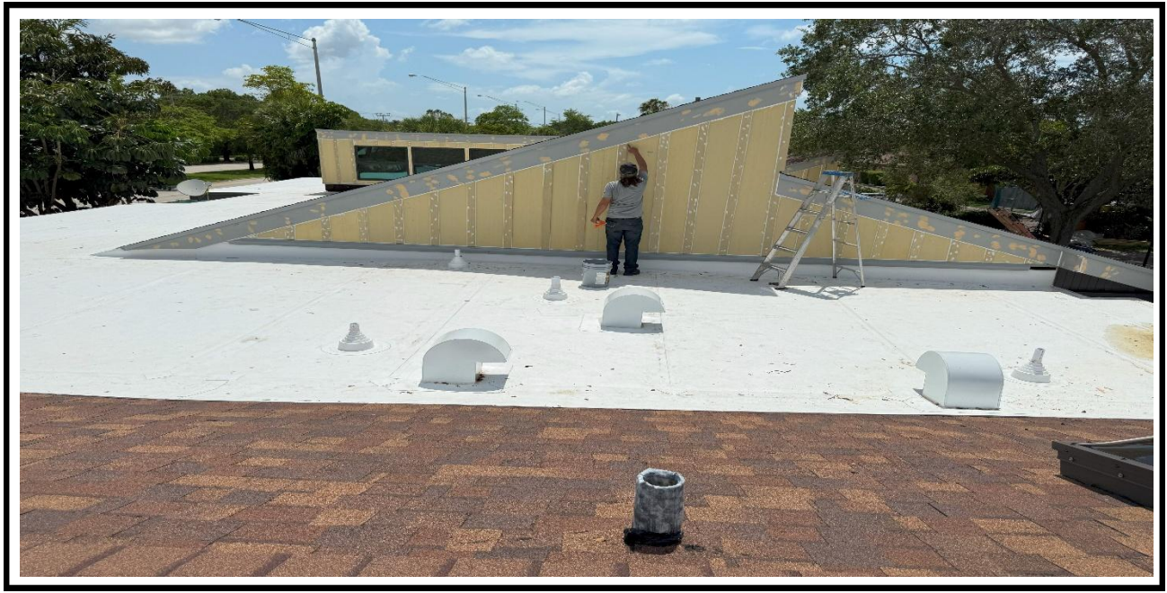
11 – Ongoing, installation of the roofing shingles and the furring strips on hardie board, BLDG 10.
