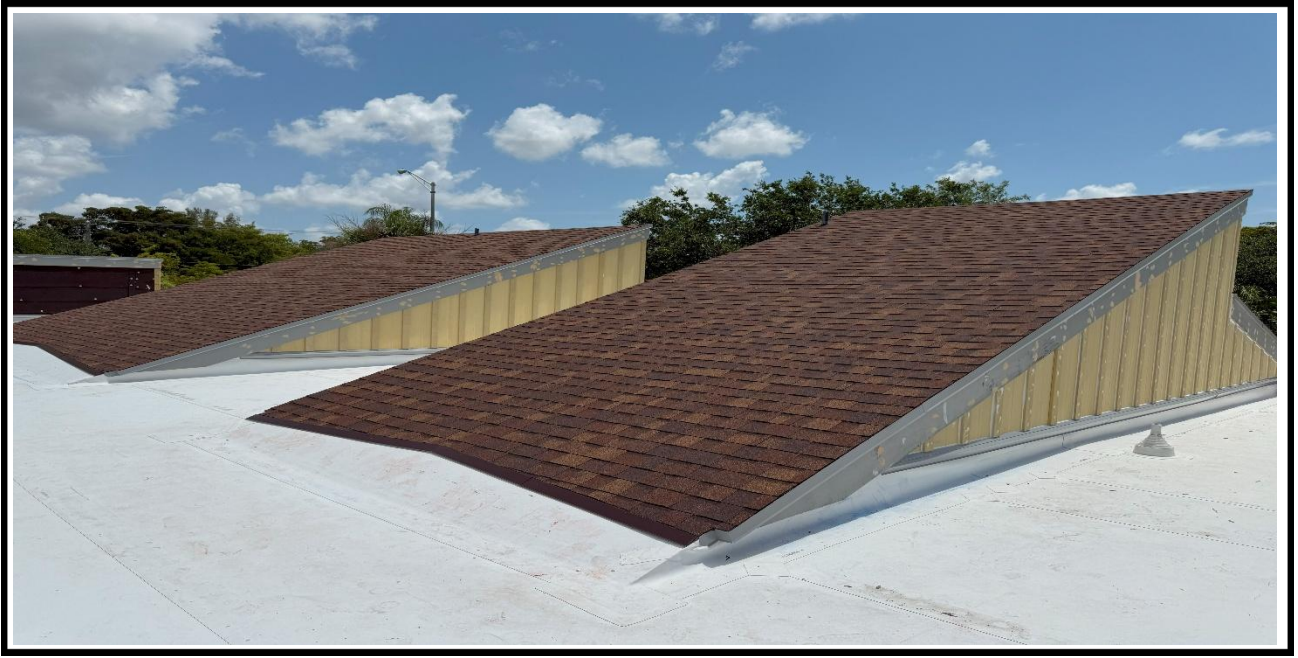
5 – Ongoing, installation of the roofing shingles, BLDG 11.
