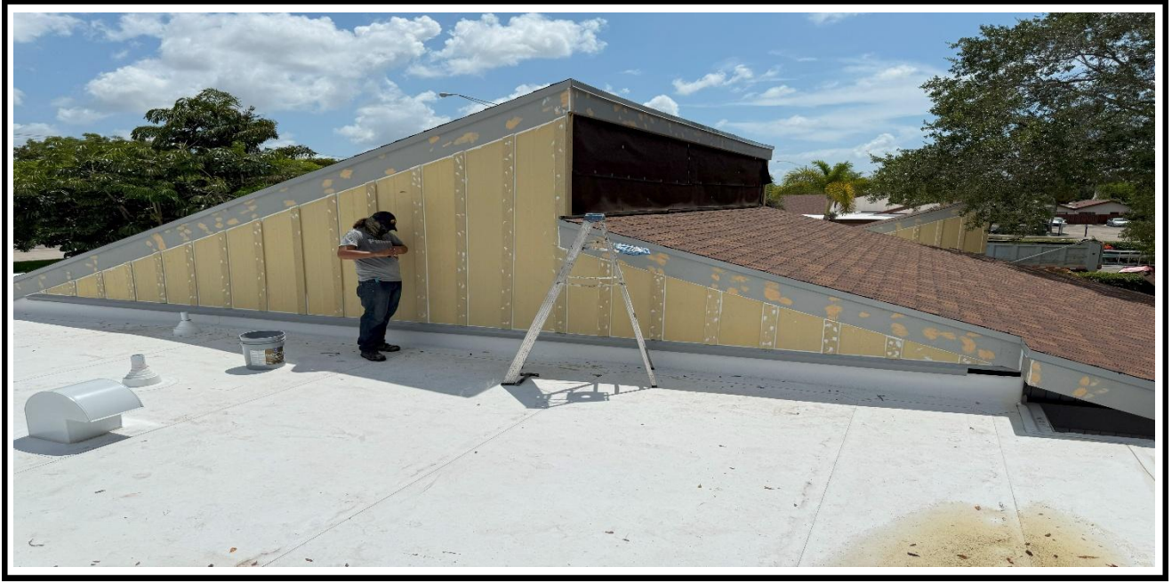
1 – Ongoing, Installation of the furring strips on hardie board, BLDG 09.
