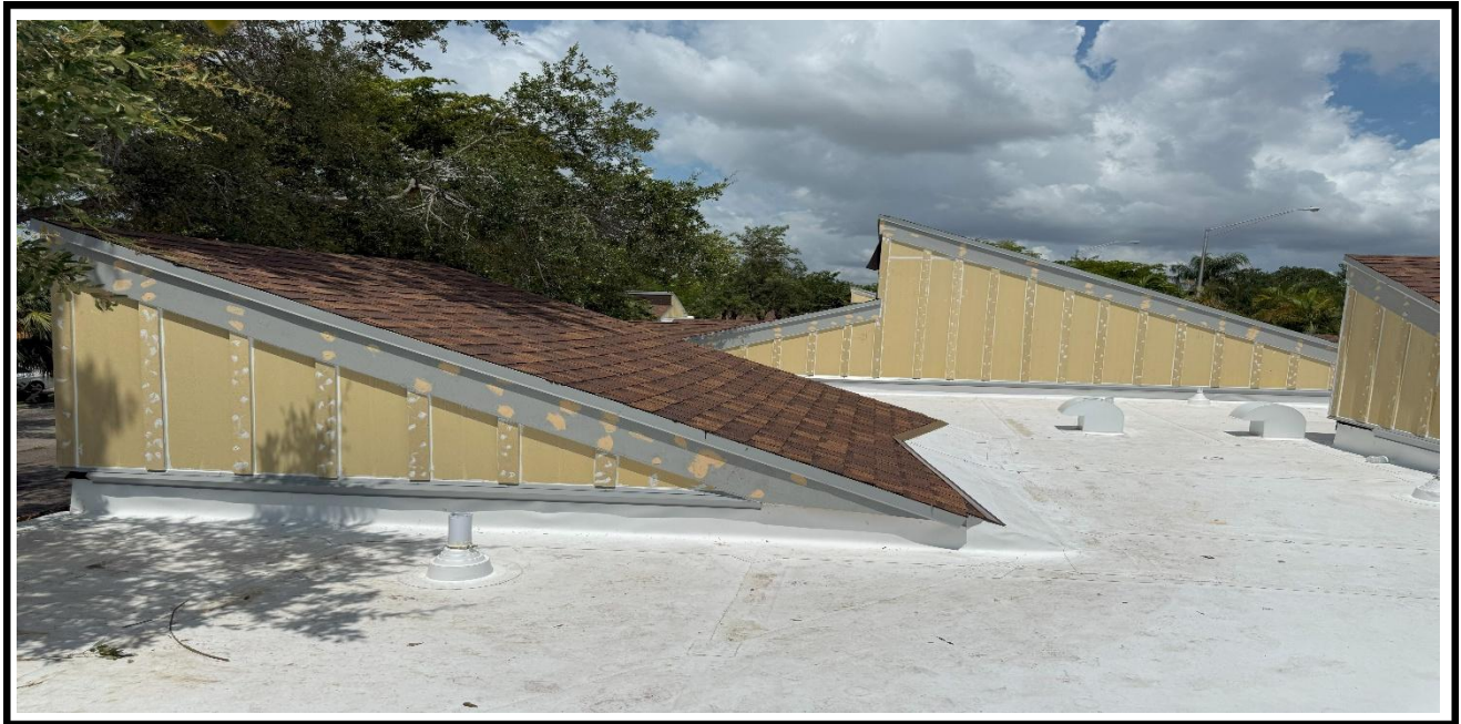
2 – Ongoing, Installation of the hardie board at siding, BLDG 09.
