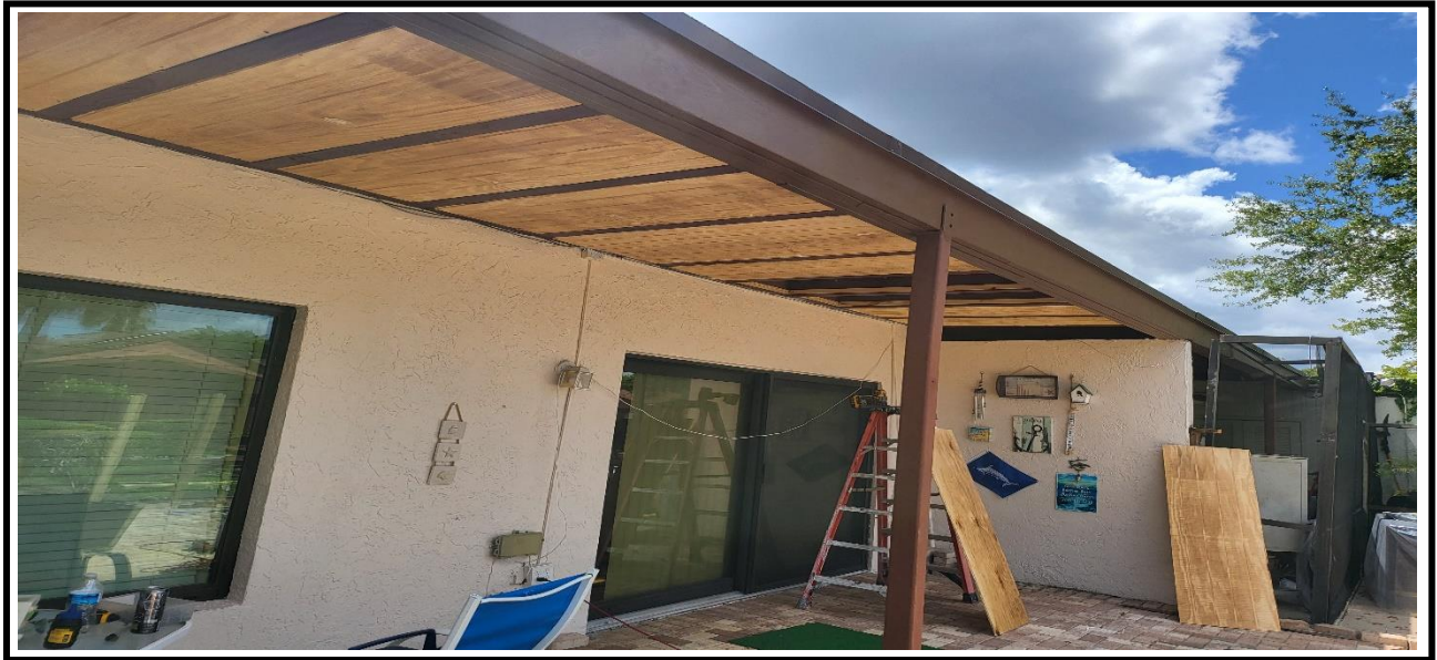
5 – Ongoing, Installation of the wood false ceiling at the back of the building.
