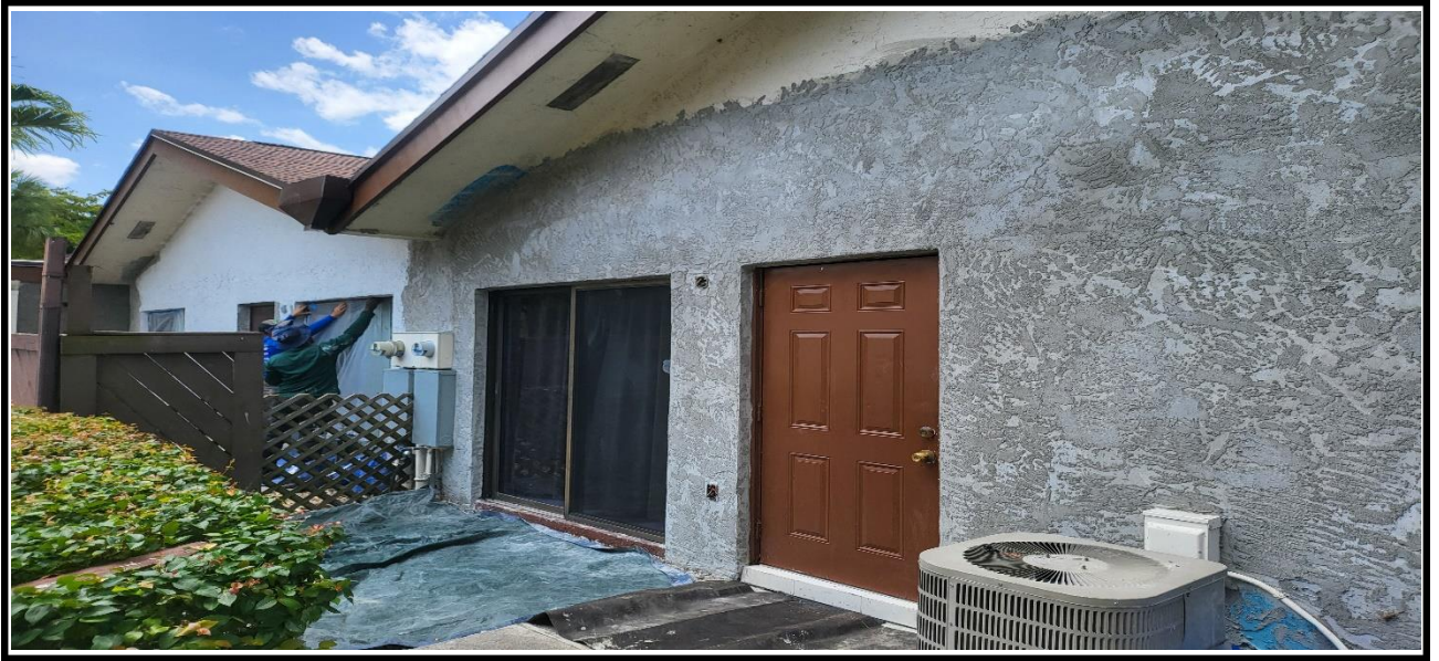
1 – Application of the new stucco at the exterior walls and around the window's perimeter.
