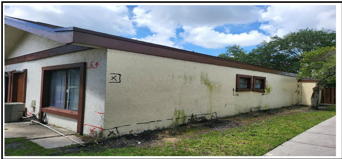
8 – Ongoing, Inspection of the old stucco at the exterior walls.
