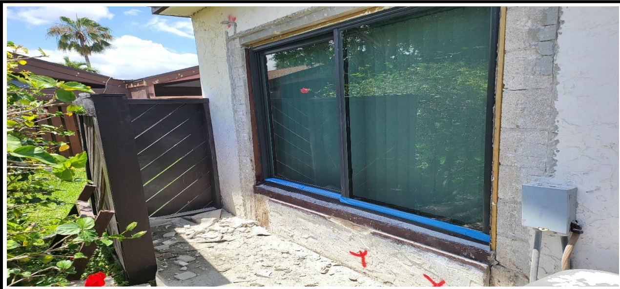
3 – Ongoing, Cutting and chipping of the delaminated and cracked stucco at the exterior walls.
