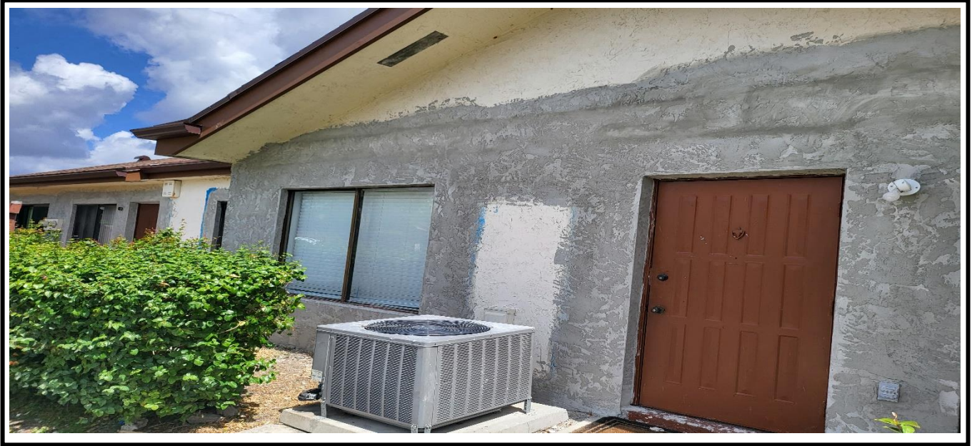
9 – Ongoing, Application of the new stucco at exterior walls.
