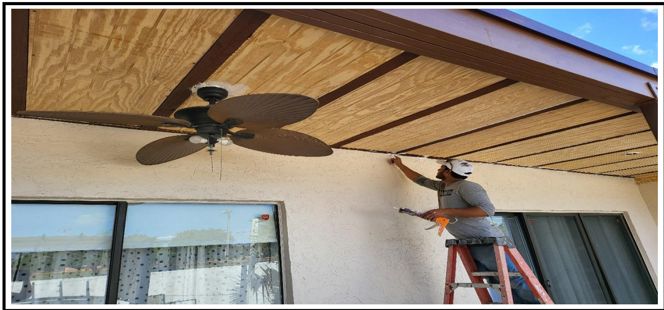
7 – Ongoing, Application of the filler material and caulking at exterior surfaces.
