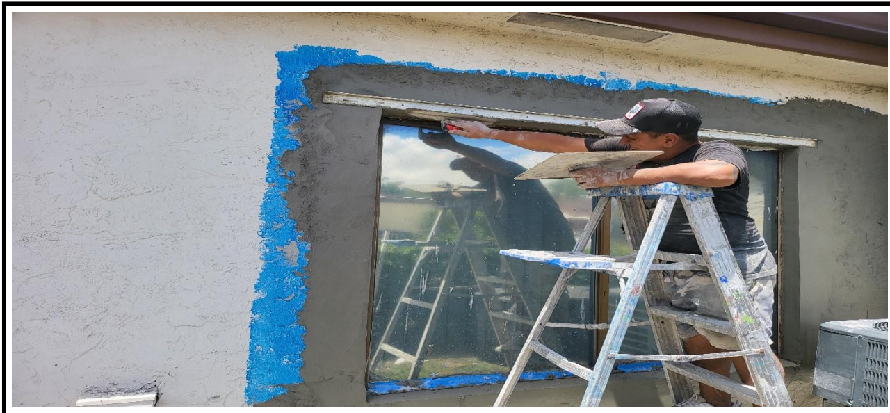
5 – Ongoing, Application of the bonding agent and the new stucco at exterior walls.
