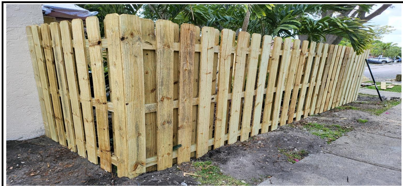
9 – Ongoing, Installation of the wooden fence.
