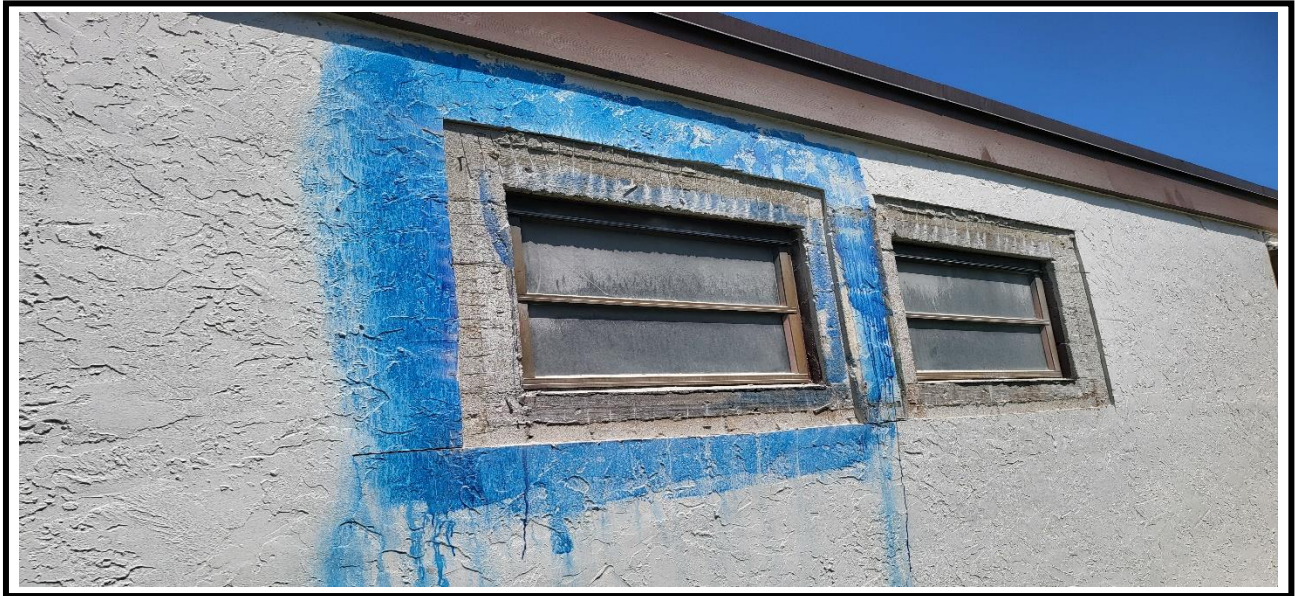
3 – Ongoing, Chipping of the marked and deteriorated stucco on exterior walls.
