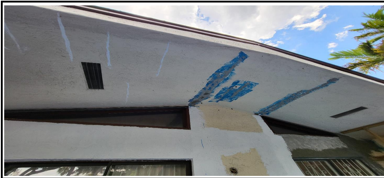
5 – Ongoing, Application of the crack filler at at the ceiling
