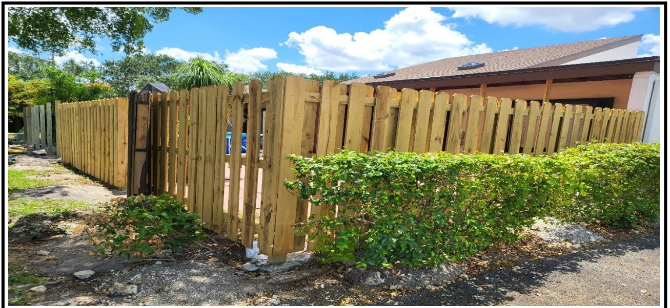
8 – Ongoing, Installation of the wooden fence.
