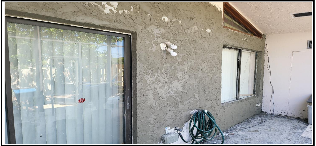
7 – Ongoing, Application of the new stucco at the exterior walls
