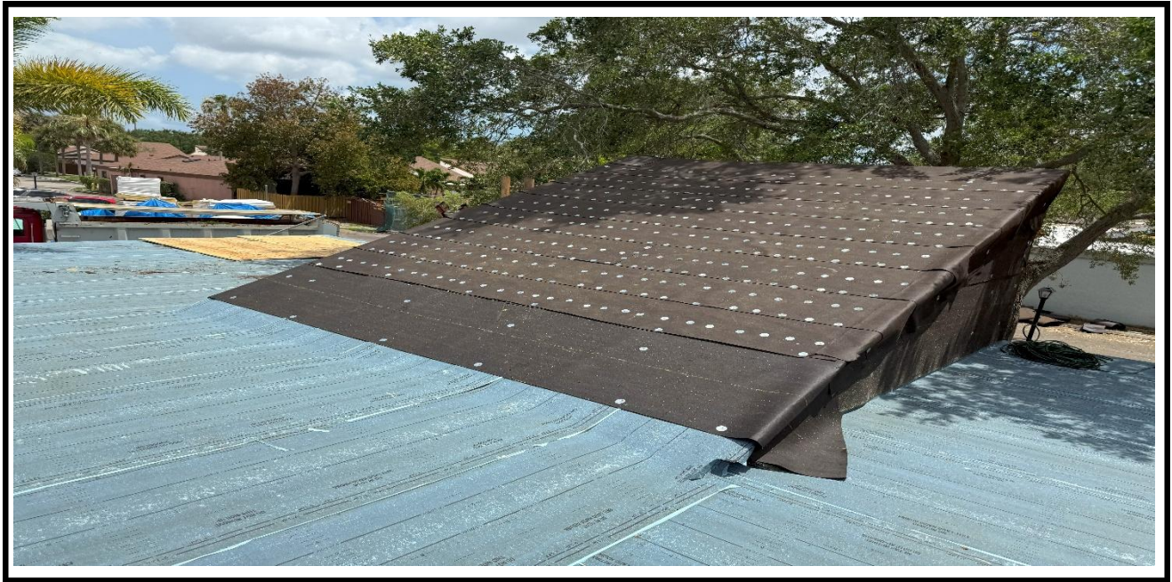
2 – Ongoing, Laying down the roofing insulation sheets on top of the plywood and waterproof sheets, BLDG 11.
