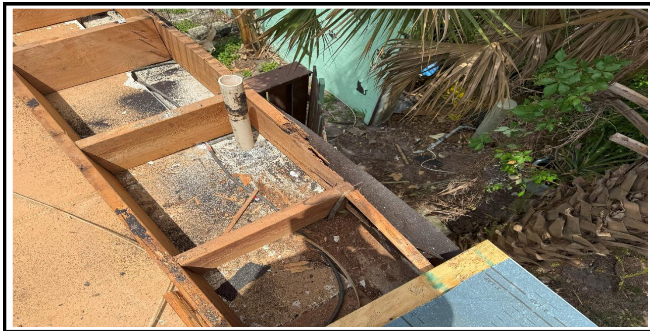
8 – Ongoing, replacement of the bad plywood and wood beams, BLDG 10.
