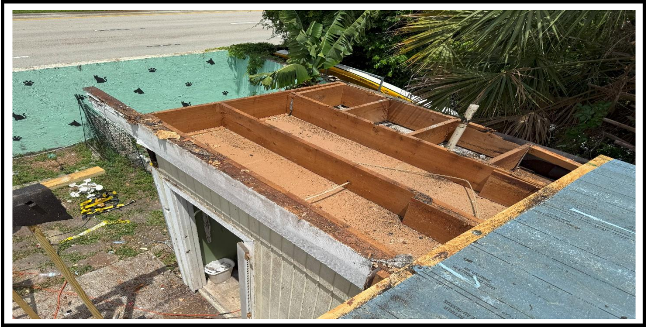
3 – Ongoing, replacement of the bad plywood and wood beams, BLDG 10.
