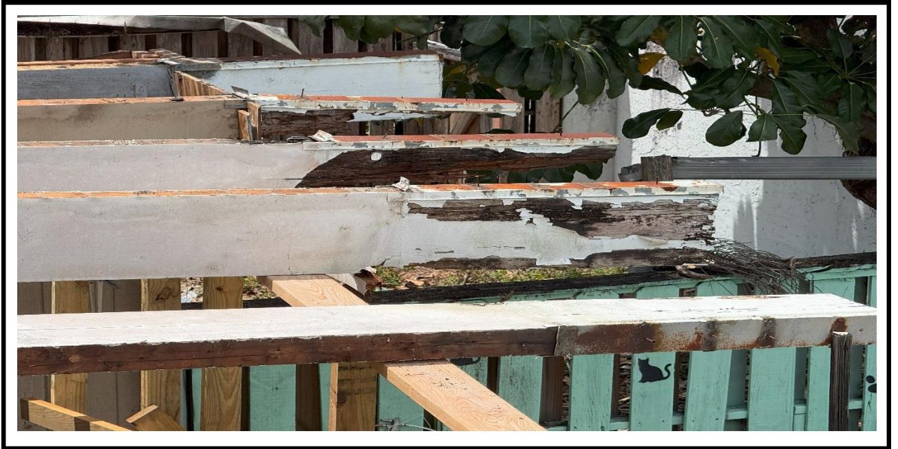
4 – Ongoing, replacement of the bad plywood and wood beams, BLDG 10.
