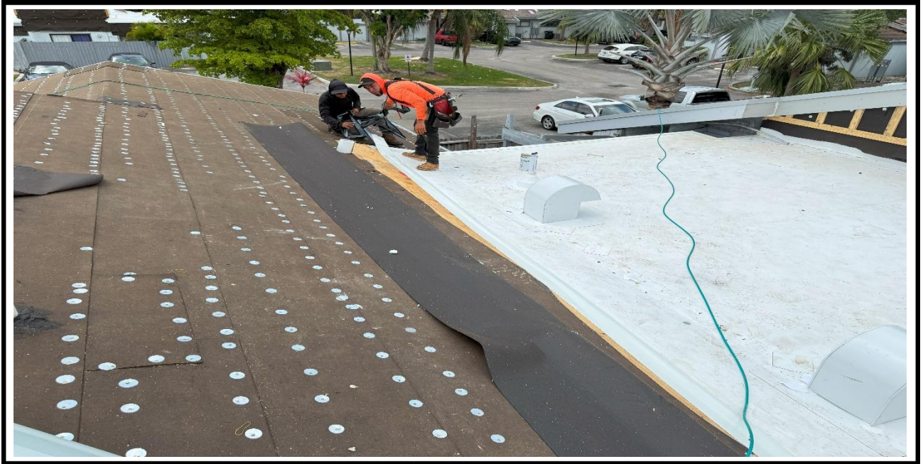
10 – Ongoing, Laying down the insulation sheets and tin caps / TPO Sheets, BLDG 10.
