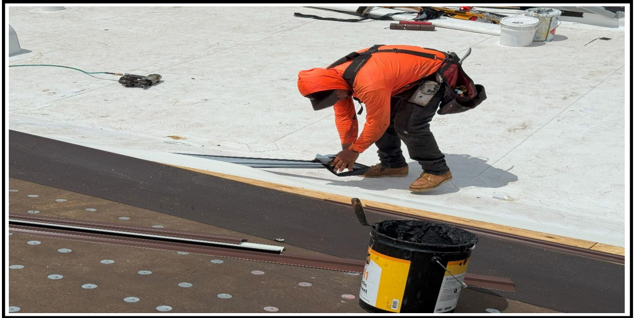
6 – Ongoing, installation of the waterproof sheets, wood furring strips, fascia board and metal drip edges , BLDG 09.
