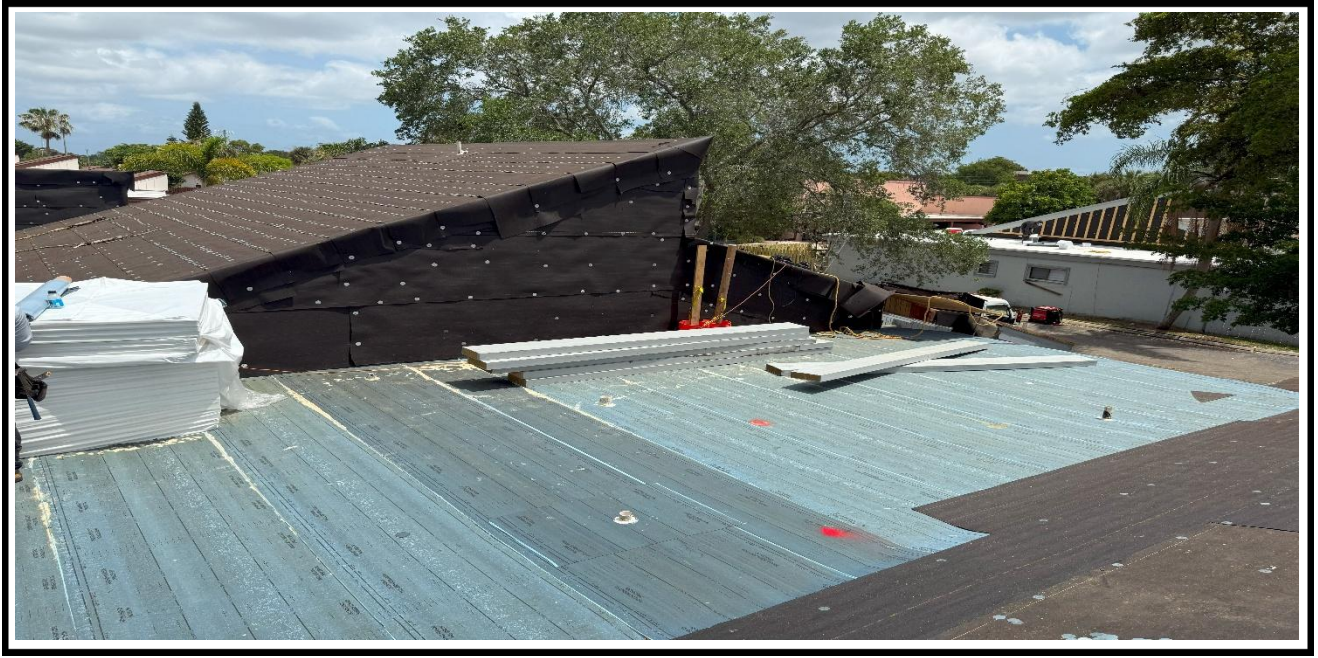
1 – Ongoing, Laying down the roofing insulation sheets on top of the plywood, BLDG 11.
