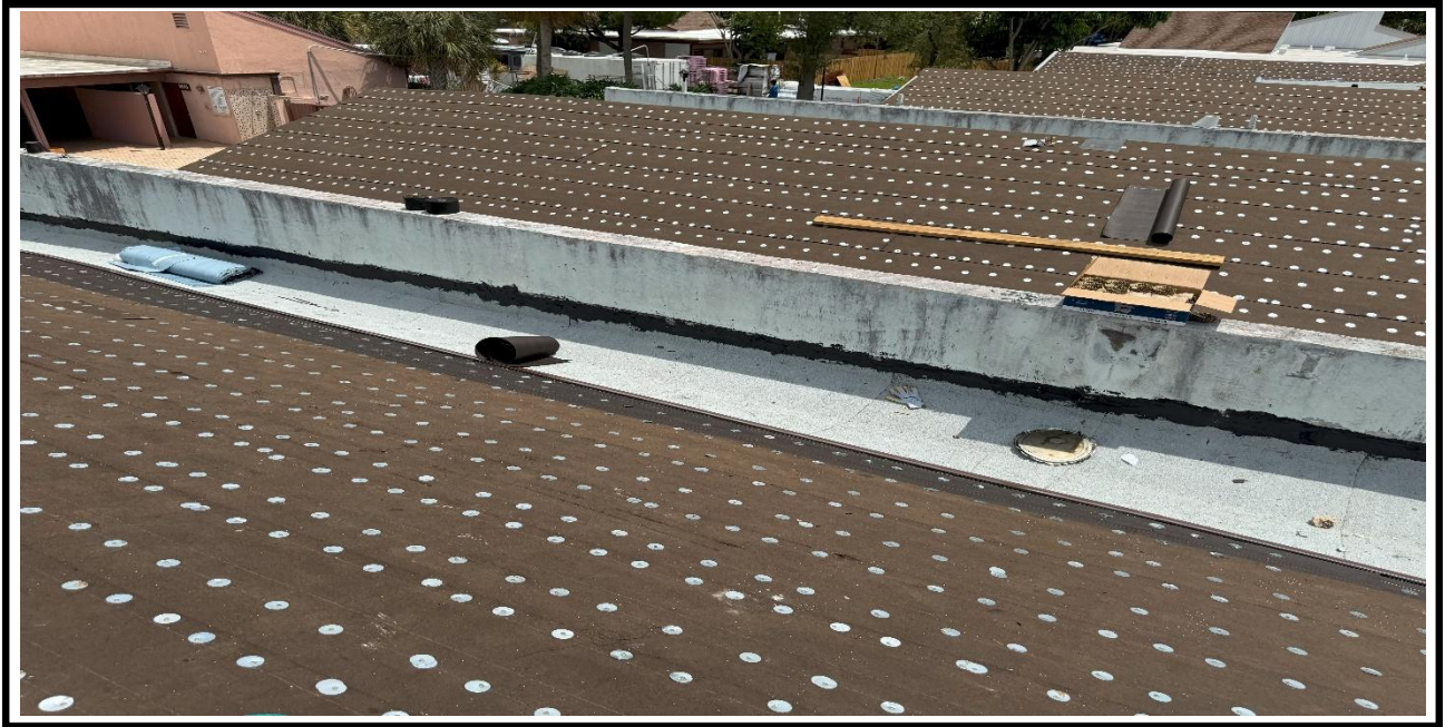
12 – Ongoing, installation of the waterproofing sheets and tin caps, BLDG 10.
