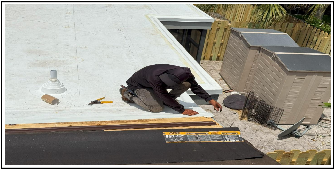
11 – Ongoing, laying down the TPO sheets and welding it, BLDG 10.
