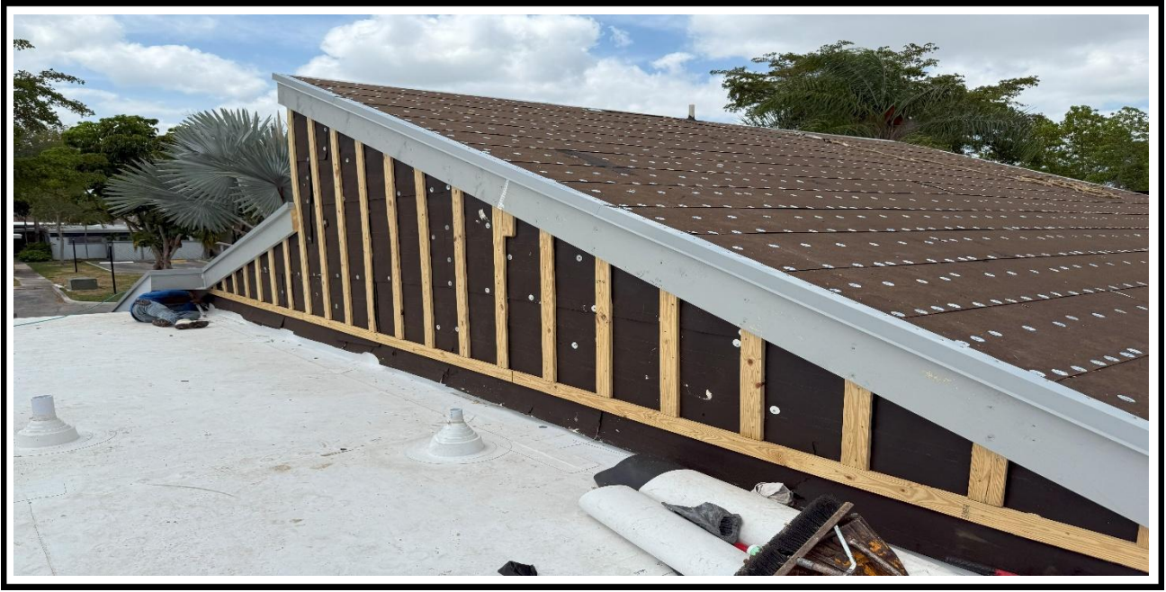
5 – Ongoing, installation of the waterproof sheets, wood furring strips, fascia board and metal drip edges , BLDG 10.
