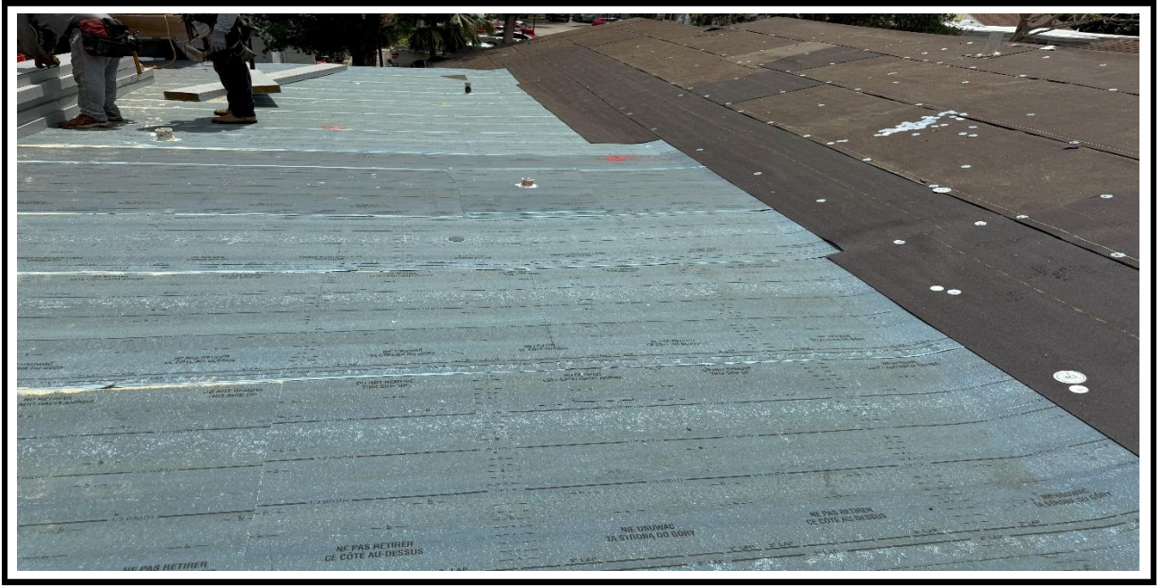
9 – Ongoing, Laying down the insulation sheets and tin caps, BLDG 10.
