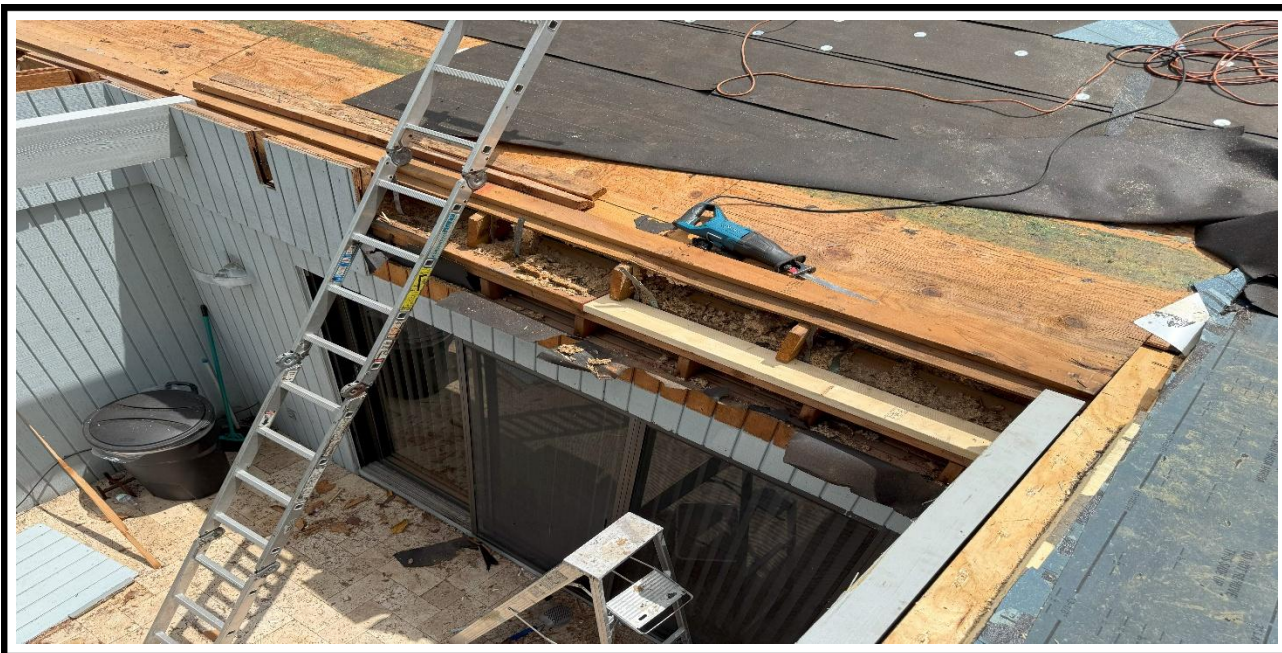
7 – Ongoing, replacement of the bad plywood and wood beams, BLDG 10.
