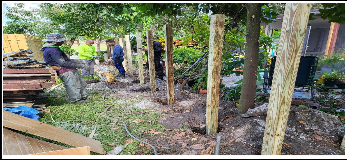
9 – Ongoing, Installation of the wooden fence.
