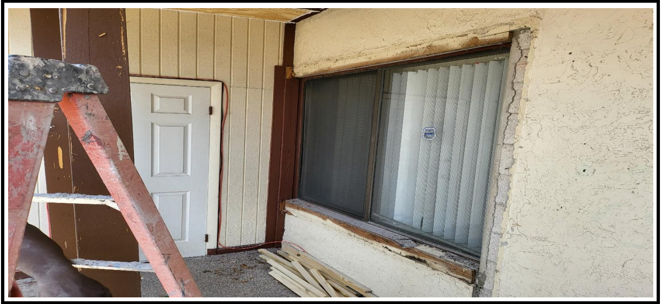
1 – Ongoing, Chipping of the marked and deteriorated stucco on exterior walls.
