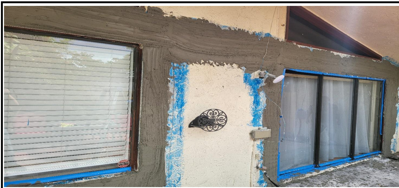
3 – Ongoing, Application of the new stucco at the exterior walls, around the window's perimeter.
