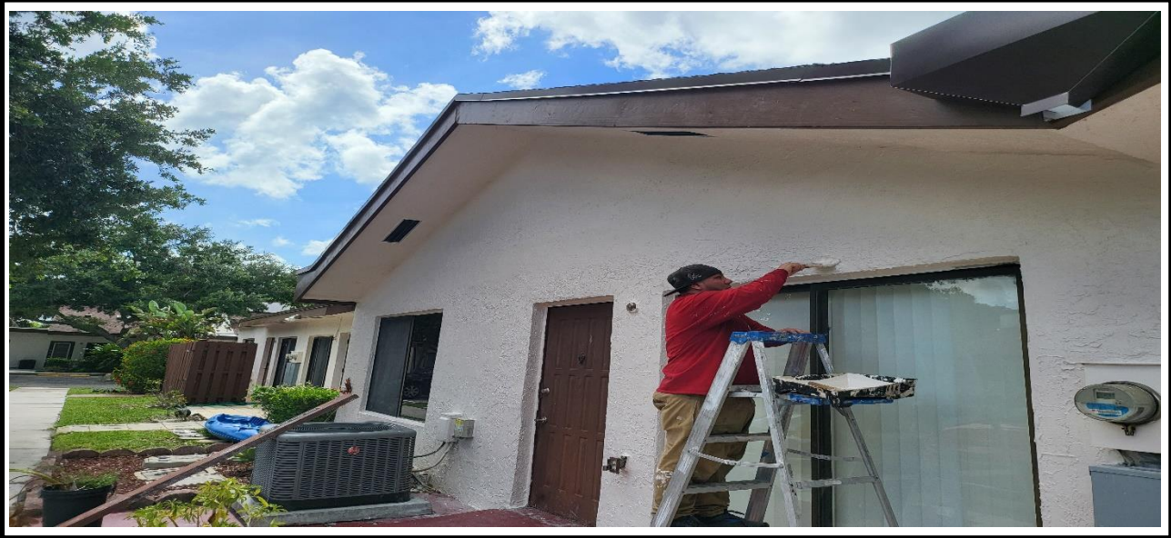
5 – Ongoing, Application of the primer layer on the exterior walls.
