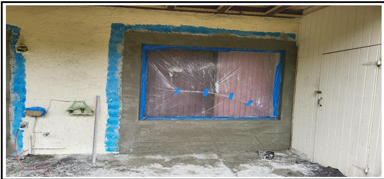
3 – Ongoing, Application of the new stucco at the exterior walls, around the window's perimeter, BLDG 24.
