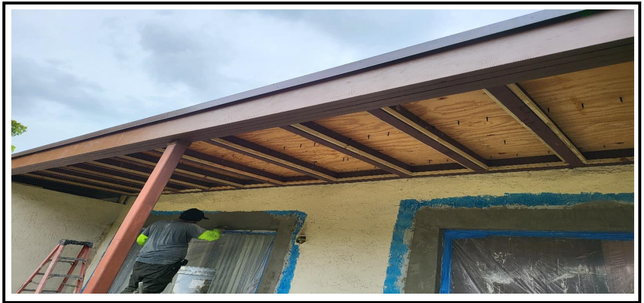
7 – Ongoing, Installation of the wooden ceiling at the back of the building, BLDG 24.
