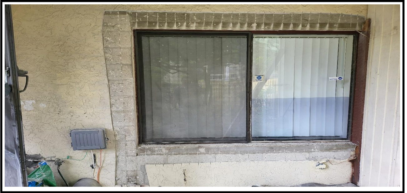
1 – Ongoing, Removal of old wood and Chipping of the deteriorated stucco on exterior walls, BLDG 24.
