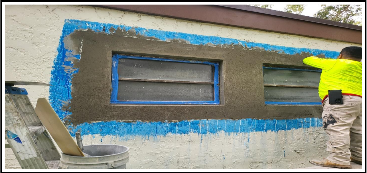
5 – Ongoing, Application of the new stucco at the exterior walls, around the window's perimeter, BLDG 24.
