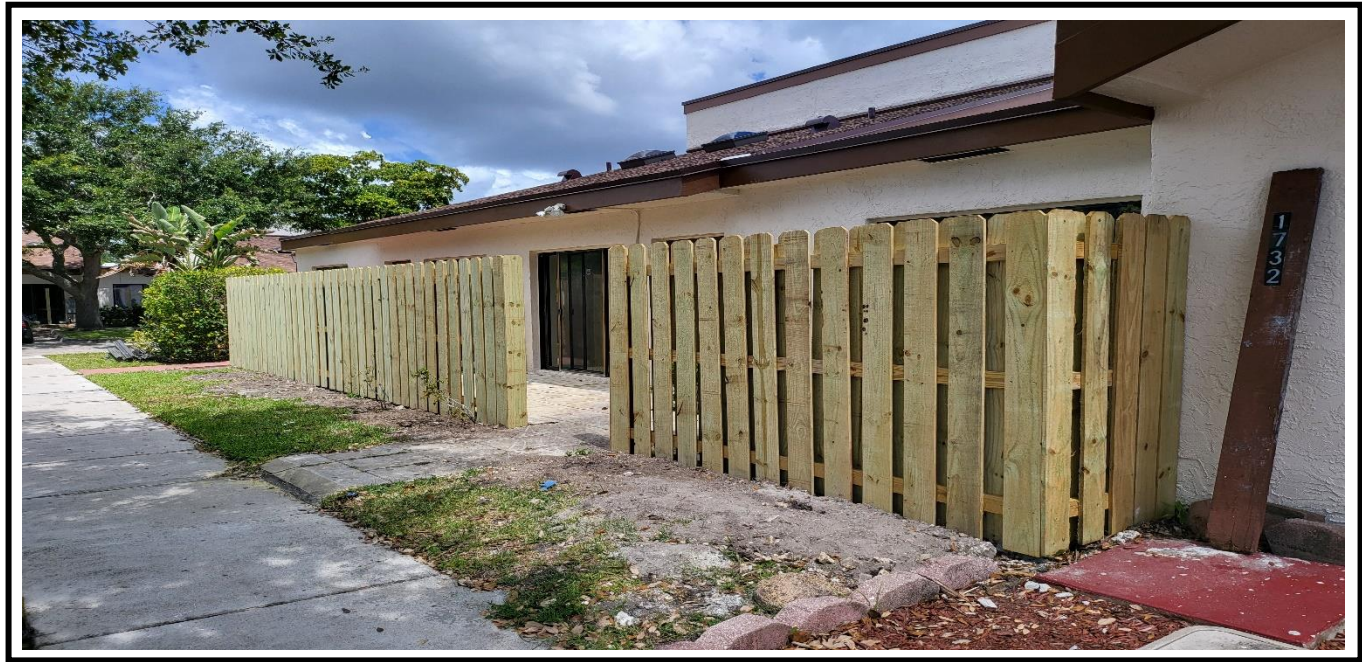
9 – Ongoing, Installation of the wooden fence, BLDG 23.
