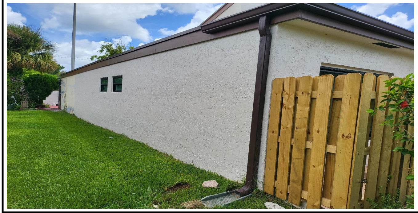
11 – Ongoing, Installation of the gutter system, BLDG 21.
