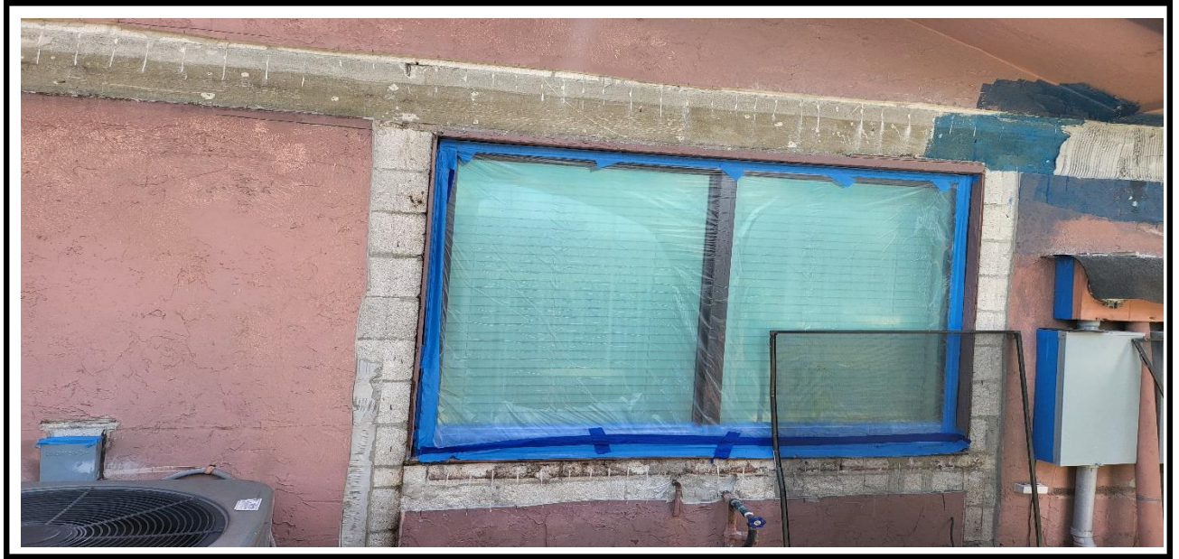
1 – Ongoing, Removal of old wood and Chipping of the deteriorated stucco on exterior walls, BLDG 17.
