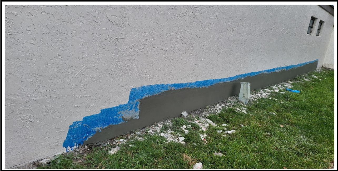
5 – Ongoing, Application of the new stucco at the exterior walls, BLDG 23.
