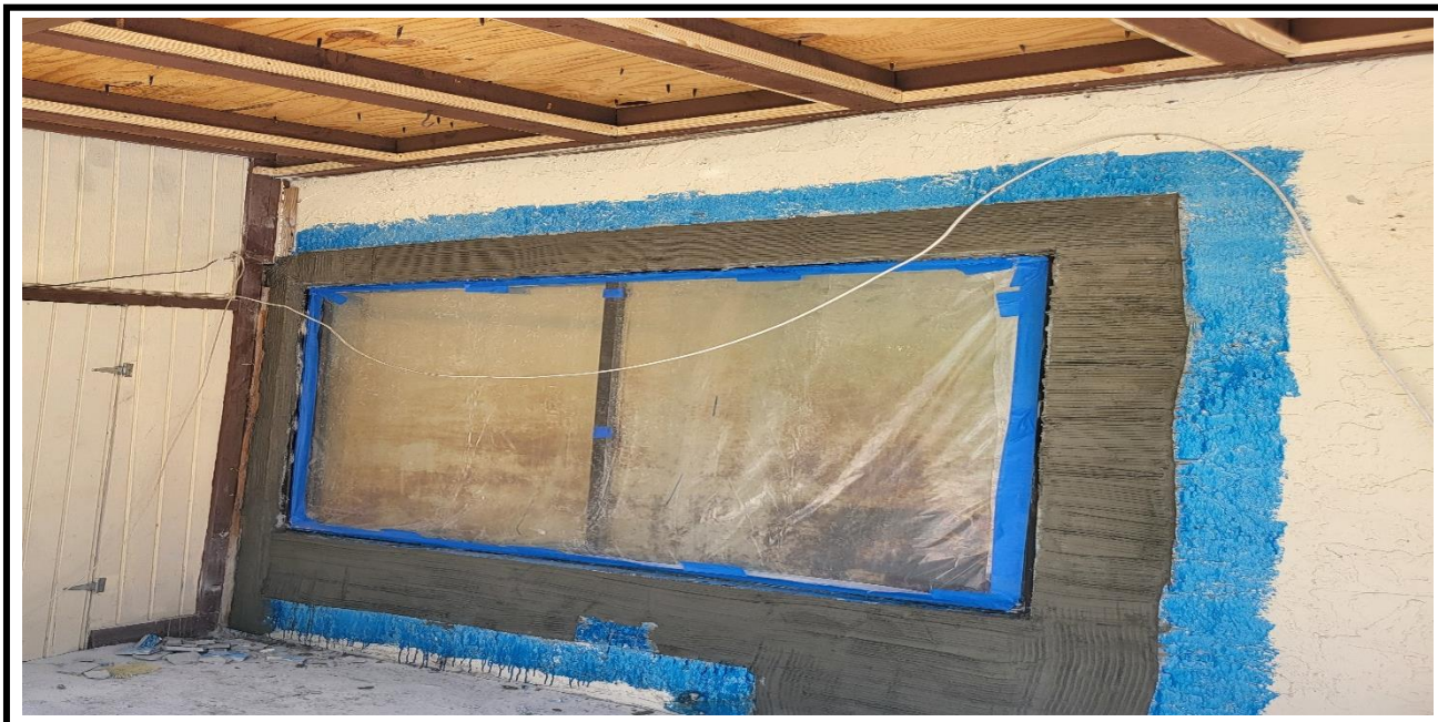
3 – Ongoing, Application of the new stucco at the exterior walls, around the window's perimeter, BLDG 24.
