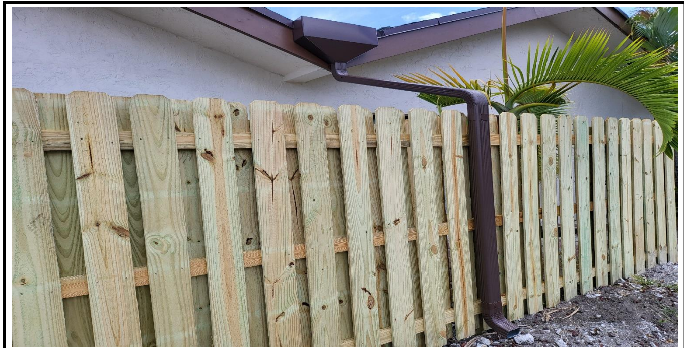
12 - Ongoing, Application of the new primer and paint at the exterior walls, BLDG 21.
