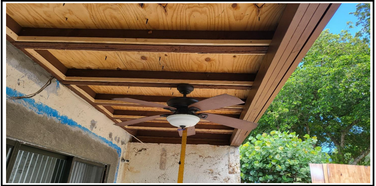
7 – Ongoing, Installation of the wooden ceiling at the back of the building, BLDG 24.
