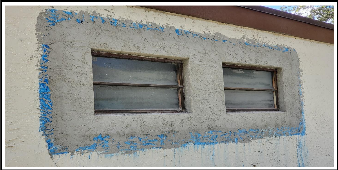
6 – Ongoing, Application of the new stucco at the exterior walls, around the window's perimeter, BLDG 24.
