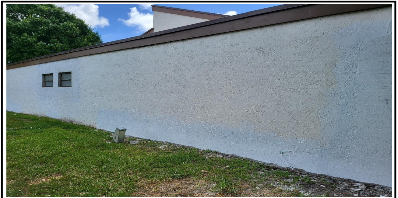
8 – Ongoing, Application of the new primer and paint at the exterior walls, BLDG 24.
