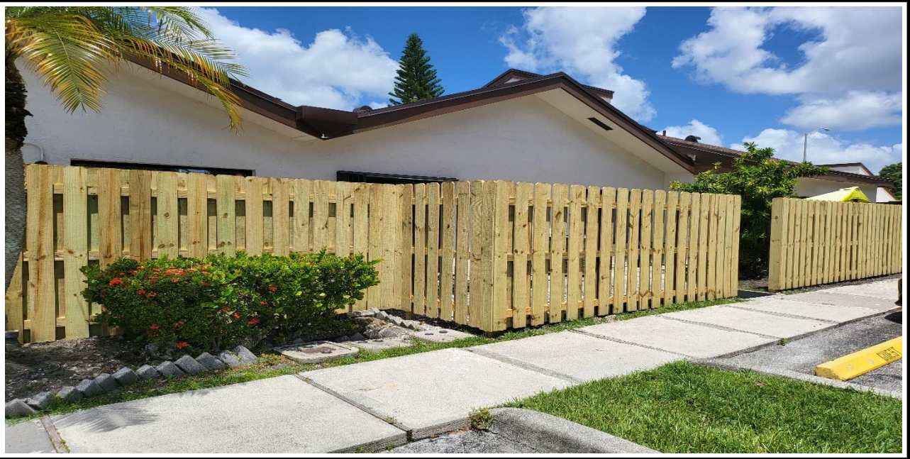
12 – Ongoing, installation of the wooden fence, BLDG 20.
