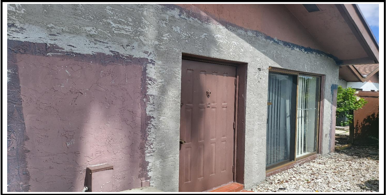
8 – Ongoing, application of the new stucco on the exterior walls, BLDG 17.
