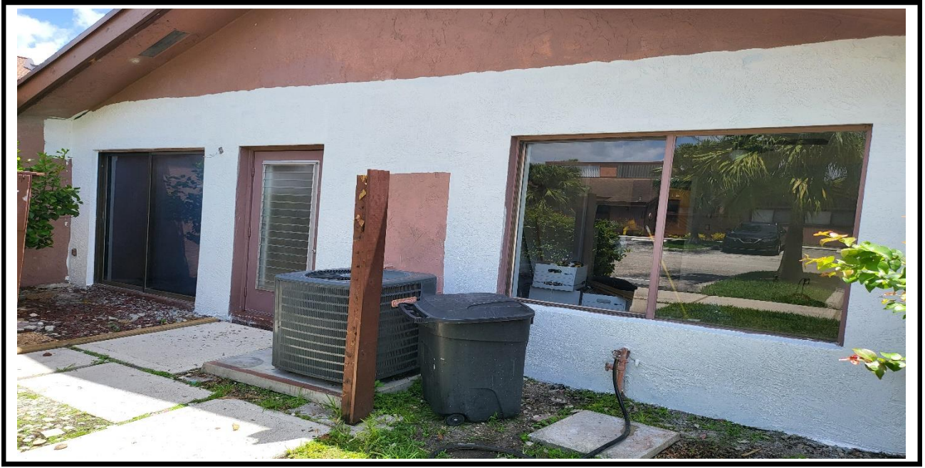
9 – Ongoing, application of the primer paint at exterior walls, BLDG 17.
