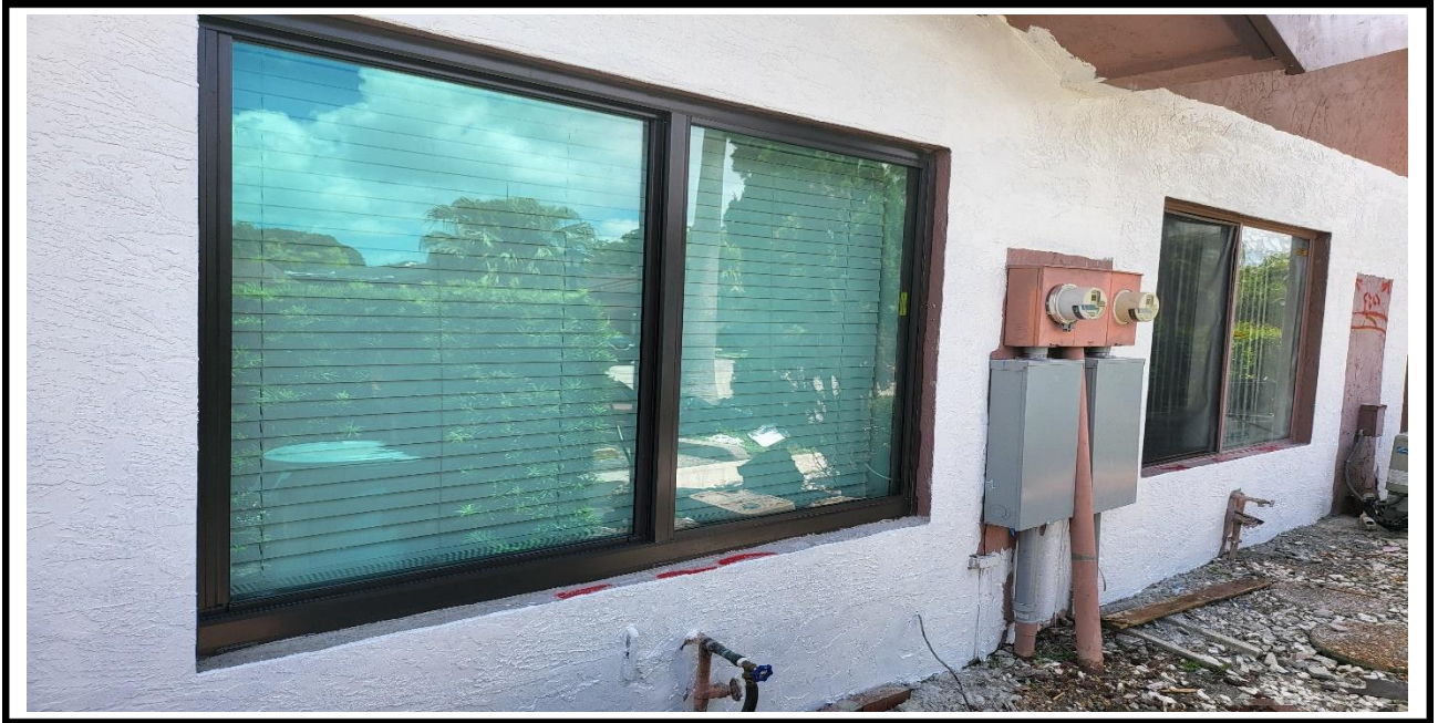
10 – Ongoing, application of the primer paint at exterior walls, BLDG 17.
