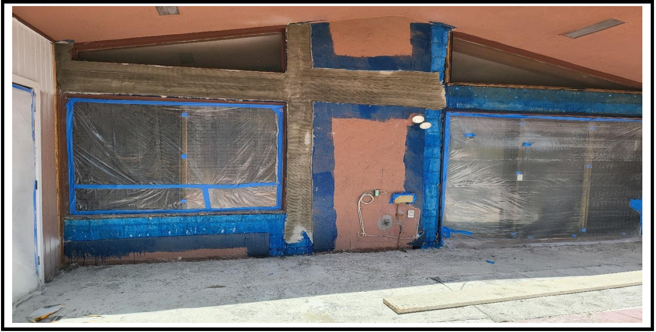
3 – Ongoing, application of the new stucco on the exterior walls, BLDG 17.
