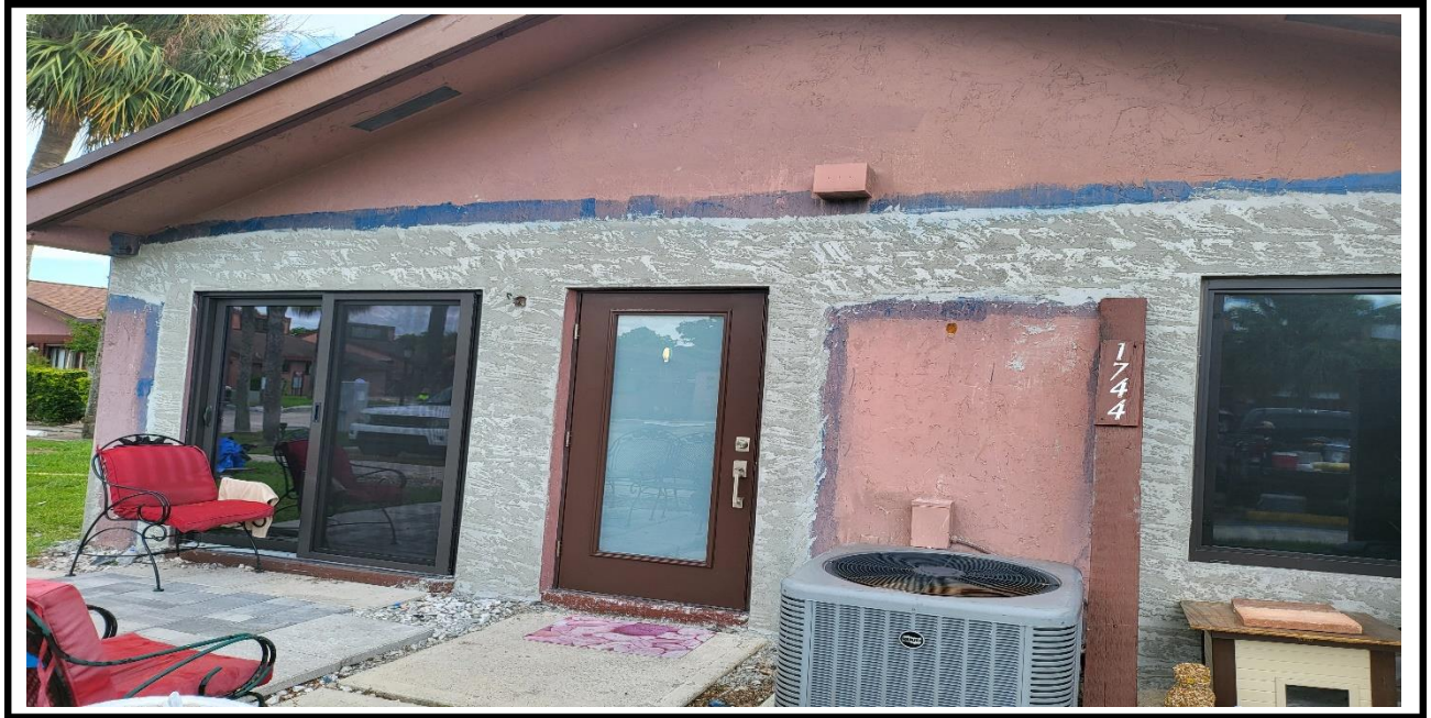
6 – Ongoing, application of the new stucco on the exterior walls, BLDG 17.
