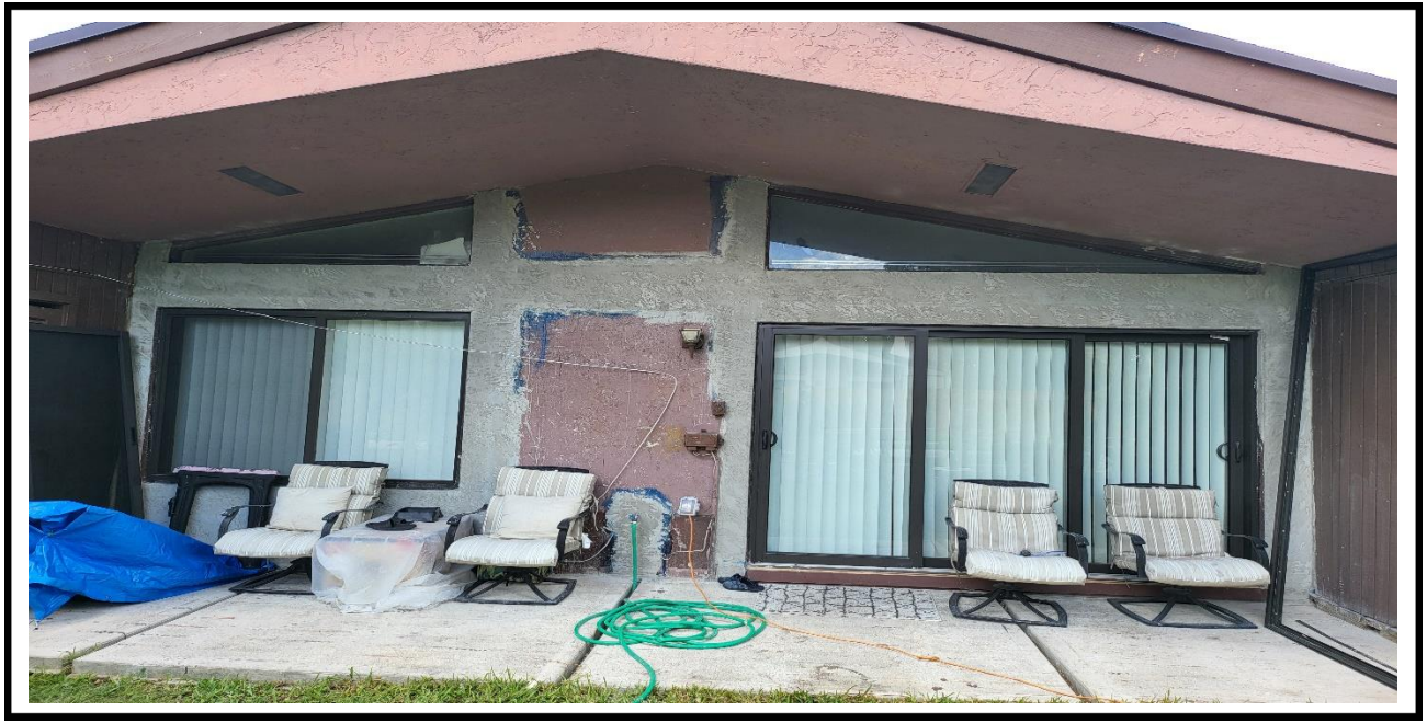
5 – Ongoing, application of the new stucco on the exterior walls, BLDG 17.
