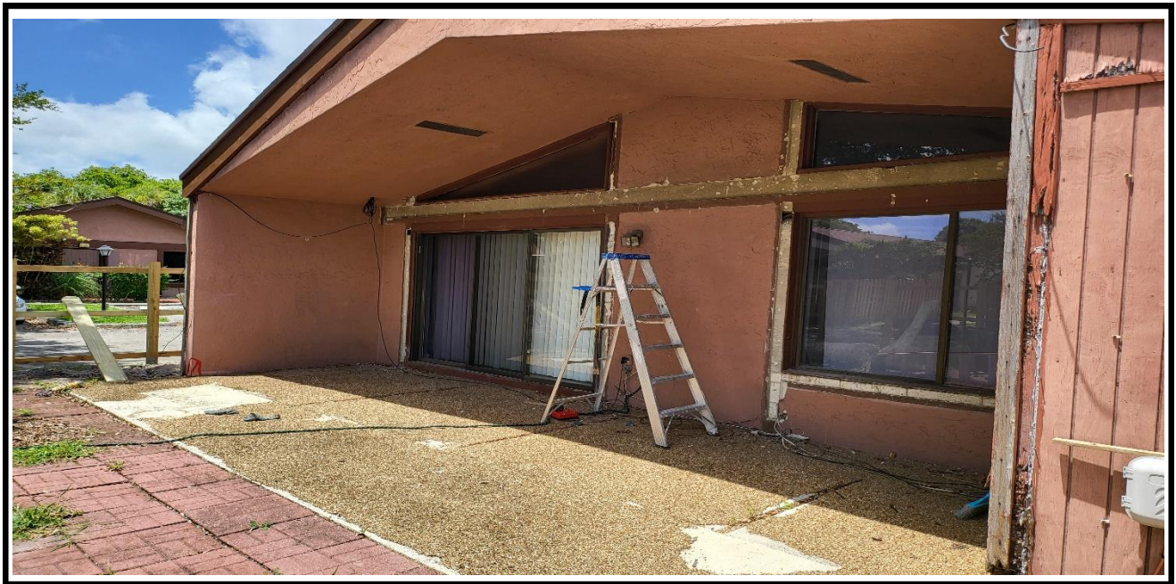
2 – Ongoing, chipping of the delaminated stucco at exterior wall, BLDG 17.
