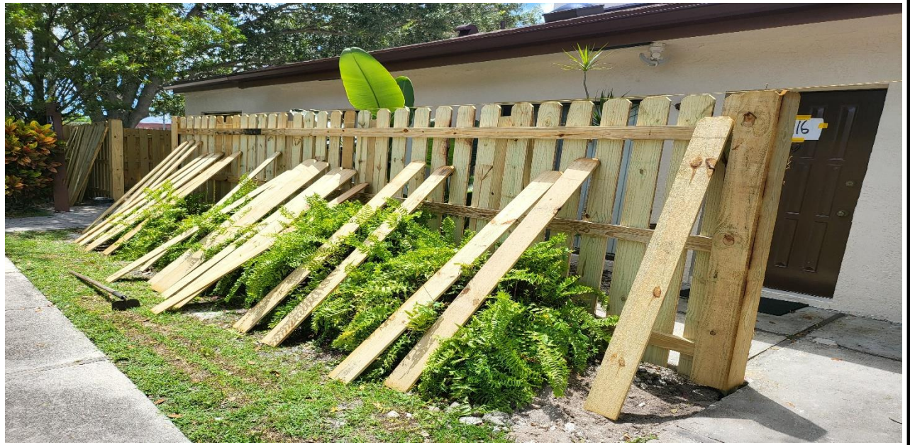
11 – Ongoing, installation of the wooden fence, BLDG 24.
