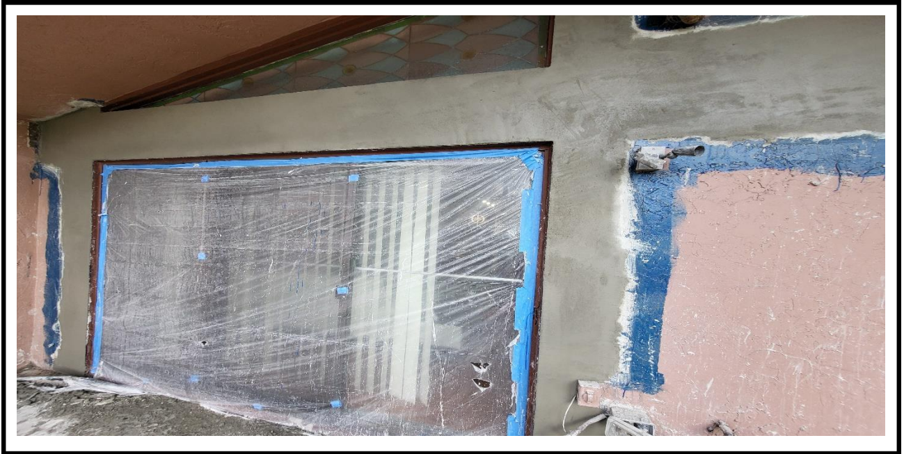
4 – Ongoing, application of the new stucco on the exterior walls, BLDG 17.
