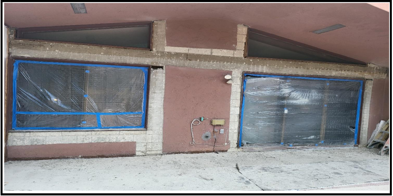
1 – Ongoing, chipping of the delaminated stucco at exterior wall, BLDG 17.
