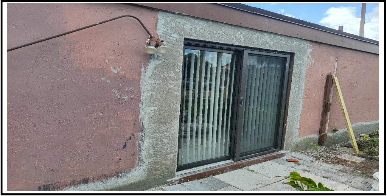
7 – Ongoing, application of the new stucco on the exterior walls, BLDG 17.
