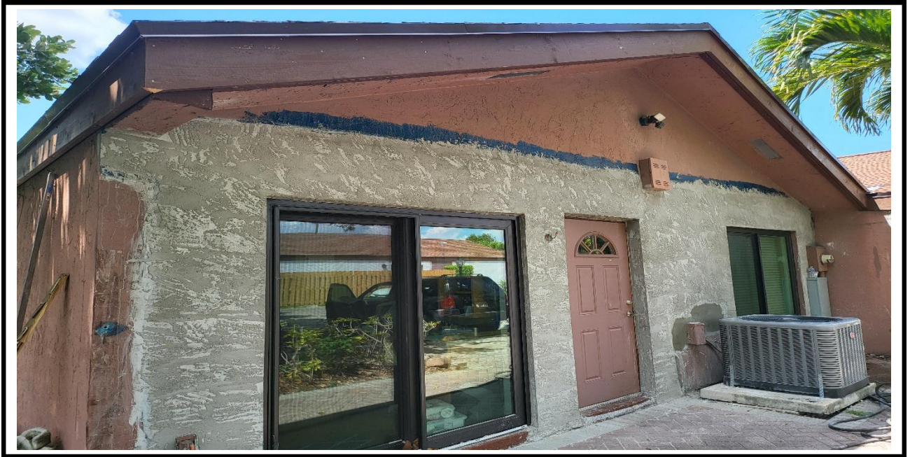
6 – Ongoing, application of the new stucco on the exterior walls, BLDG 18.
