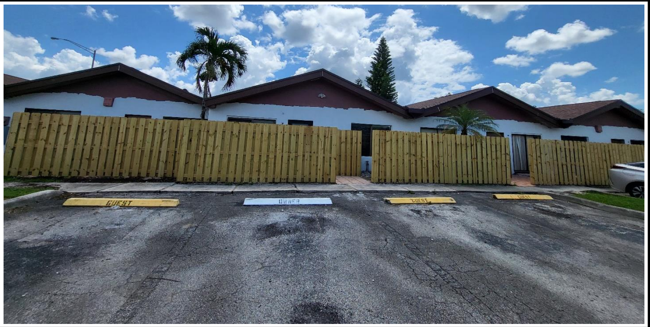
10– Ongoing, installation of the wooden fence, BLDG 17.
