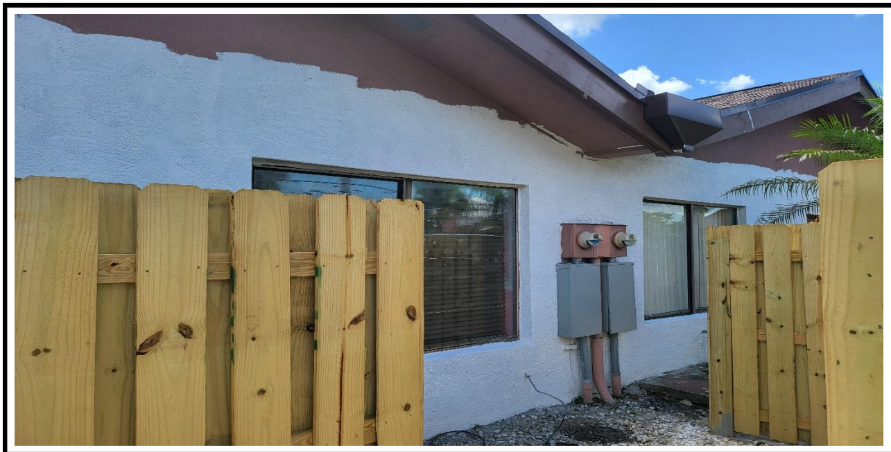
7 – Ongoing, application of the primer on the exterior walls, BLDG 18.
