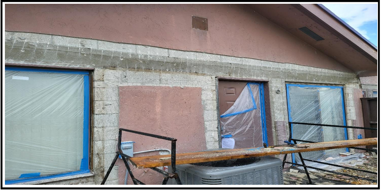
1 – Ongoing, chipping of the delaminated stucco at exterior wall, BLDG 18.
