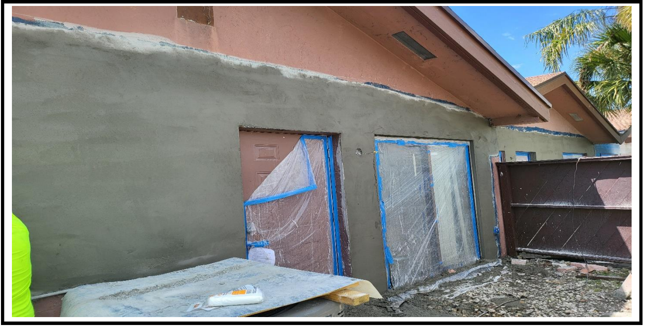
5 – Ongoing, application of the new stucco on the exterior walls, BLDG 18.
