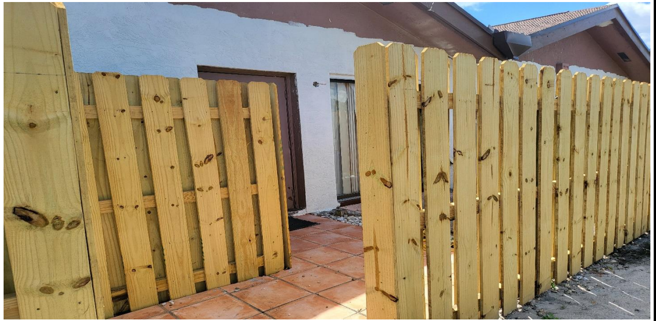
9 – Ongoing, installation of the wooden fence, BLDG 17.
