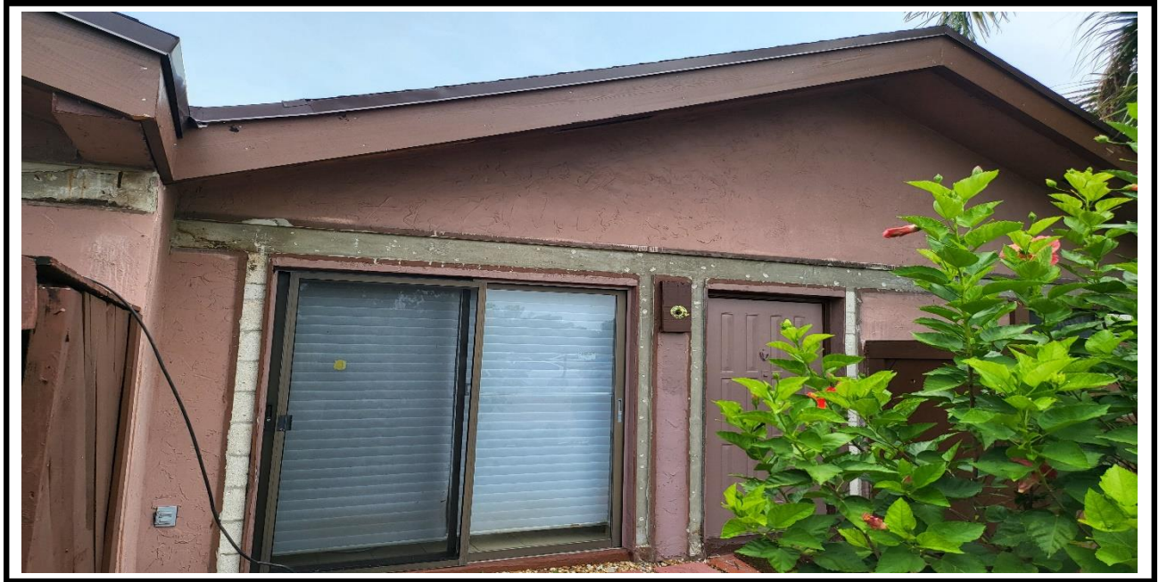
4 – Ongoing, removal of the wood trims around the windows and doors at the exterior walls, BLDG 18.
