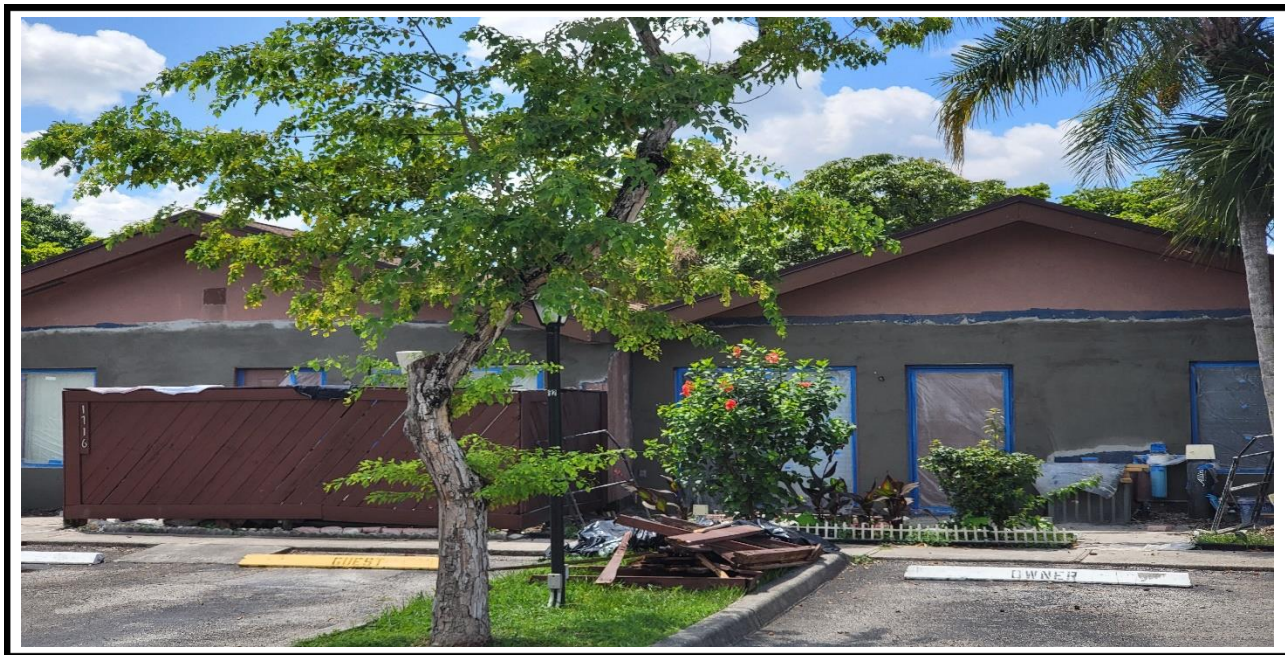
8 – Ongoing, application of the new stucco on the exterior walls, BLDG 18.
