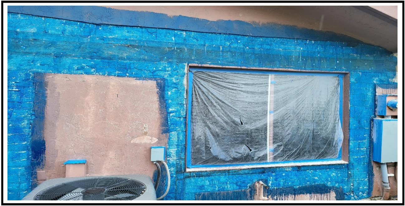
3 – Ongoing, application of the bonding agent prior to application of new stucco on the exterior walls, BLDG 18.
