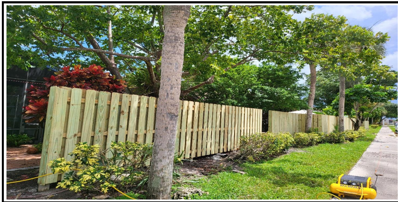
10– Ongoing, installation of the wooden fence, BLDG 18.
