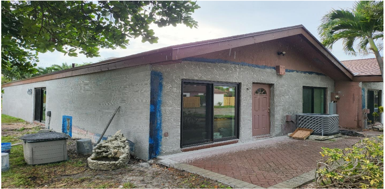
7 – Ongoing, application of the new stucco on the exterior walls, BLDG 18.
