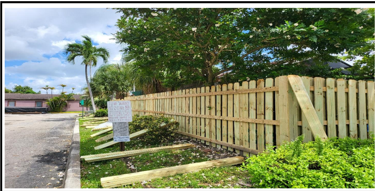
9 – Ongoing, installation of the wooden fence, BLDG 18.
