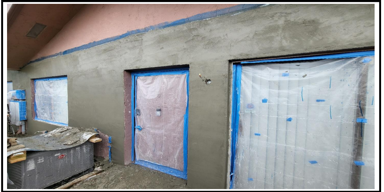
4 – Ongoing, application of the new stucco on the exterior walls, BLDG 18.
