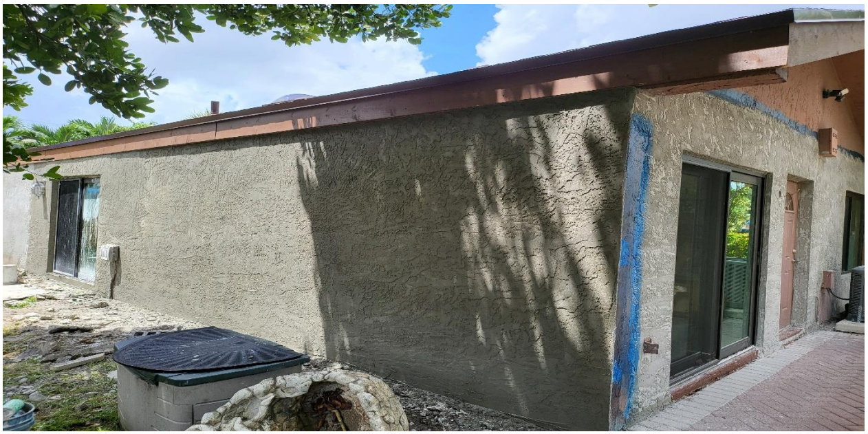
8 – Ongoing, application of the new stucco on the exterior walls, BLDG 18.
