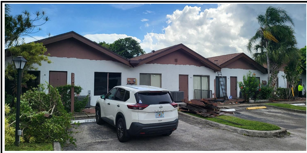
1 – Ongoing, application of the primer paint on the exterior walls, BLDG 18.
