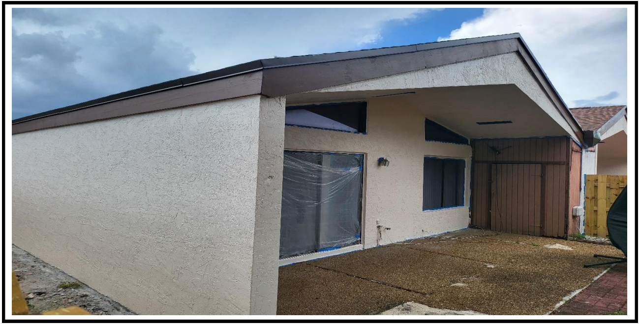
3 – Ongoing, application of the primer paint on the exterior walls, BLDG 17.
