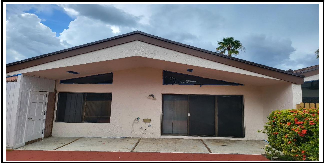
4 – Ongoing, application of the primer paint on the exterior walls, BLDG 17.
