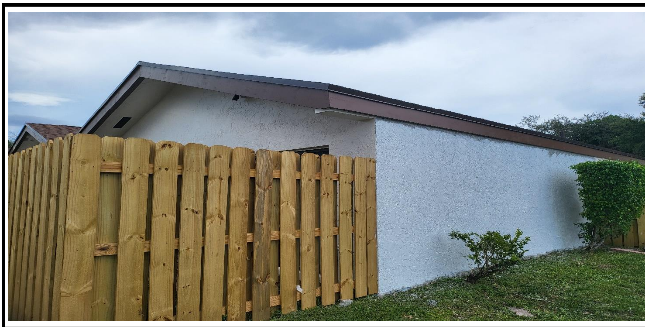
2 – Ongoing, application of the primer paint on the exterior walls, BLDG 17.
