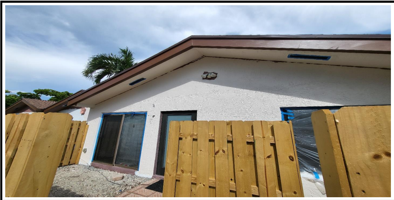
5 – Ongoing, application of the primer paint on the exterior walls, BLDG 16.
