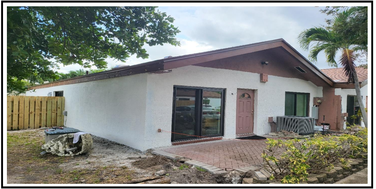
7 – Ongoing, application of the Caulking, Primer and Paint on the exterior walls, BLDG 18.
