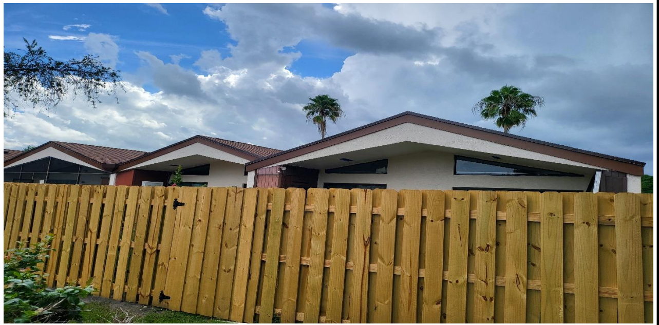
9 – Ongoing, installation of the wooden fence, BLDG 17.
