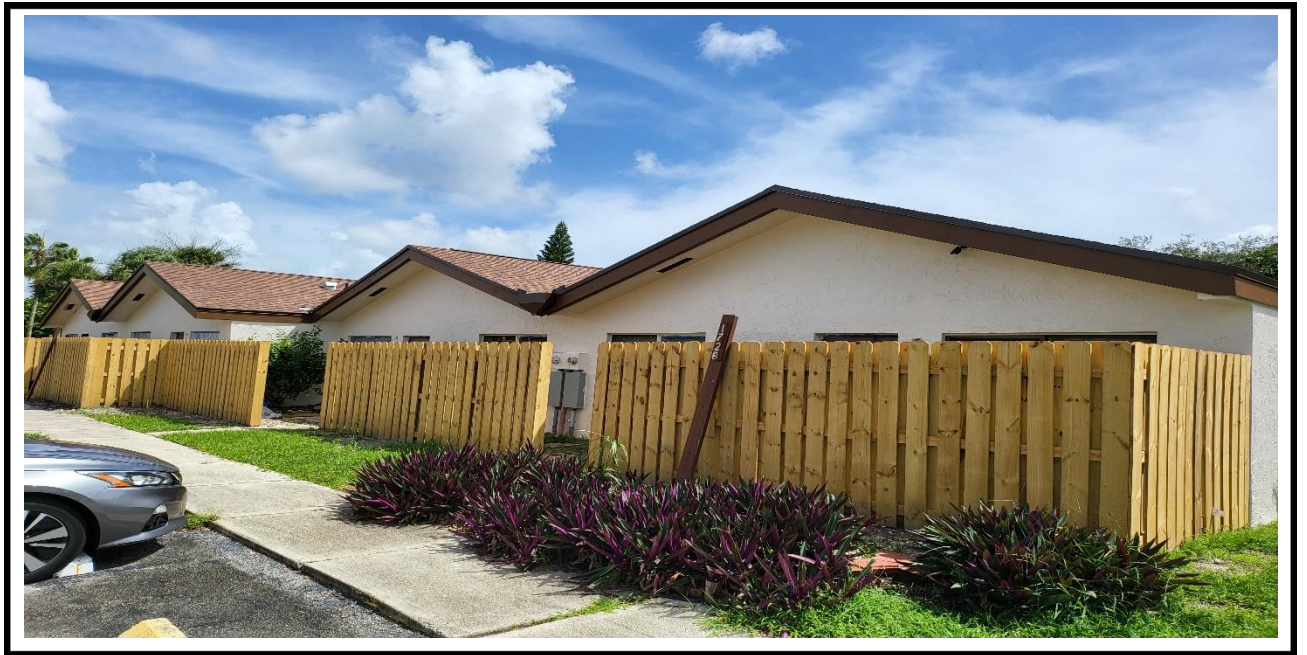
8 – Ongoing, application of the Caulking, Primer and Paint on the exterior walls, BLDG 17.
