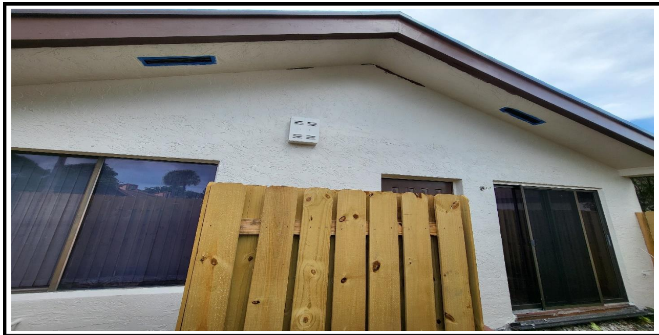
6 – Ongoing, application of the primer paint on the exterior walls, BLDG 16.
