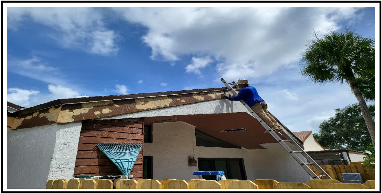
3 – Ongoing, application of the wood filler at fascia board, BLDG 18.
