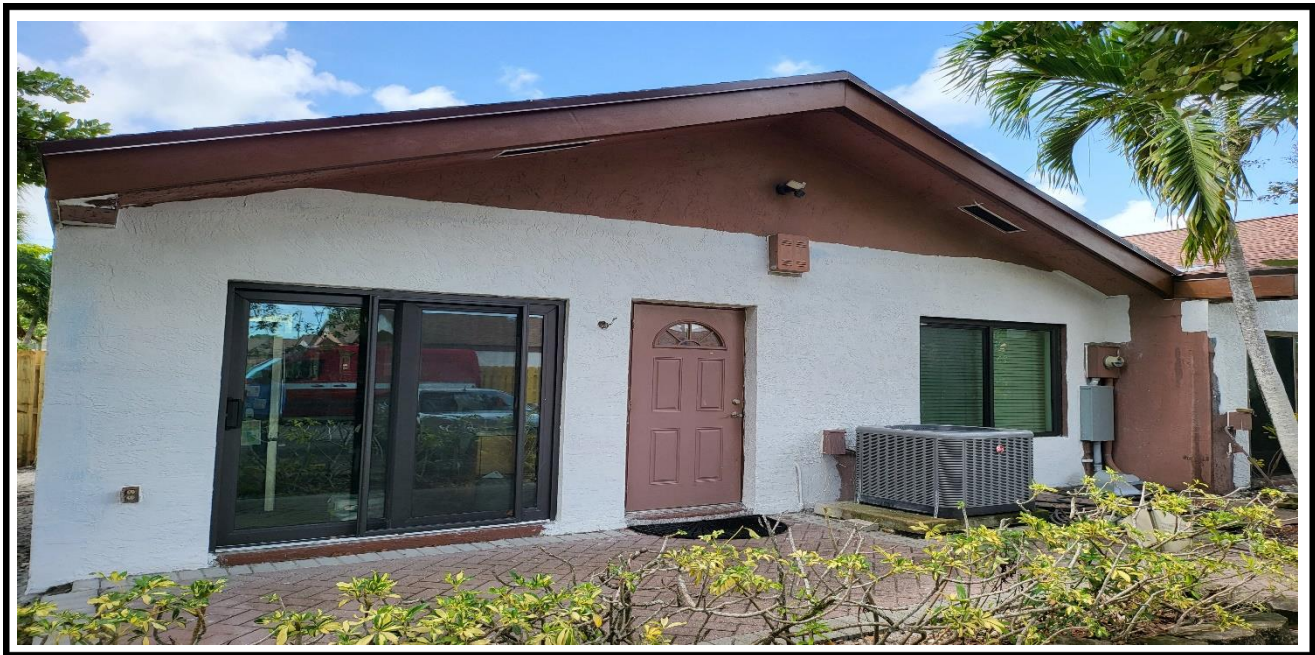
2 – Ongoing, application of the primer paint on the exterior walls, BLDG 18.
