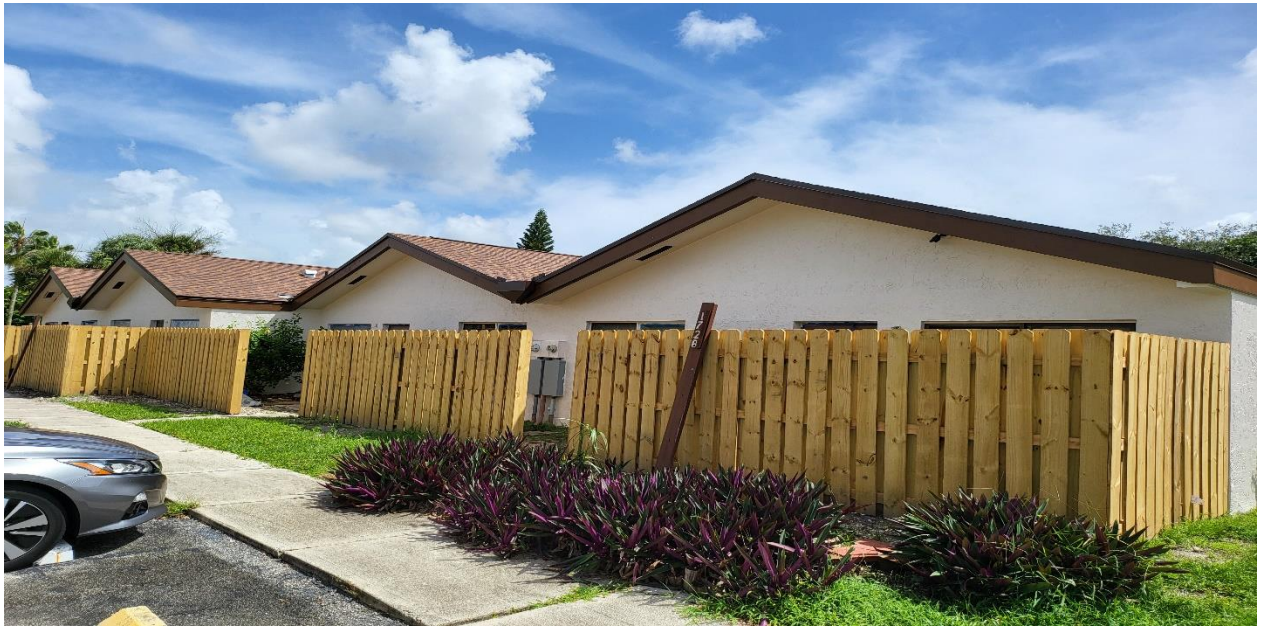
7 – Ongoing, application of the Caulking, Primer and Paint on the exterior walls, BLDG 17.
