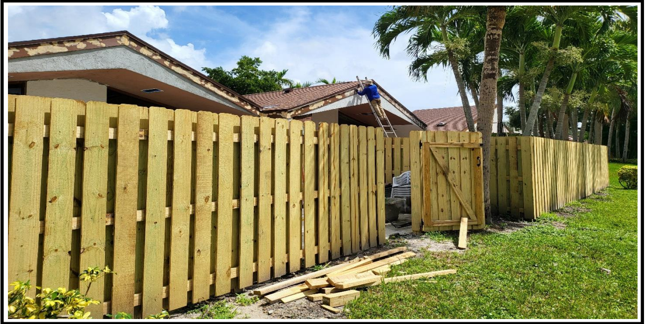
10– Ongoing, installation of the wooden fence, BLDG 18.
