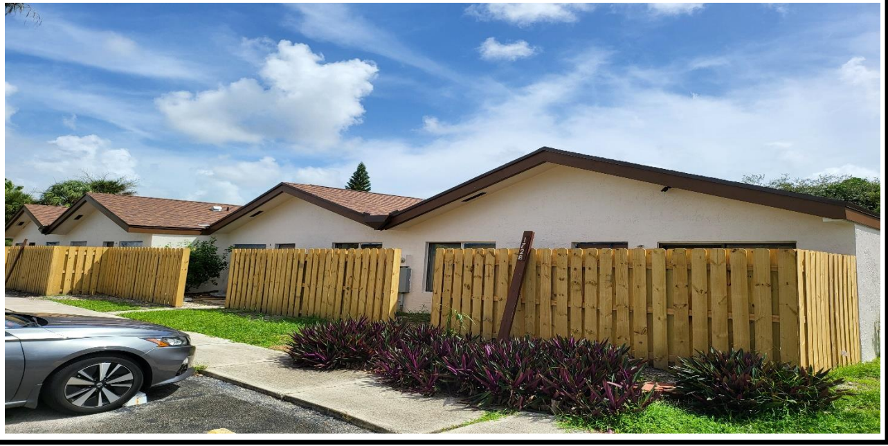
9 – Ongoing, installation of the wooden fence, BLDG 17.
