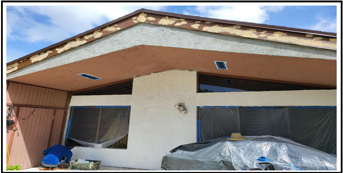
4 – Ongoing, application of the wood filler at fascia board, BLDG 18.
