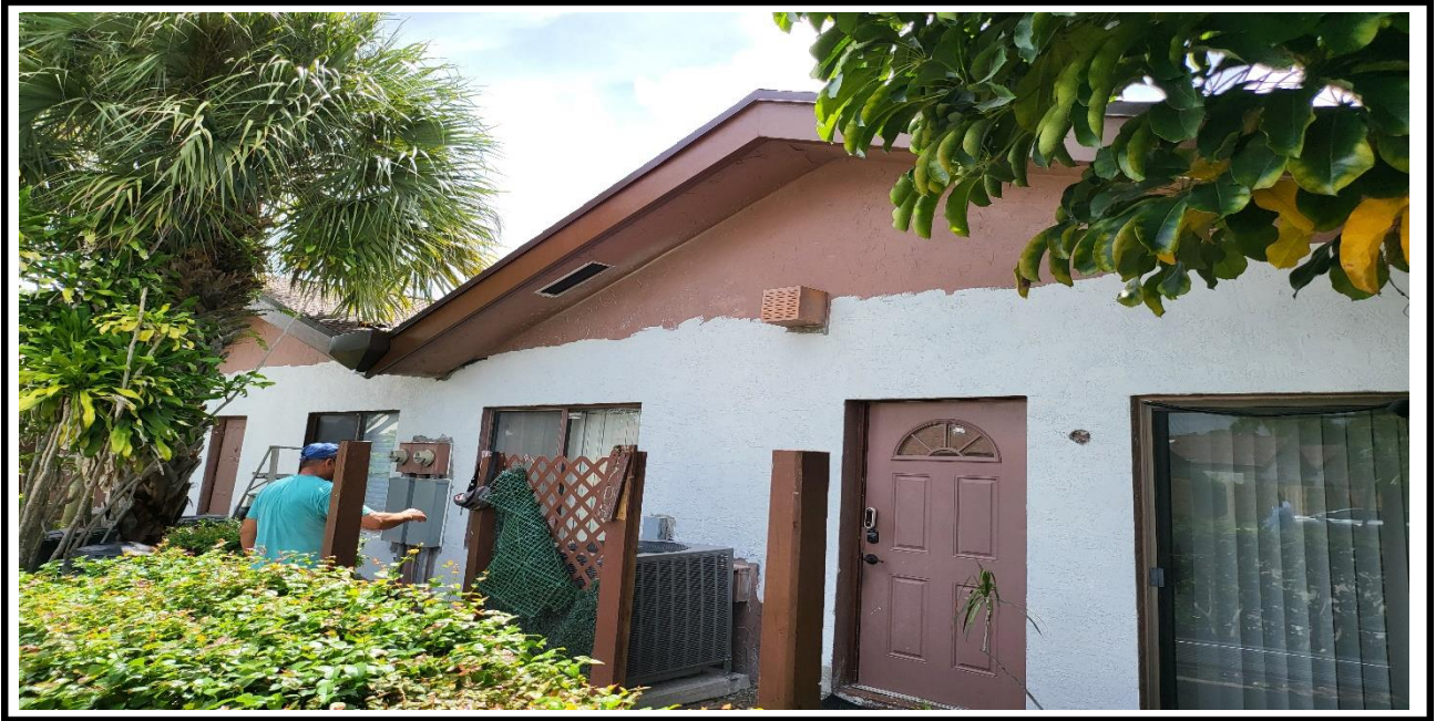
6 – Ongoing, application of the primer paint on the exterior walls, BLDG 18.
