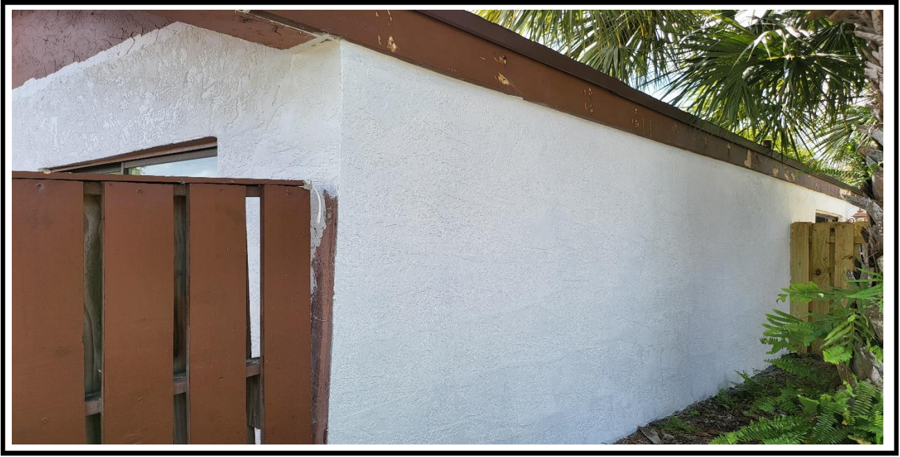
5 – Ongoing, application of the primer paint on the exterior walls, BLDG 18.
