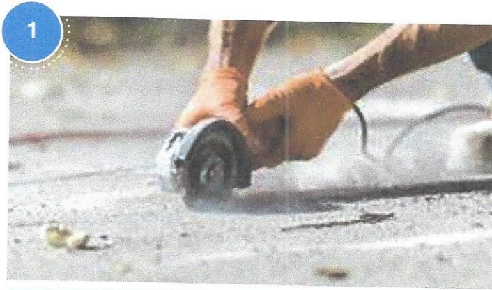
Grind, rout and prepare cracks and joints.
