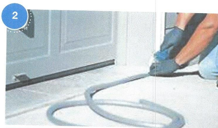
Fill large, deep cracks and joints with flexible foam backer rod.
