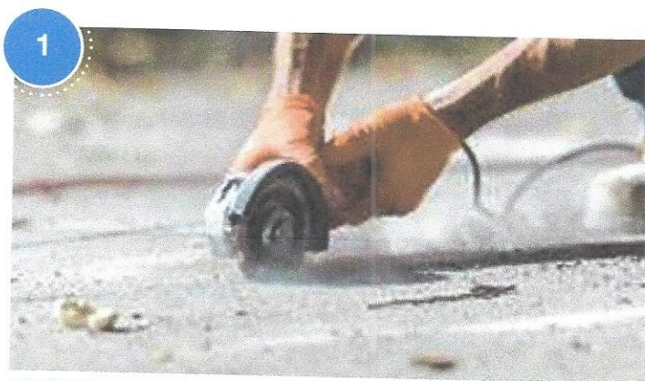
Grind, rout and prepare cracks and joints.
