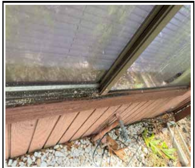
Photo 4 : Existing non-impact-rated window frame
