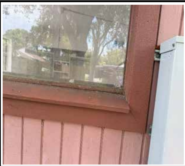
Photo 3 : Existing non-impact-rated window frame
