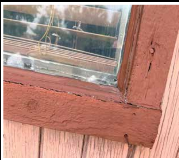
Photo 3 : Existing non-impact-rated window frame
