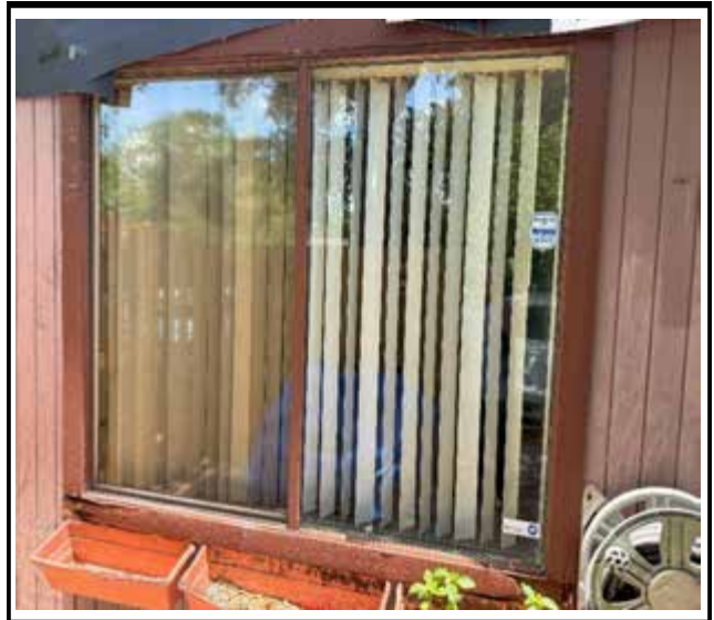
Photo 2 : Existing non-impact-rated window frame
