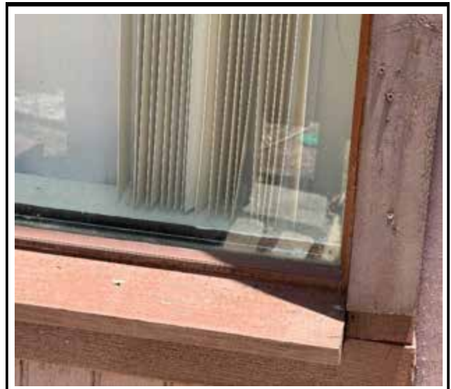
Photo 4 : Existing non-impact-rated window frame
