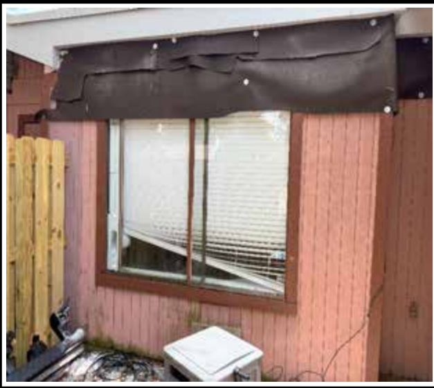
Photo 1 : Existing non-impact-rated window frame
