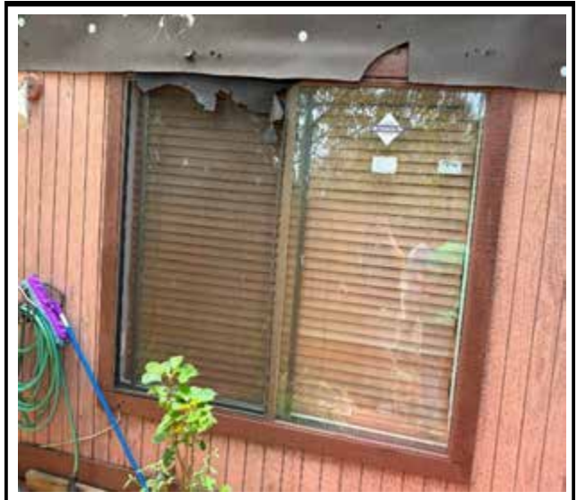
Photo 2 : Existing non-impact-rated window frame
