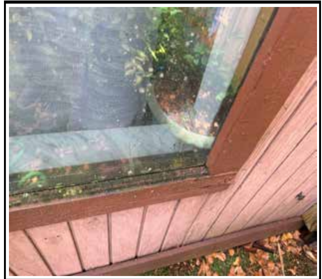
Photo 2 : Existing non-impact-rated window frame
