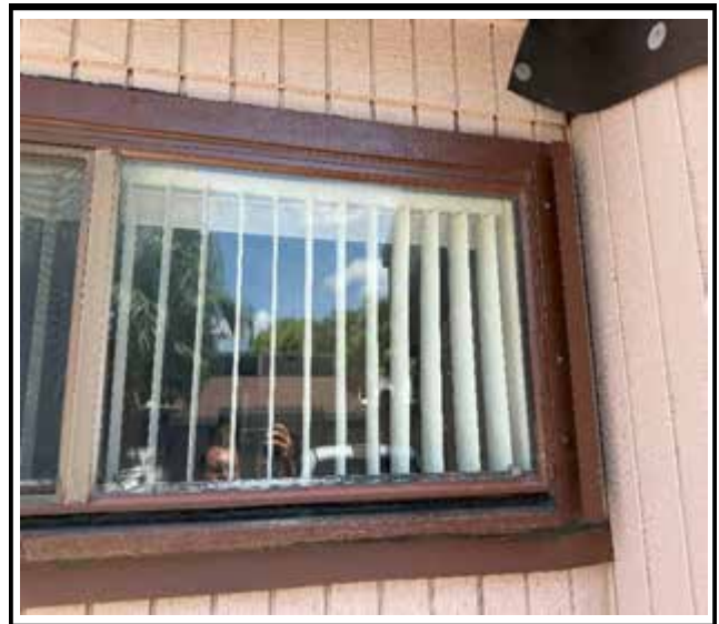
Photo 2 : Existing non-impact-rated window frame
