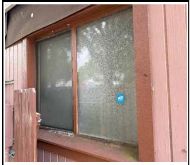
Photo 2 : Existing non-impact-rated window frame
