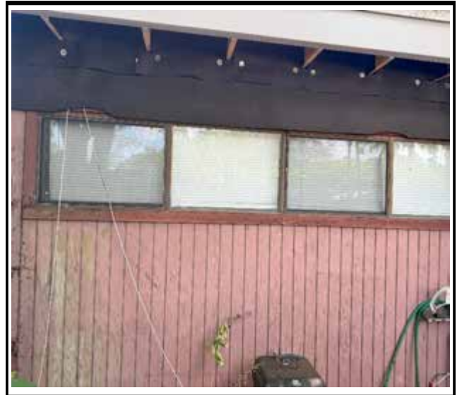
Photo 2 : Existing non-impact-rated window frame
