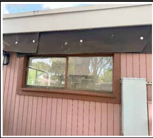
Photo 1 : Existing non-impact-rated window frame
