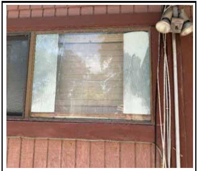
Photo 4 : Existing non-impact-rated window frame
