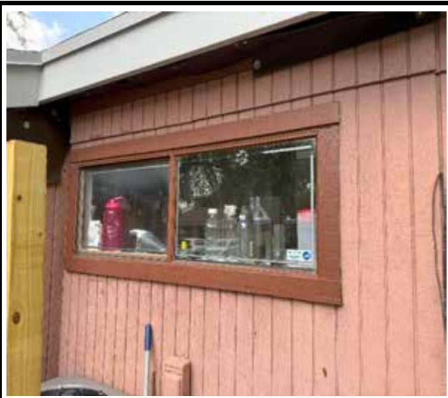
Photo 3 : Existing non-impact-rated window frame
