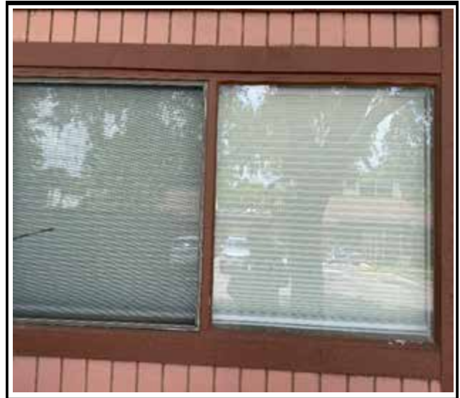
Photo 2 : Existing non-impact-rated window frame
