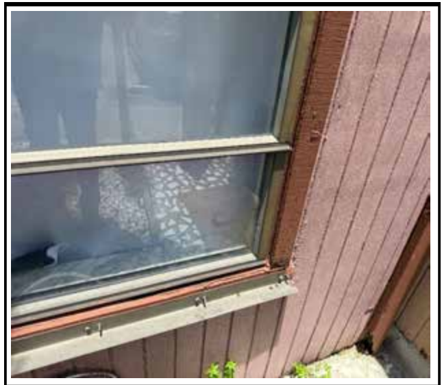
Photo 2 : Existing non-impact-rated window frame
