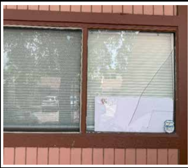
Photo 1 : Existing non-impact-rated window frame
