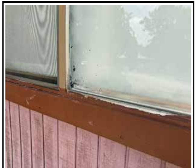
Photo 4 : Existing non-impact-rated window frame
