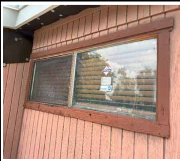
Photo 1 : Existing non-impact-rated window frame
