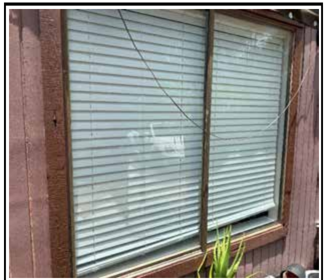
Photo 4 : Existing non-impact-rated window frame
