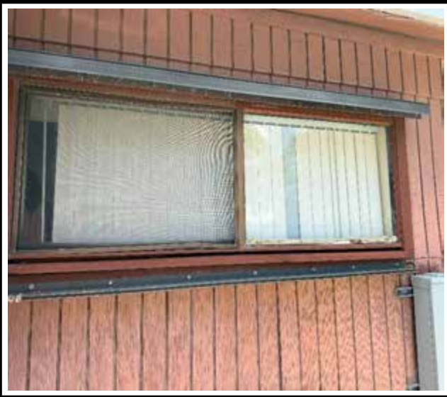
Photo 1 : Existing non-impact-rated window frame
