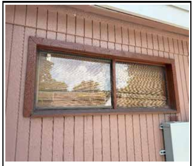
Photo 4 : Existing non-impact-rated window frame
