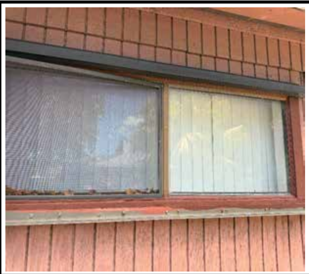
Photo 3 : Existing non-impact-rated window frame
