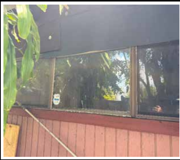
Photo 1 : Existing non-impact-rated window frame
