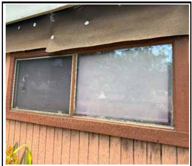
Photo 4 : Existing non-impact-rated window frame
