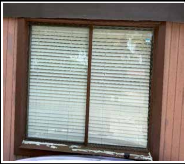
Photo 1 : Existing non-impact-rated window frame
