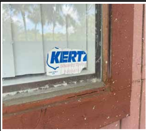
Photo 3 : Existing non-impact-rated window frame
