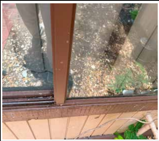
Photo 3 : Existing non-impact-rated window frame
