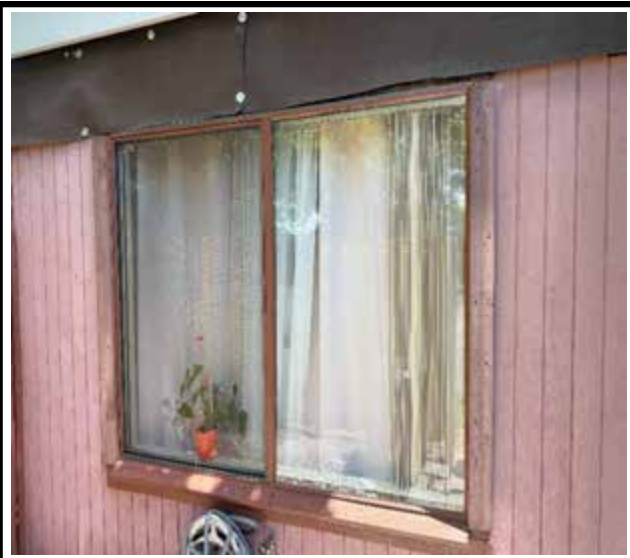
Photo 3 : Existing non-impact-rated window frame
