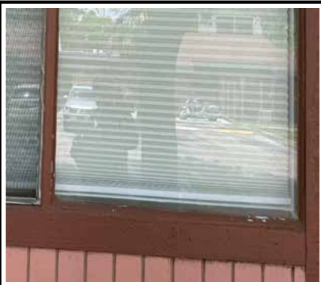
Photo 3 : Existing non-impact-rated window frame
