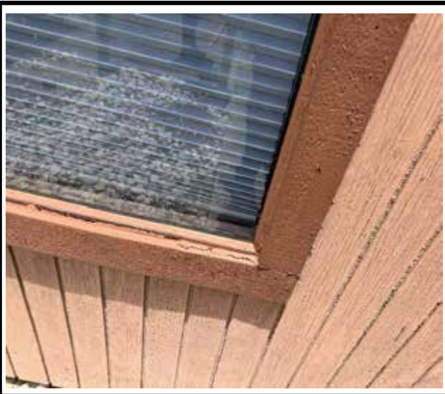
Photo 3 : Existing non-impact-rated window frame
