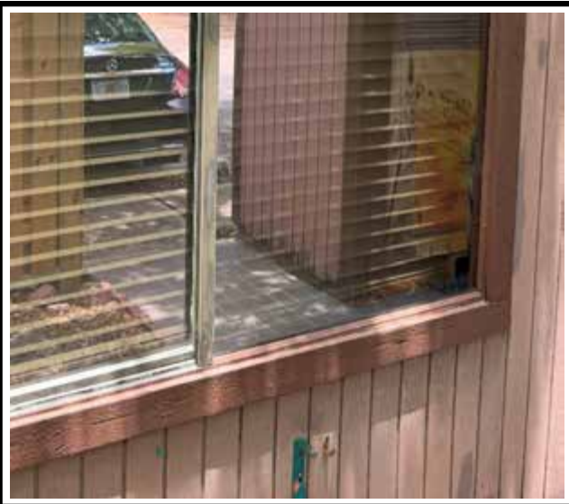
Photo 3 : Existing non-impact-rated window frame
