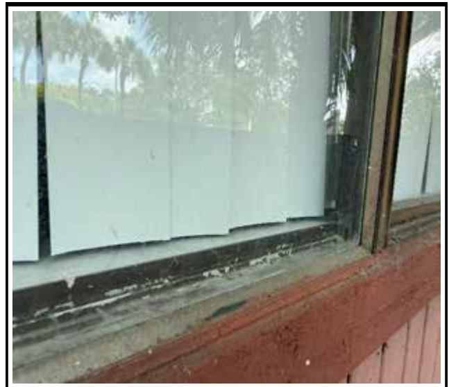
Photo 4 : Existing non-impact-rated window frame
