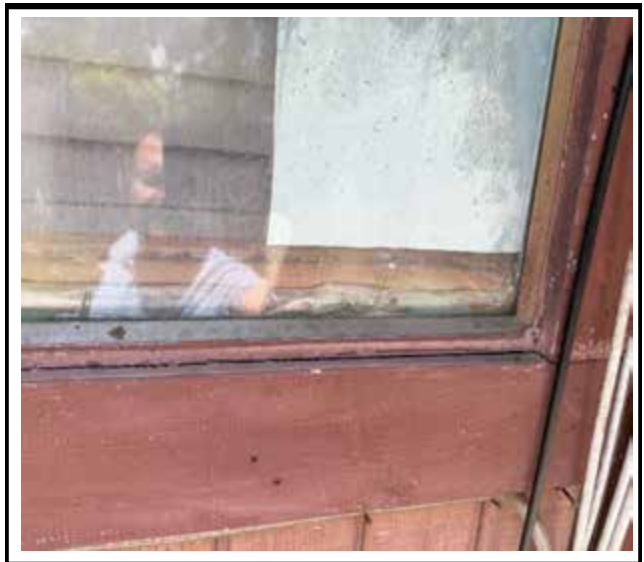
Photo 2 : Existing non-impact-rated window frame
