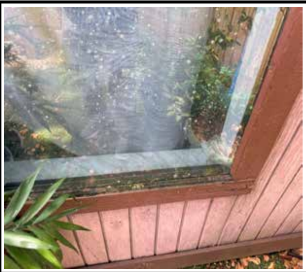
Photo 3 : Existing non-impact-rated window frame
