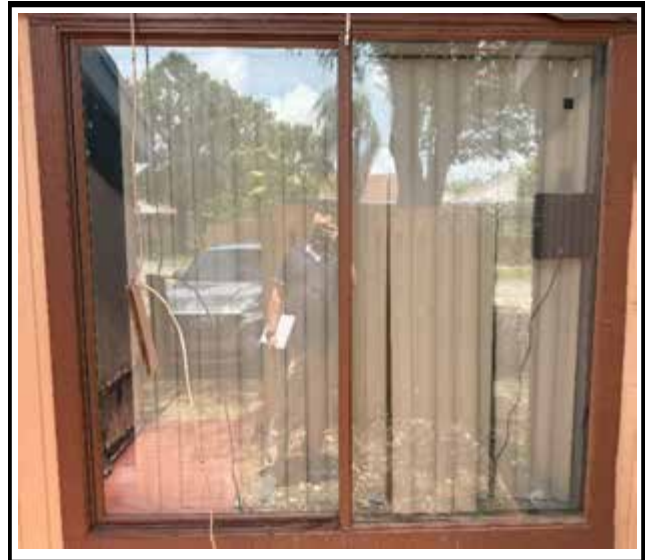
Photo 2 : Existing non-impact-rated window frame
