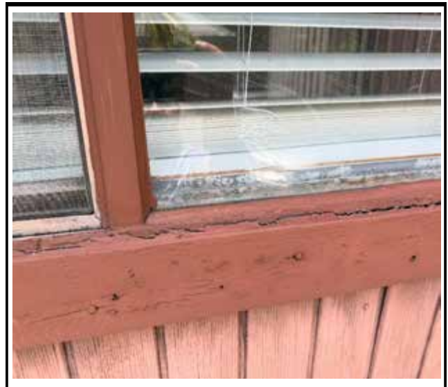
Photo 2 : Existing non-impact-rated window frame
