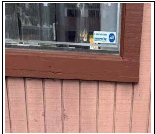
Photo 4 : Existing non-impact-rated window frame
