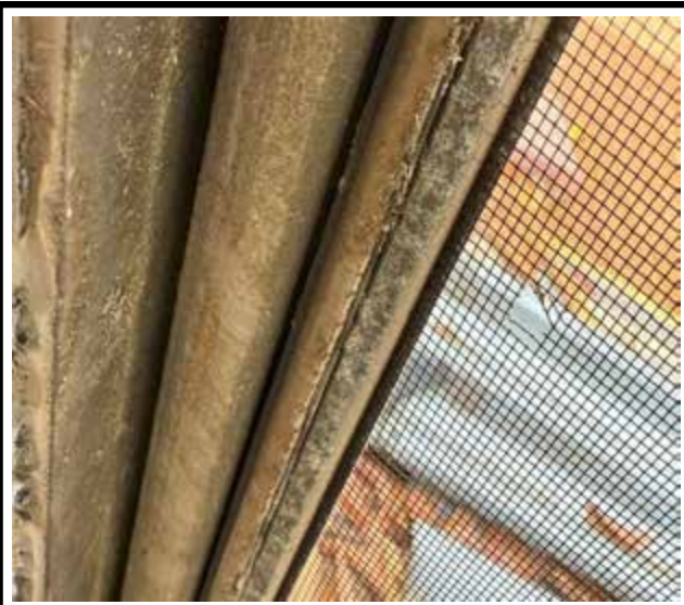
Photo 3 : Existing non-impact-rated window frame
