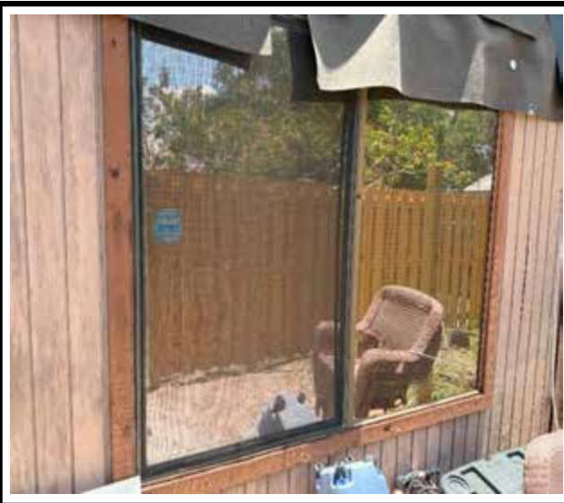
Photo 3 : Existing non-impact-rated window frame
