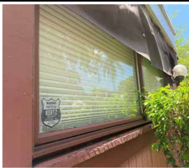
Photo 3 : Existing non-impact-rated window frame
