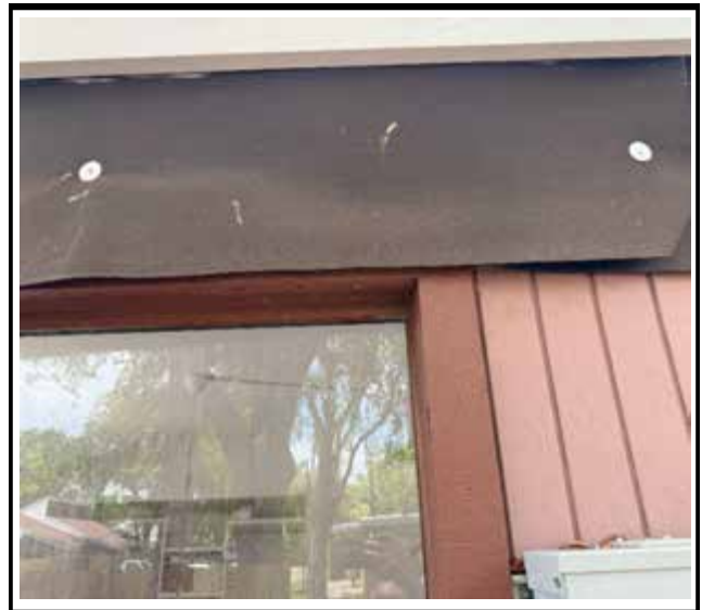
Photo 2 : Existing non-impact-rated window frame
