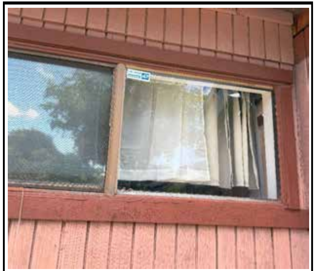
Photo 4 : Existing non-impact-rated window frame
