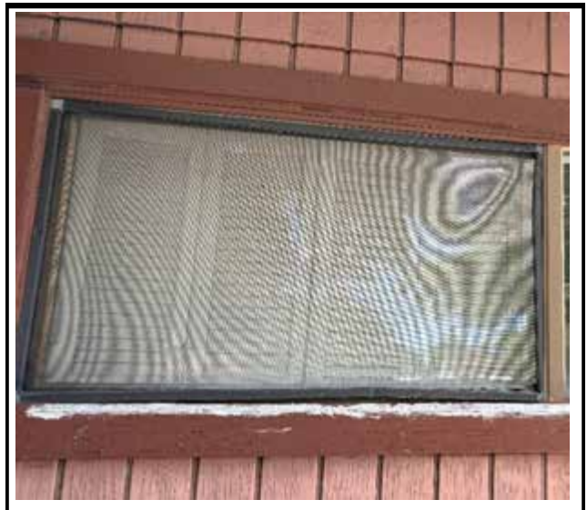
Photo 4 : Existing non-impact-rated window frame
