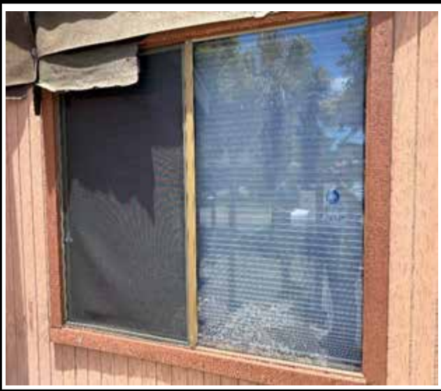
Photo 1 : Existing non-impact-rated window frame
