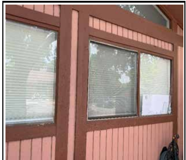
Photo 4 : Existing non-impact-rated window frame
