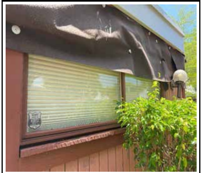
Photo 2 : Existing non-impact-rated window frame
