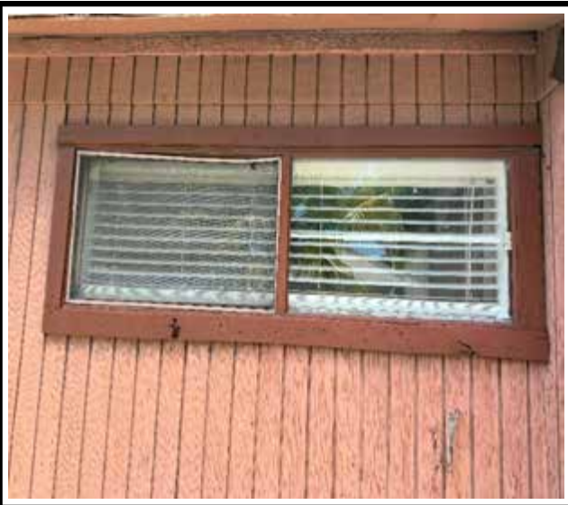
Photo 1 : Existing non-impact-rated window frame
