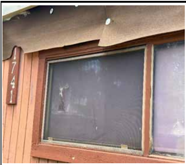
Photo 3 : Existing non-impact-rated window frame
