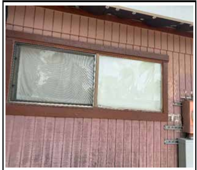
Photo 2 : Existing non-impact-rated window frame
