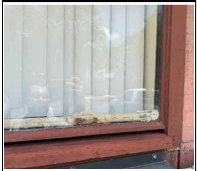
Photo 2 : Existing non-impact-rated window frame
