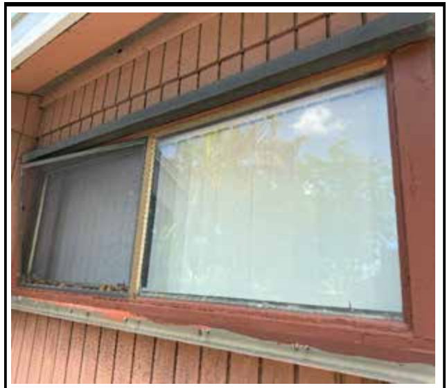
Photo 4 : Existing non-impact-rated window frame
