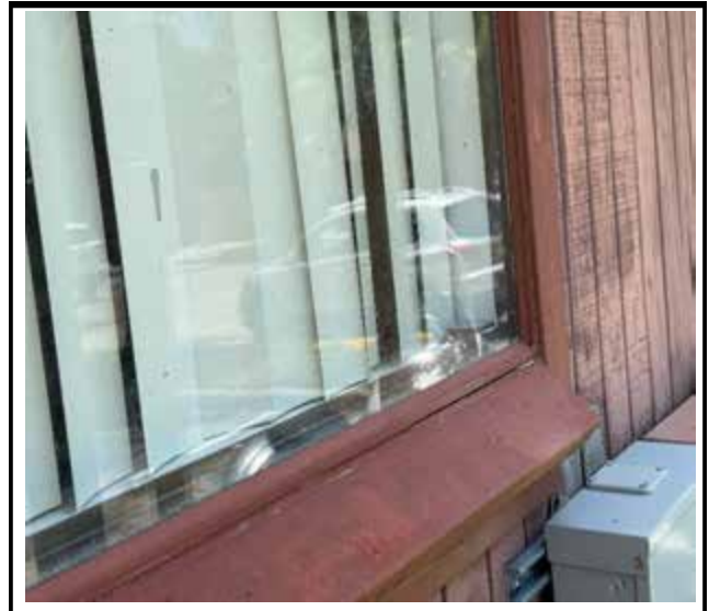
Photo 2 : Existing non-impact-rated window frame
