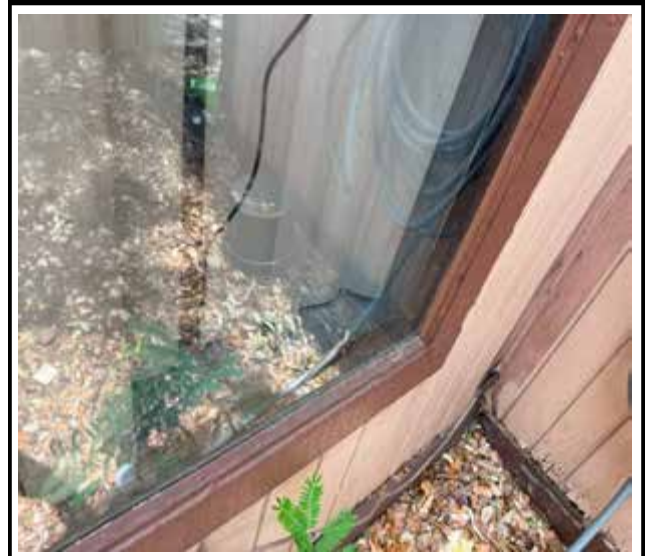
Photo 4 : Existing non-impact-rated window frame
