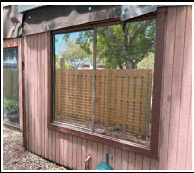
Photo 1 : Existing non-impact-rated window frame
