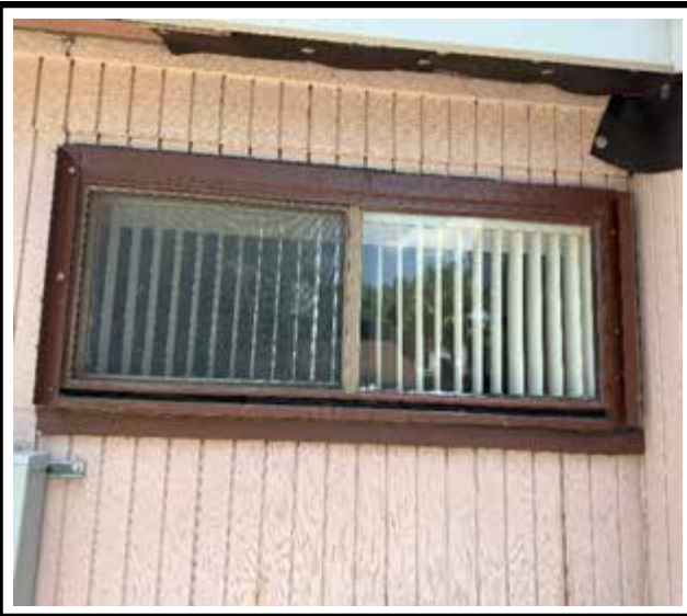
Photo 1 : Existing non-impact-rated window frame
