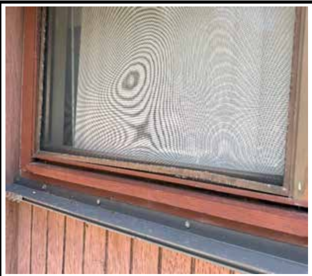
Photo 3 : Existing non-impact-rated window frame
