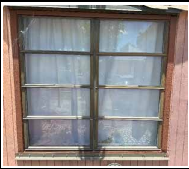
Photo 1 : Existing non-impact-rated window frame
