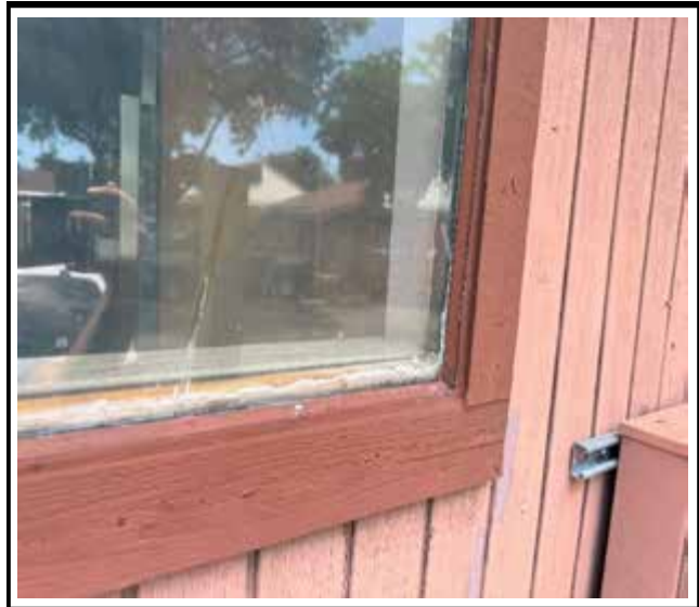
Photo 2 : Existing non-impact-rated window frame
