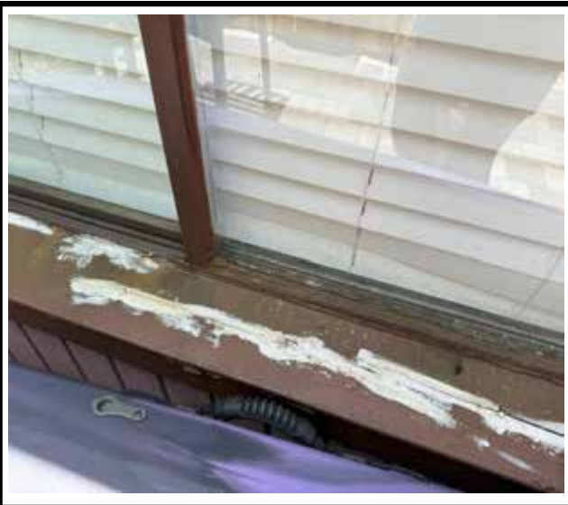
Photo 3 : Existing non-impact-rated window frame
