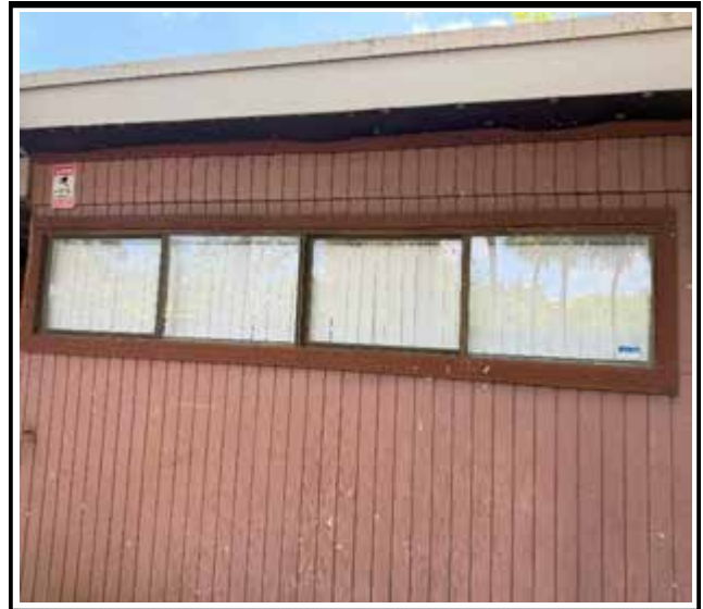
Photo 2 : Existing non-impact-rated window frame
