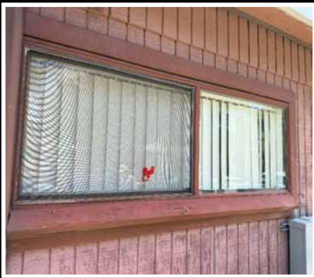
Photo 1 : Existing non-impact-rated window frame
