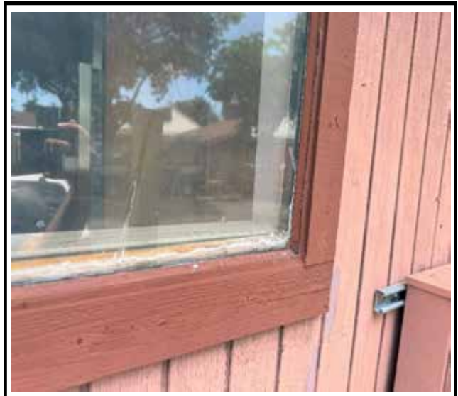
Photo 2 : Existing non-impact-rated window frame
