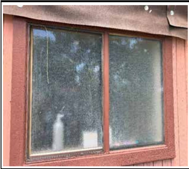
Photo 1 : Existing non-impact-rated window frame
