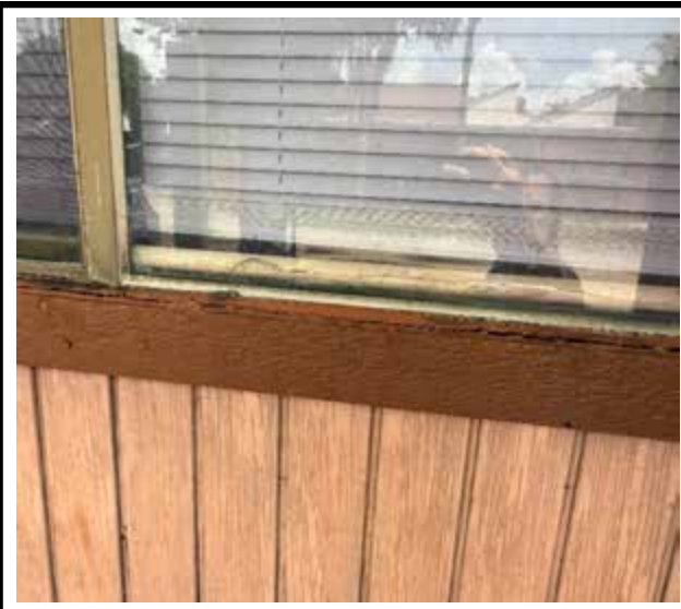
Photo 3 : Existing non-impact-rated window frame
