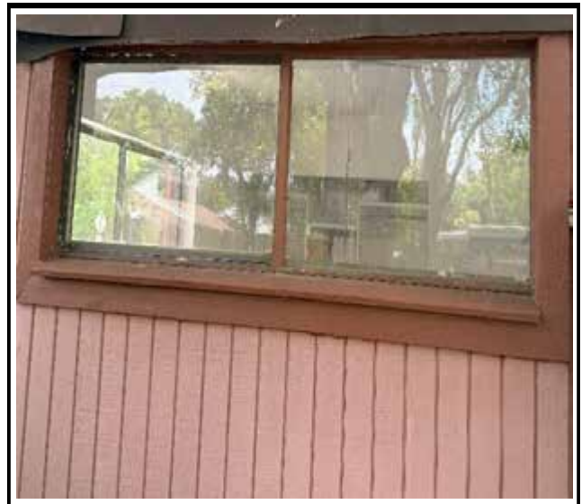
Photo 4 : Existing non-impact-rated window frame
