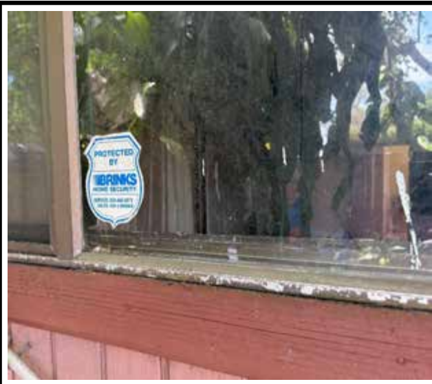
Photo 3 : Existing non-impact-rated window frame
