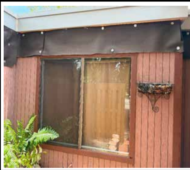
Photo 1 : Existing non-impact-rated window frame
