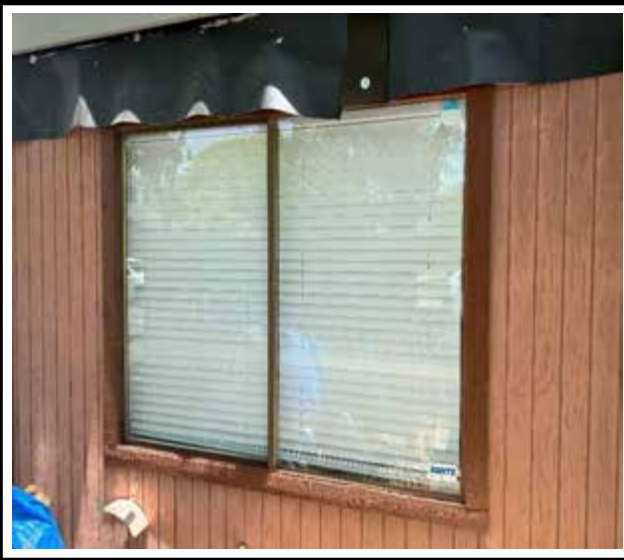
Photo 1 : Existing non-impact-rated window frame
