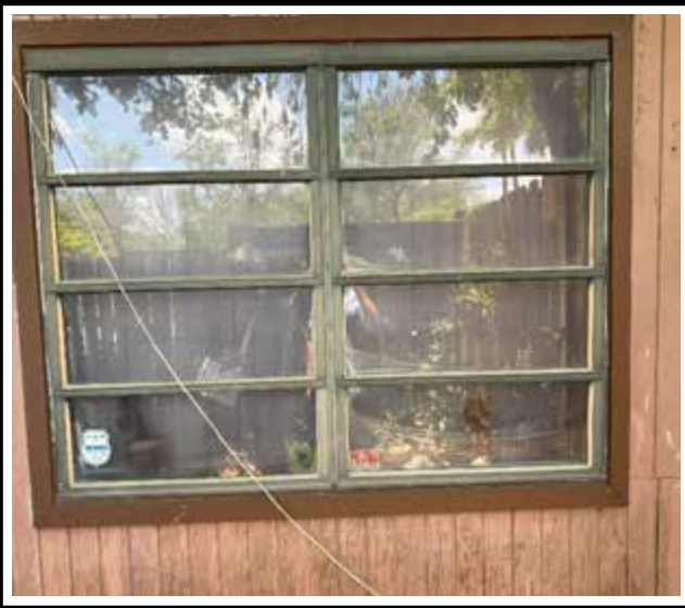
Photo 1 : Existing non-impact-rated window frame
