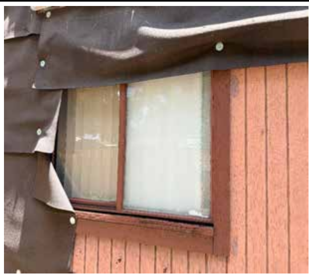
Photo 1 : Existing non-impact-rated window frame
