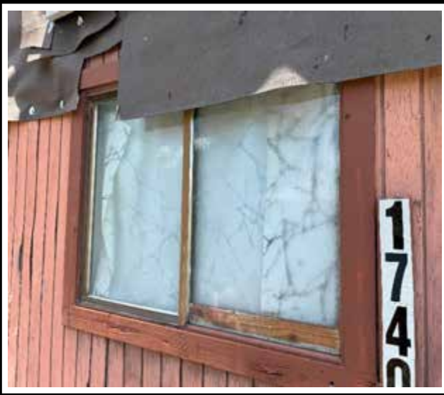
Photo 1 : Existing non-impact-rated window frame
