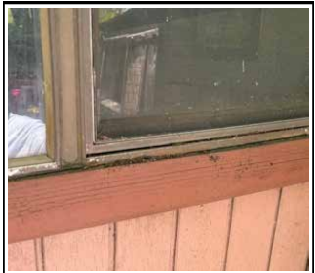
Photo 4 : Existing non-impact-rated window frame
