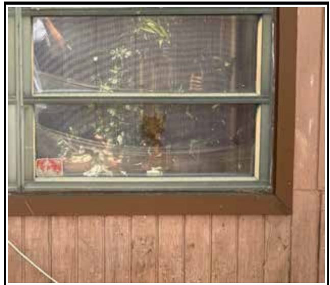
Photo 4 : Existing non-impact-rated window frame
