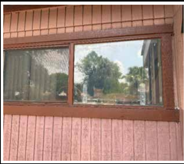
Photo 1 : Existing non-impact-rated window frame
