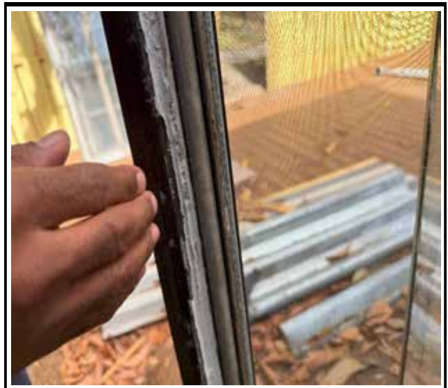
Photo 4 : Existing non-impact-rated window frame
