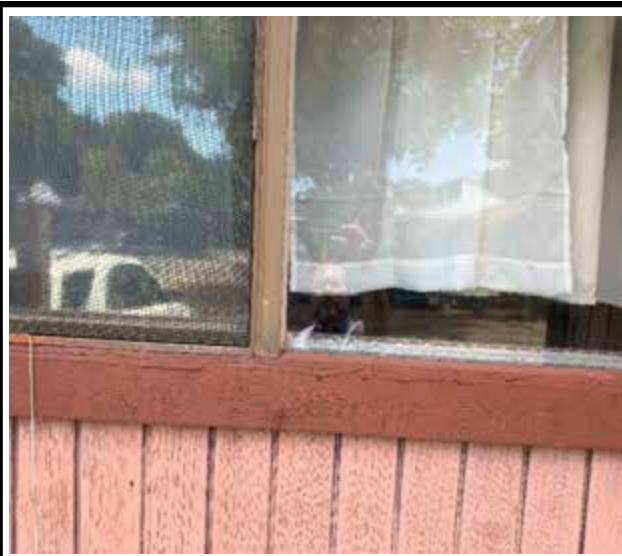
Photo 3 : Existing non-impact-rated window frame
