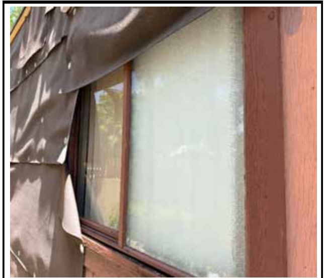
Photo 4 : Existing non-impact-rated window frame
