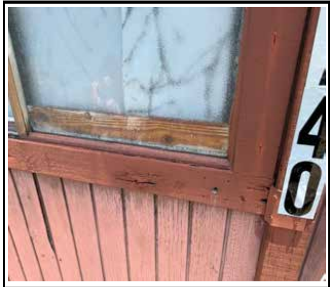
Photo 2 : Existing non-impact-rated window frame
