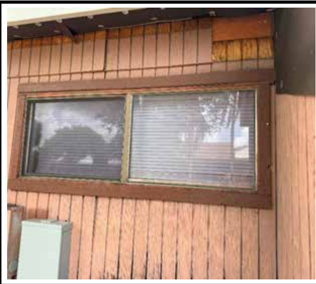
Photo 1 : Existing non-impact-rated window frame
