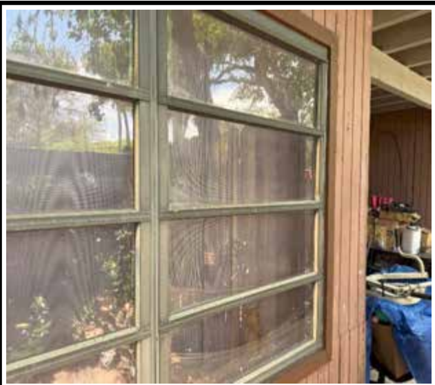
Photo 3 : Existing non-impact-rated window frame
