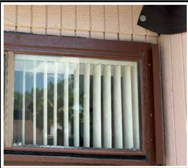
Photo 3 : Existing non-impact-rated window frame
