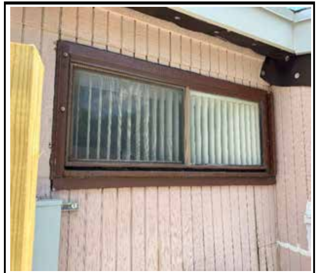
Photo 4 : Existing non-impact-rated window frame
