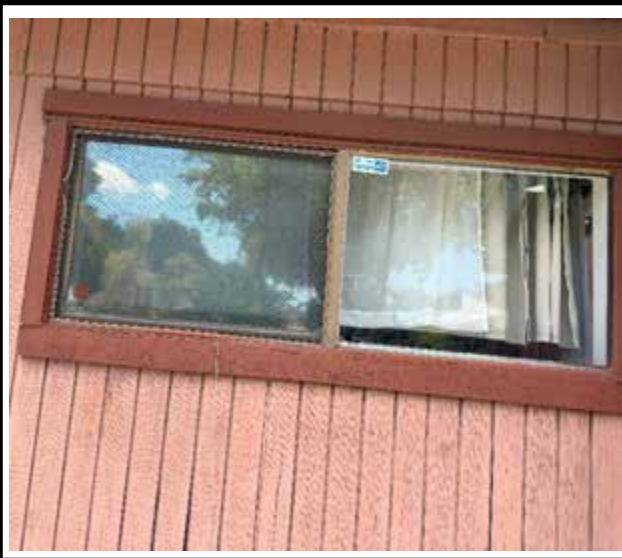
Photo 1 : Existing non-impact-rated window frame
