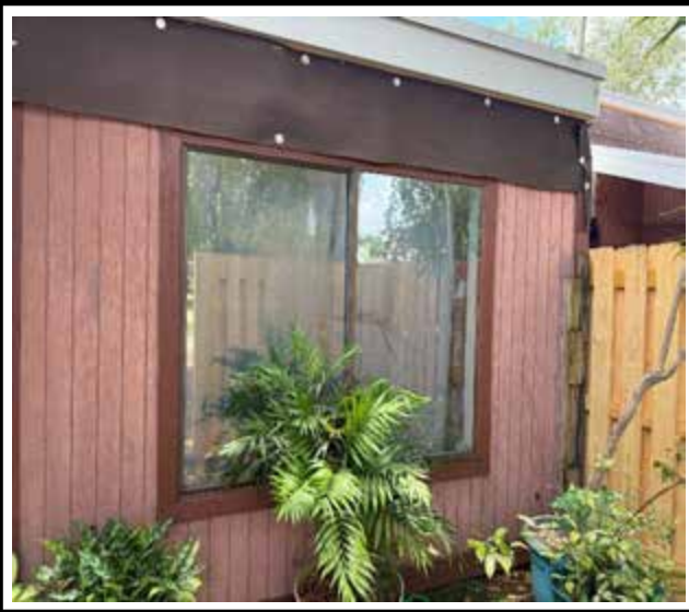
Photo 1 : Existing non-impact-rated window frame
