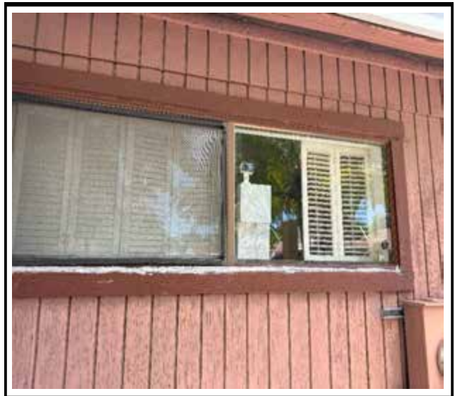
Photo 2 : Existing non-impact-rated window frame
