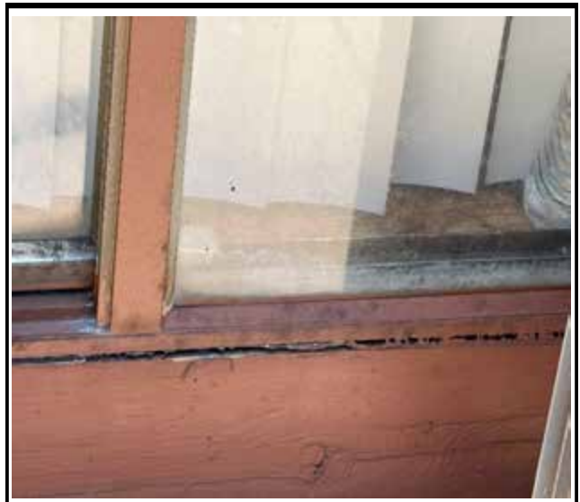
Photo 4 : Existing non-impact-rated window frame
