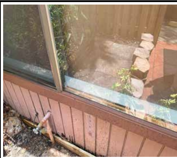
Photo 3 : Existing non-impact-rated window frame
