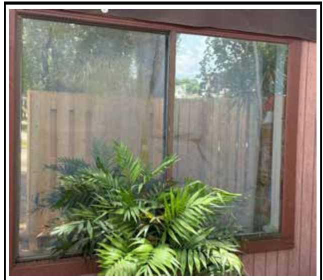
Photo 4 : Existing non-impact-rated window frame
