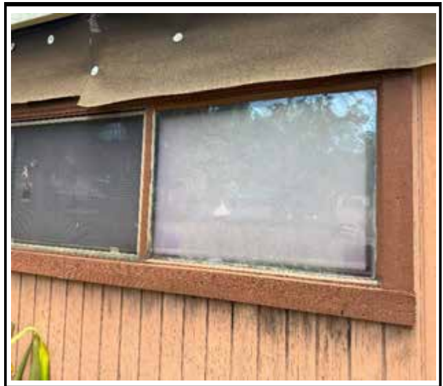
Photo 2 : Existing non-impact-rated window frame
