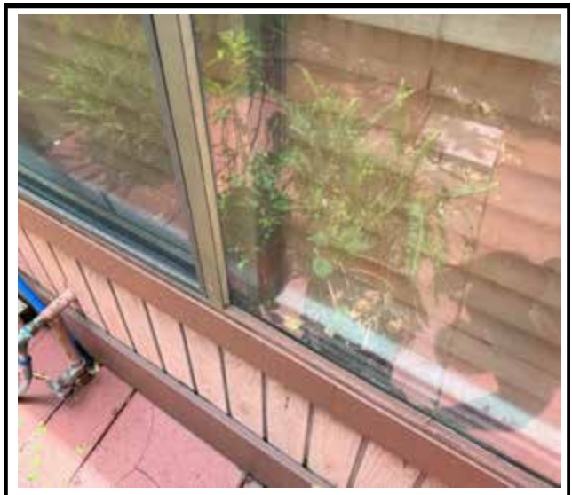
Photo 4 : Existing non-impact-rated window frame
