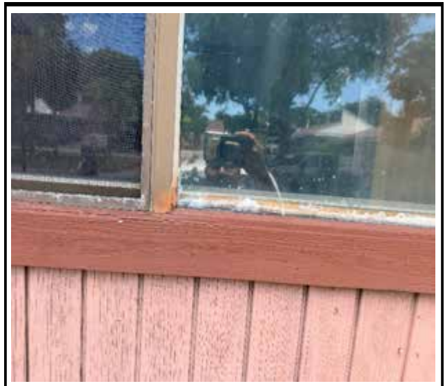
Photo 4 : Existing non-impact-rated window frame
