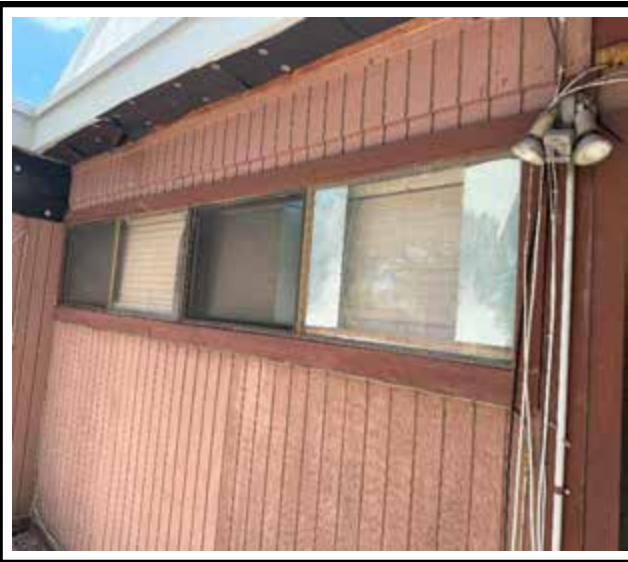
Photo 1 : Existing non-impact-rated window frame
