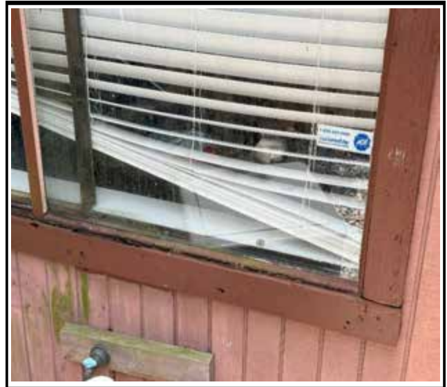
Photo 2 : Existing non-impact-rated window frame
