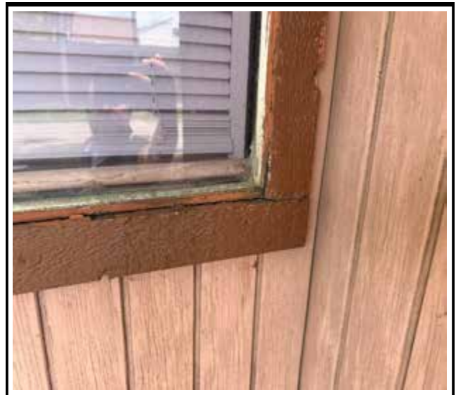
Photo 2 : Existing non-impact-rated window frame
