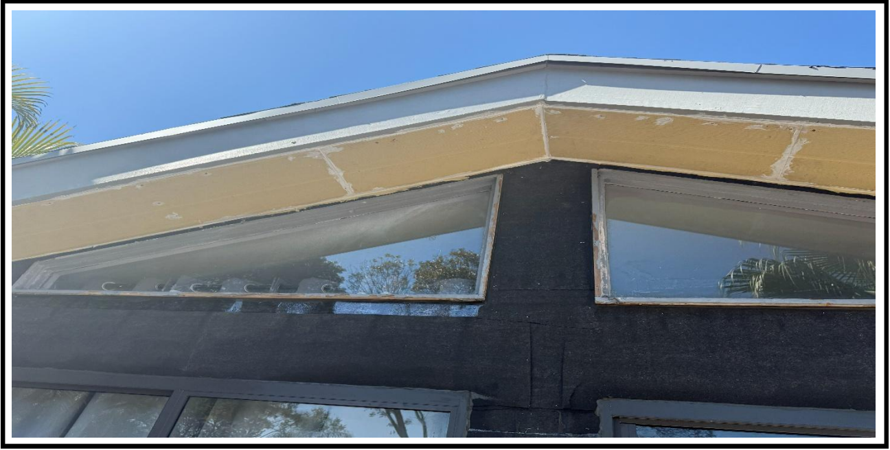
9 – Ongoing, Application of the Caulking at the Hardie board panels connections, BLDG 9.
