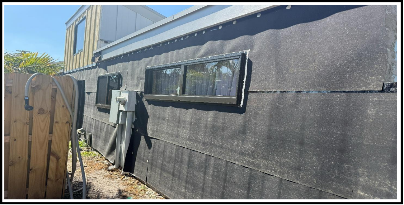
7 – Ongoing, Removal of the black paper vapor barrier over the Plywood at the exterior walls, BLDG 9.
