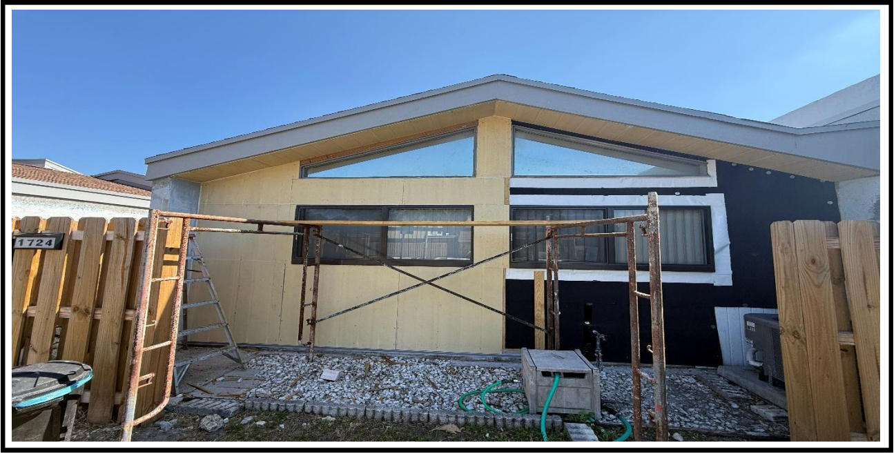
3 – Ongoing, Installation of the Hardie Board panels at the exterior walls, BLDG 11
