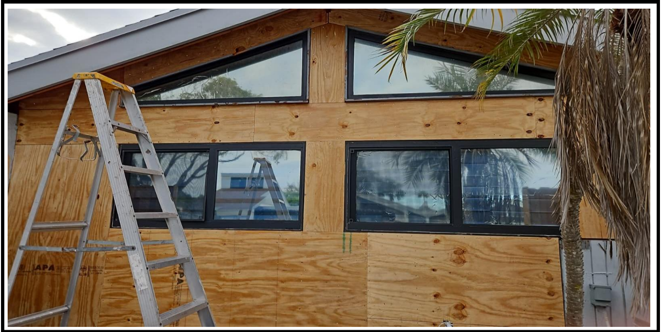
8 – Ongoing, Install of the plywood on exterior walls, BLDG 9.
