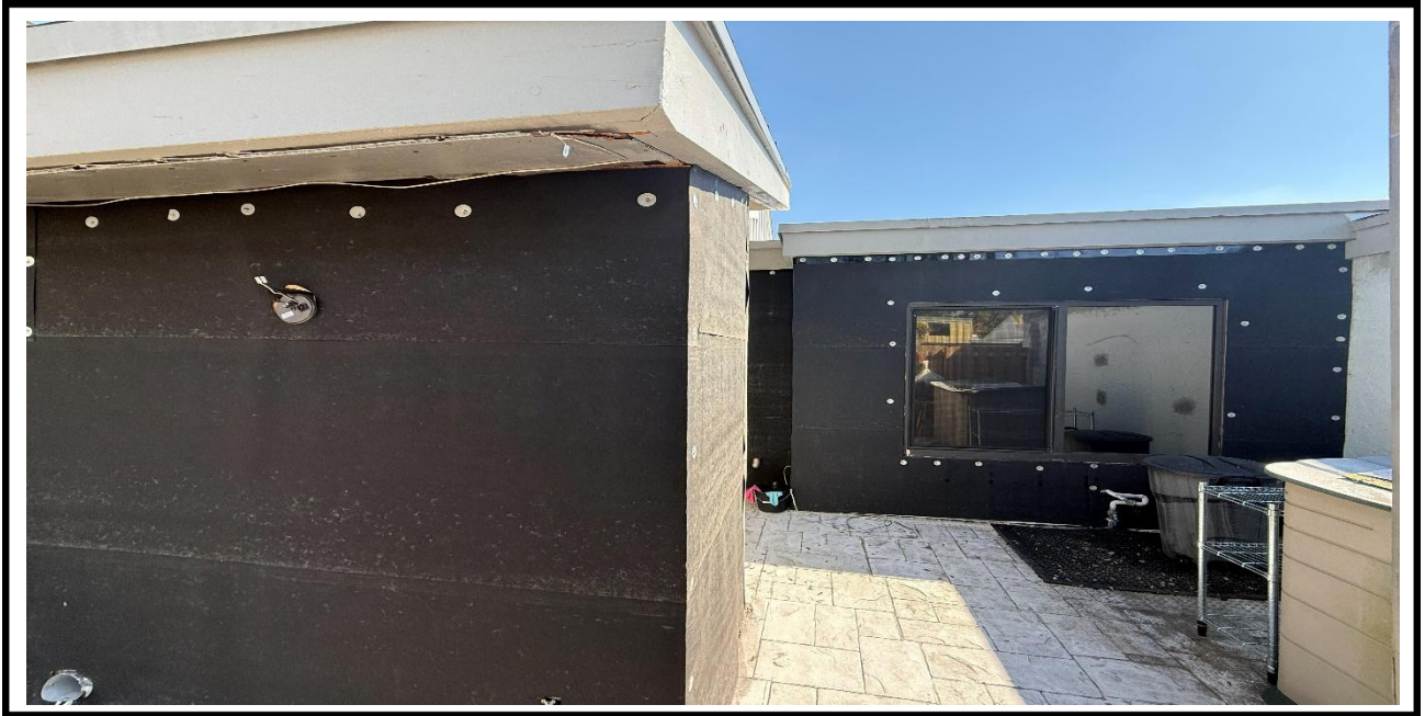
6 – Ongoing, Installation of the black paper vapor barrier over the Plywood at the exterior walls, BLDG 11.
