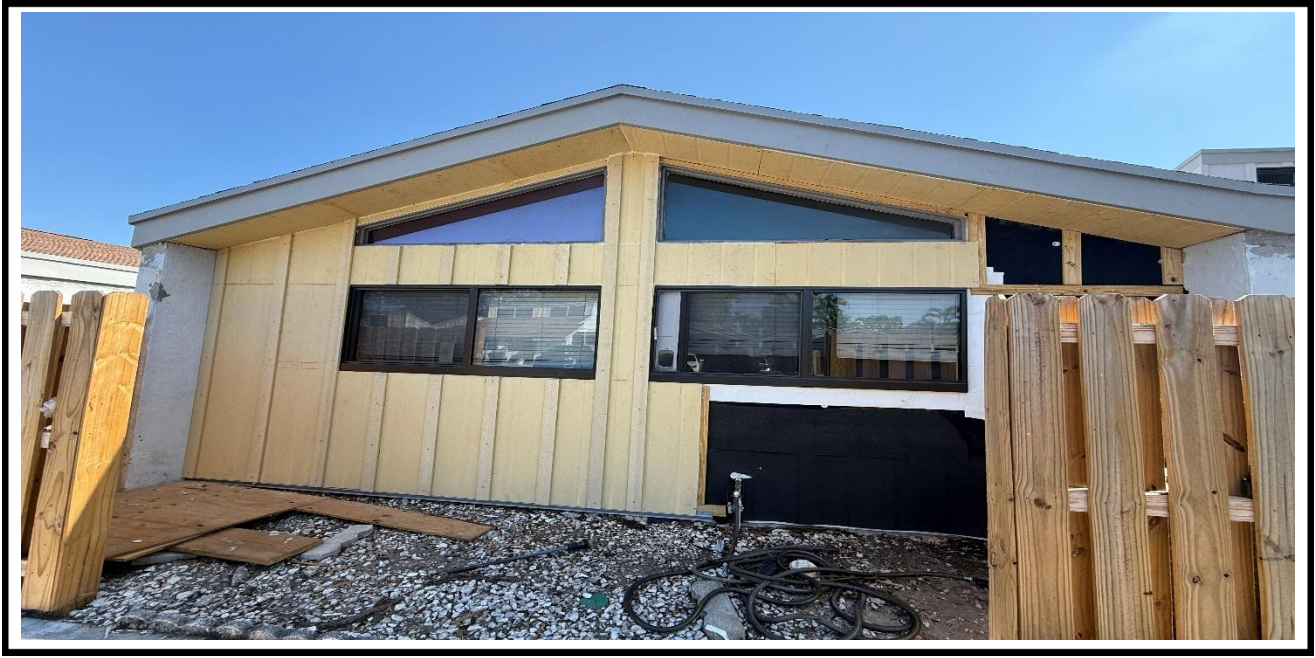
1 – Ongoing, Installation of the Hardie Board panels at the exterior walls, BLDG 11
