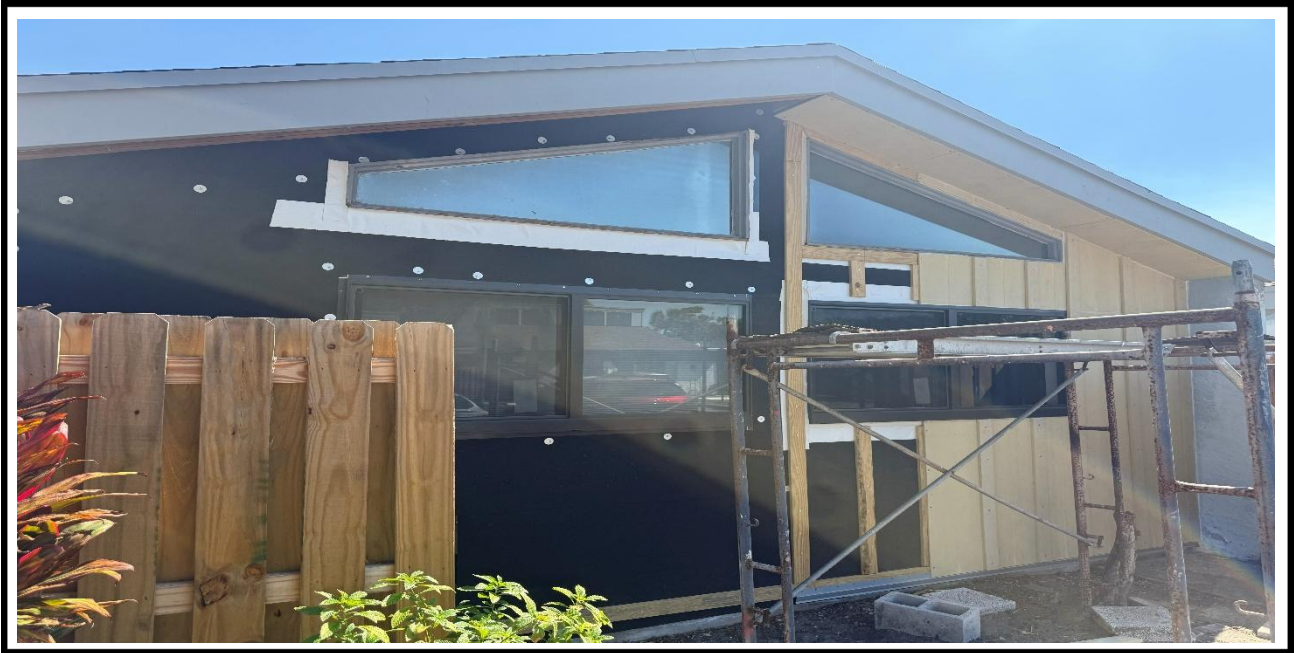
4 – Ongoing, Installation of the Hardie Board panels at the exterior walls, BLDG 11
