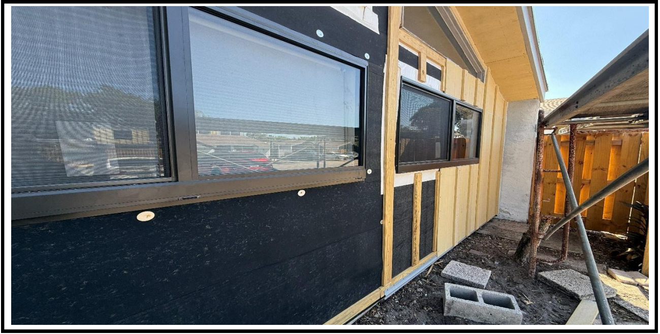
5 – Ongoing, Installation of the black paper vapor barrier over the Plywood at the exterior walls, BLDG 11.
