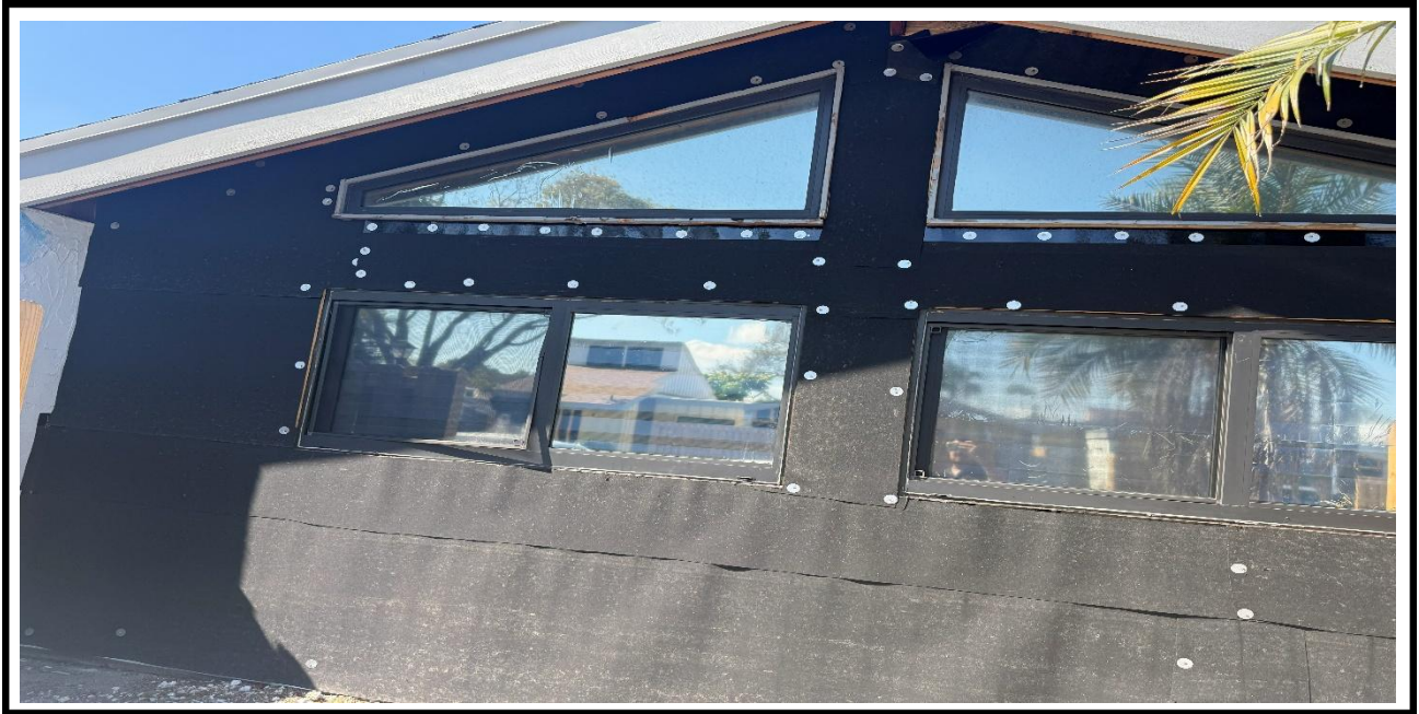
10 – Ongoing, Installation of the vapor barrier on top of Plywood at the exterior walls, BLDDG 9.
