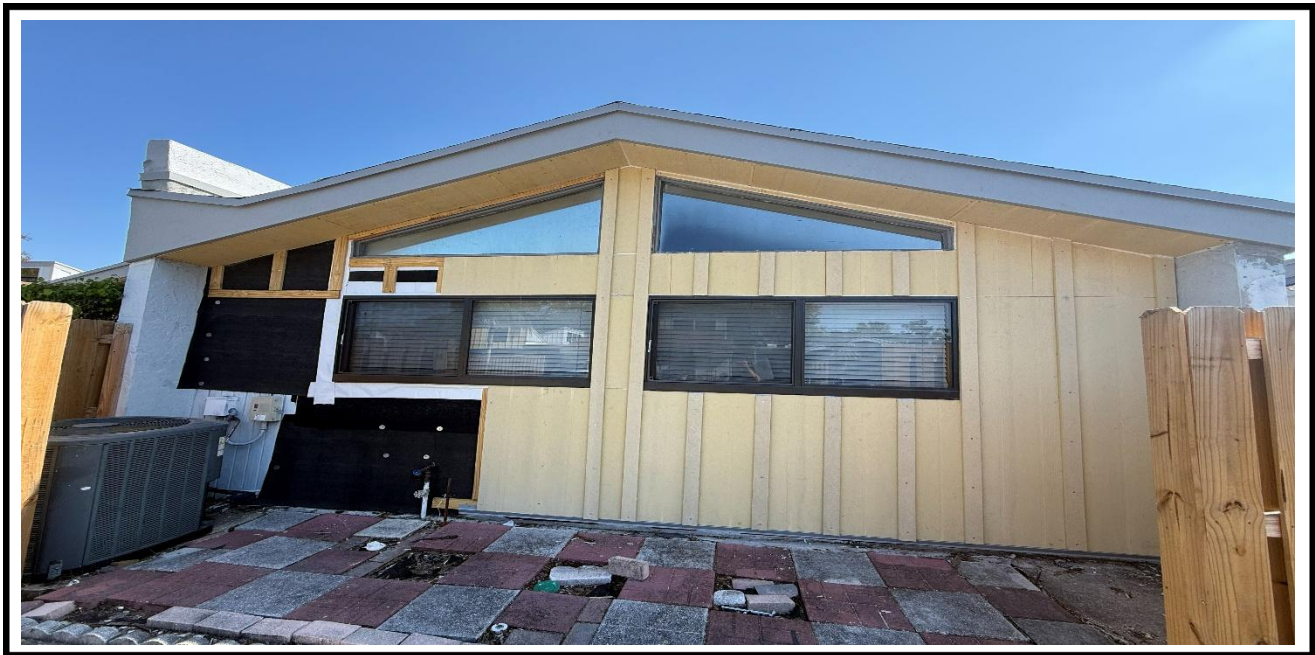
2 – Ongoing, Installation of the Hardie Board panels at the exterior walls, BLDG 11
