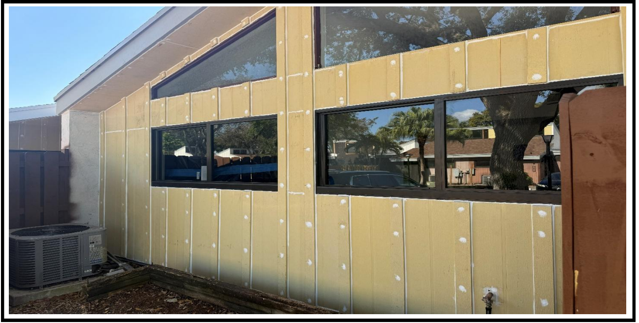
3 – Ongoing, Installation of the Hardie Board panels at the exterior walls, BLDG 2
