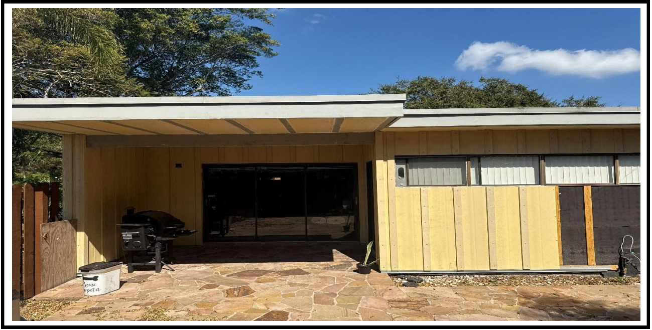
5 – Ongoing, Installation of the Hardie Board Panels, BLDG 2.
