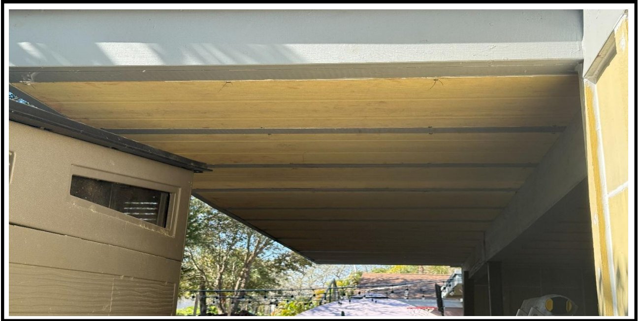
4 – Ongoing, Installation of the Hardie Board panels at the exterior walls, BLDG 02
