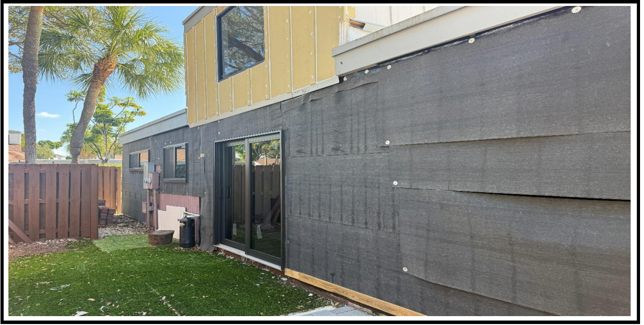
9 – Ongoing, Installation of the Vapor Barriers at the exterior walls, BLDG 9.
