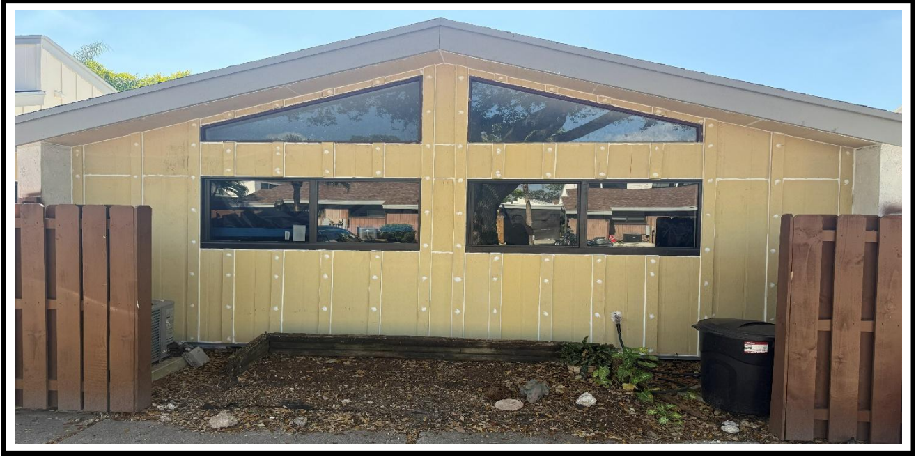
1 – Ongoing, Installation of the Hardie Board panels at the exterior walls, BLDG 2.
