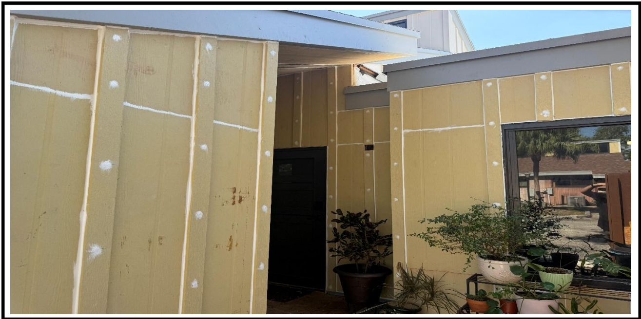
2 – Ongoing, Installation of the Hardie Board panels at the exterior walls, BLDG 06
