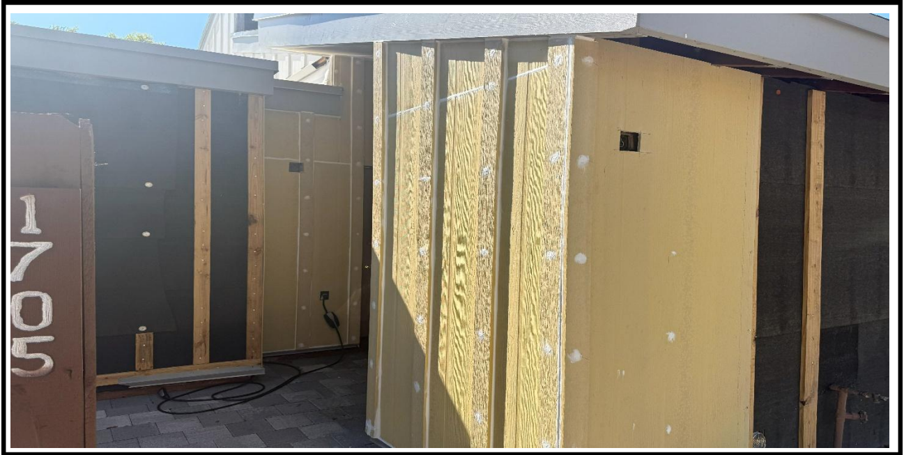
8 – Ongoing, Application of Caulking and Install of the Hardie Board on exterior walls, BLDG 2.
