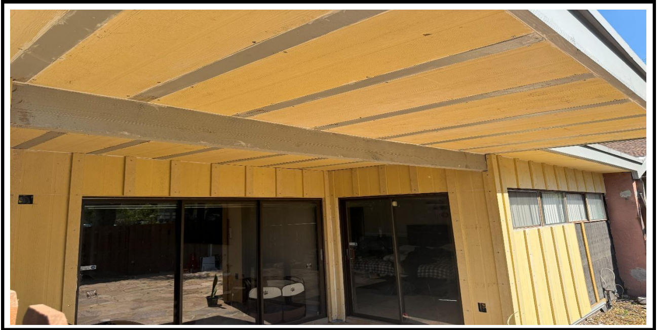
6 – Ongoing, Installation of the Hardie Board Panels, BLDG 2.
