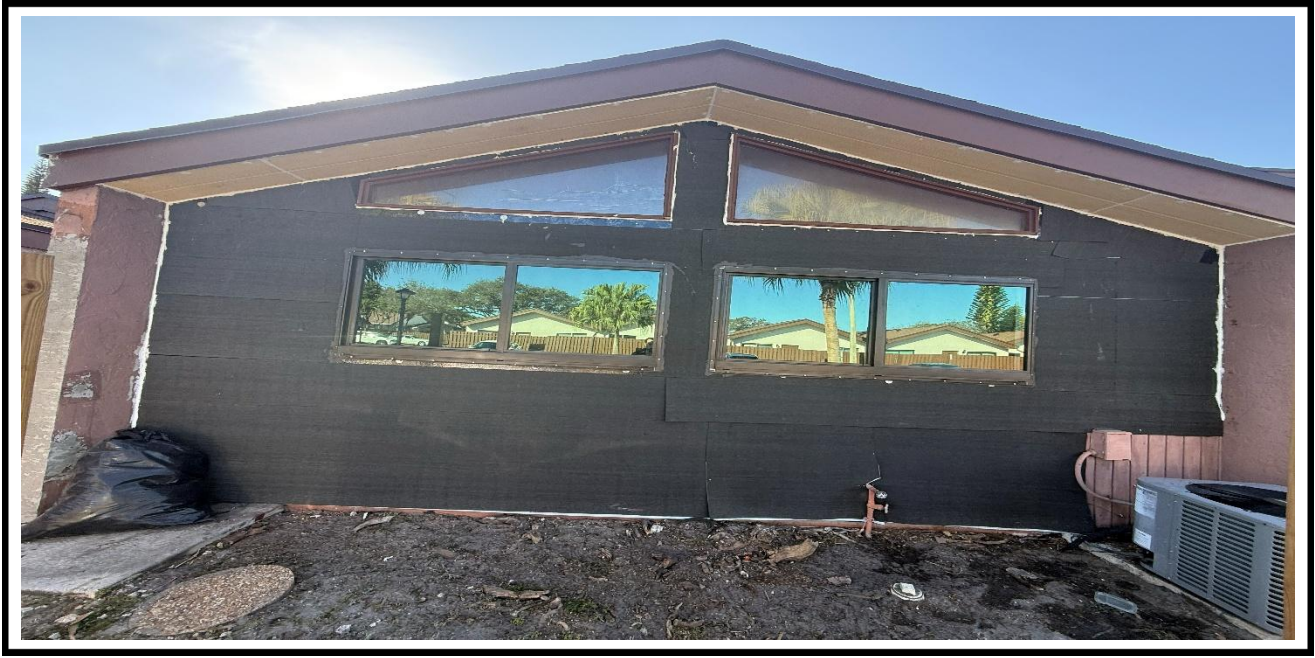
1 – Ongoing, Installation of the Vapor Barrier at the exterior walls, BLDG 14
