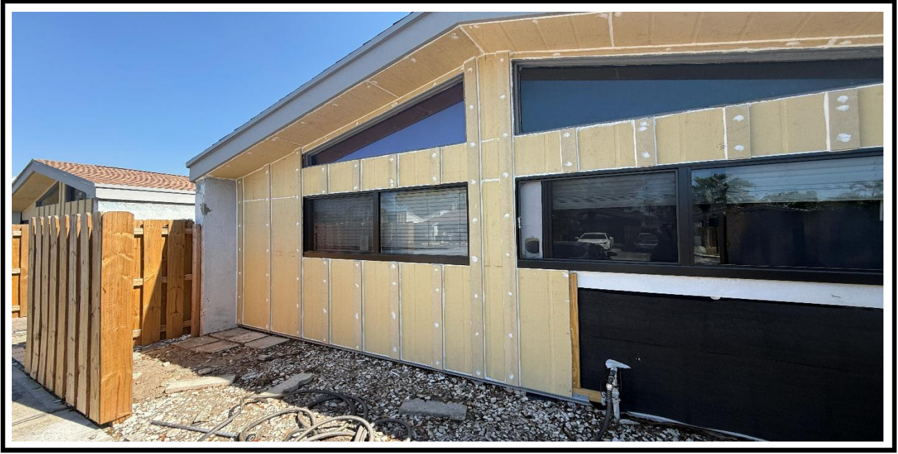
9 – Ongoing, Application of Caulking and Install of the Hardie Board on exterior walls, BLDG 9.
