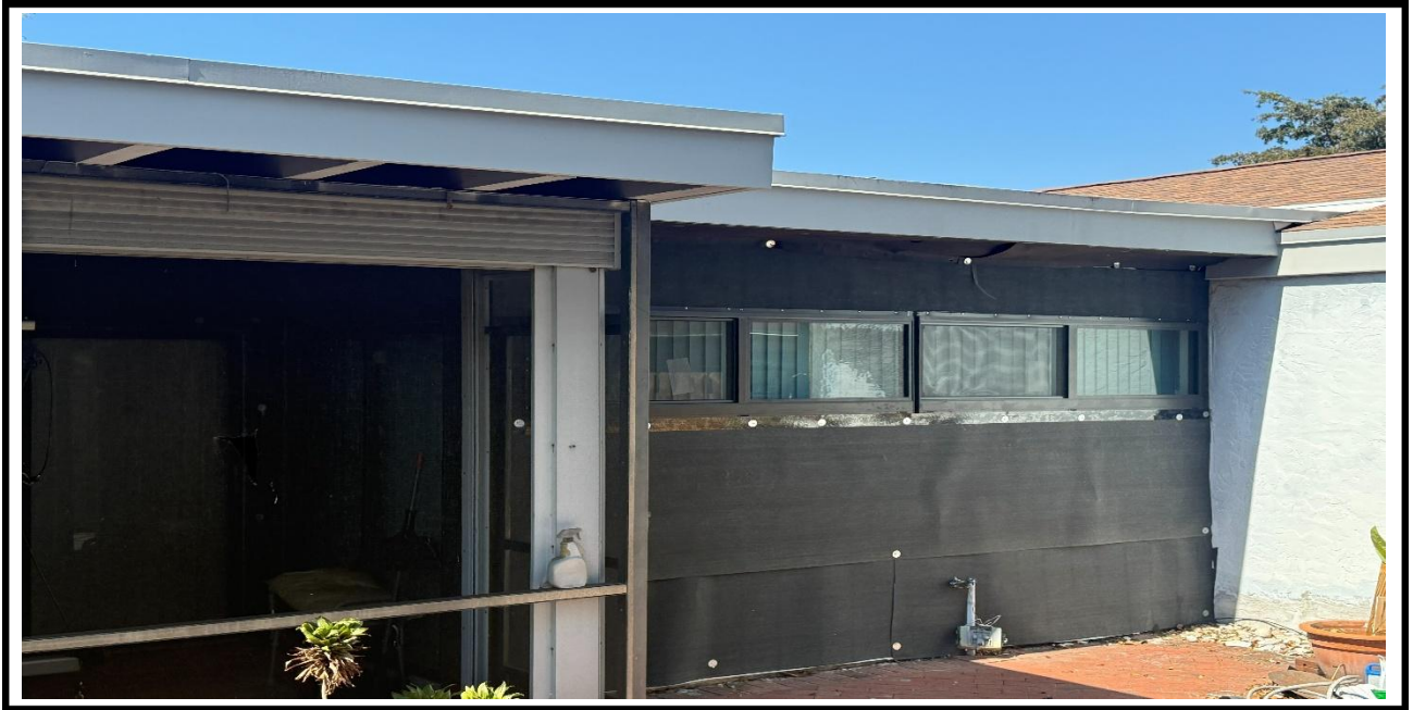
4 – Ongoing, Installation of the Vapor Barrier at the exterior walls, BLDG 11
