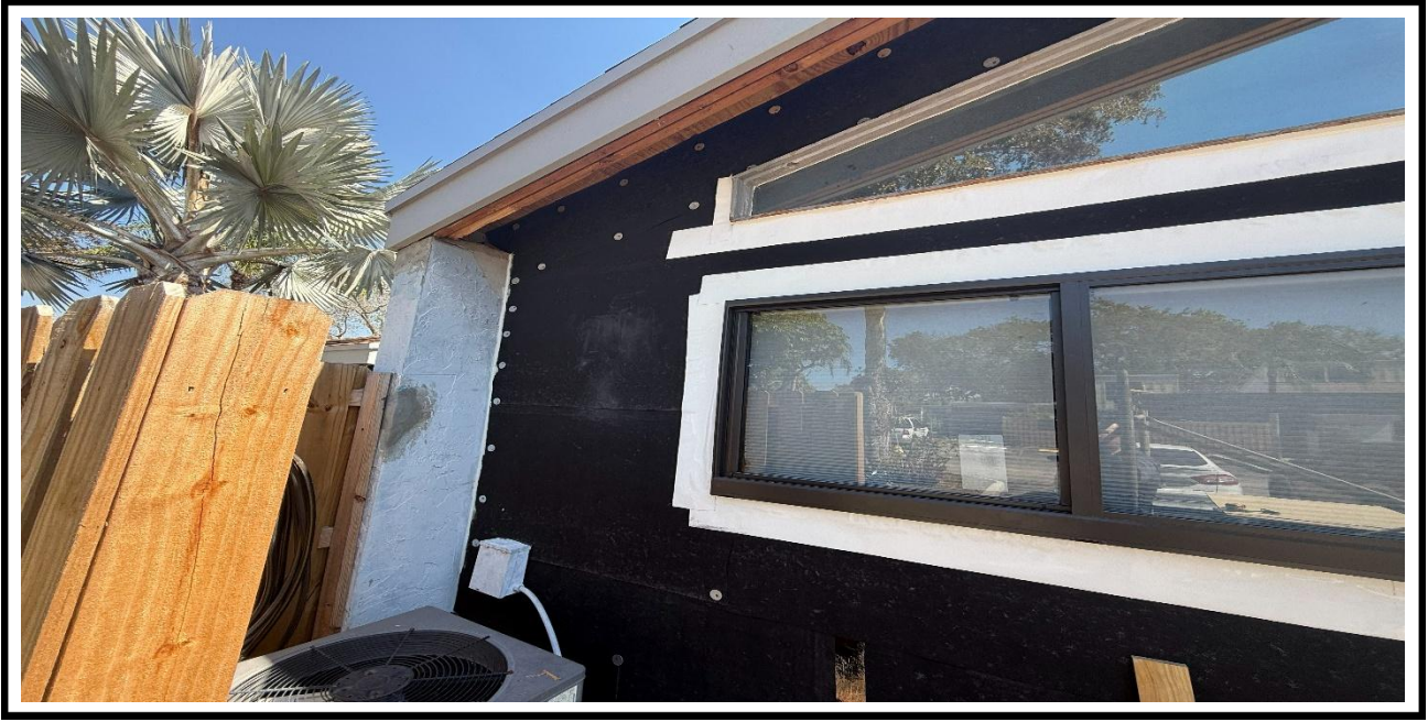
7 – Ongoing, Installation of the Vapor Barrier at the exterior walls , BLDG 2.
