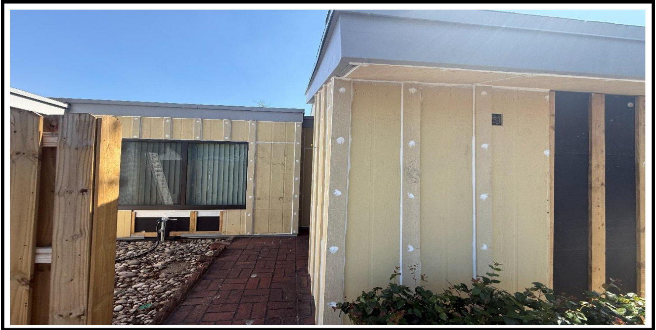
8 – Ongoing, Application of Caulking and Install of the Hardie Board on exterior walls, BLDG 11.
