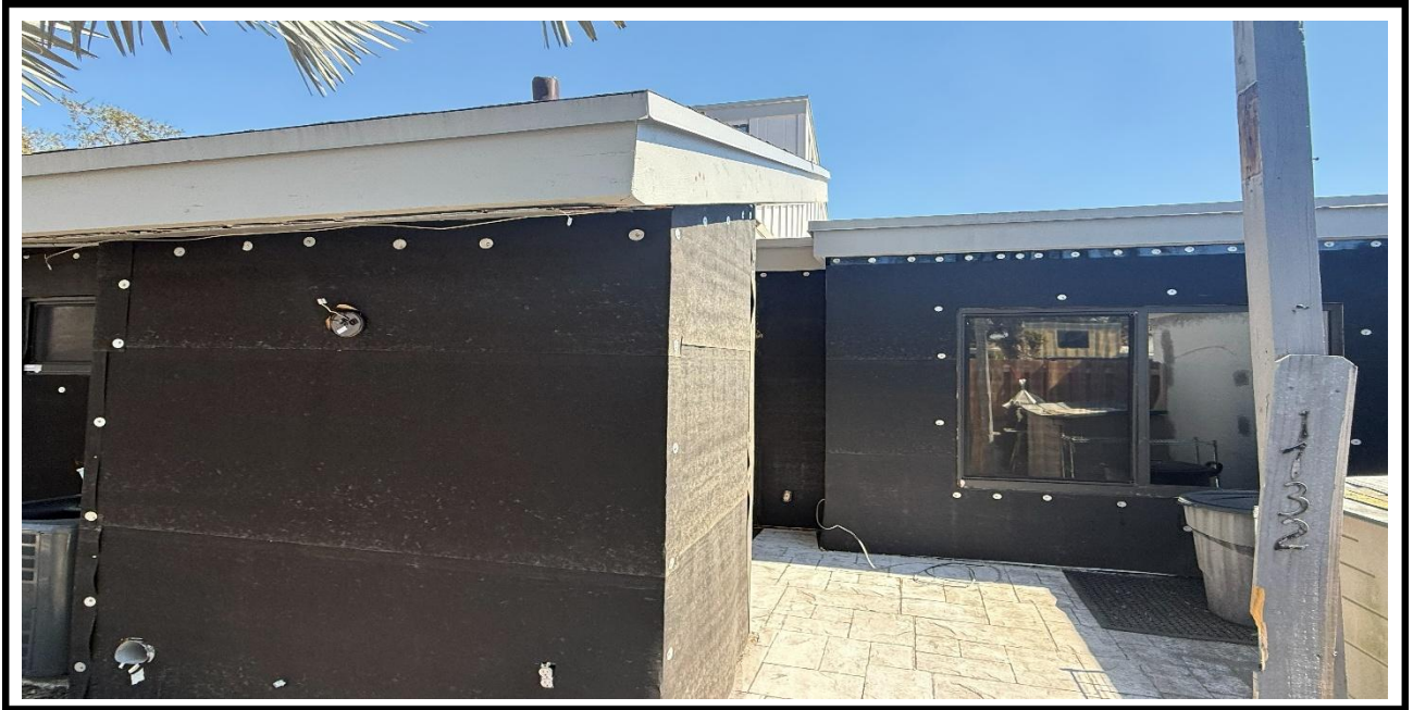
6 – Ongoing, Installation of the Vapor Barrier at the exterior walls, BLDG 11.
