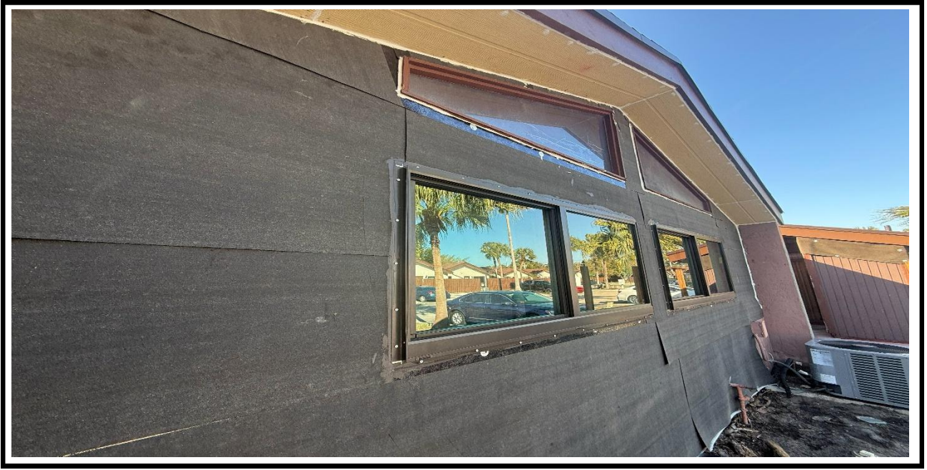
3 – Ongoing, Installation of the Hardie Board panels at the exterior walls, BLDG 14
