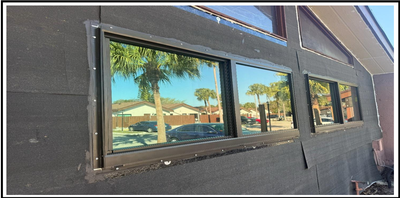
2 – Ongoing, Installation of the Vapor Barrier at the exterior walls, BLDG 14
