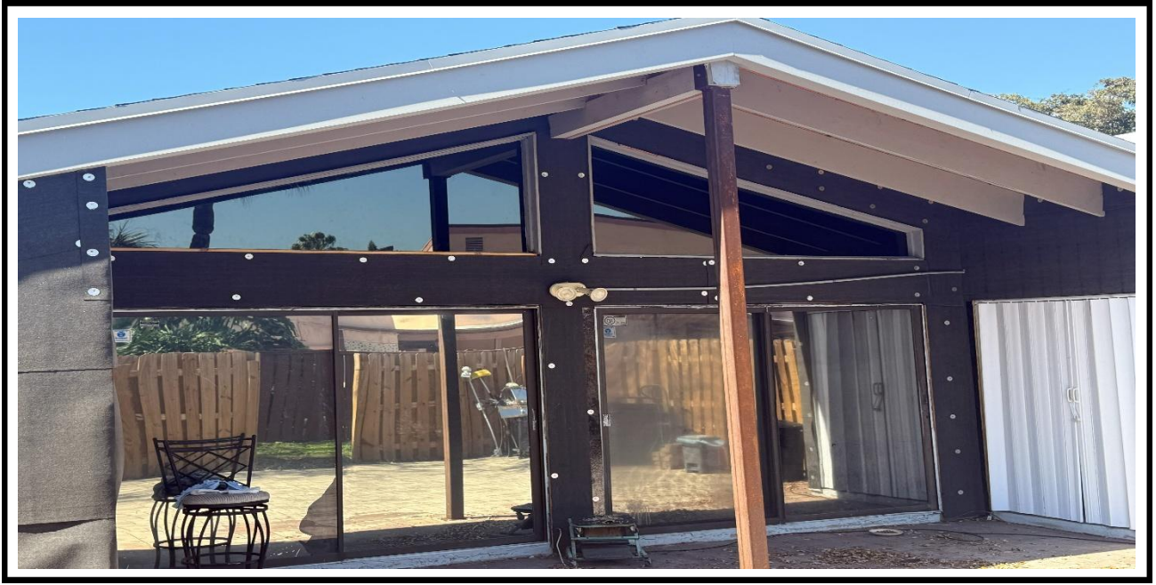
5 – Ongoing, Installation of the Hardie Board Panels, BLDG 11.
