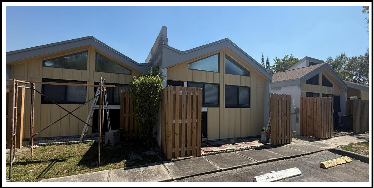
10 – Ongoing, Application of Caulking and Install of the Hardie Board on exterior walls, BLDG 11.
