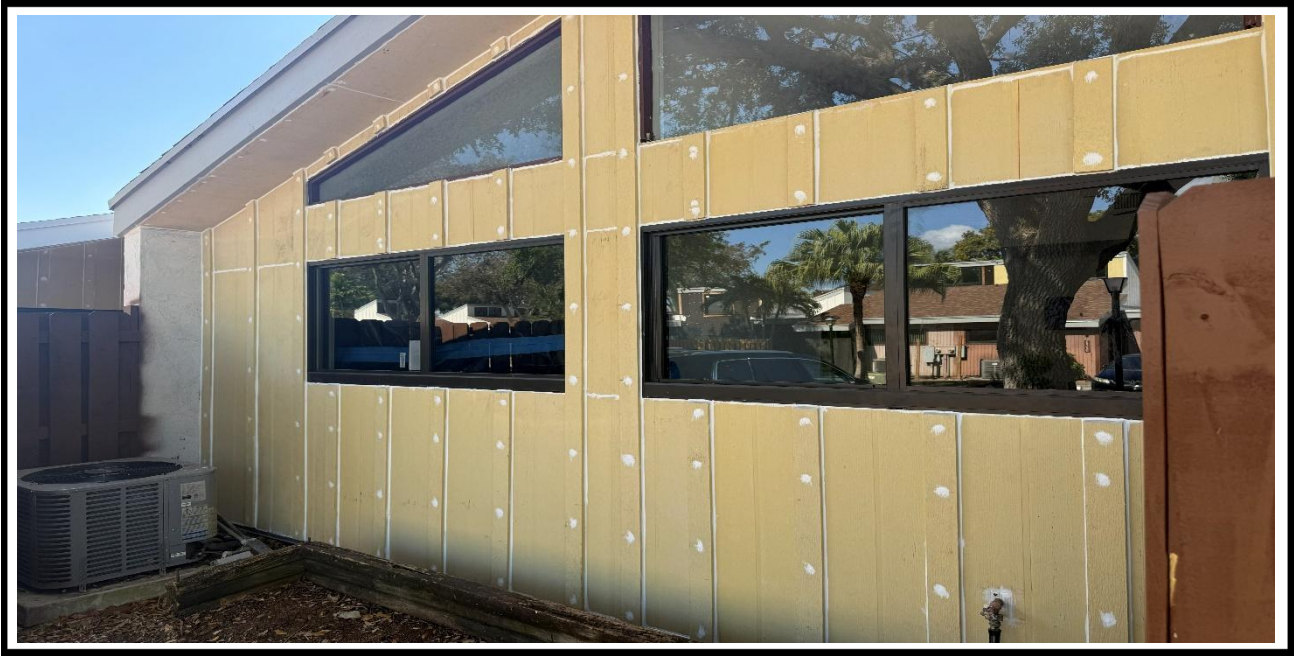
9 – Ongoing, Installation of the Hardie Board Panels at the exterior walls, BLDG 2.
