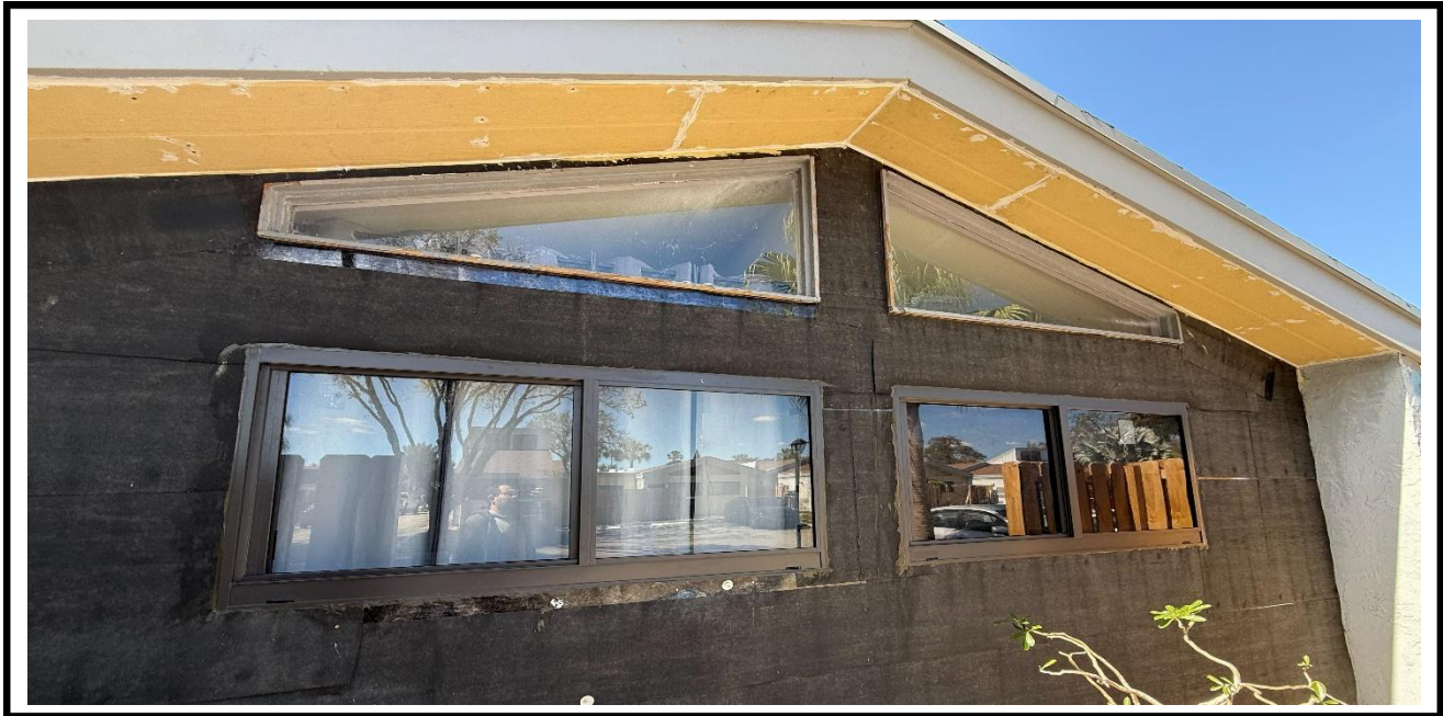
2 – Ongoing, Installation of the Vapor Barrier at the exterior walls, BLDG 08
