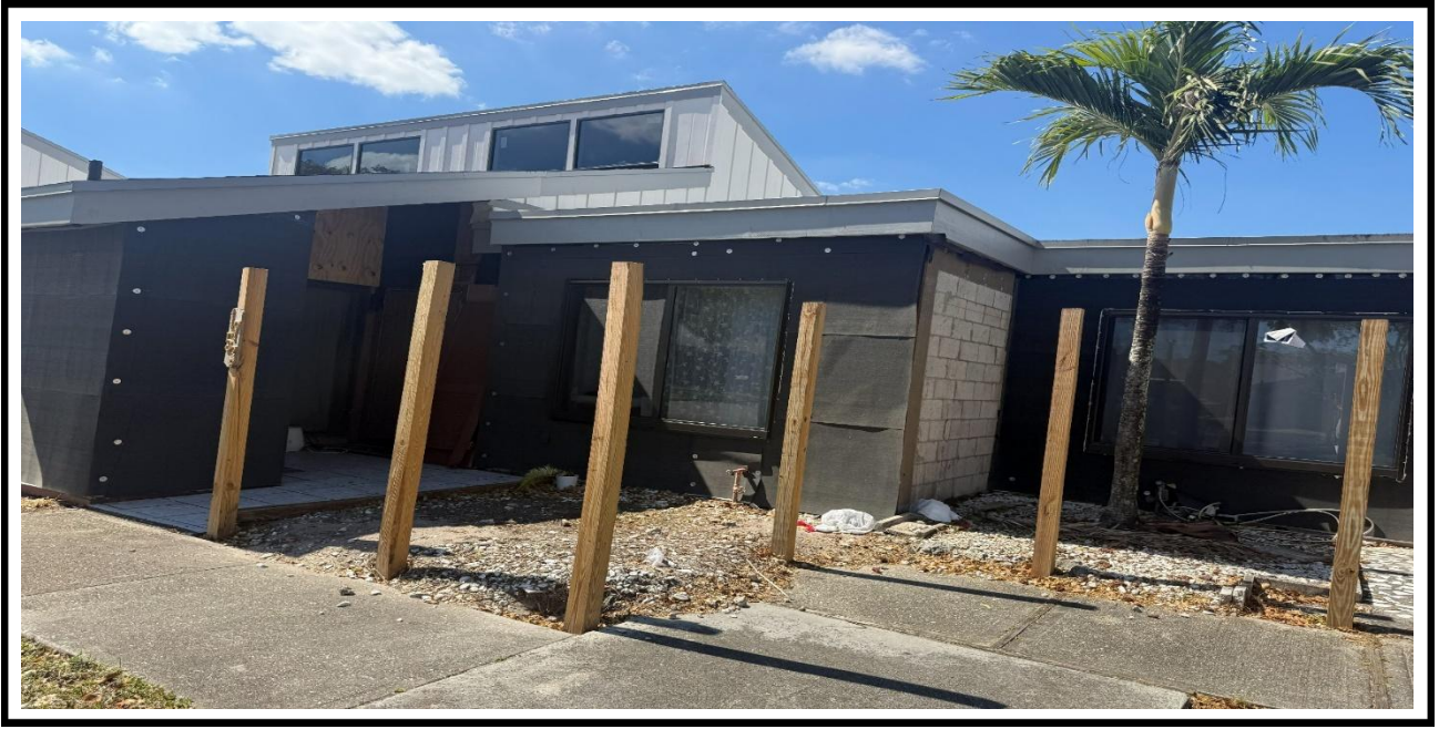
5 – Ongoing, Installation of Vapor Barrier at exterior wall , BLDG 2.
