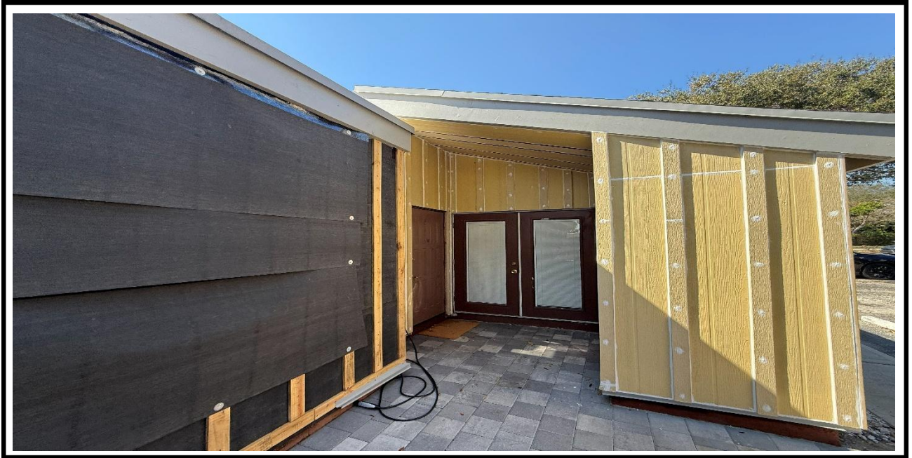
10 – Ongoing, Installation of the Hardie Board Panels at the exterior walls, BLDDG 2.
