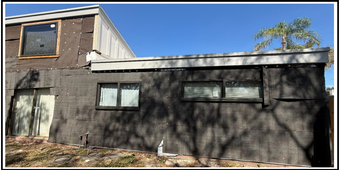
8 – Ongoing, Installation of the Vapor Barrier at the exterior walls, BLDG 2.
