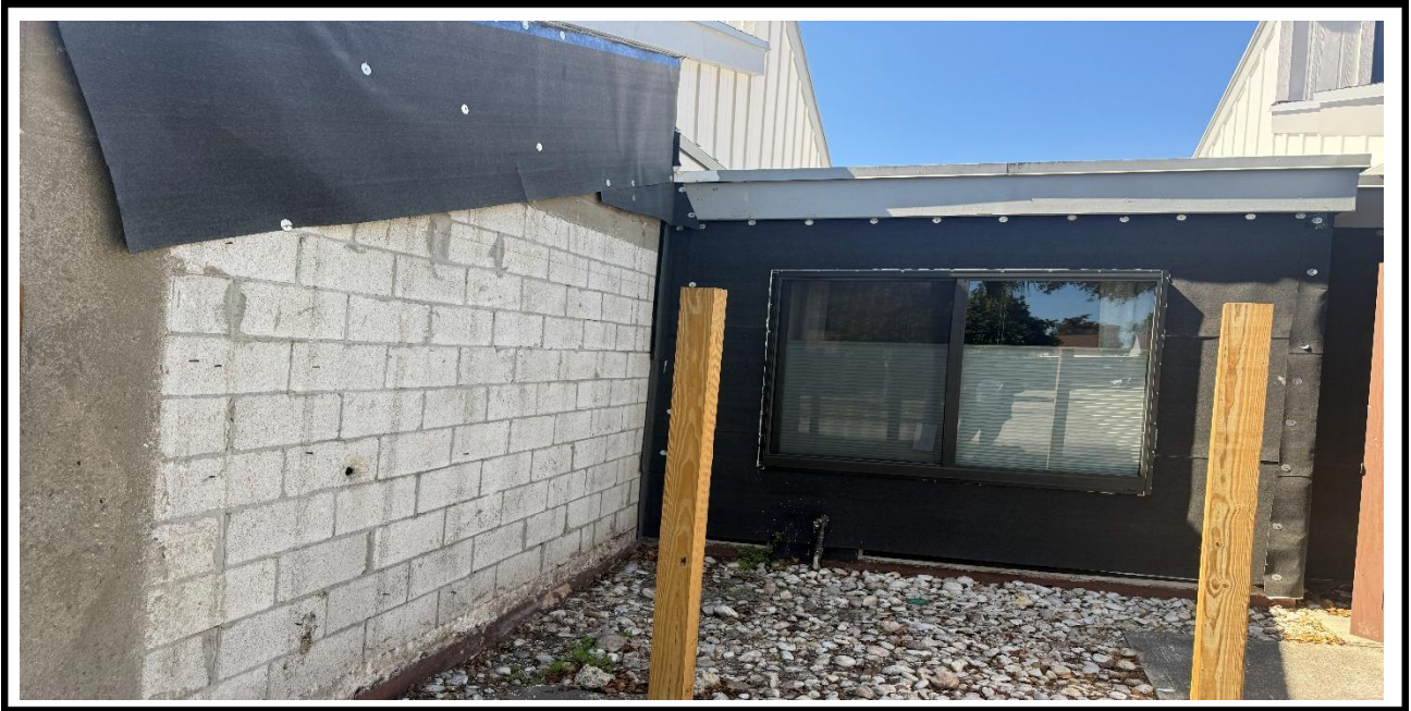
4 – Ongoing, Installation of the Vapor Barrier at the exterior walls, BLDG 03
