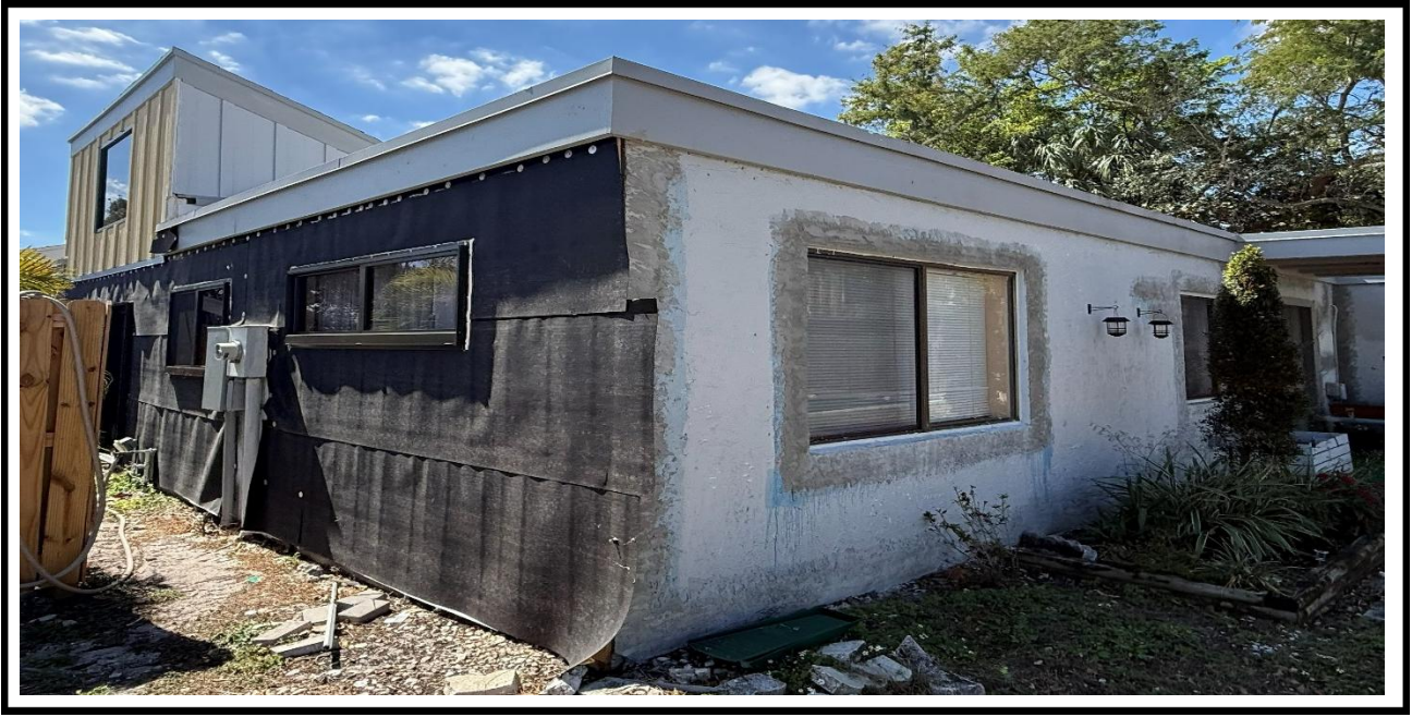
3 – Ongoing, Installation of the Vapor Barrier at the exterior walls, BLDG 08
