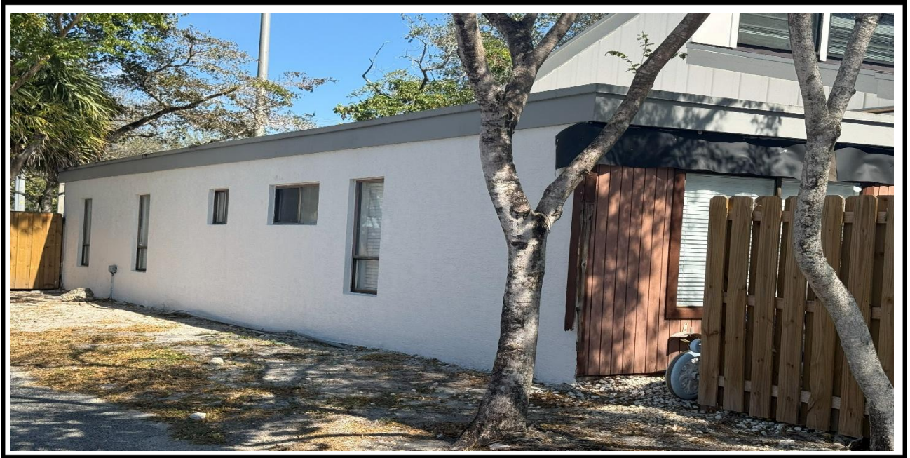
6 – Ongoing, Application of the stucco and paint at exterior wall, BLDG 4.
