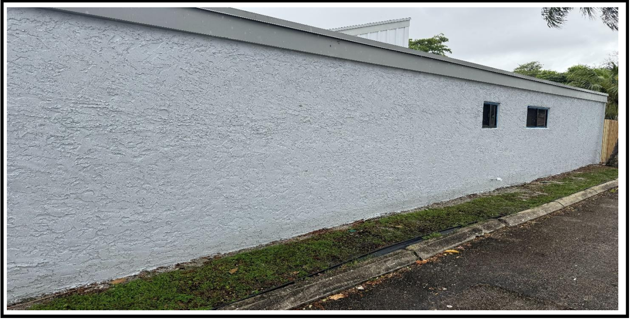
3 – Ongoing, Application of skim coat at the exterior walls, BLDG 08
