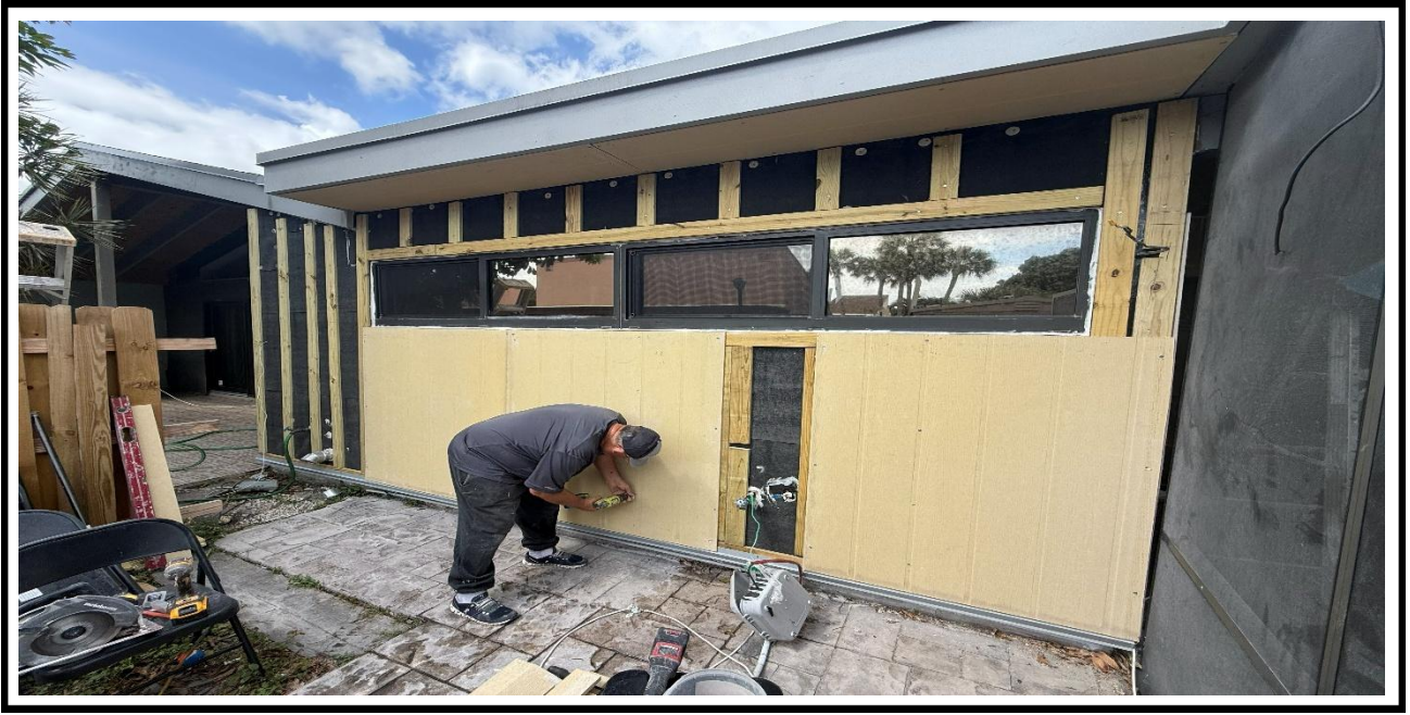
9 – Ongoing, Installation of the Hardie Board Panels at the exterior walls of the buildings.
