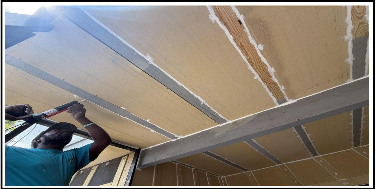
10 – Ongoing, Application of the caulking at the Hardie Panels at exterior walls of the buildings.
