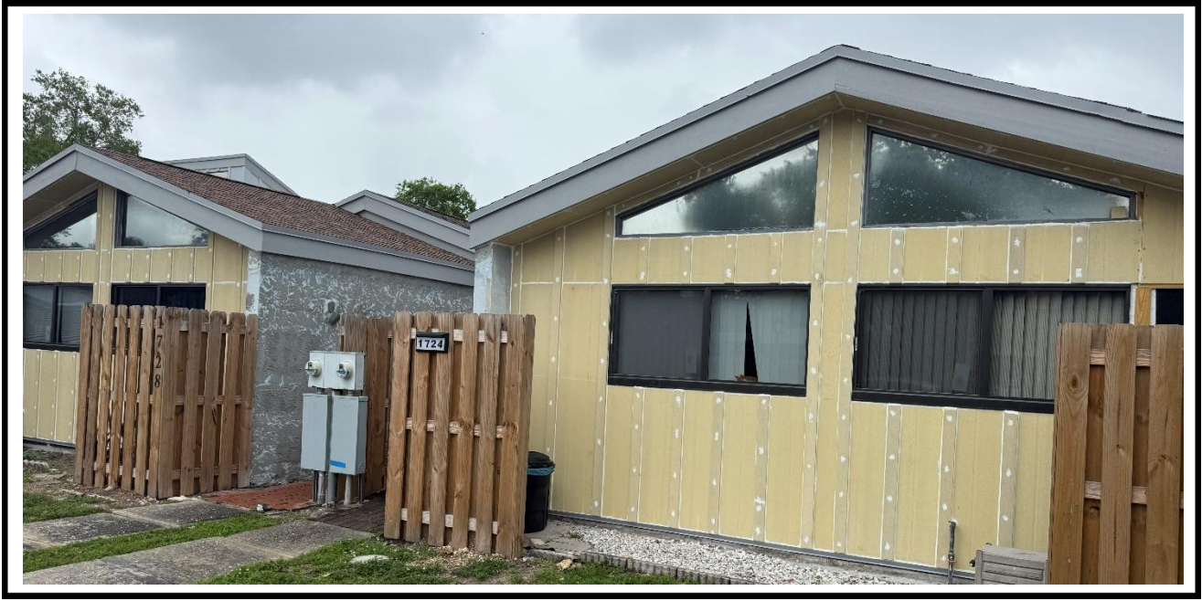
1 – Ongoing, Installation of the Hardie Panels at the exterior walls, BLDG 08
