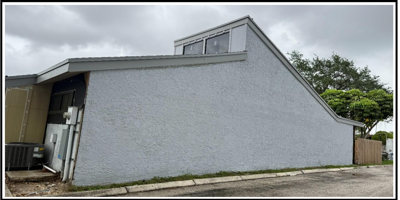
6 – Ongoing, Application of the stucco and paint at exterior wall, BLDG 11.
