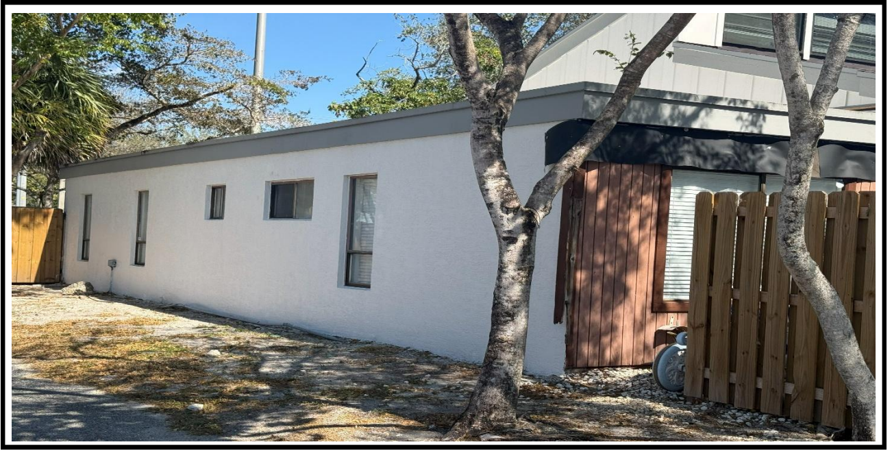
5 – Ongoing, Application of the stucco and paint at exterior wall, BLDG 4.
