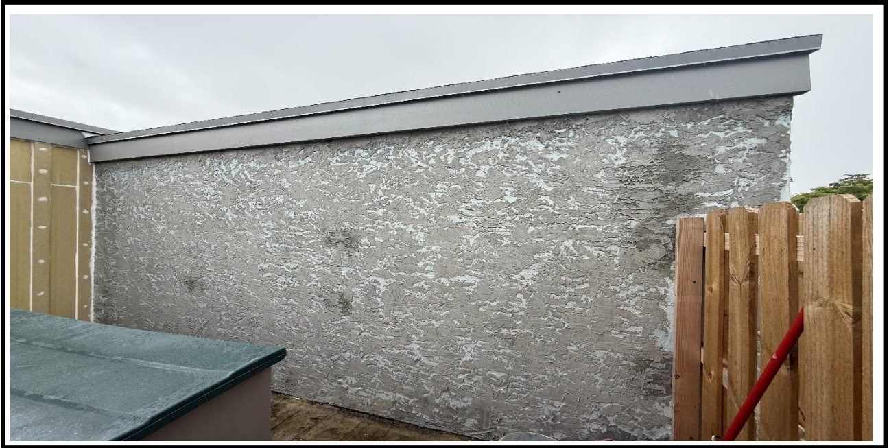
4 – Ongoing, Application of skim coat at the exterior walls, BLDG 03
