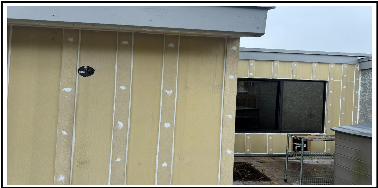
2 – Ongoing, Installation of the Hardie Panels at the exterior walls, BLDG 08
