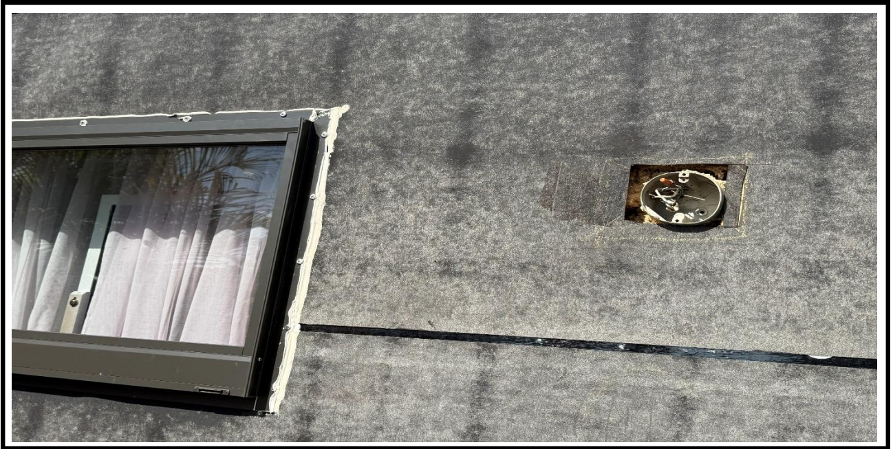
8 – Ongoing, Installation of the extension for outer fixtures at the exterior walls.
