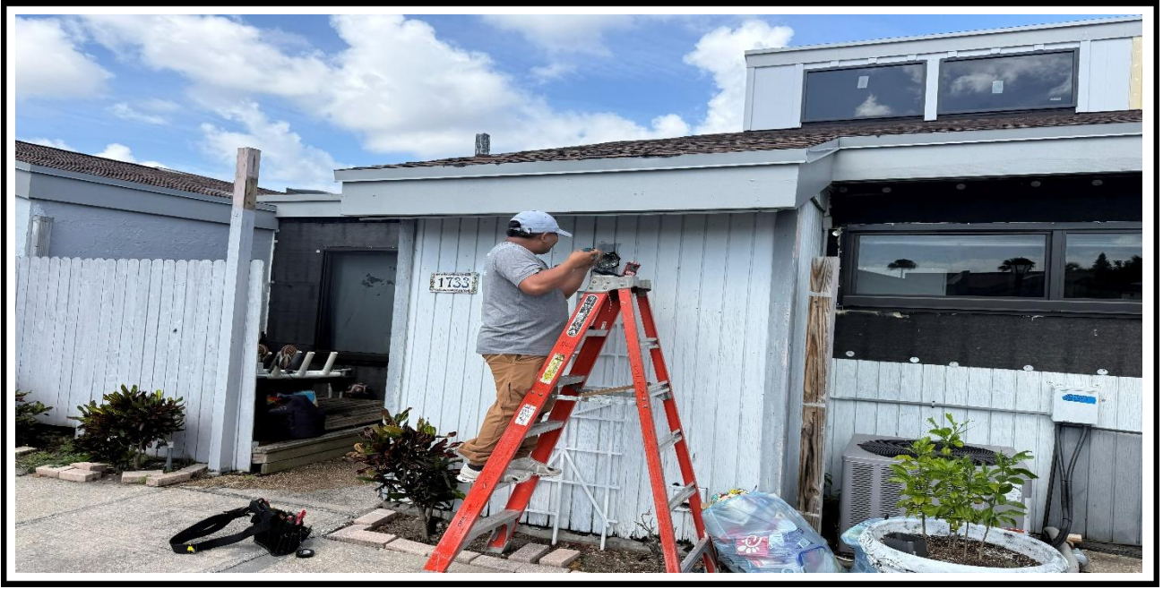
7 – Ongoing, Installation of the extension for outer fixtures at the exterior walls.
