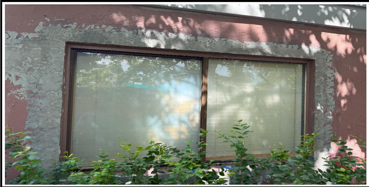
4 – Ongoing, Application of the new stucco at the exterior walls, BLDG 04 .
