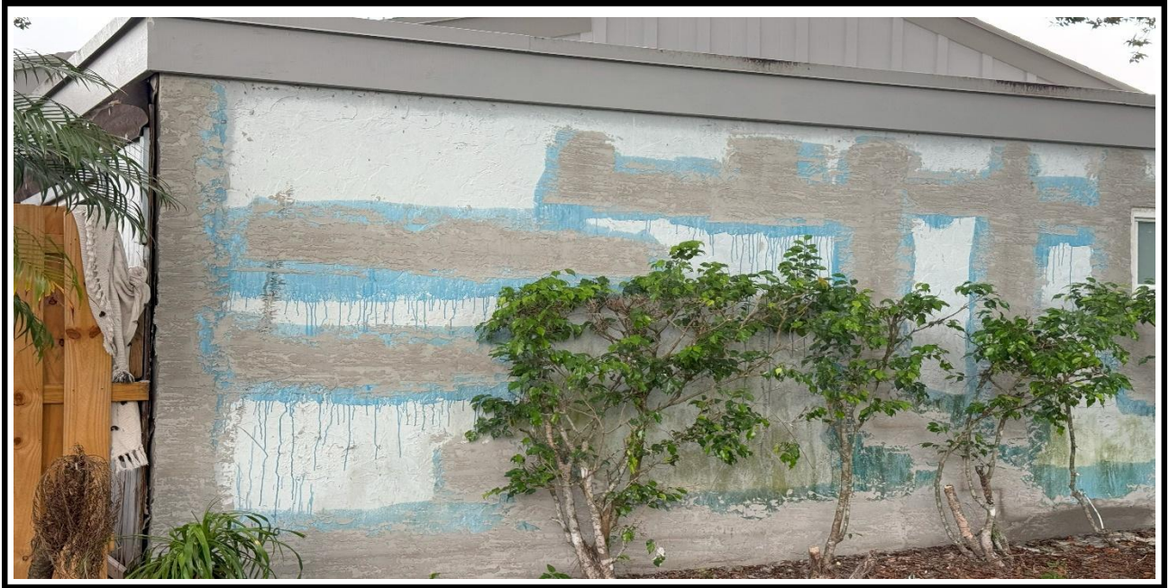
14 – Ongoing, Application of the new stucco at the exterior walls, BLDG 13 .
