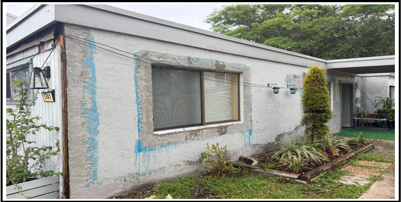
18 – Ongoing, Application of the new stucco at the exterior walls, BLDG 08 .
