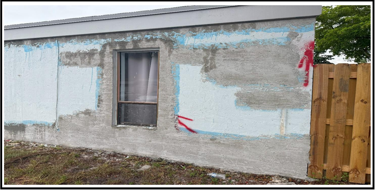
15 – Ongoing, Application of the new stucco at the exterior walls, BLDG 07 .
