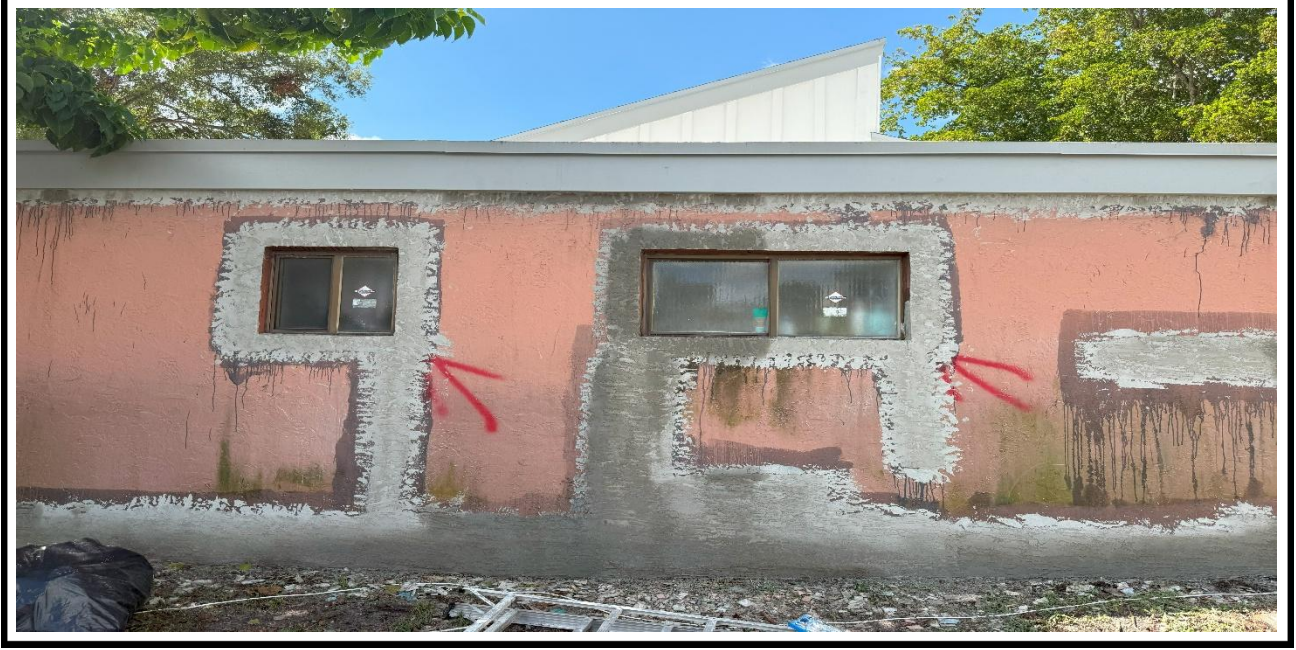
5 – Ongoing, Application of the new stucco at the exterior walls, BLDG 05 .
