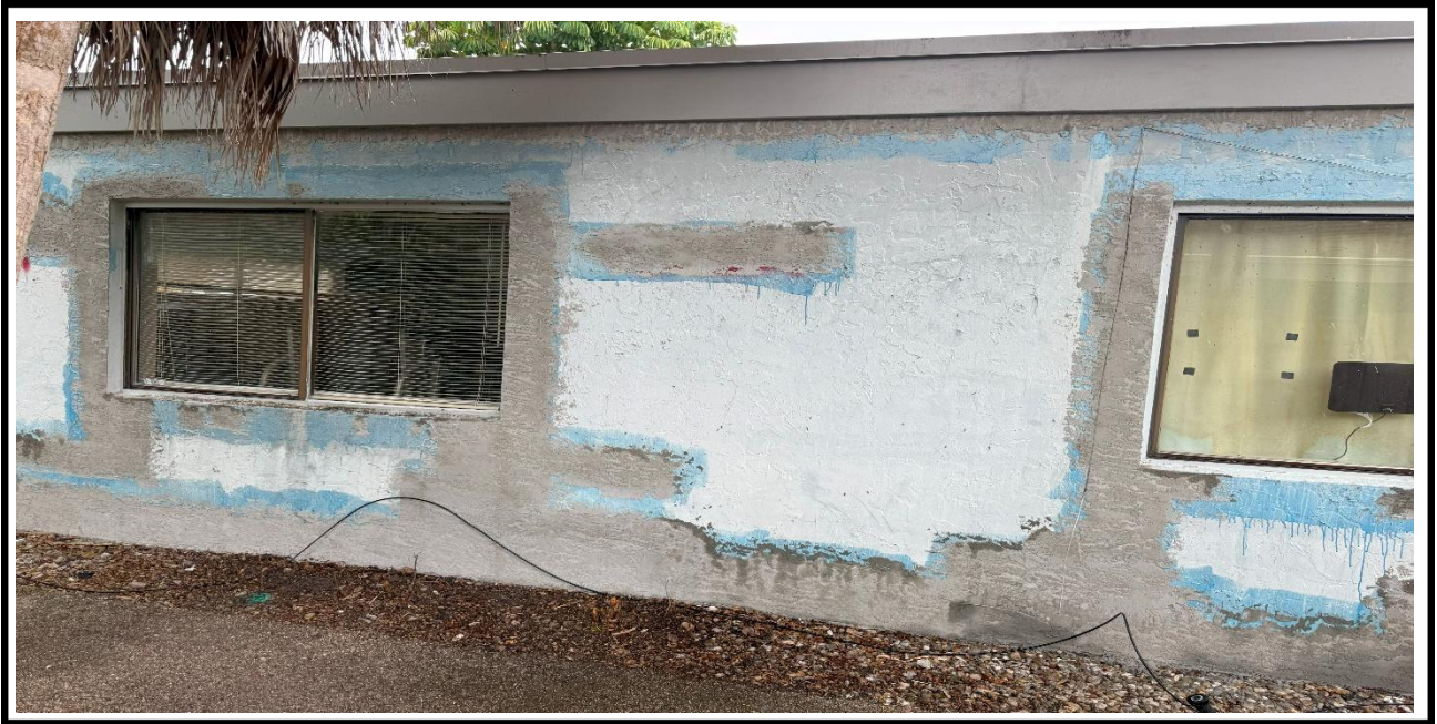
16 – Ongoing, Application of the new stucco at the exterior walls, BLDG 07 .
