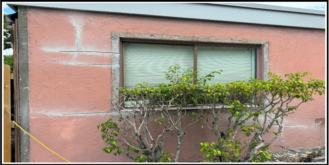
12 – Ongoing, Application of the new stucco at the exterior walls, BLDG 02 .
