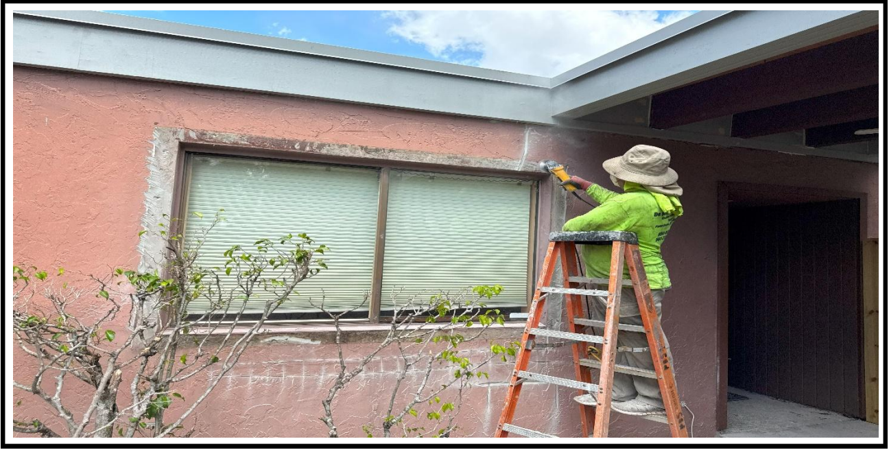
11 – Ongoing, Application of the new stucco at the exterior walls, BLDG 02 .
