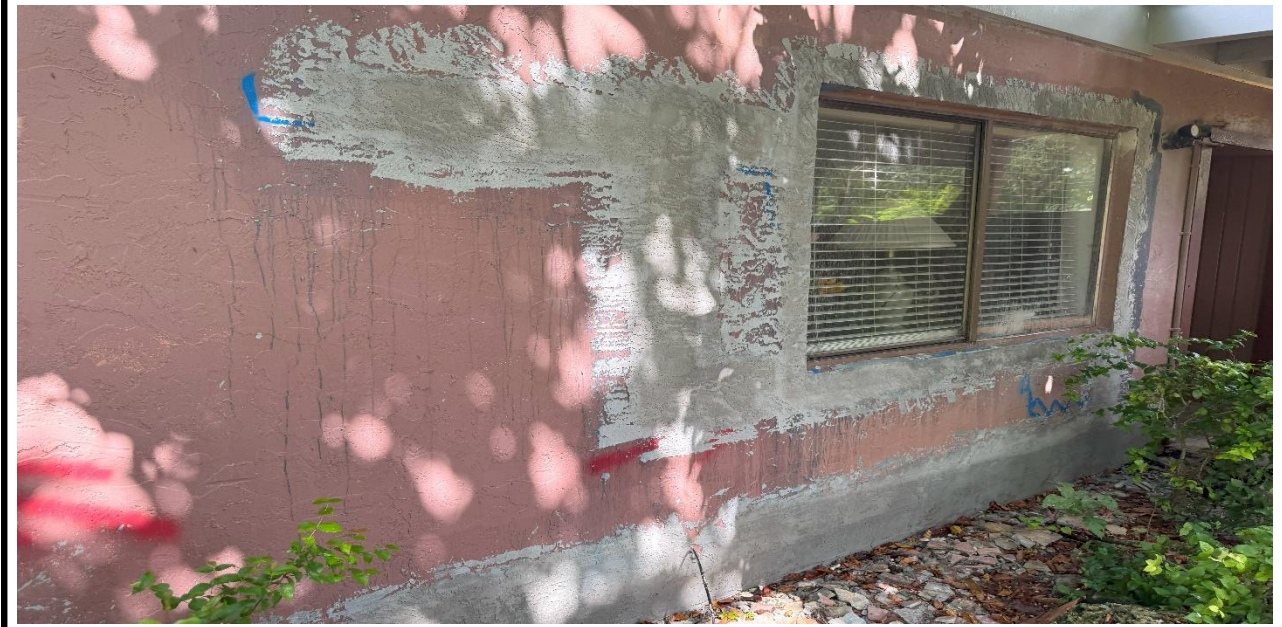
3 – Ongoing, Application of the new stucco at the exterior walls, BLDG 04 .
