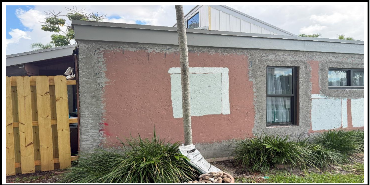
8 – Ongoing, Application of the new stucco at the exterior walls, BLDG 06 .
