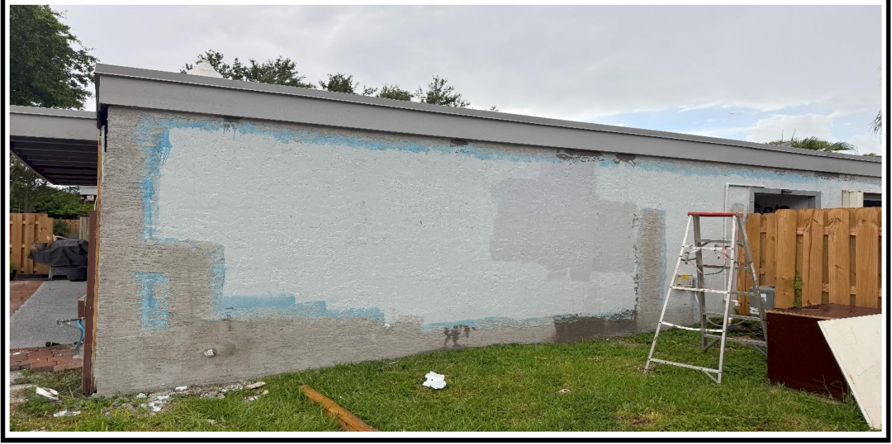
13 – Ongoing, Application of the new stucco at the exterior walls, BLDG 13 .
