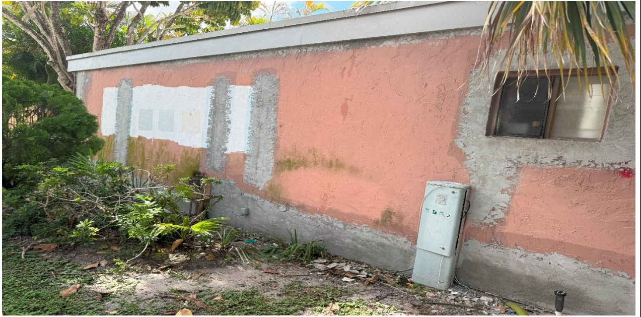
7 – Ongoing, Application of the new stucco at the exterior walls, BLDG 06 .
