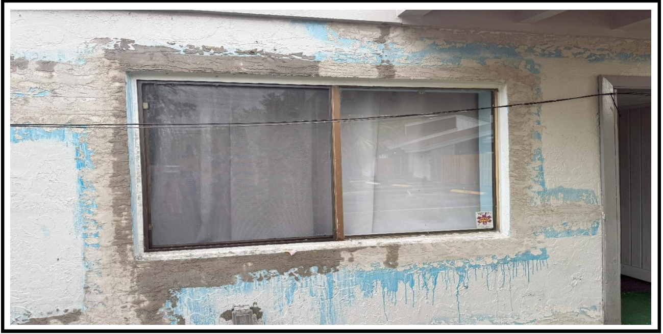
17 – Ongoing, Application of the new stucco at the exterior walls, BLDG 08 .
