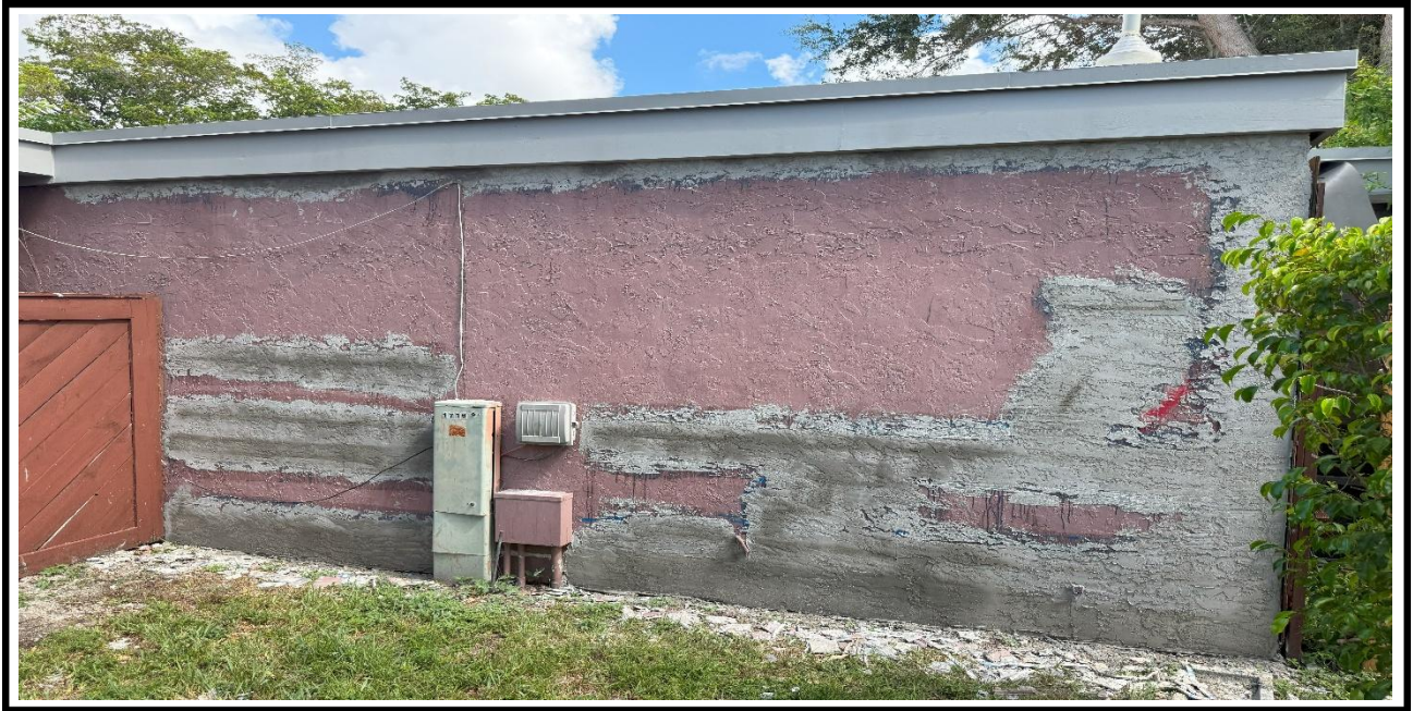
6 – Ongoing, Application of the new stucco at the exterior walls, BLDG 05 .
