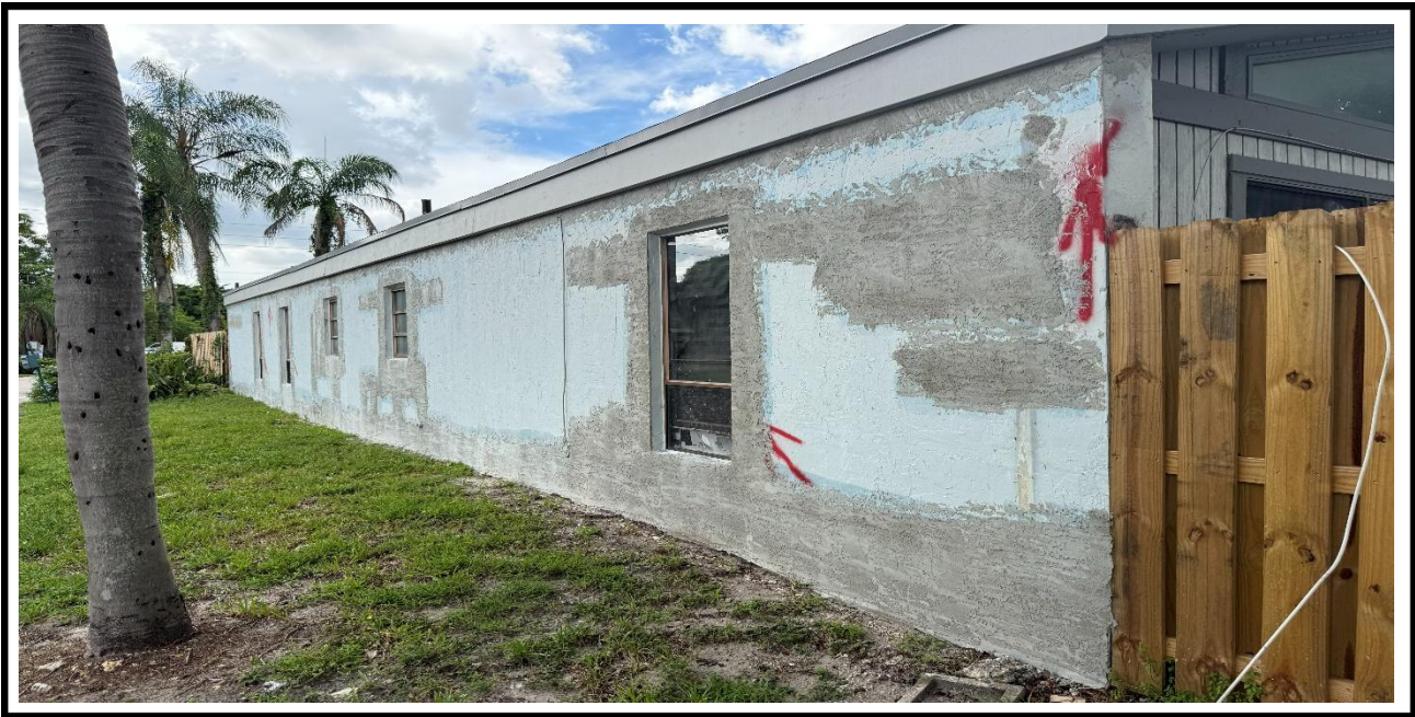
3 – Ongoing, Application of the new stucco at the exterior walls.
