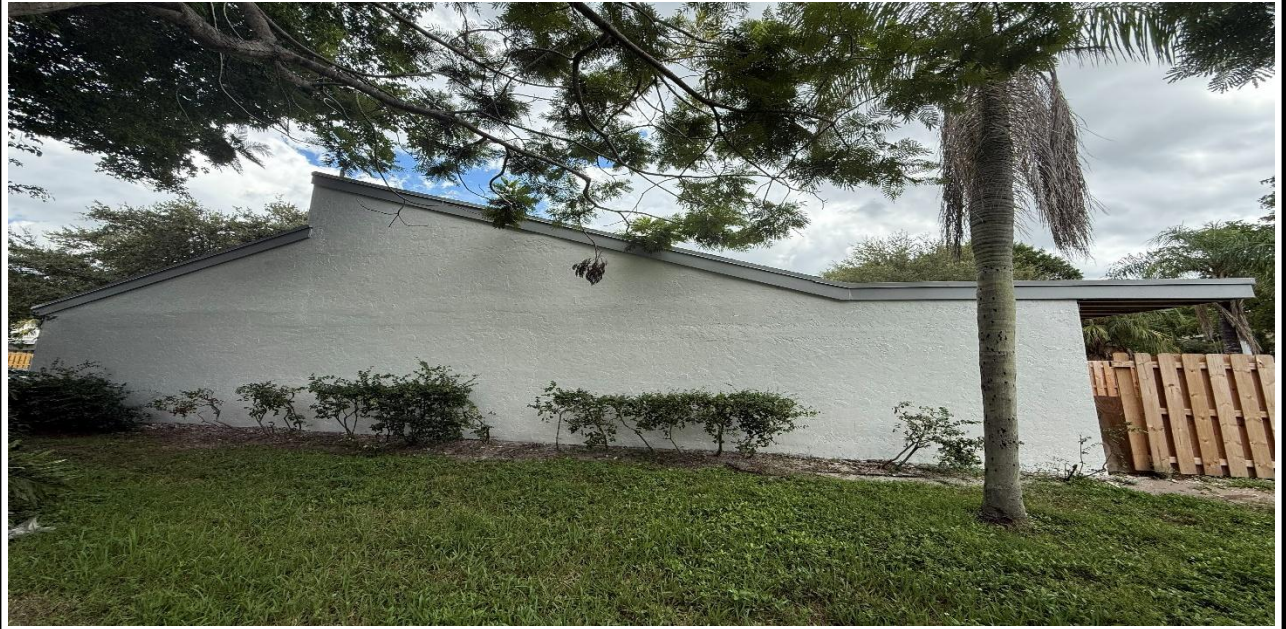
13 – Ongoing, Application of the new Paint at the exterior walls.
