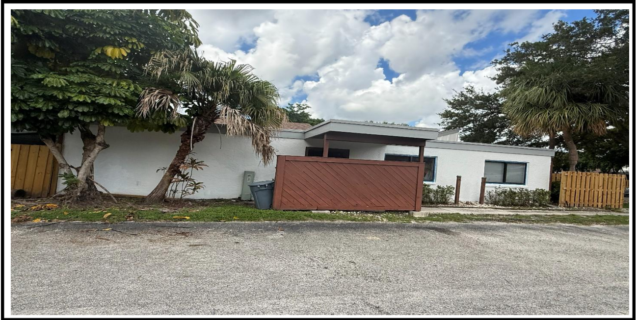
12 – Ongoing, Application of the new Paint at the exterior walls.
