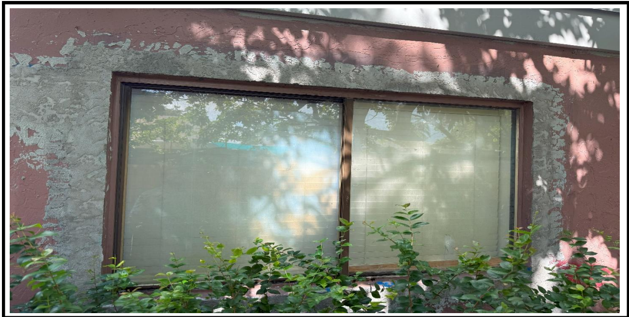
4 – Ongoing, Application of the new stucco at the exterior walls.
