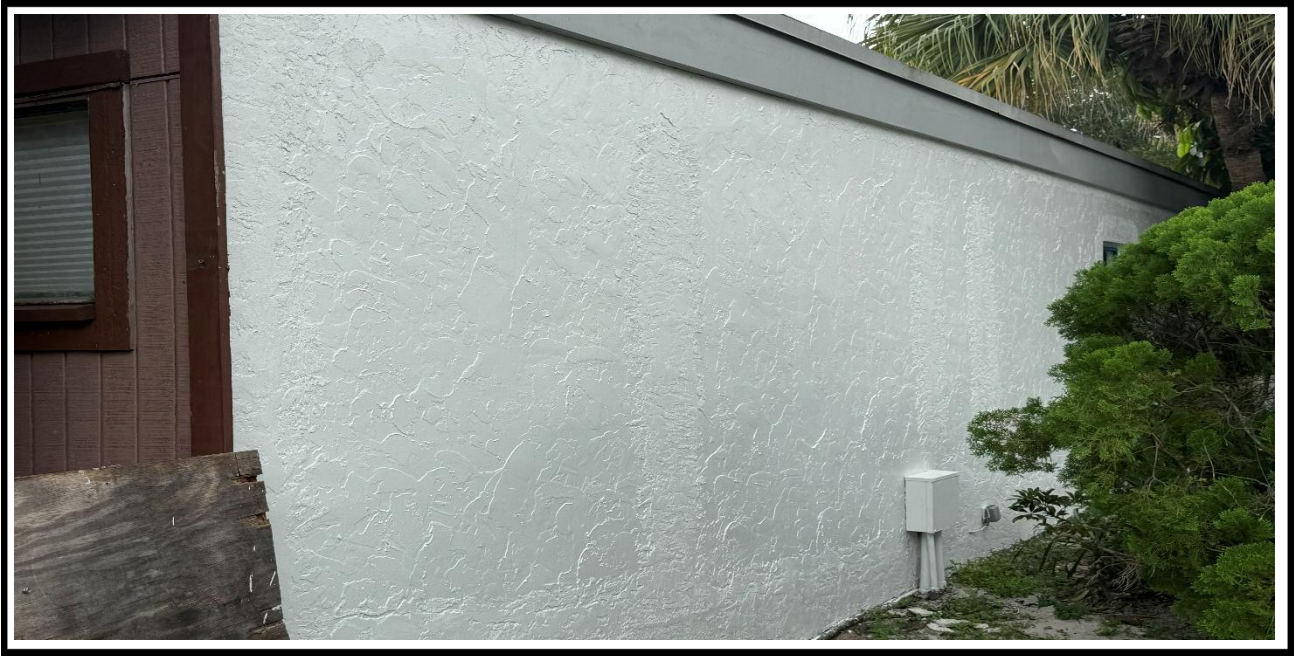
9 – Ongoing, Application of the new Paint at the exterior walls.
