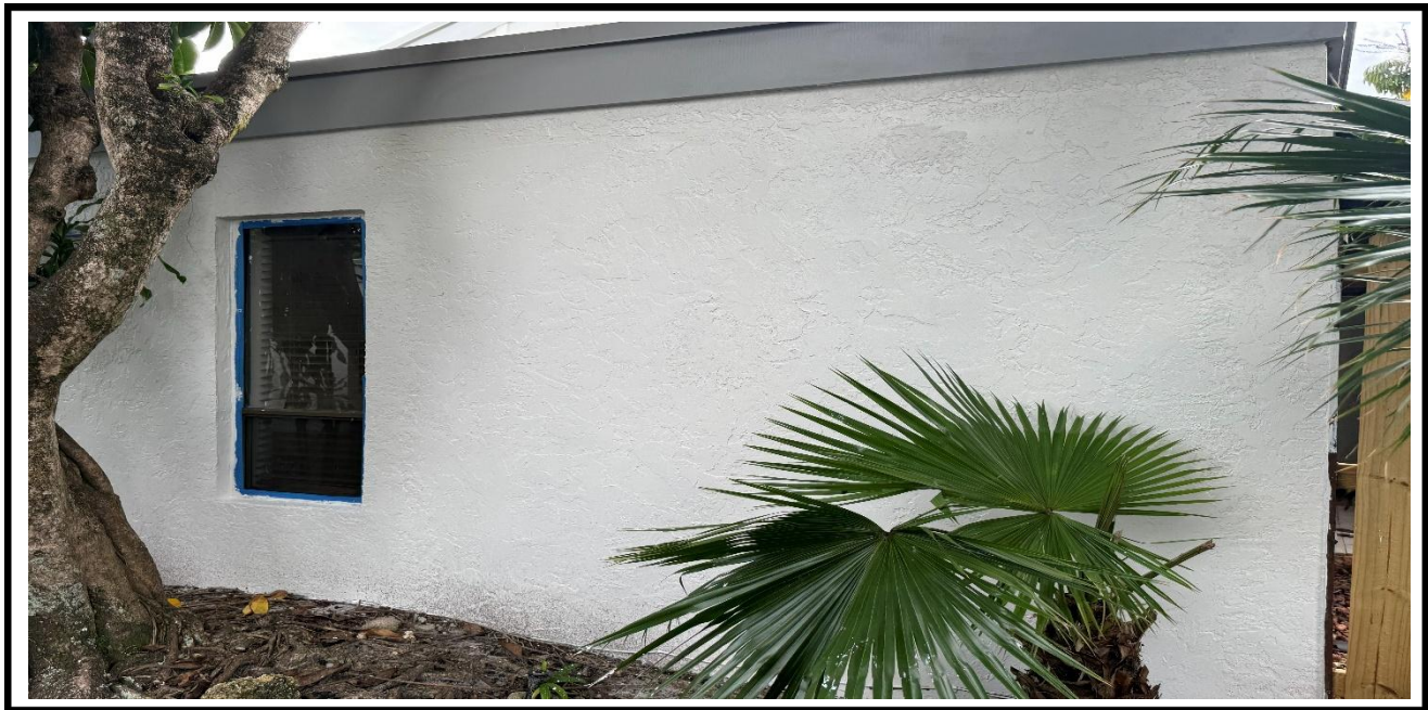
2 – Ongoing, Application of the new Paint at the exterior walls.
