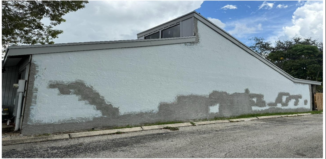
5 – Ongoing, Application of the new stucco at the exterior walls.
