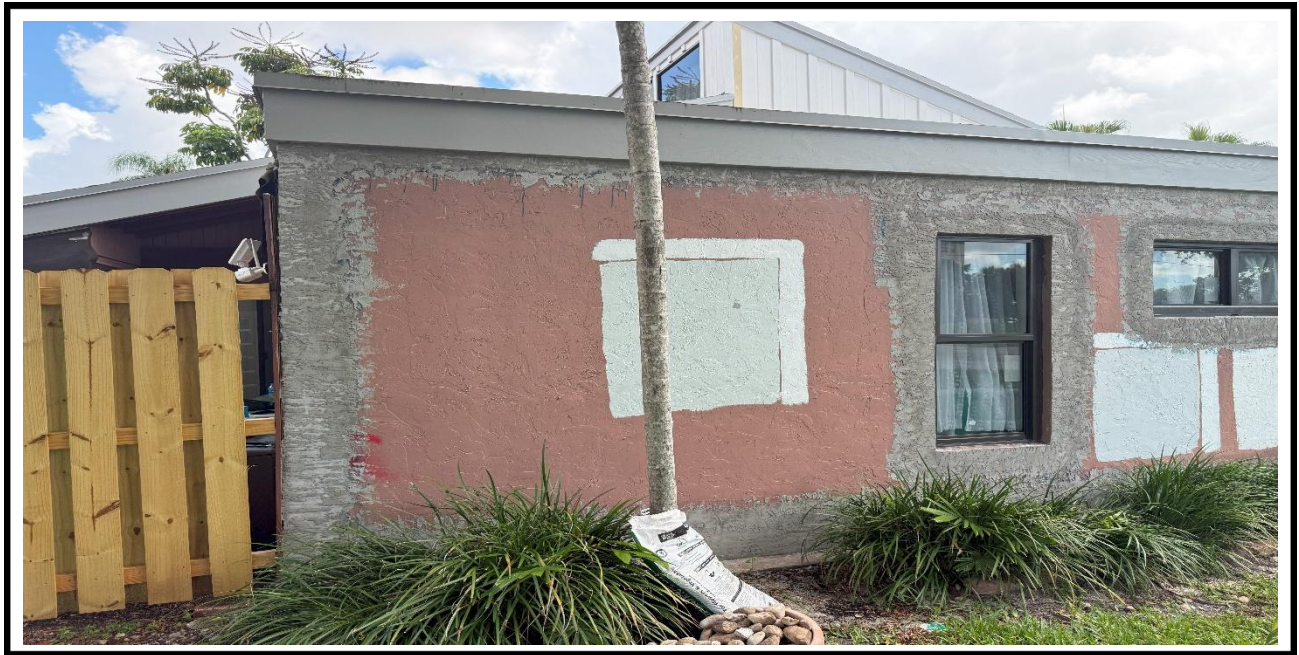
8 – Ongoing, Application of the new stucco at the exterior walls.
