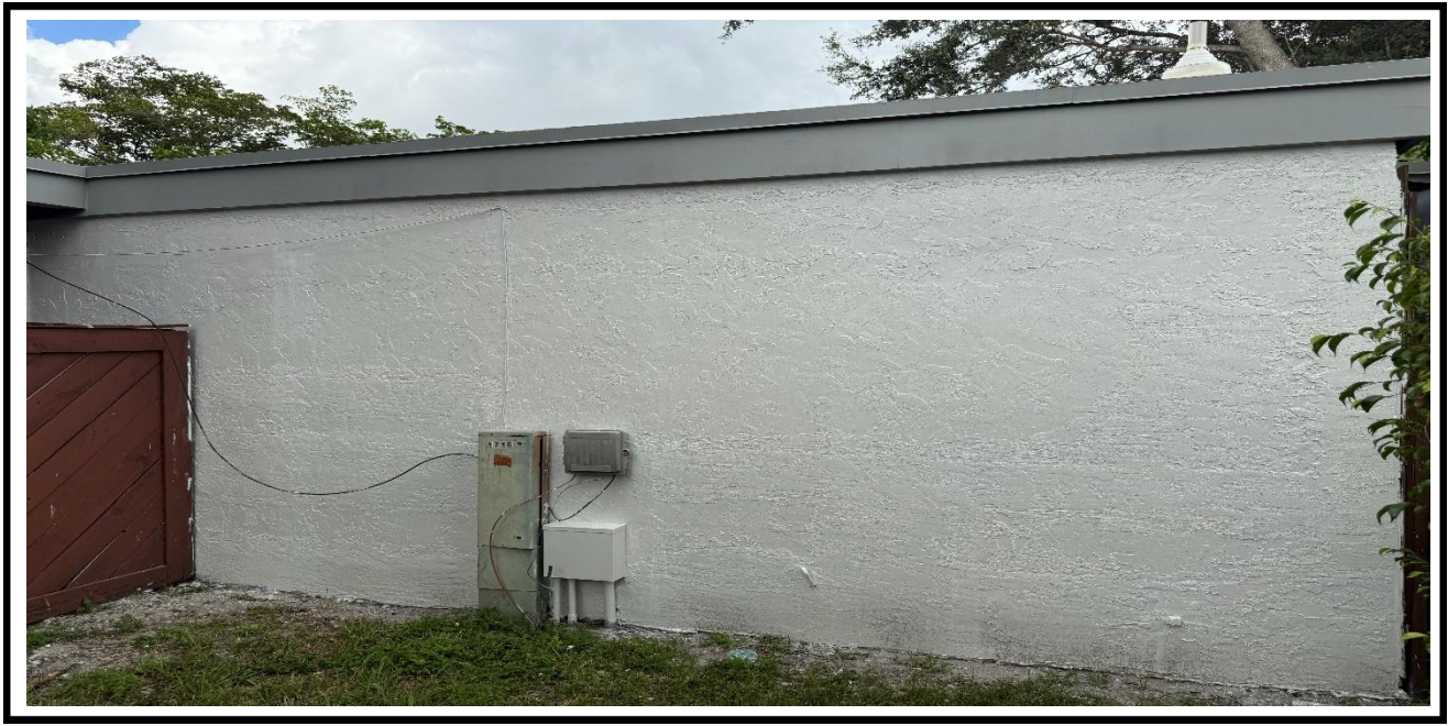
1 – Ongoing, Application of the new Paint at the exterior walls.
