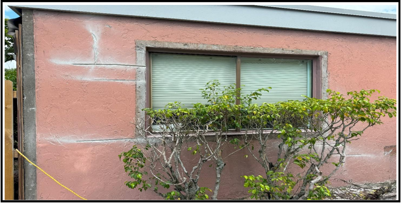
11 – Ongoing, Application of the new stucco at the exterior walls and chipping of the old stucco.
