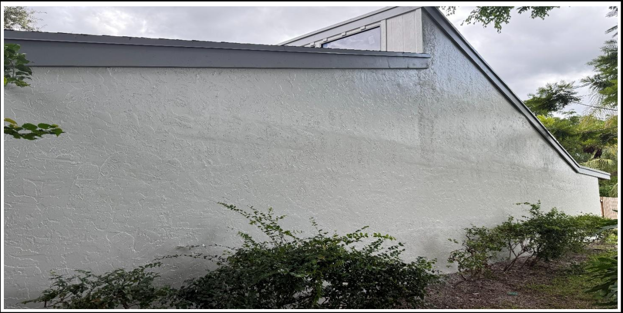
14 – Ongoing, Application of the new Paint at the exterior walls.
