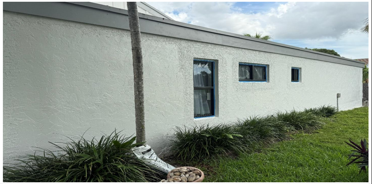
6 – Ongoing, Application of the new Paint at the exterior walls.
