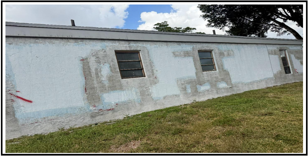
7 – Ongoing, Application of the new stucco at the exterior walls.
