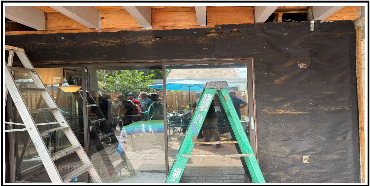
6 – Ongoing, Removal of the old Hardie board at the exterior walls.
