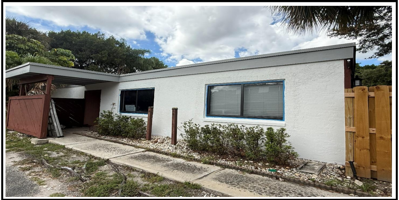
10 – Ongoing, Application of the new Paint at the exterior walls.
