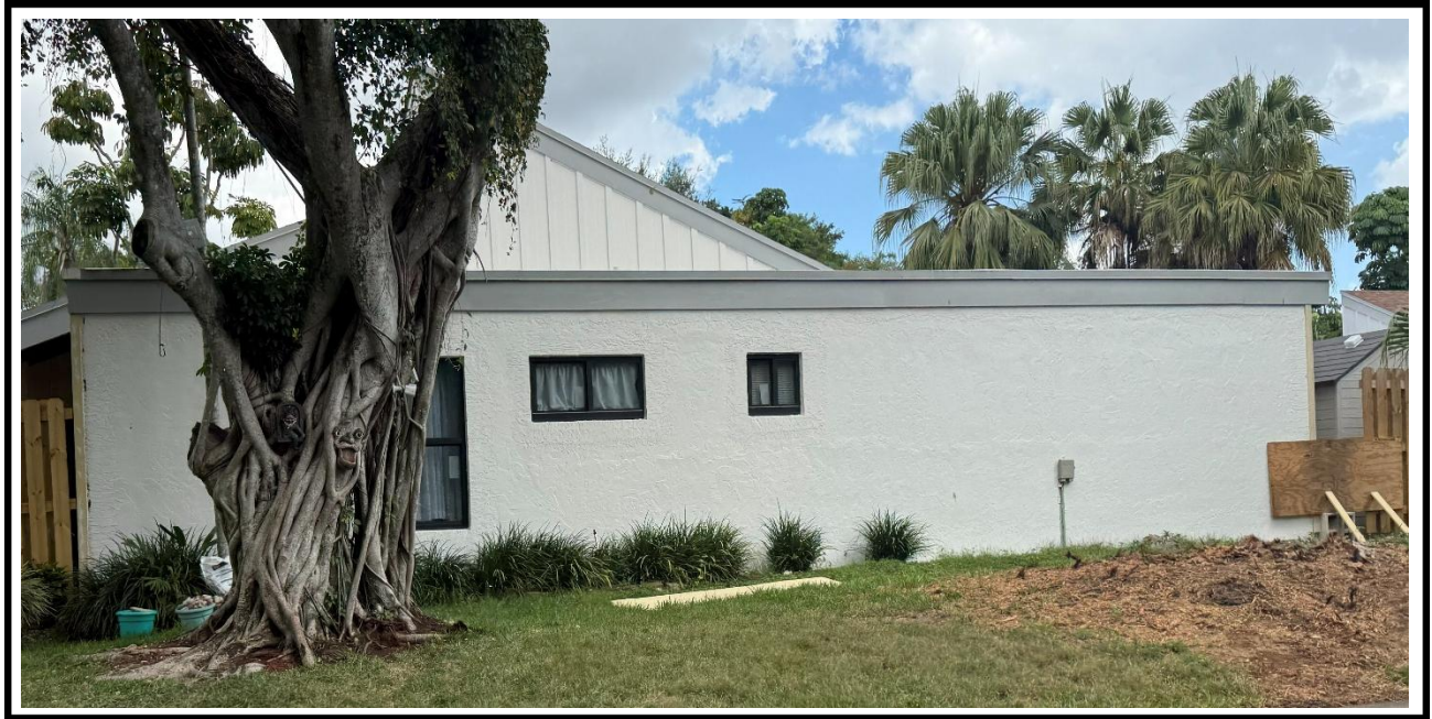
8 – Ongoing, Application of the new Paint at the exterior walls.
