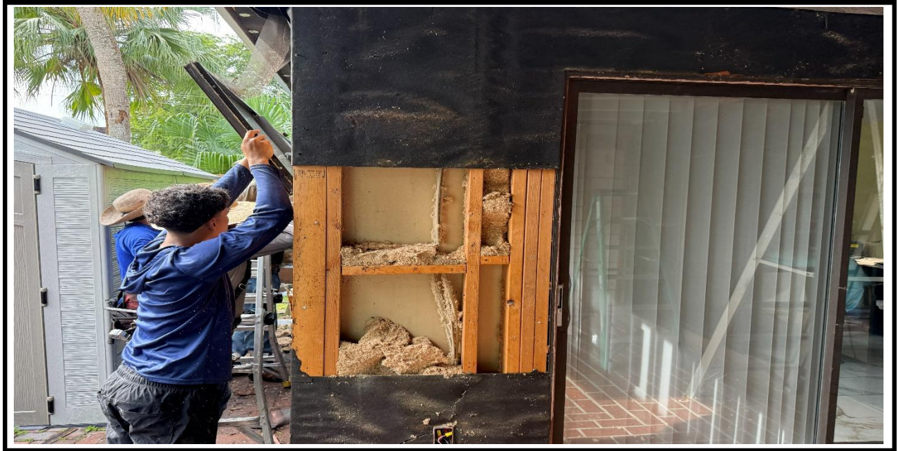
4 – Ongoing, Removal of the old Hardie board at the exterior walls.
