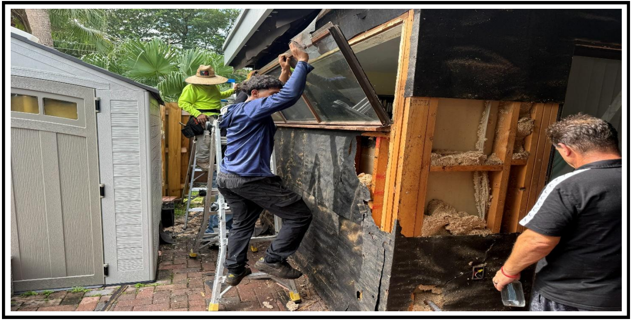
5 – Ongoing, Removal of the old Hardie board at the exterior walls.
