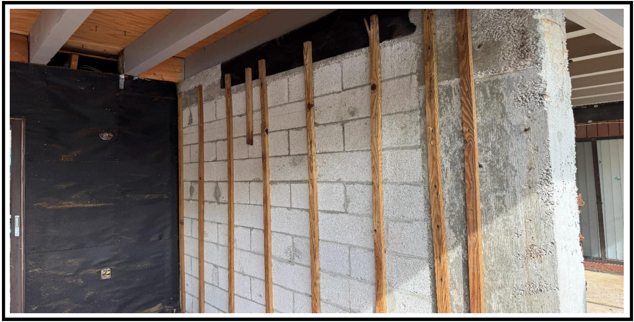
3 – Ongoing, Removal of the old Hardie board at the exterior walls.
