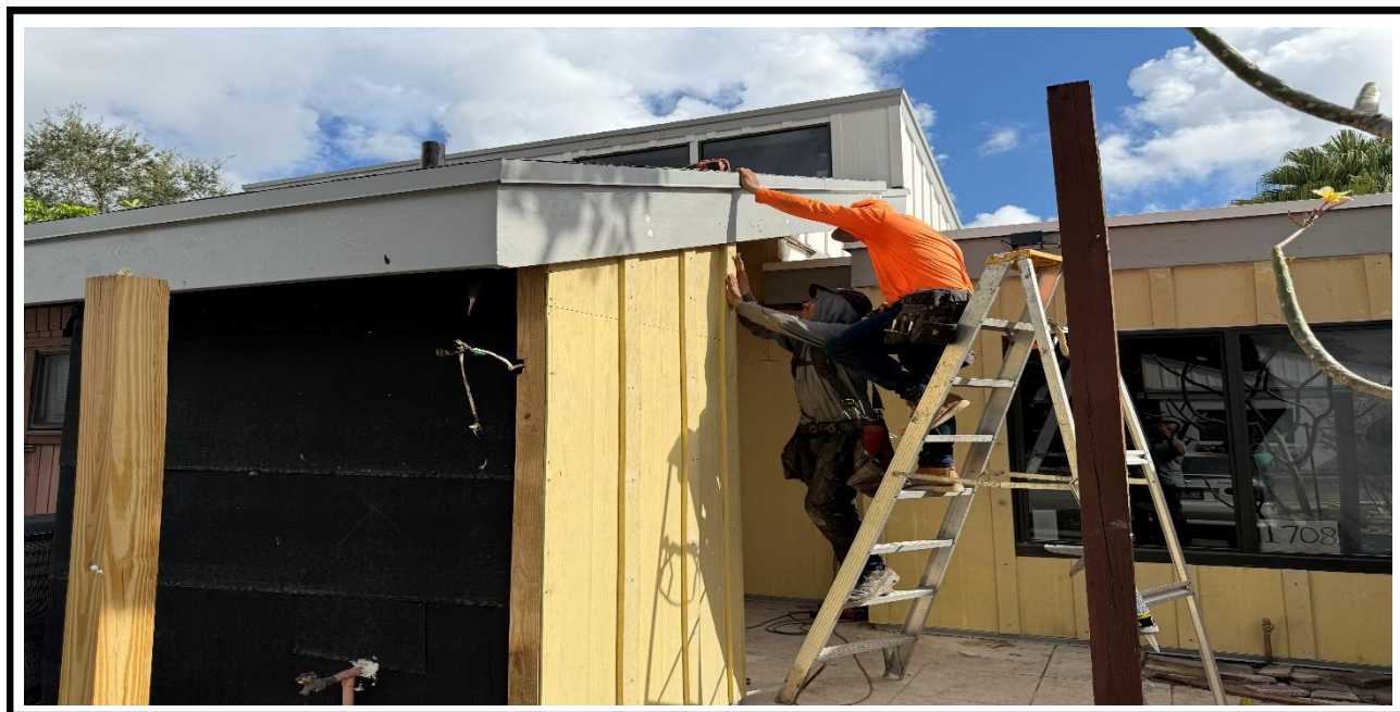
10 – Ongoing, Installation of the Hardie Board at the exterior walls, BLDDG 6.
