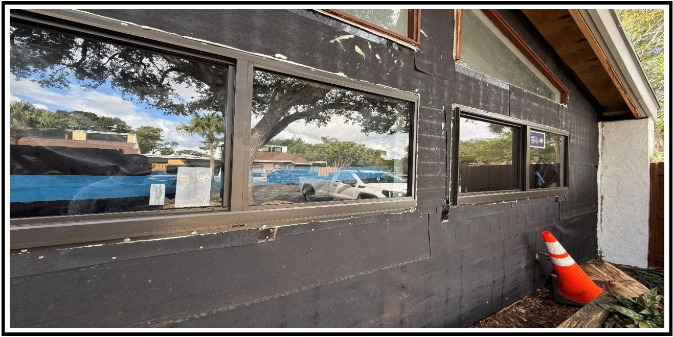
1 – Ongoing, Installation of the black paper vapor barrier over the Plywood at the exterior walls, BLDG 1
