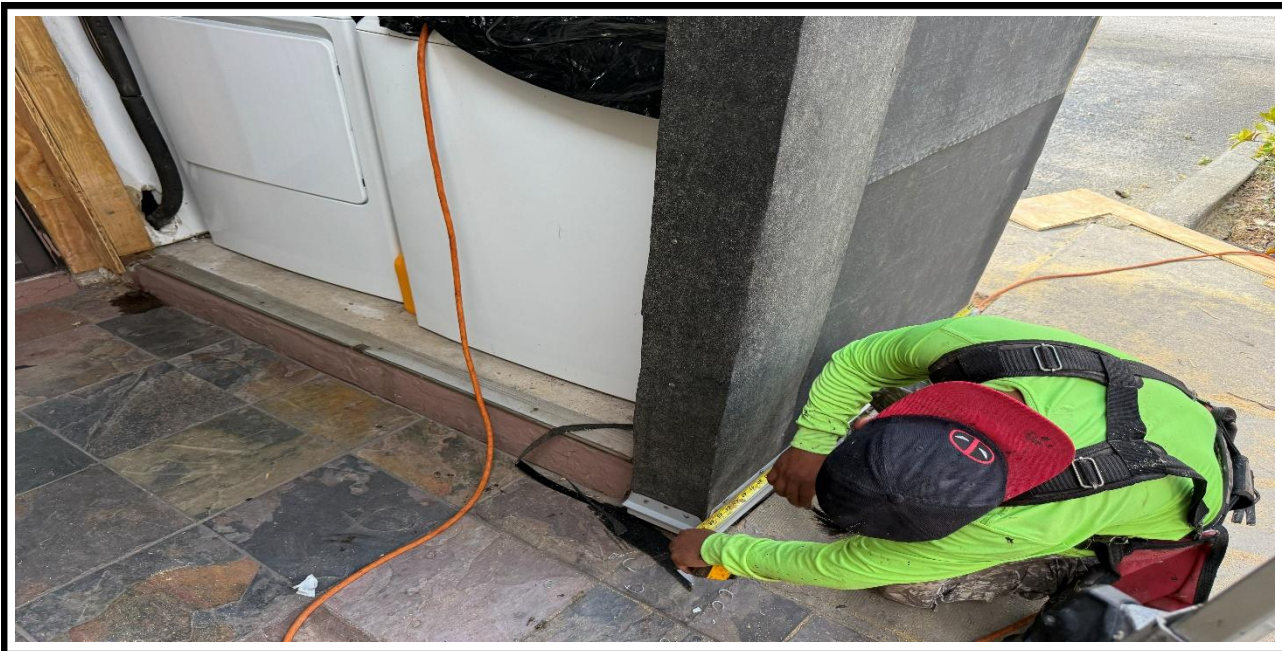
9 – Ongoing, Installation of the black paper vapor barrier over the Plywood at the exterior walls, BLDG 6.
