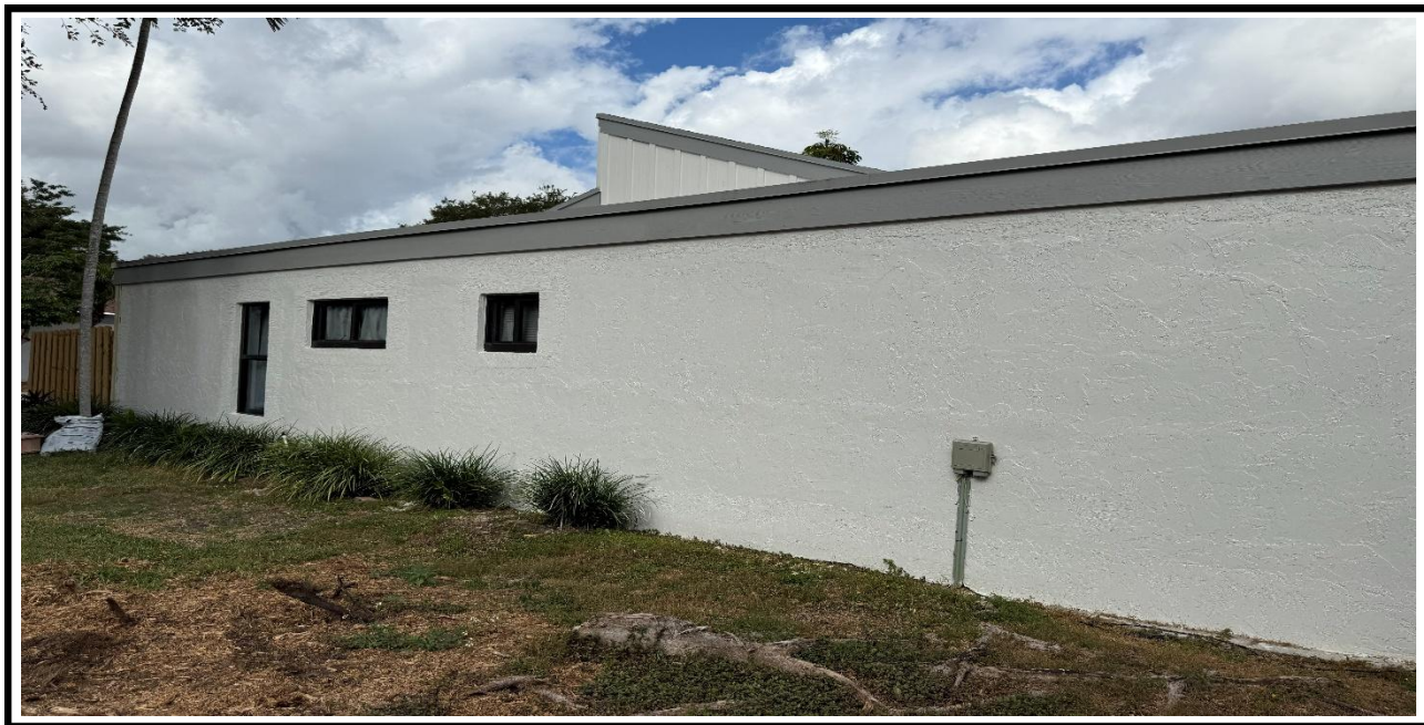
8 – Ongoing, Application of the new Paint at the exterior walls, BLDG 6.
