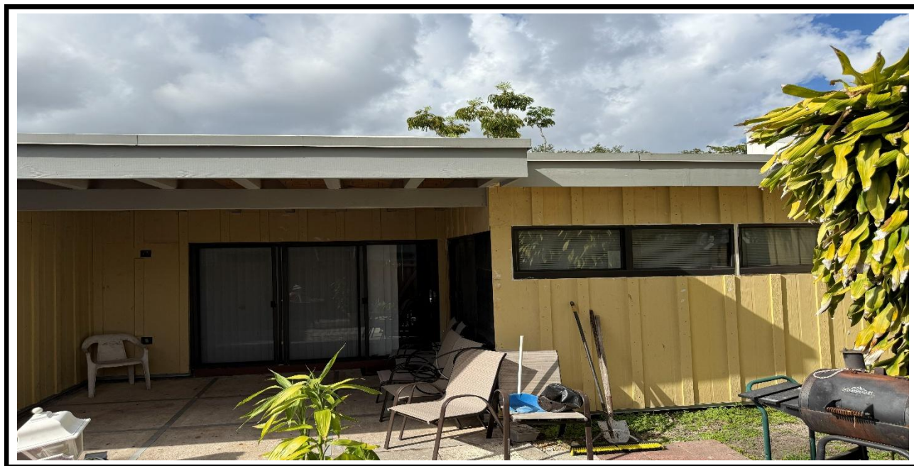
12 – Ongoing, Installation of the Hardie Board at the exterior walls, BLDG 6.
