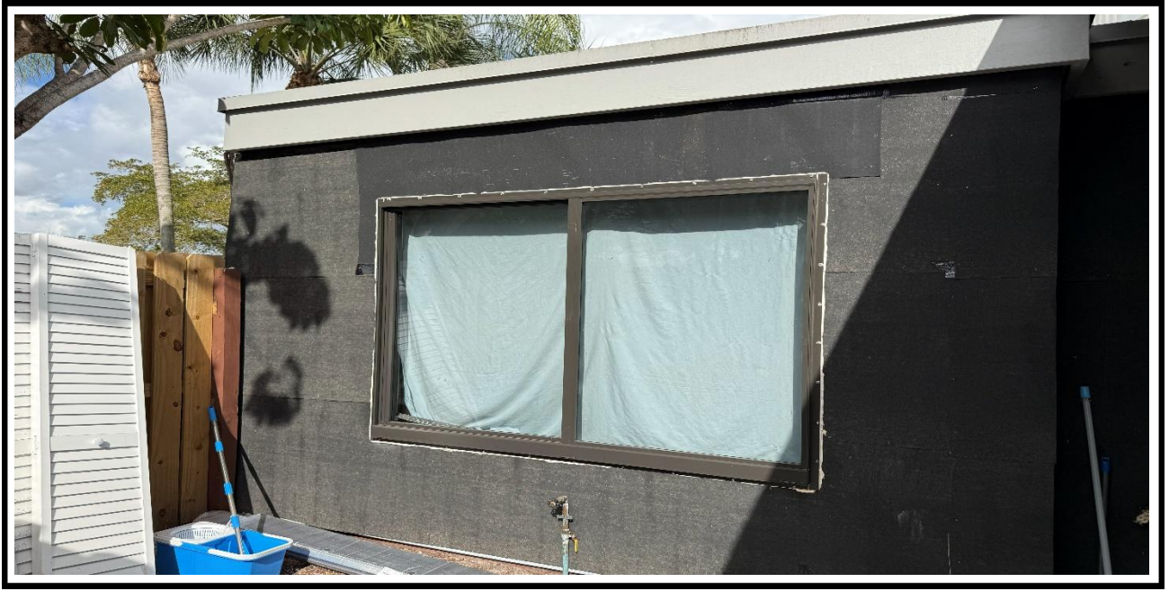
5 – Ongoing, Installation of the black paper vapor barrier over the Plywood at the exterior walls, BLDG 2.
