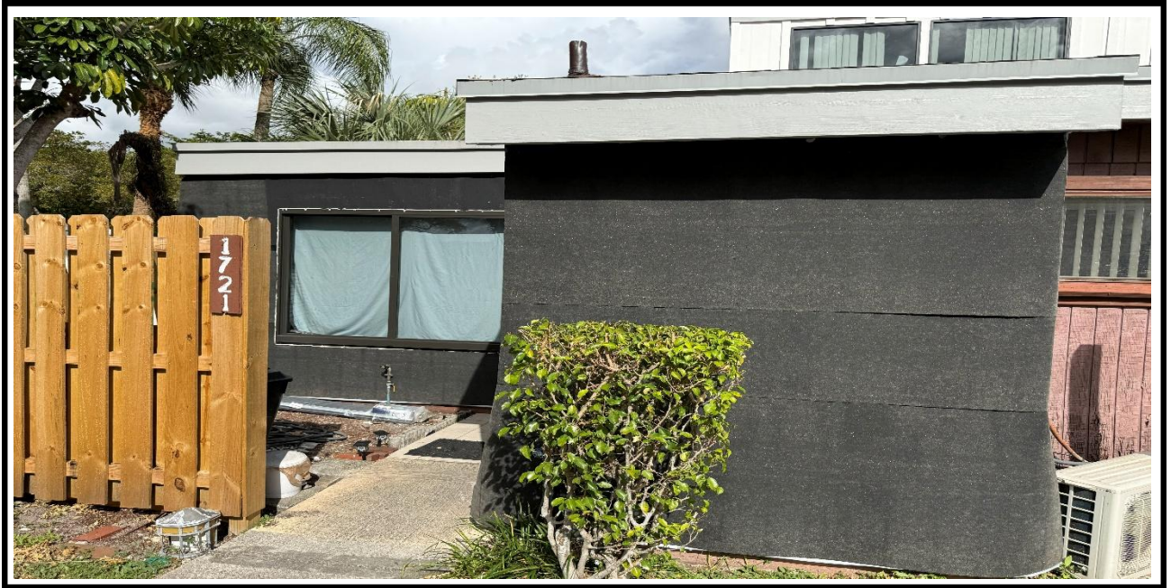
6 – Ongoing, Installation of the black paper vapor barrier over the Plywood at the exterior walls, BLDG 2.
