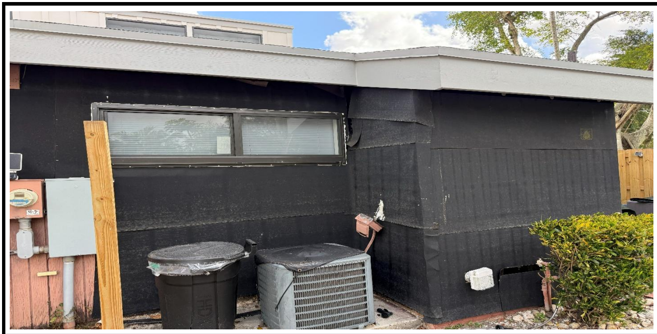
7 – Ongoing, Installation of the black paper vapor barrier over the Plywood at the exterior walls, BLDG 6.
