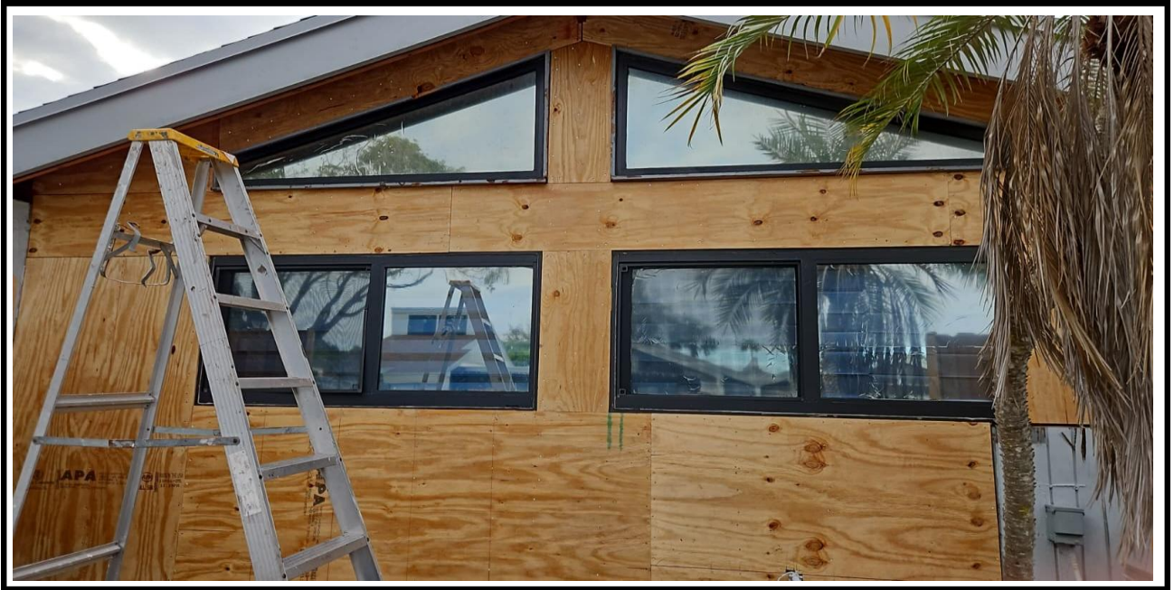
8 – Ongoing, Install of the plywood on exterior walls, BLDG 6.
