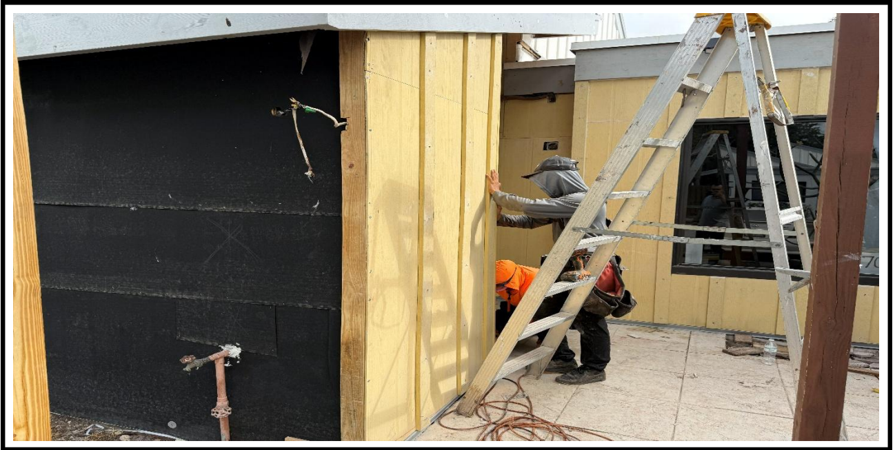
11 – Ongoing, Installation of the Hardie Board at the exterior walls, BLDG 6.
