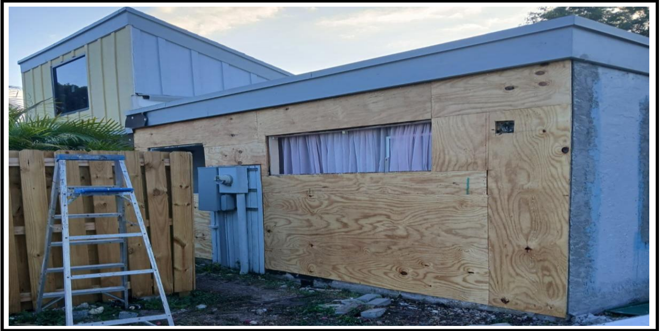
10 – Ongoing, Installation of the Plywood at the exterior walls, BLDDG 6.
