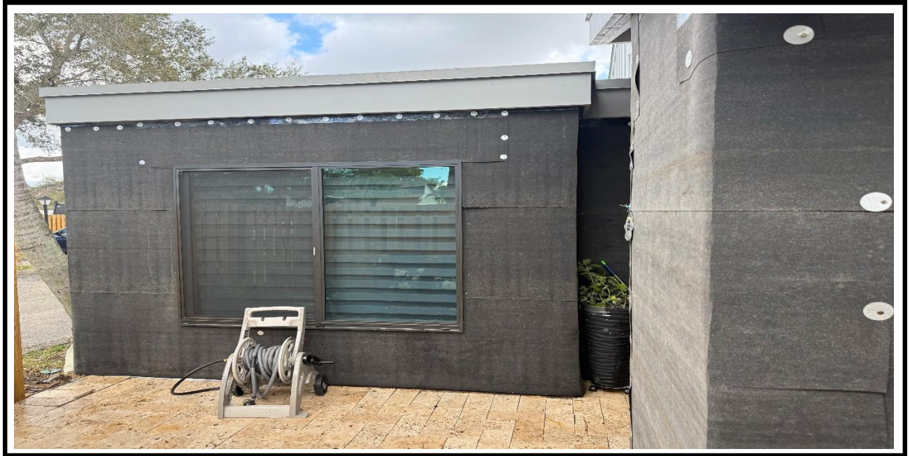
4 – Ongoing, Removal of the old Hardie board at the exterior walls, BLDG 2
