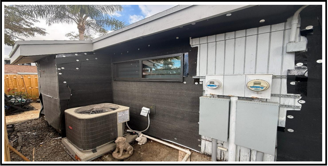
3 – Ongoing, Installation of the black paper vapor barrier over the Plywood at the exterior walls, BLDG 1
