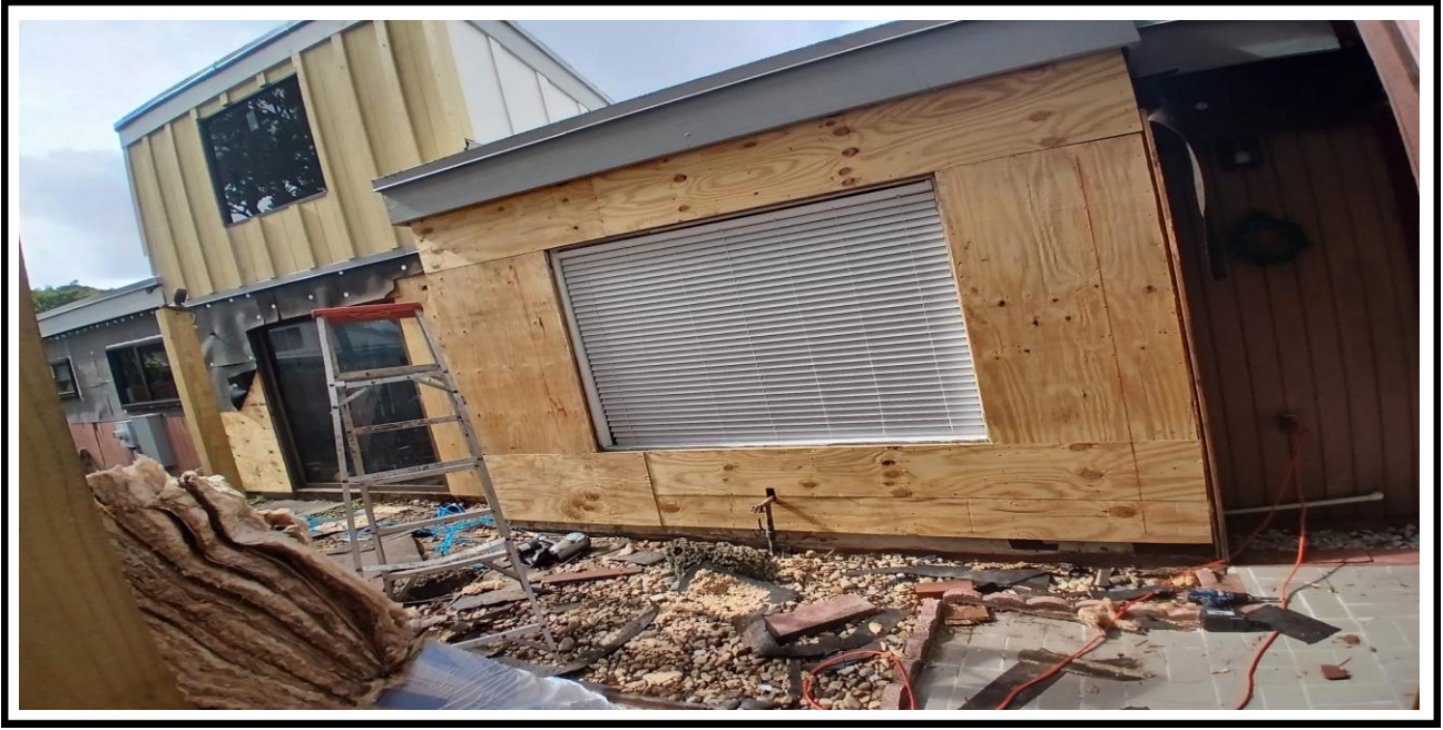
9 – Ongoing, Installation of the Plywood at the exterior walls, BLDG 6.
