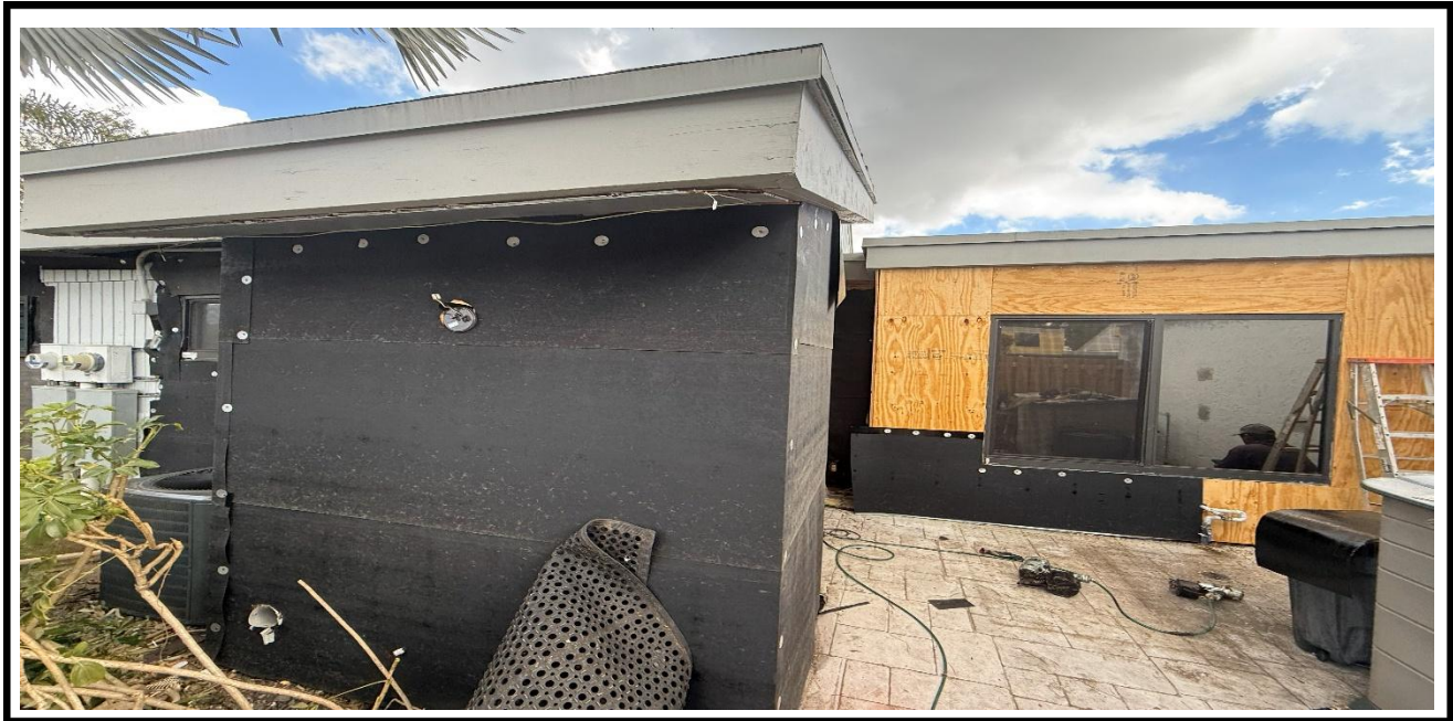
2 – Ongoing, Installation of the black paper vapor barrier over the Plywood at the exterior walls, BLDG 1
