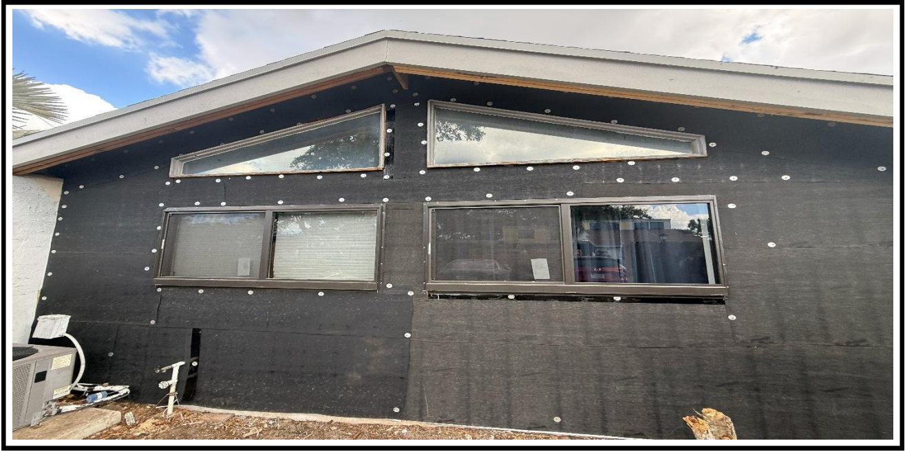
1 – Ongoing, Installation of the black paper vapor barrier over the Plywood at the exterior walls, BLDG 11
