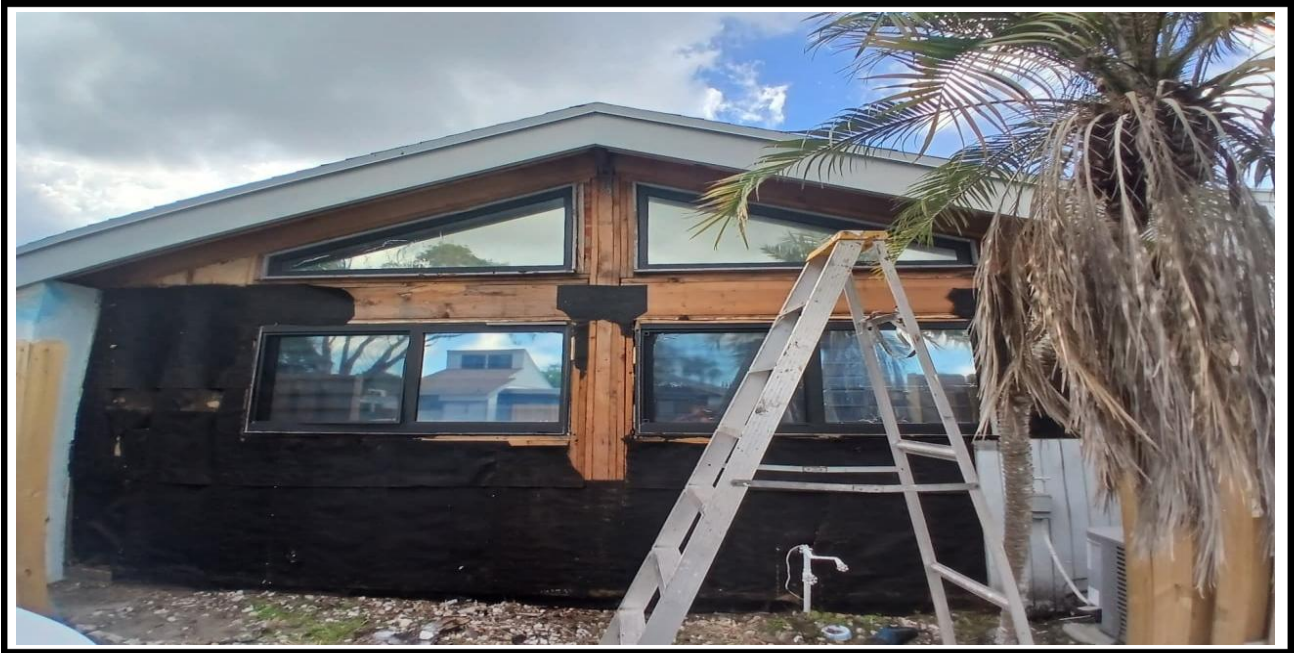
7 – Ongoing, Removal of the black paper vapor barrier over the Plywood at the exterior walls, BLDG 6.
