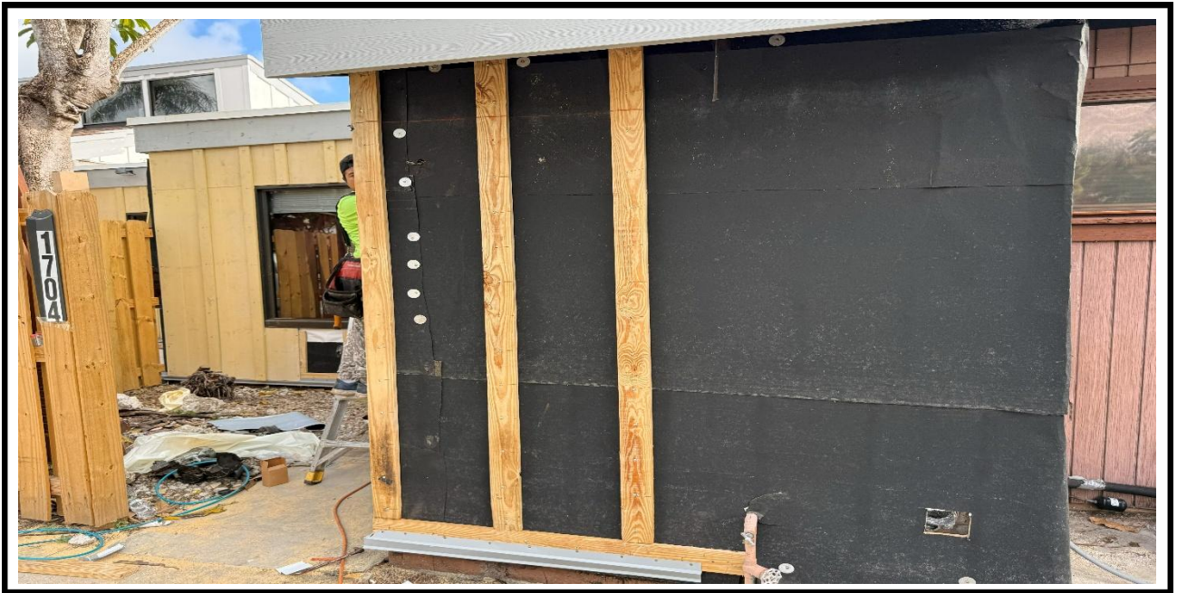
12 – Ongoing, Installation of the Hardie Board at the exterior walls, BLDG 6.
